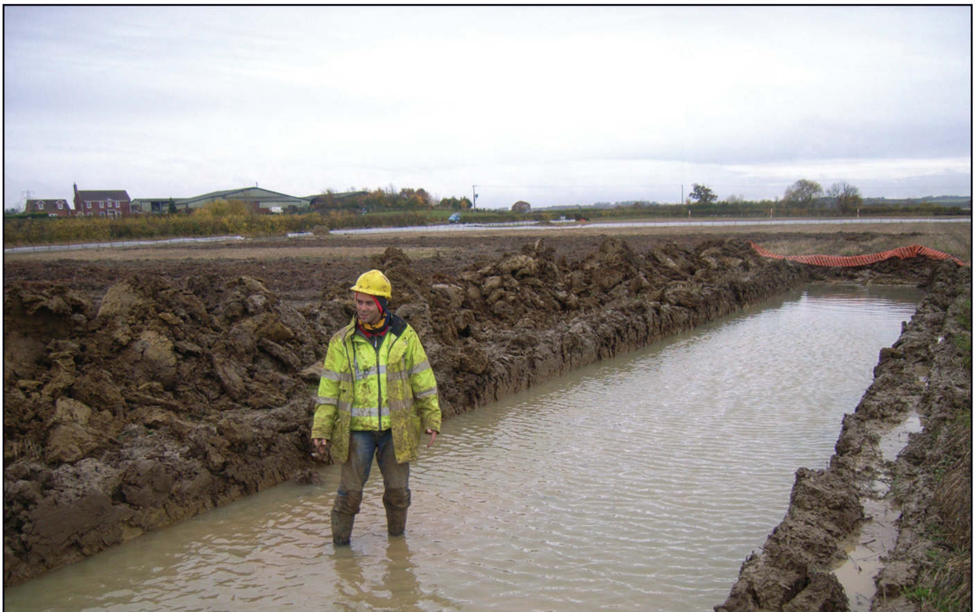
Plate 2: Flooding in Trench 58
