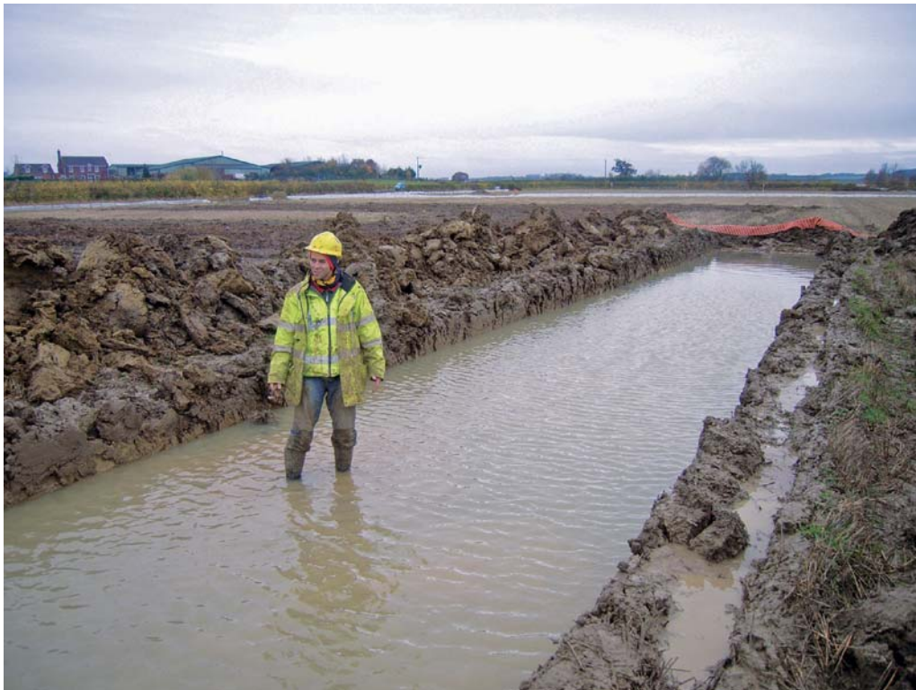
Fig. 1.6 Flooding in Evaluation Trench 58
