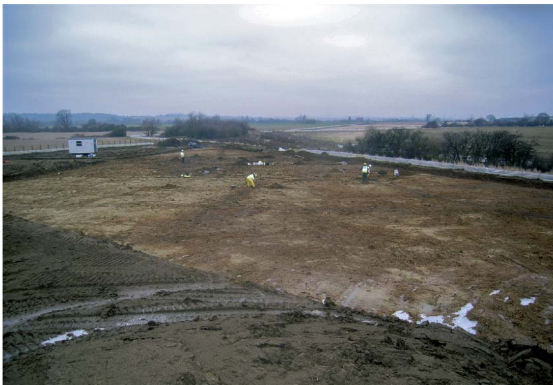
Fig. 2.34 General view of Site 3 from the south-west
