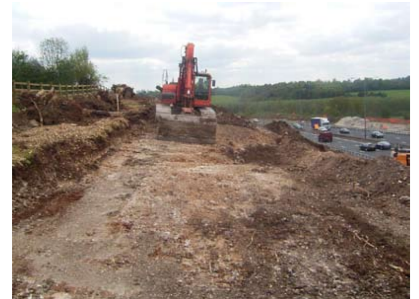
Solesbridge Lane to Sarratt Road widening
