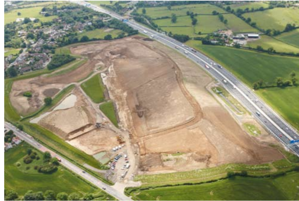
Improvements at South Mimms
