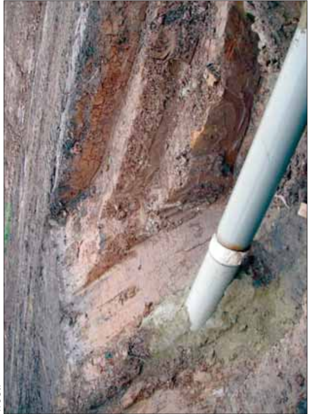
Plate 19: Stepped trench edge for new gas Pipe in central part of Area 4, view from south.
