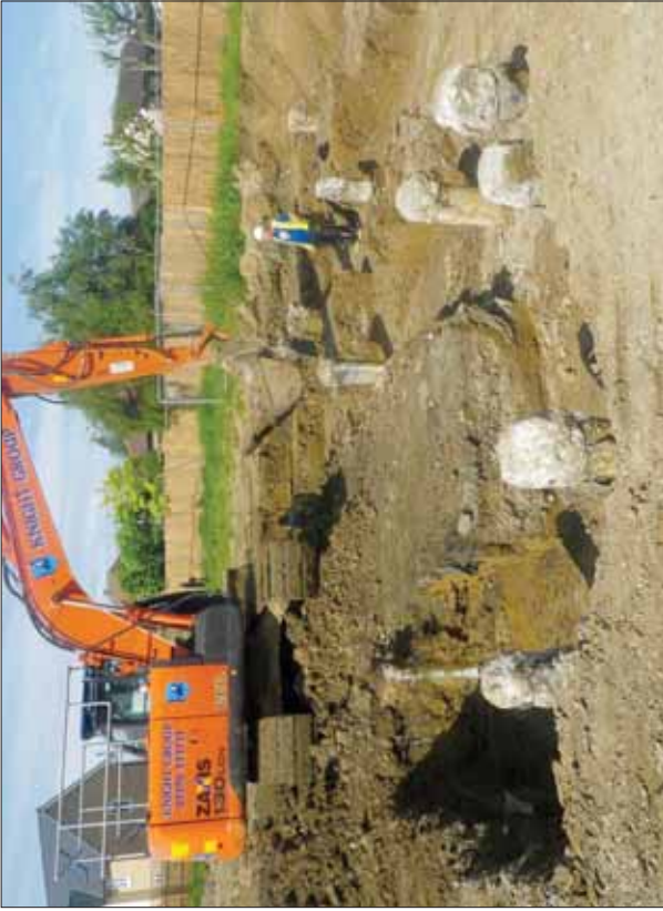
Plate 6: Digging out piles in plot 100, Area 2, view from east.
