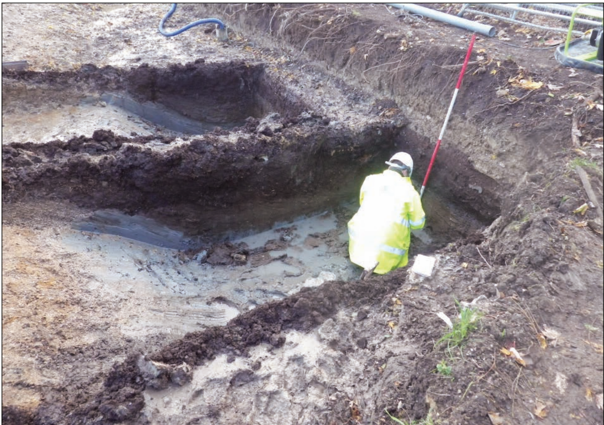
Plate 6: Period 2: excavation of Covens Moat, looking south
