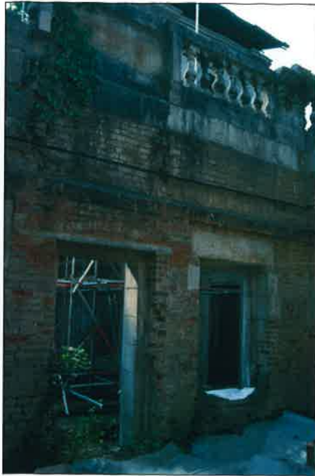
Plate 48: Interior wall of lodge, the west wall containing the front door (OA 2004, F1/16)
