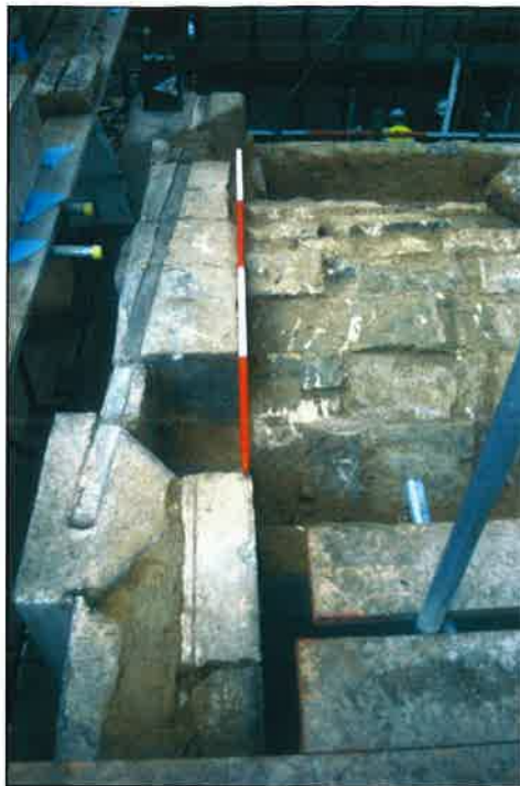
Plate 39: The angled bar-chain over the western postern arch (OA 2004, F10/12)
