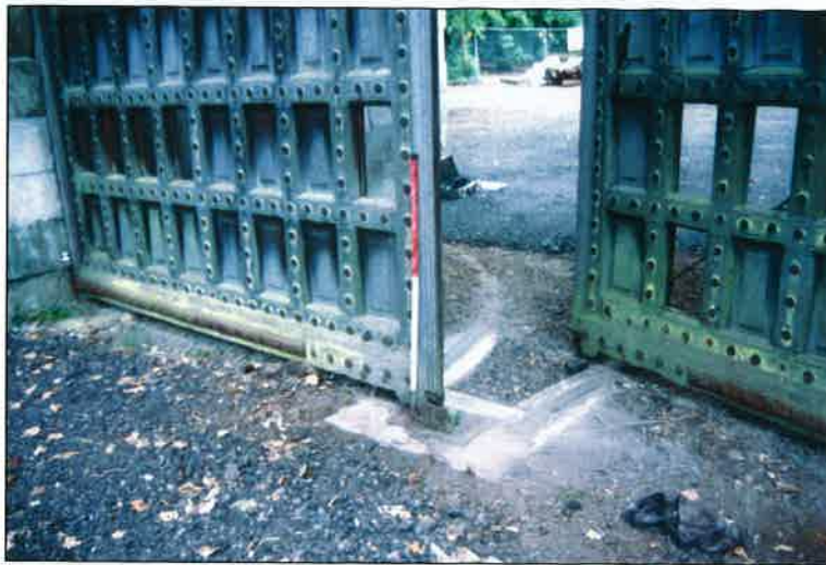
Plate 5: Detail of roller mechanism for gates (OA 2004, F4/31)
