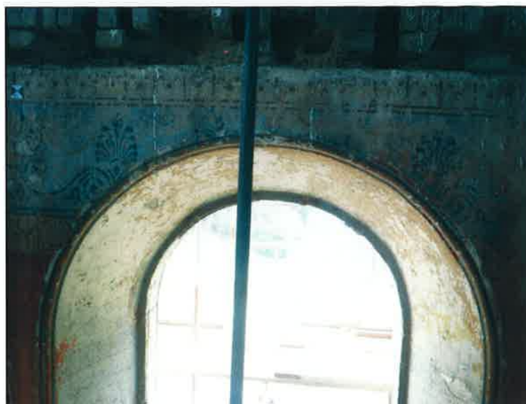
Plate 12: Painted plaster detail around the window head on south wall (Ben Jeffs 2004)
