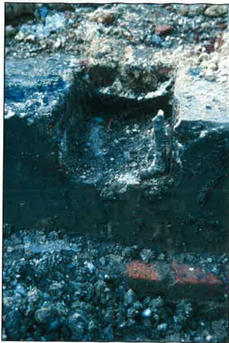
Plate 54: Test pit 2, remains of iron grill in base of the lodge's southern wall (OA 2004, F13/8)
