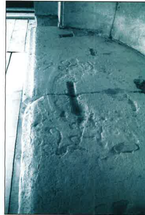
Plate 24: Niche base with curvy numbers, possibly from the first dismantling (OA 2004, F6/20)
