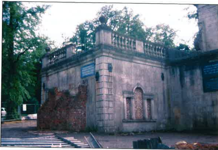
Plate 43: The rear of the lodge with brick buttresses replacing the original annexe (OA 2004, F5/17)
