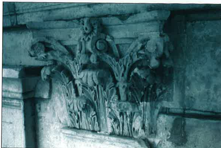
Plate 9: Detail of middle capital on the north facade, note rectangular block replacements (OA 2004, F6/28)
