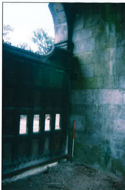
Plate 6: Detail of gate pintels and hangings (OA 2004, F4/32)
