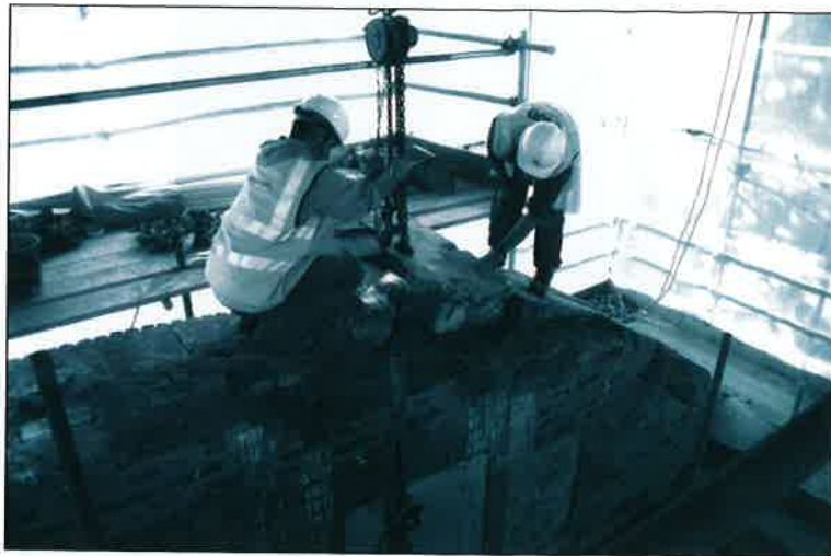
Plate 8: Pediment stone with a socket for the roof purlin being removed by CWO staff (OA 2004, F6/34)
