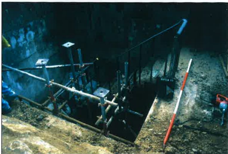
Plate 29: Stair well during dismantling (OA 2004, F10/29)
