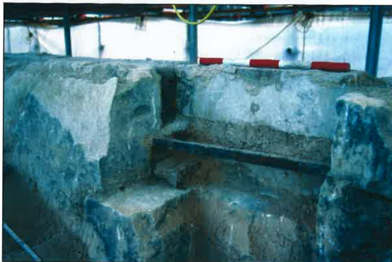
Plate 38: Square, iron tie between pilasters and voussoirs on the south-eastern side of the arch (OA 2004, F9/26)
