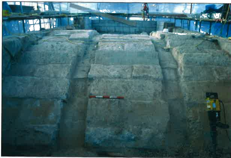
Plate 34: Eastern side of the main arch, note the use of two stones in some places (OA 2004, F9/16)
