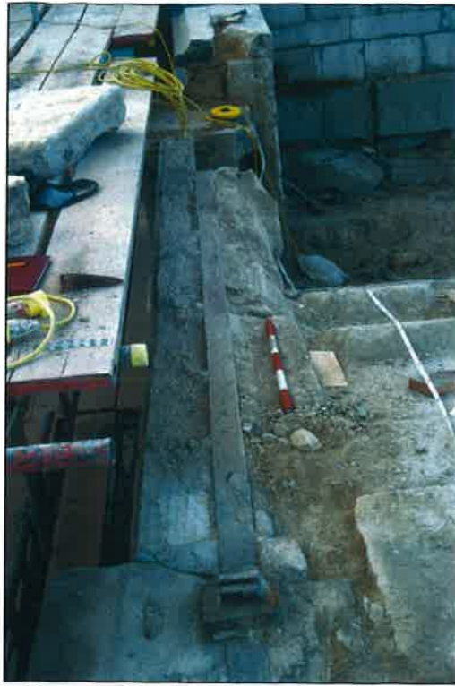
Plate 36: Socket for the bar chain over the south western voussoirs of the central arch (OA 2004, F9/34)
