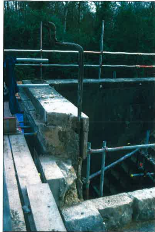
Plate 17: Pipes from radiator built into the wall and descending into the space beneath the stairs (OA 2004, F12/21)
