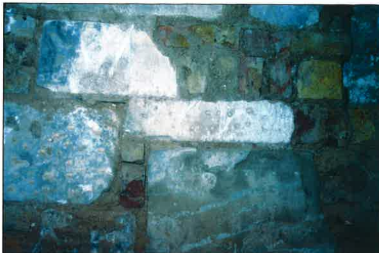
Plate 19: Pecking on stones within the upper room, providing a key for plaster (OA 2004, F3/17)
