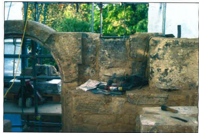
Plate 26: The back of the central window on the south side of the bar (OA 2004, F7/21)
