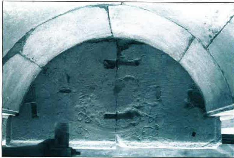
Plate 23: Base stones of niches showing sockets for missing cramps and pintel holes for lifting the stone in place (OA 2004, F6/17)
