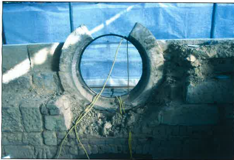
Plate 25: Back of the eastern round window, the upper inner window stones have been removed (OA 2004, F7/9)
