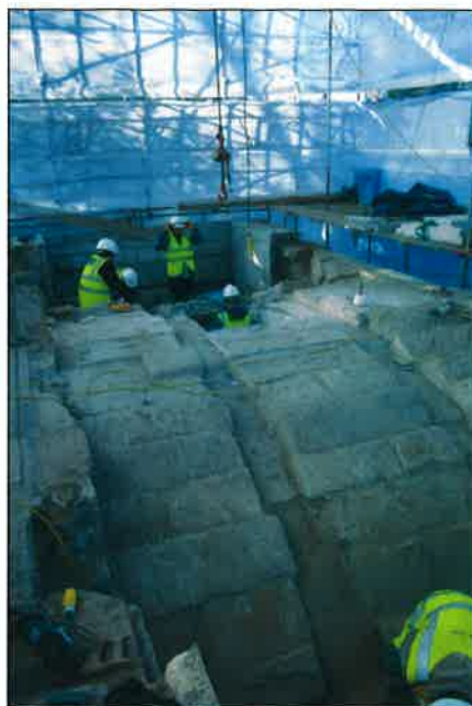
Plate 32: General shot of the dismantling work on the central arch (OA 2004, F9/3)
