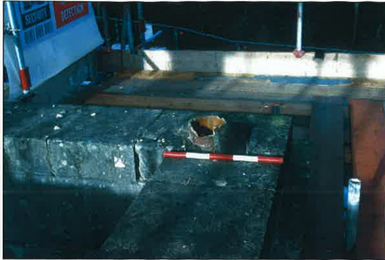
Plate 30: Flu for the boiler within the north east corner of the stair's walls (OA 2004, F11/28)
