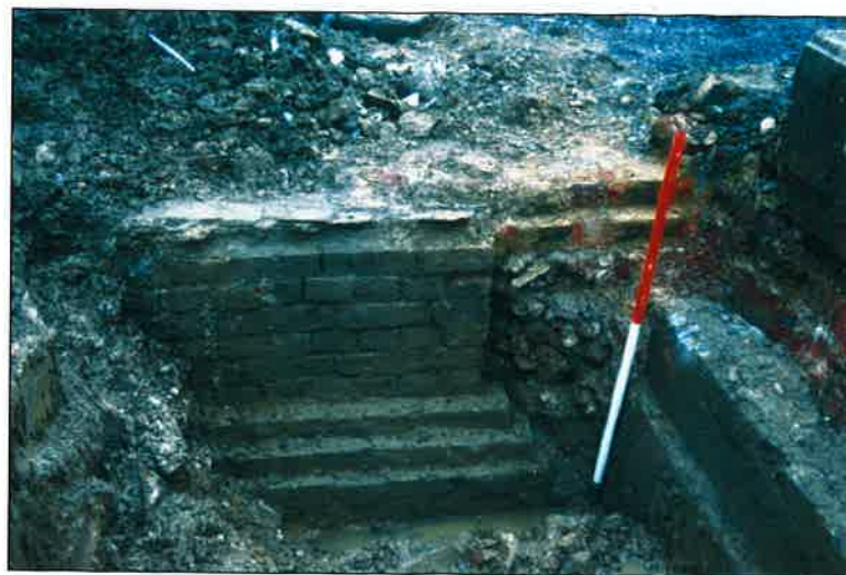
Plate 56: Test pit 3, corner shot showing rubble fill of the lodge's foundations abutting the stepped brick foundation of the bar (OA 2004, F13/22)
