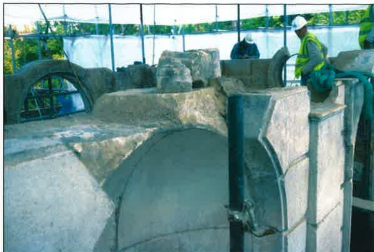
Plate 22: South western niche front with key stone and two voussoirs removed (OA 2004, F7/16)
