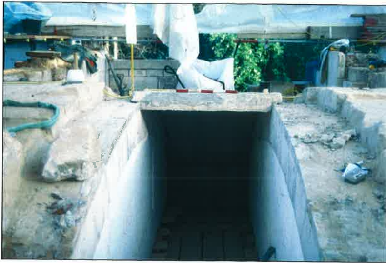
Plate 33: Partially dismantled central arch showing the soffit stones overlapping the ribs (OA 2004, F9/10)
