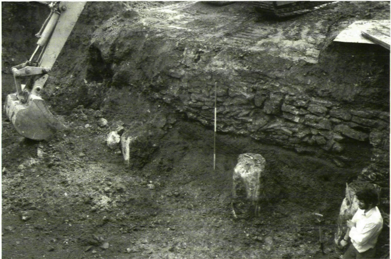
Plate 4.3 24A St Michael's St, the external (N) face of the town wall, seen in the contractors' trench.
