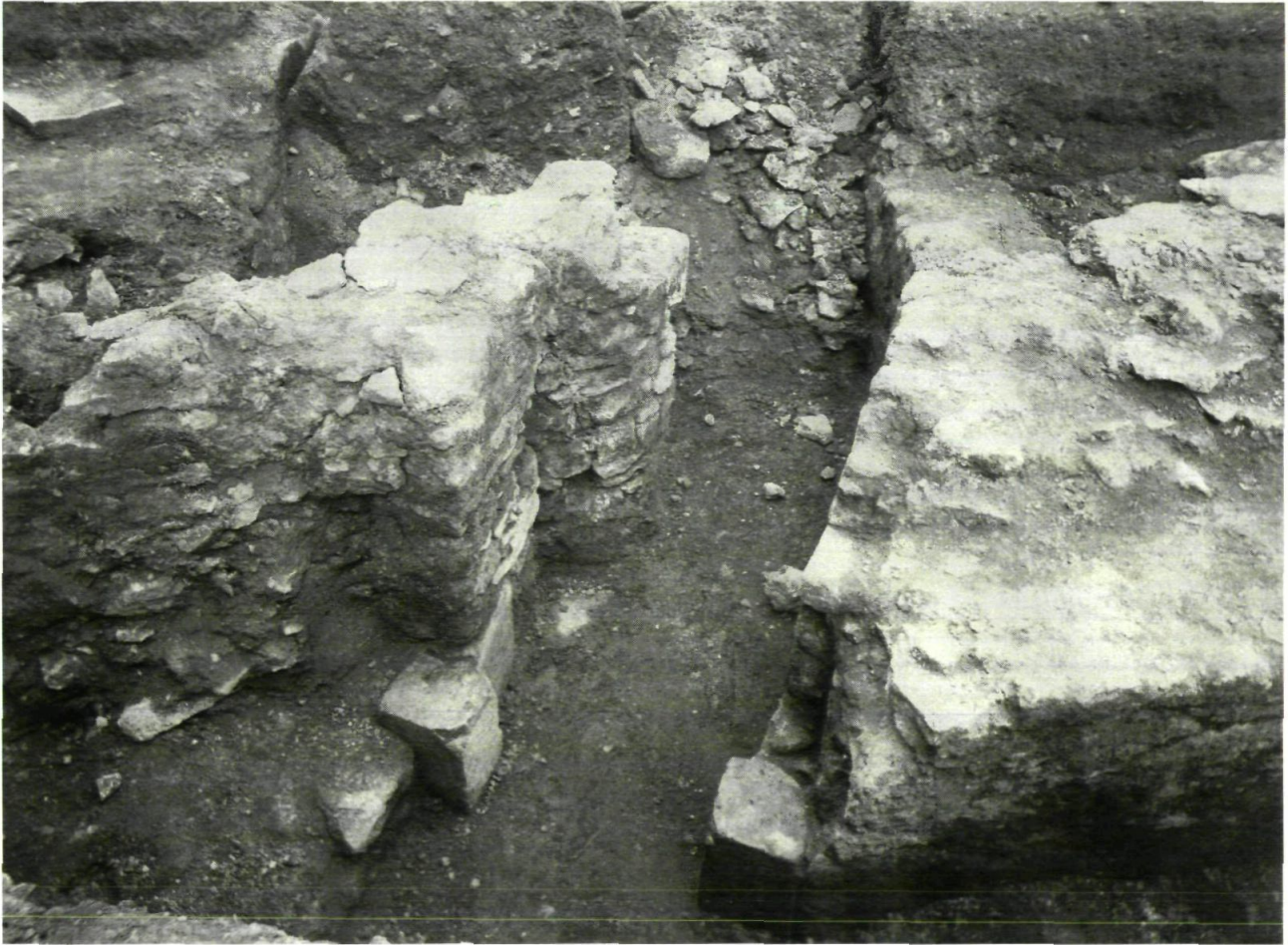
Plate 4.10 The doorway in the west side of Bastion 8, as excavated in 1899, looking west (Henry Taunt; reproduced by courtesy of OAHS).
