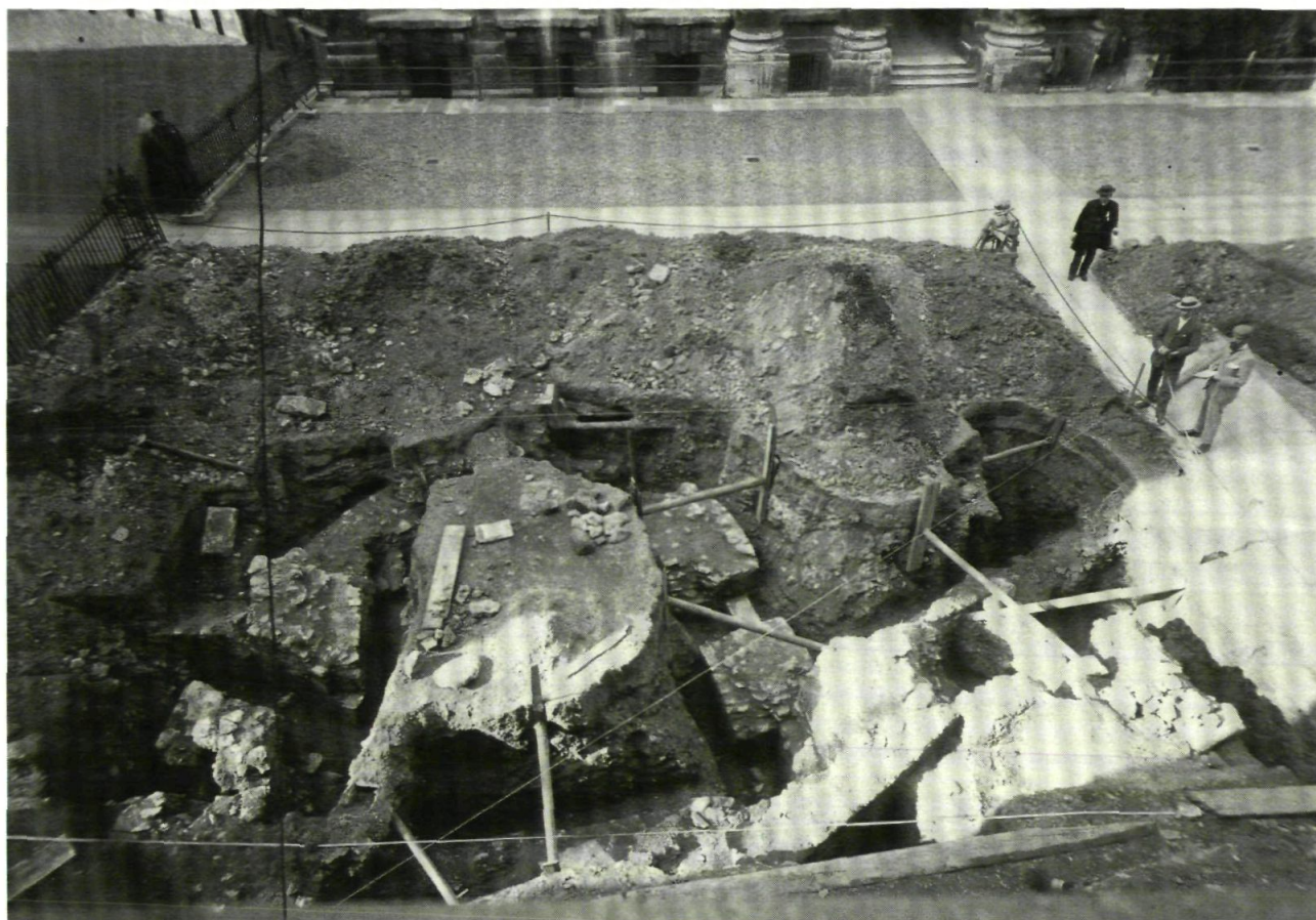
Plate 4.9 Bastion 8 in the City Wall, as excavated in 1899, looking north (Henry Taunt; reproduced by courtesy of OAHs).
