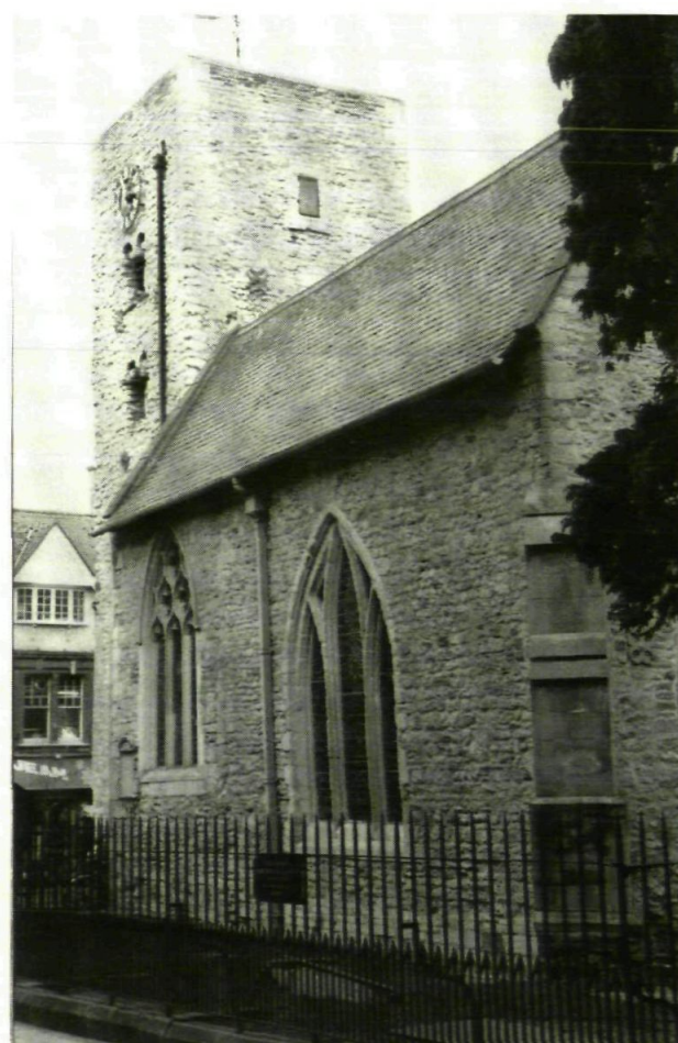
Plate 4.5 St Michael's Church and graveyard from Ship St, looking NW. Photo Mike Hallam.
