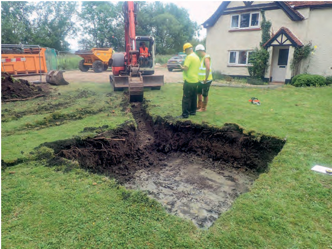
Plate 1: Trench 1, soak-away and partial pipe strip, looking north-west
