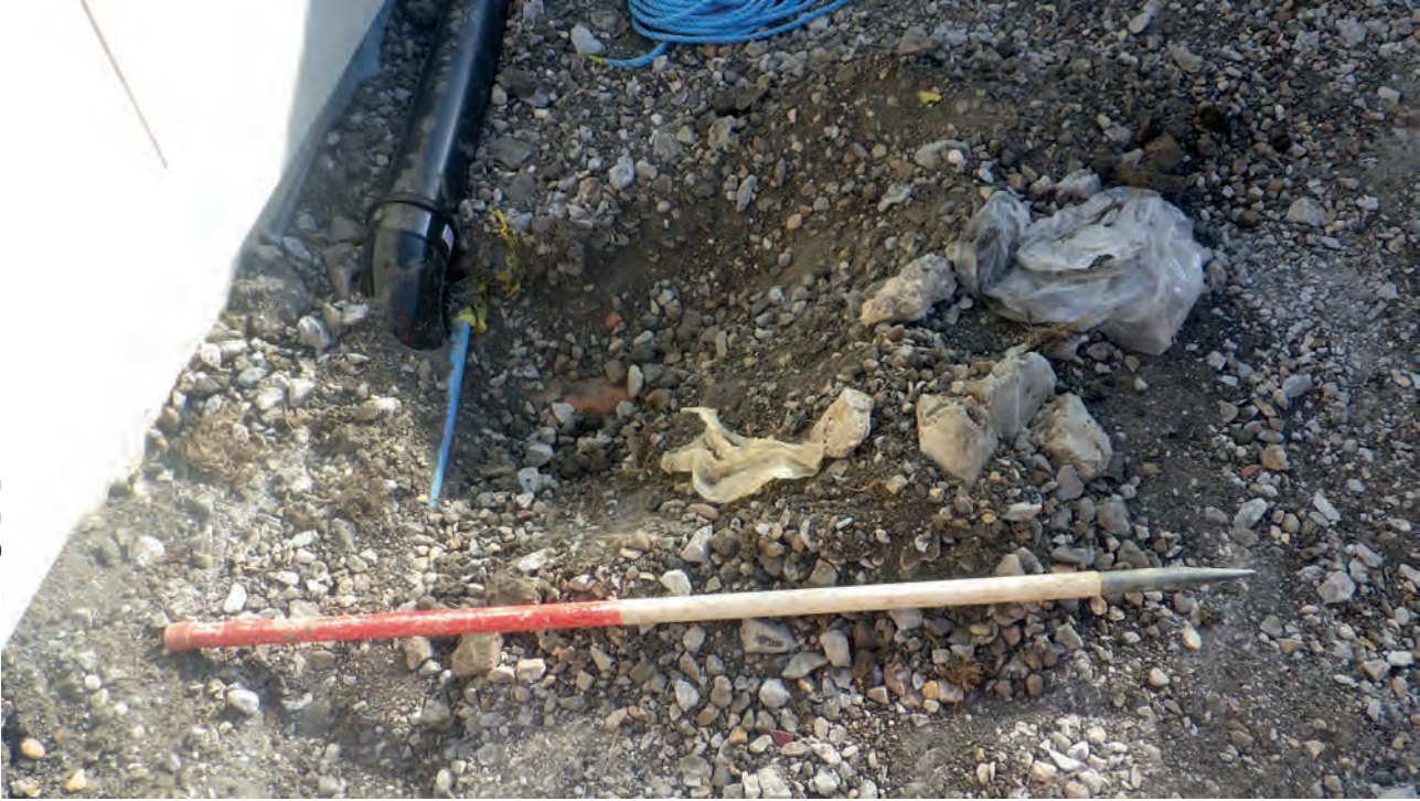
Plate 5: Trench 3, pipe trench, looking north-west
