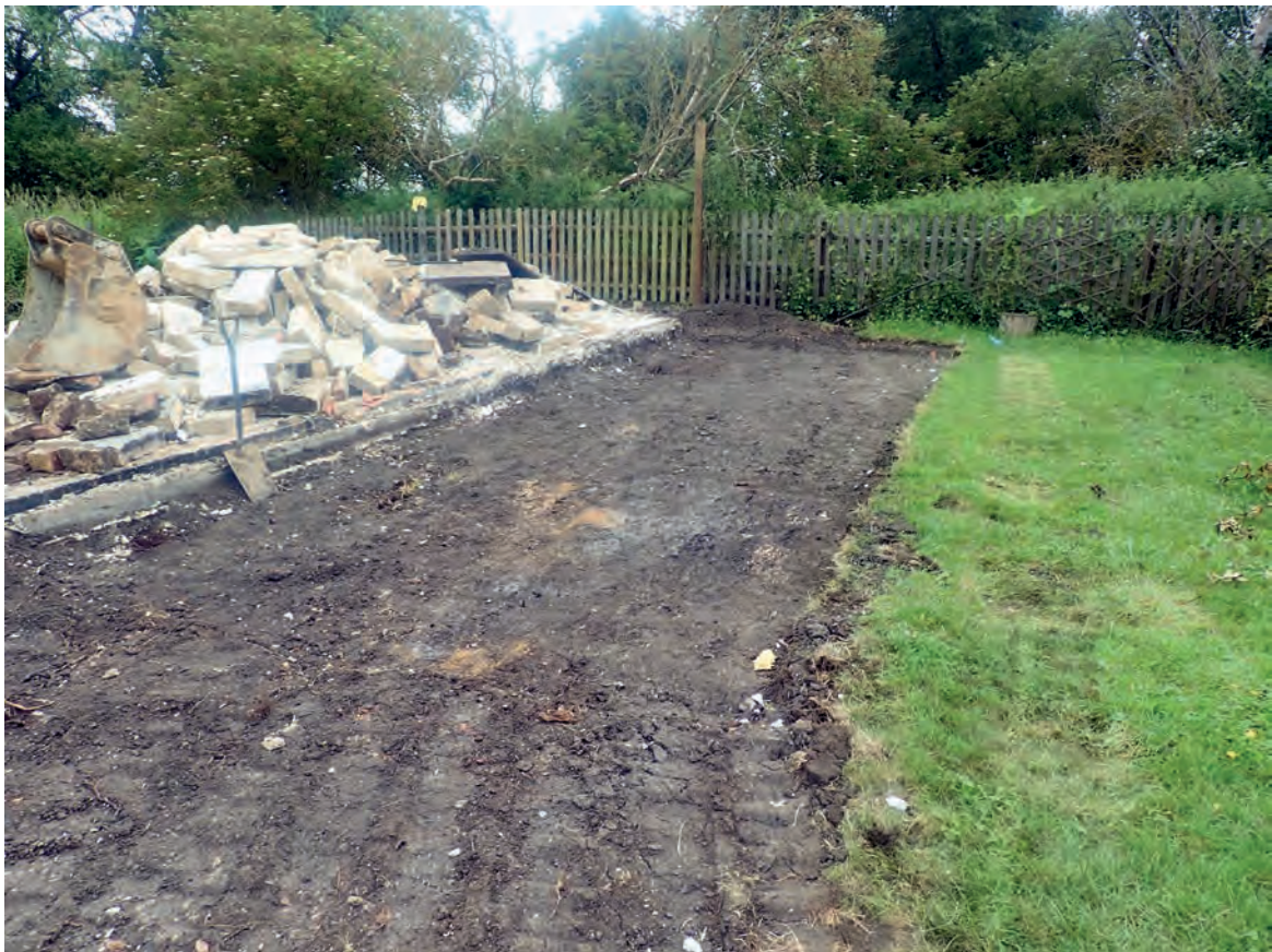
Plate 4: Trench 2, eastern building footprint, looking north-east
