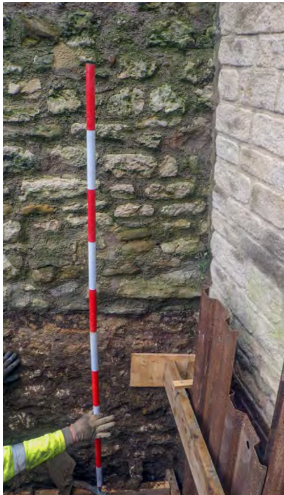
Plate 4: The College perimeter wall, looking east
