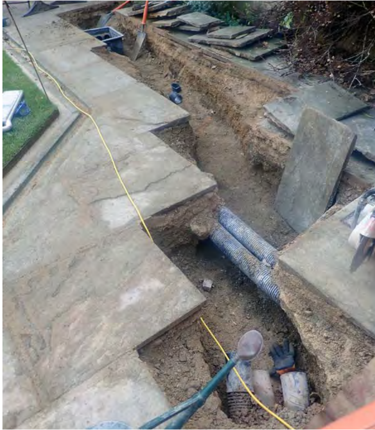
Plate 3: The trench in the south-west corner of Old Quad, looking south-east
