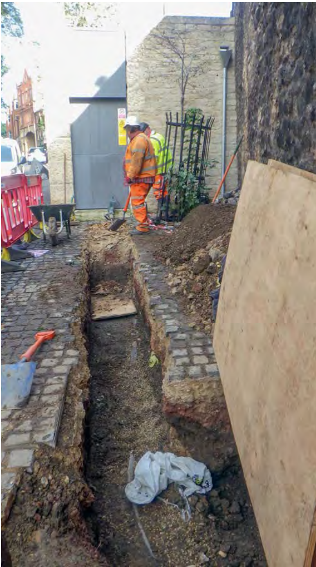
Plate 1: The trench in St Ebbes Road, looking north.
