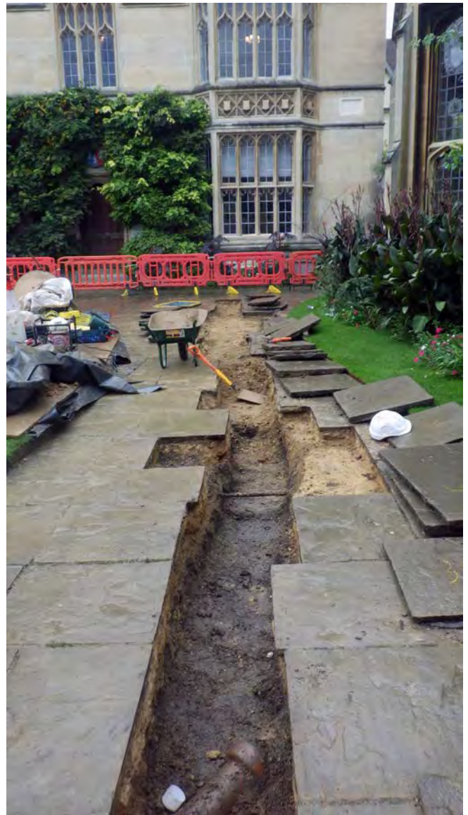
Plate 2: The trench in the north side of the Chapel Quad, looking east.
