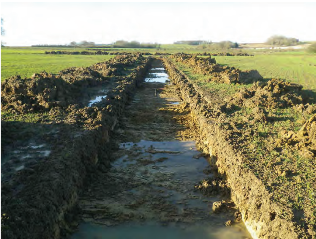
Plate 12: Photograph of Trench 23, showing the pooling of water on the surface and the poor drainage of the land, especially the field in the top right corner. Photograph taken from the west
