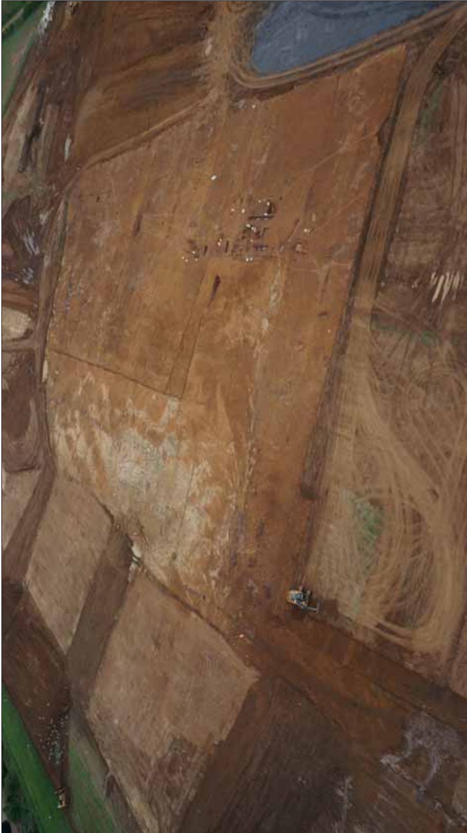
Plate 1: General overview of site (Areas P3 and P4)
