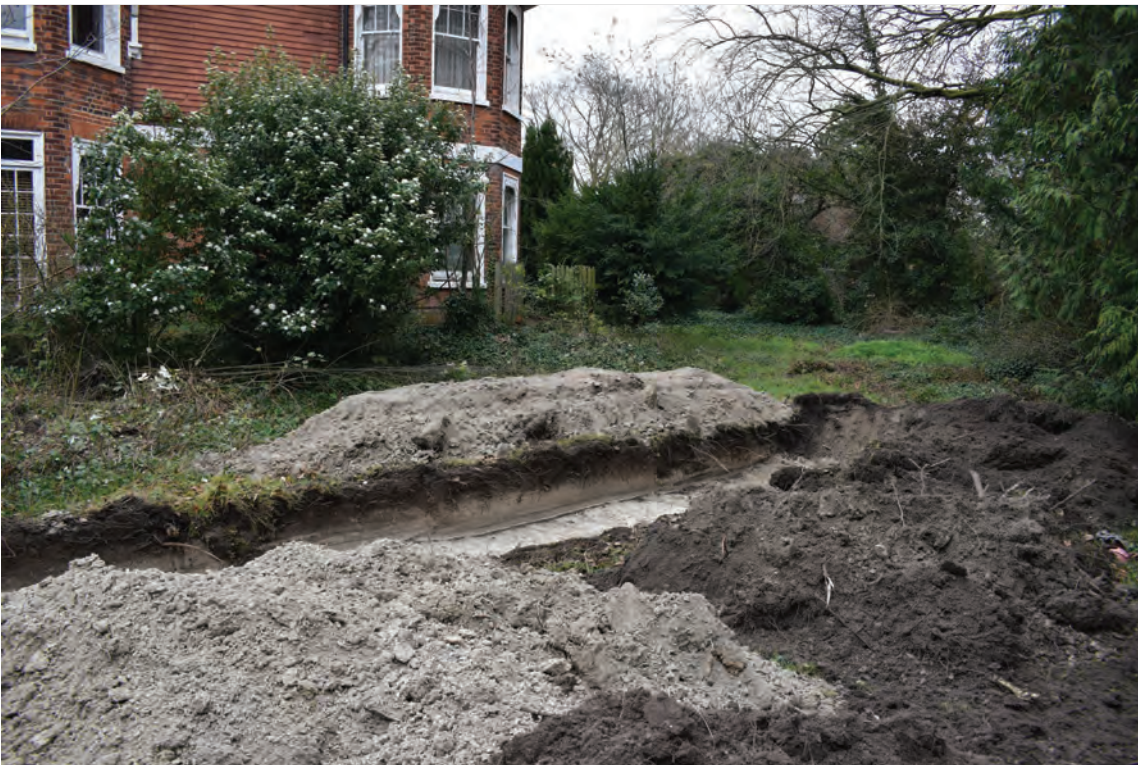
Plate 2: Site view, showing Trench 1 in the front garden of the house, looking east
