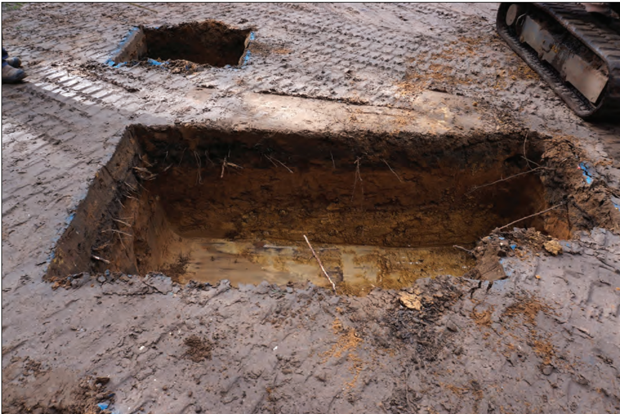
Plate 4: Excavation slot to south east of site
