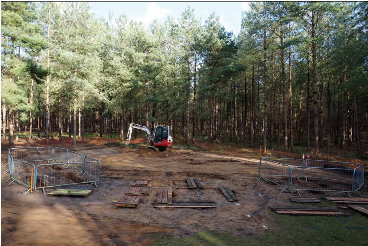
Plate 6: General work shot, looking south
