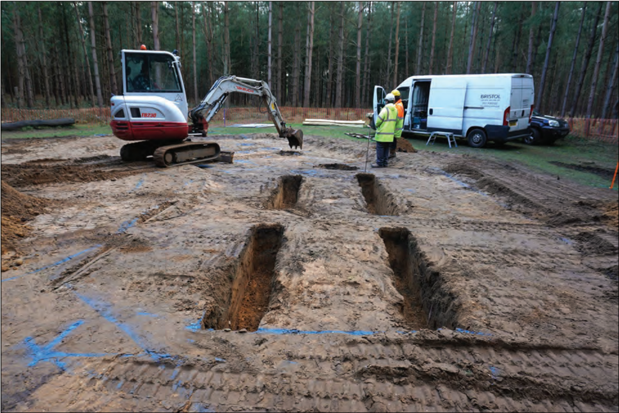
Plate 3: Timber Trailer slots, looking east
