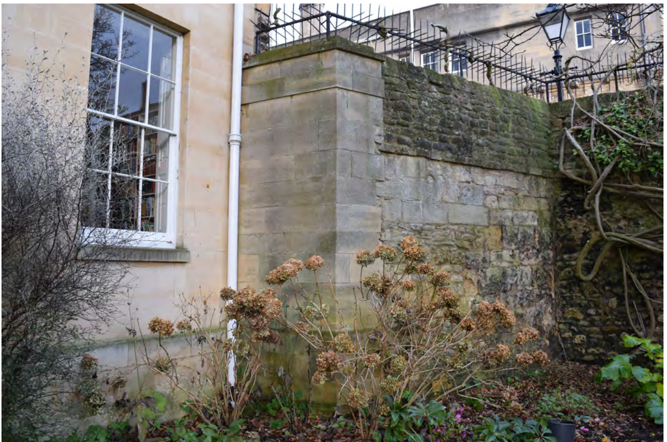
Plate 2: General view of east face of wall
