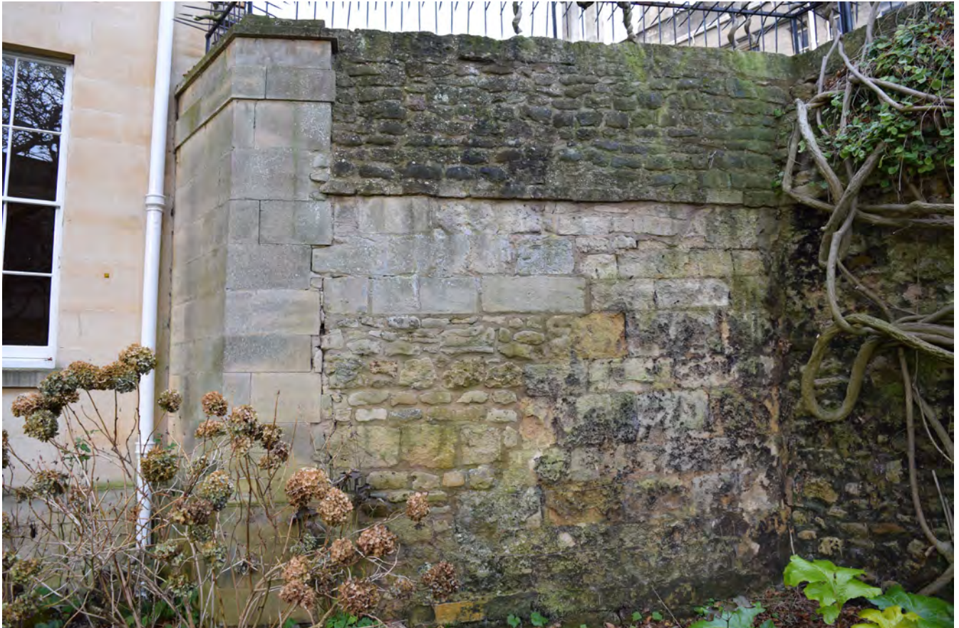
Plate 1: General view of west face of wall
