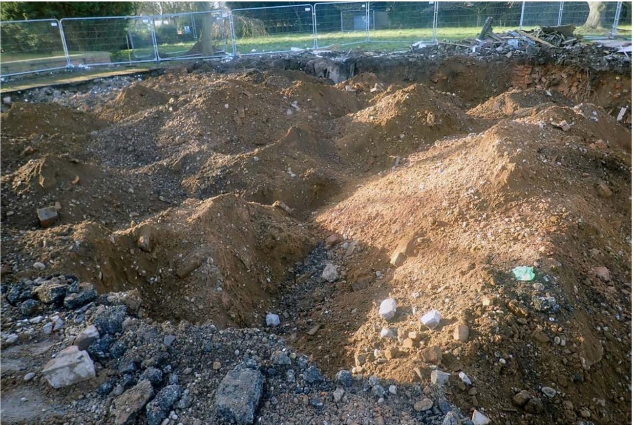
Plate 4: Grubbing out of Building 6 demolition area, looking south-west
