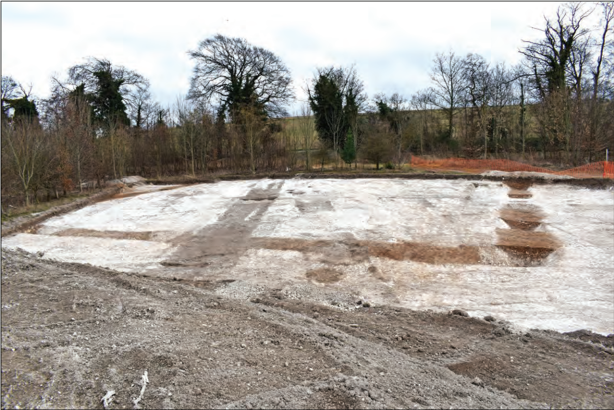
Plate 2: Mid-excavation shot of the site from the north
