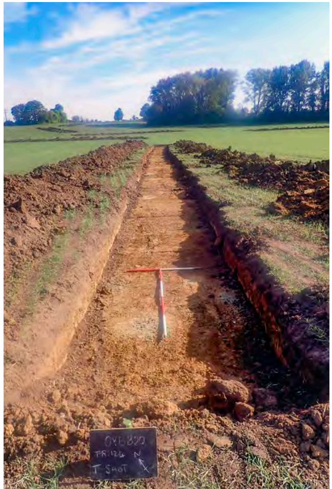
Plate 5: Trench 124, view to NE
