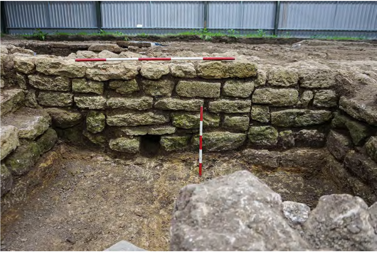
Plate 12: Room 1, internal faces of south walls 2071 and 2072, looking S
