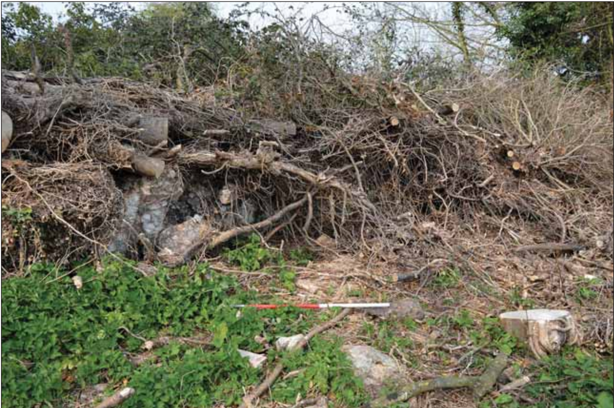
Plate 3: Wall, Feature 16, from north-west. Area C
