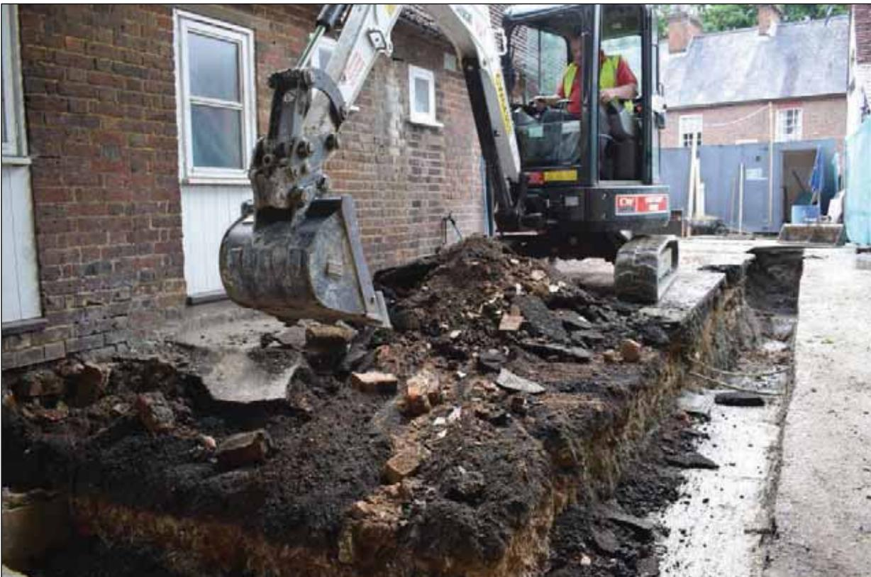
Plate 24: Working shot. Removing over burden
