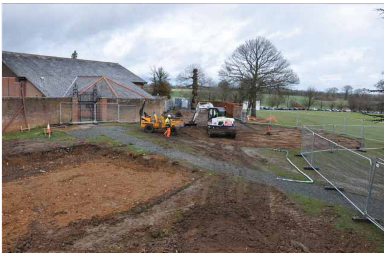
Plate 9: Removal of the building slab
