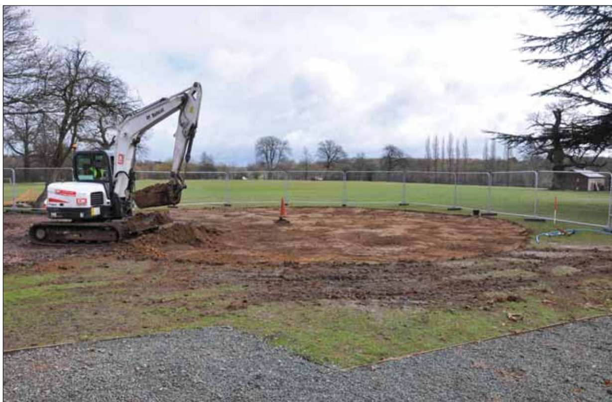
Plate 10: Soil removal in the area of the turning circle
