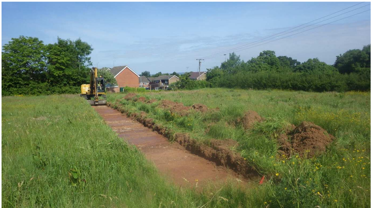
Plate 2: Machine stripping in field 3 looking northwest
