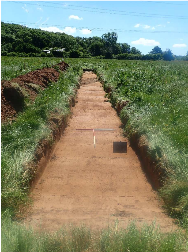
Plate 23: Trench 47 looking southeast (2x 1m scales)
