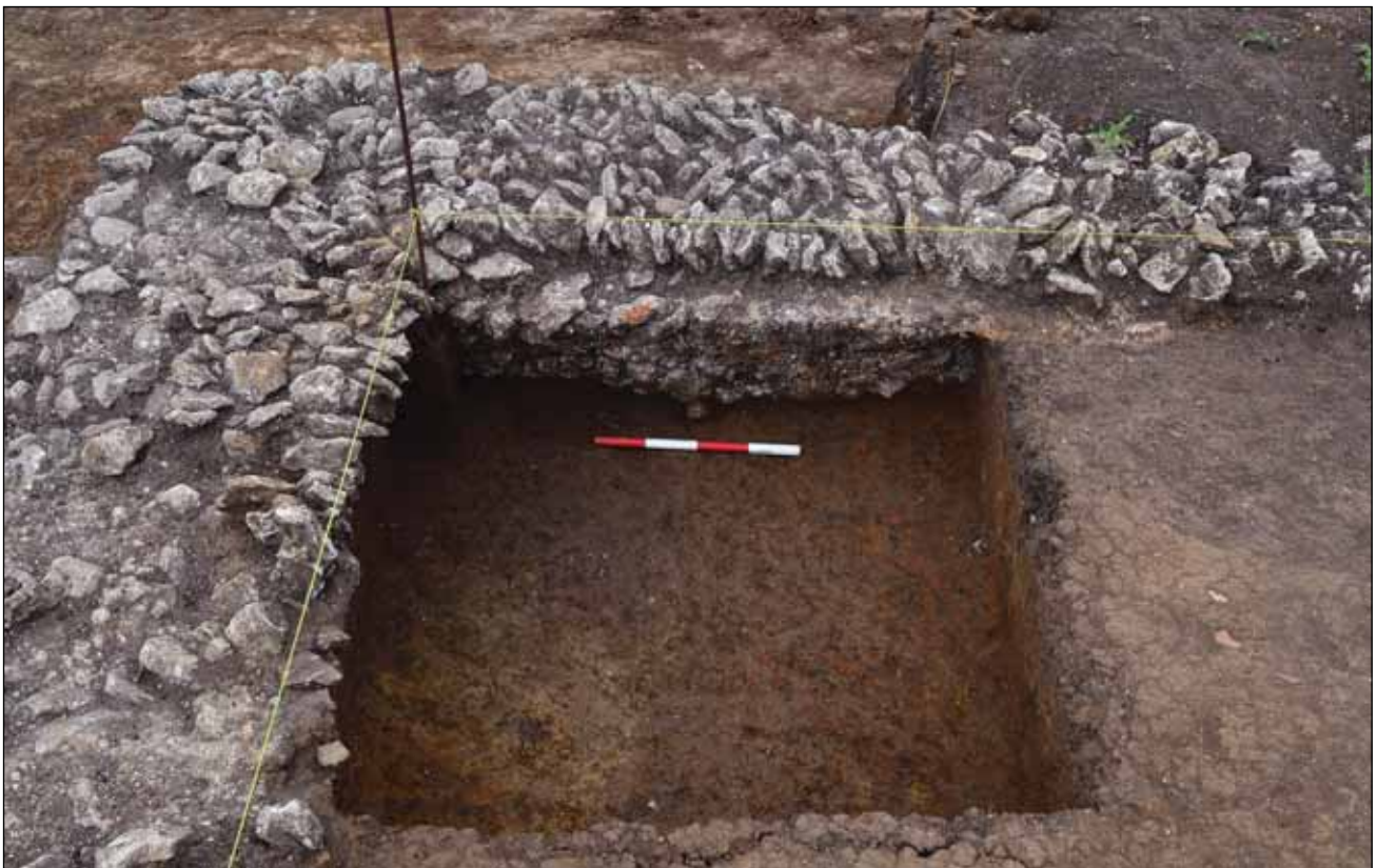
Plate 6: Exposed stone footing in Test Pit J4 at the southeast corner of Building 815 , looking west
