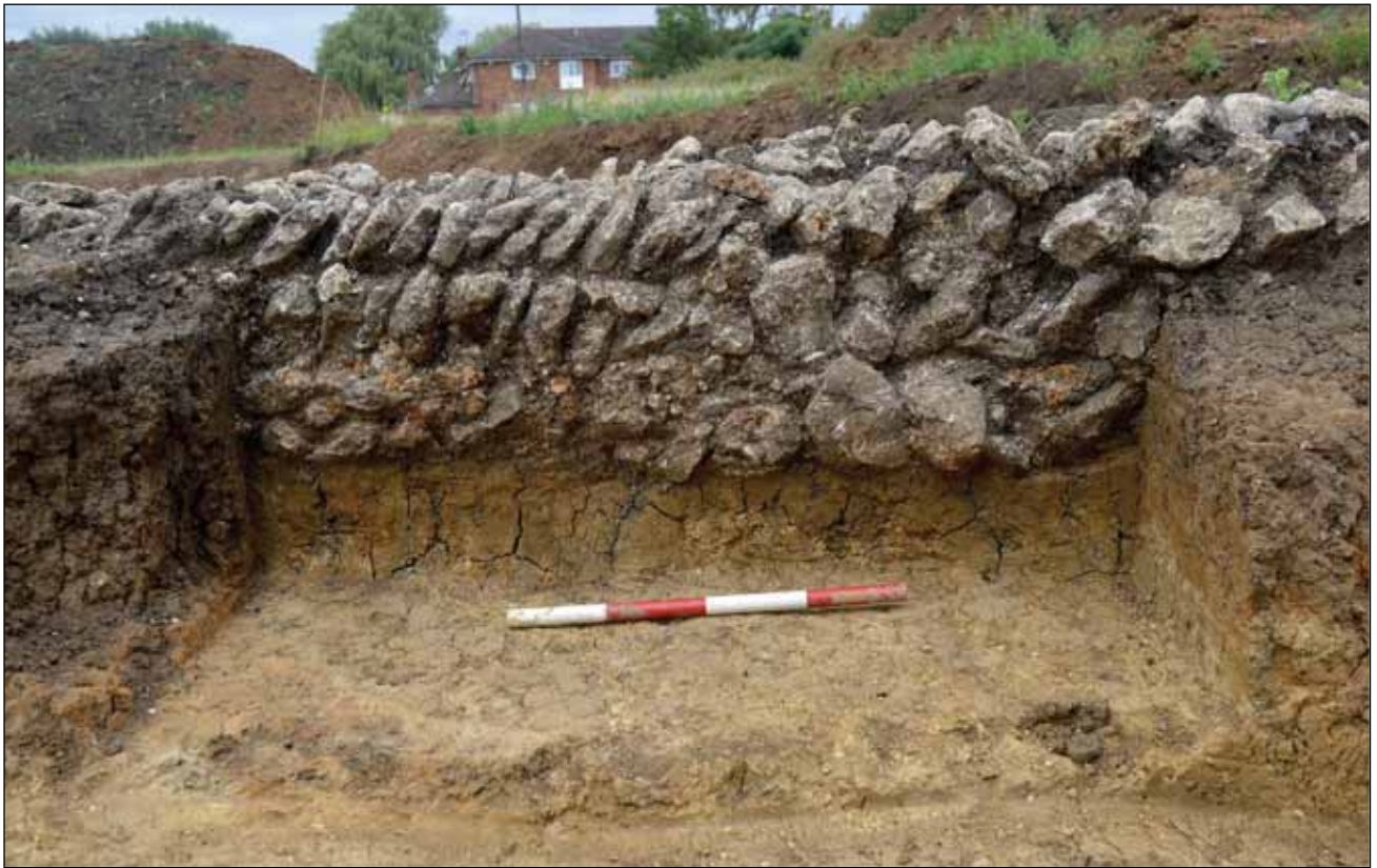
Plate 7: Detail of footing construction of aisled building 815
