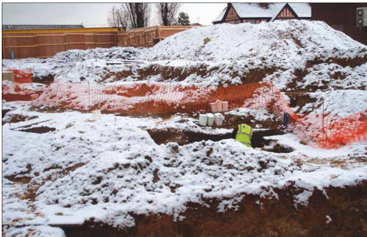
Plate 2: Site, looking north-east
