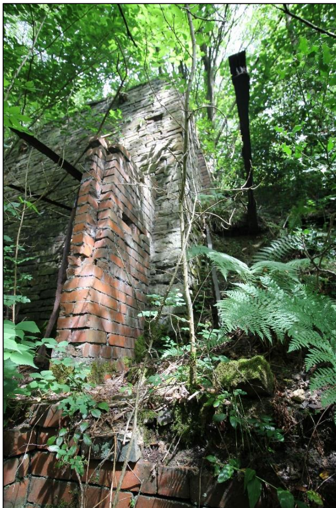
Plate 57: Corner of stone-built revetment wall, with redundant roof beam extend to right of centre
