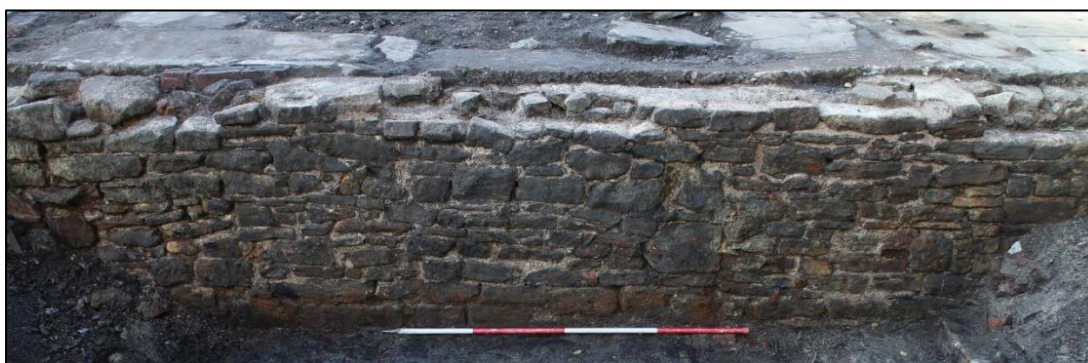
Plate 15: The north-eastern exterior elevation of the Phase 1 wall defining the southern bay of the mill/bleach works
