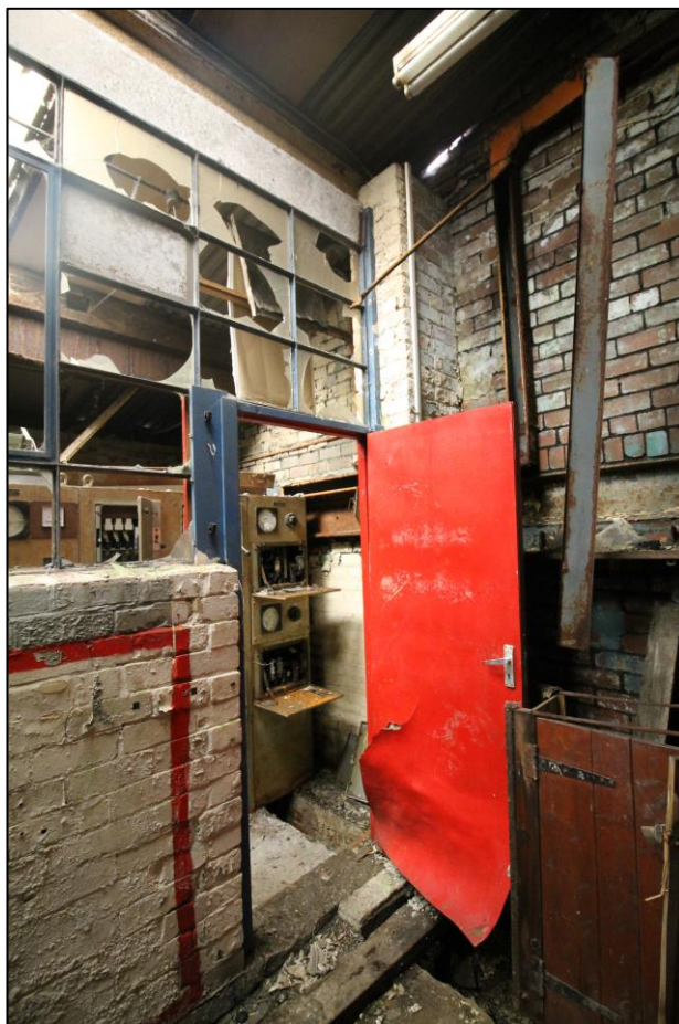
Plate 52: Electrical generation equipment at southern end of the eastern wall of the larger cell, facing south-west
