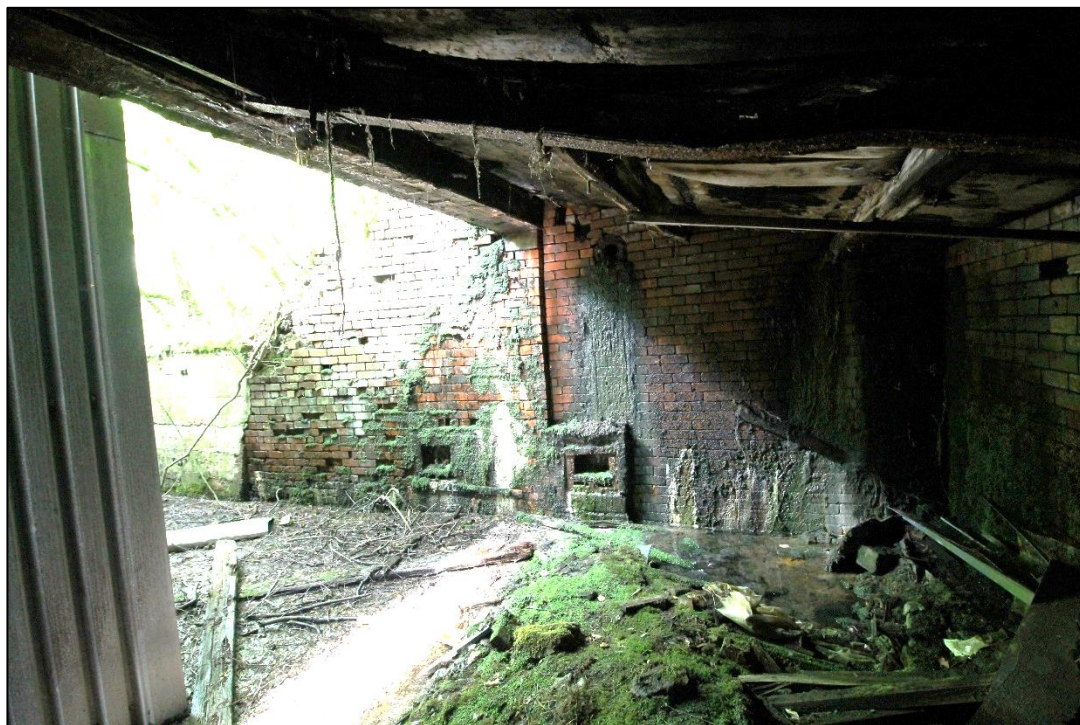
Plate 58: Open-sided brick-built structure, facing south-west
