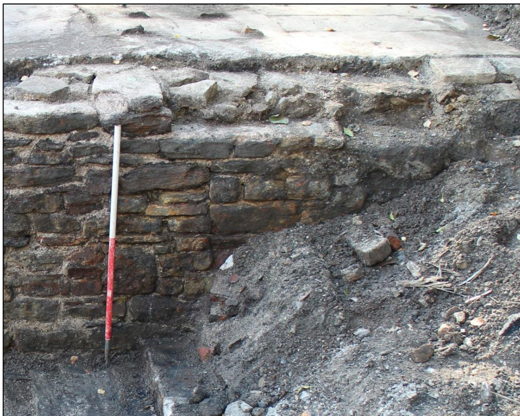
Plate 18: Infilled masonry (right) in the Phase 1 wall defining the southern bay of the mill/bleach works
