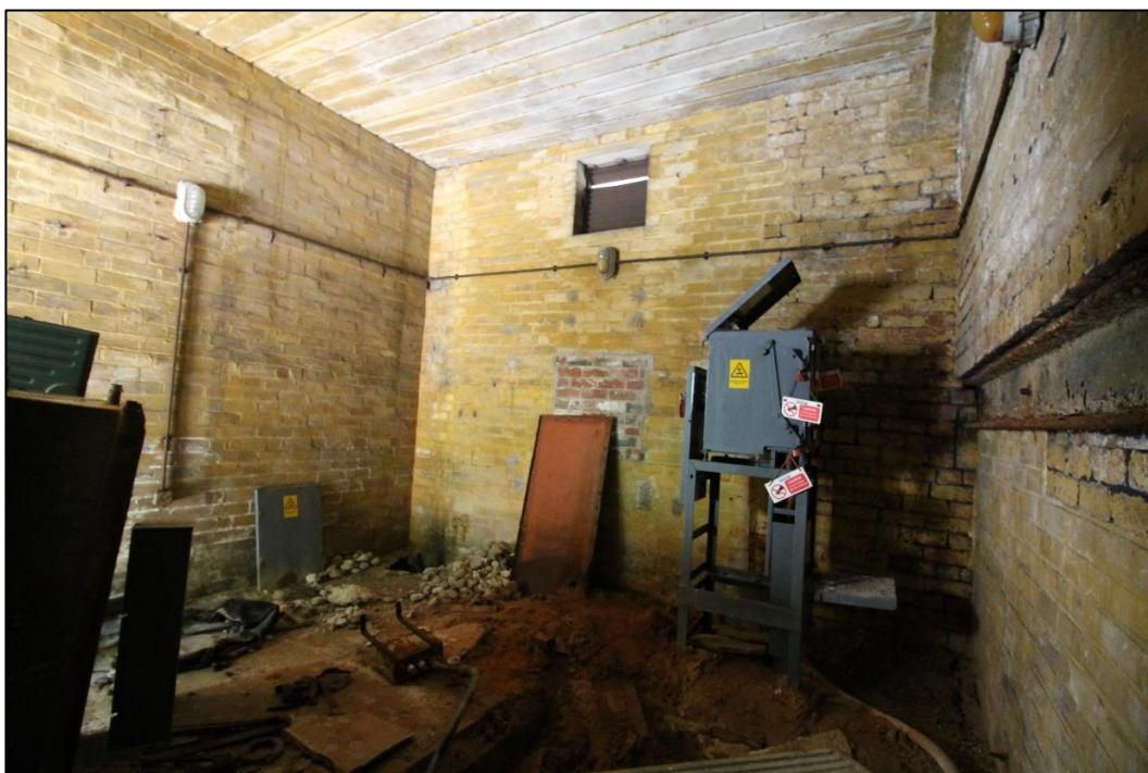
Plate 47: Interior of the smaller square cell, facing north
