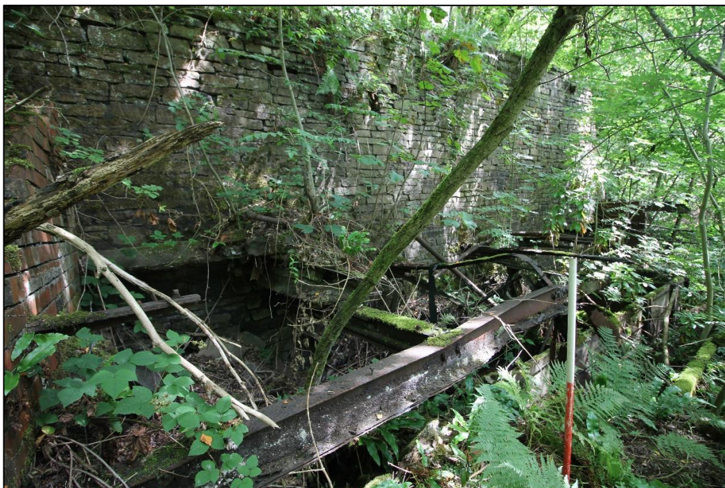
Plate 55: Steel frame above timber tanks, facing east
