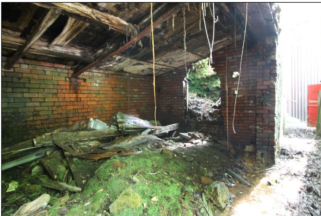
Plate 60: South-eastern end of open-sided building
