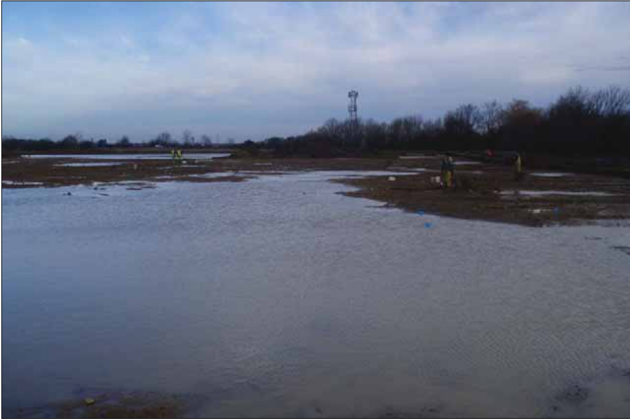
Plate 1: The excavation area from the south-west, showing the extent of flooding during excavation
