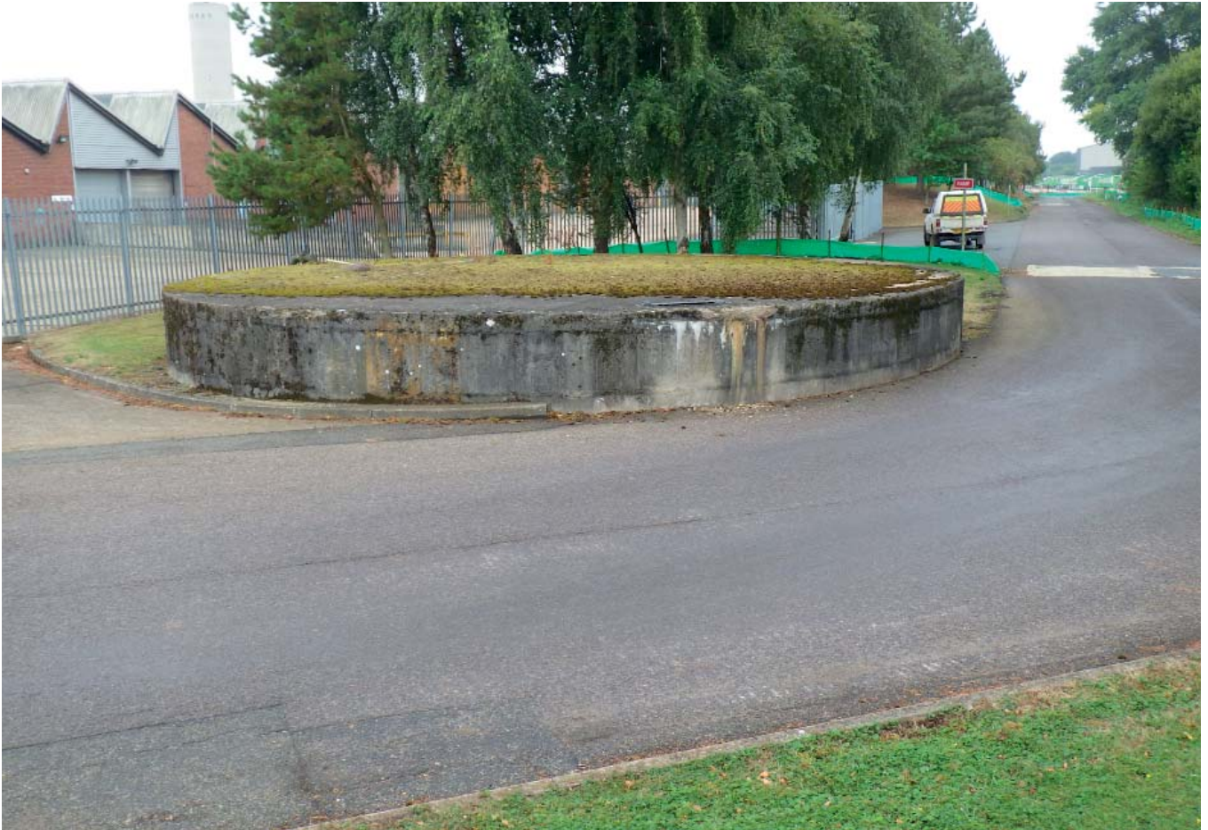
Plate 21 Large concrete water tank at north-west corner of the derelict distribution centre, looking south
