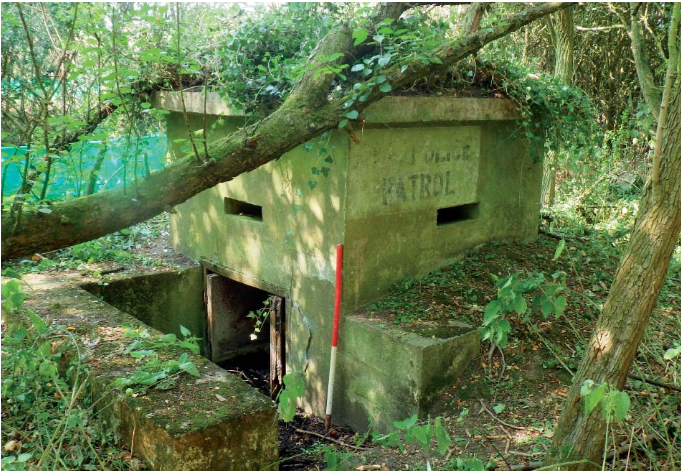
Plate 16 Western Pillbox, looking north-west
