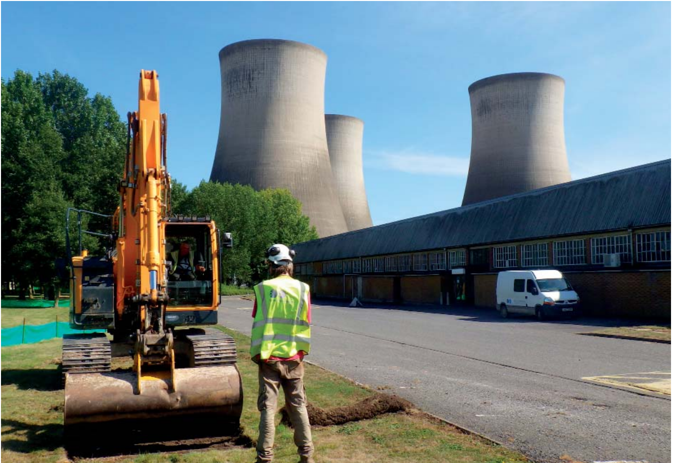
Plate 1 Trench 23; excavation of trench, facing east-south-east (cover photo)
