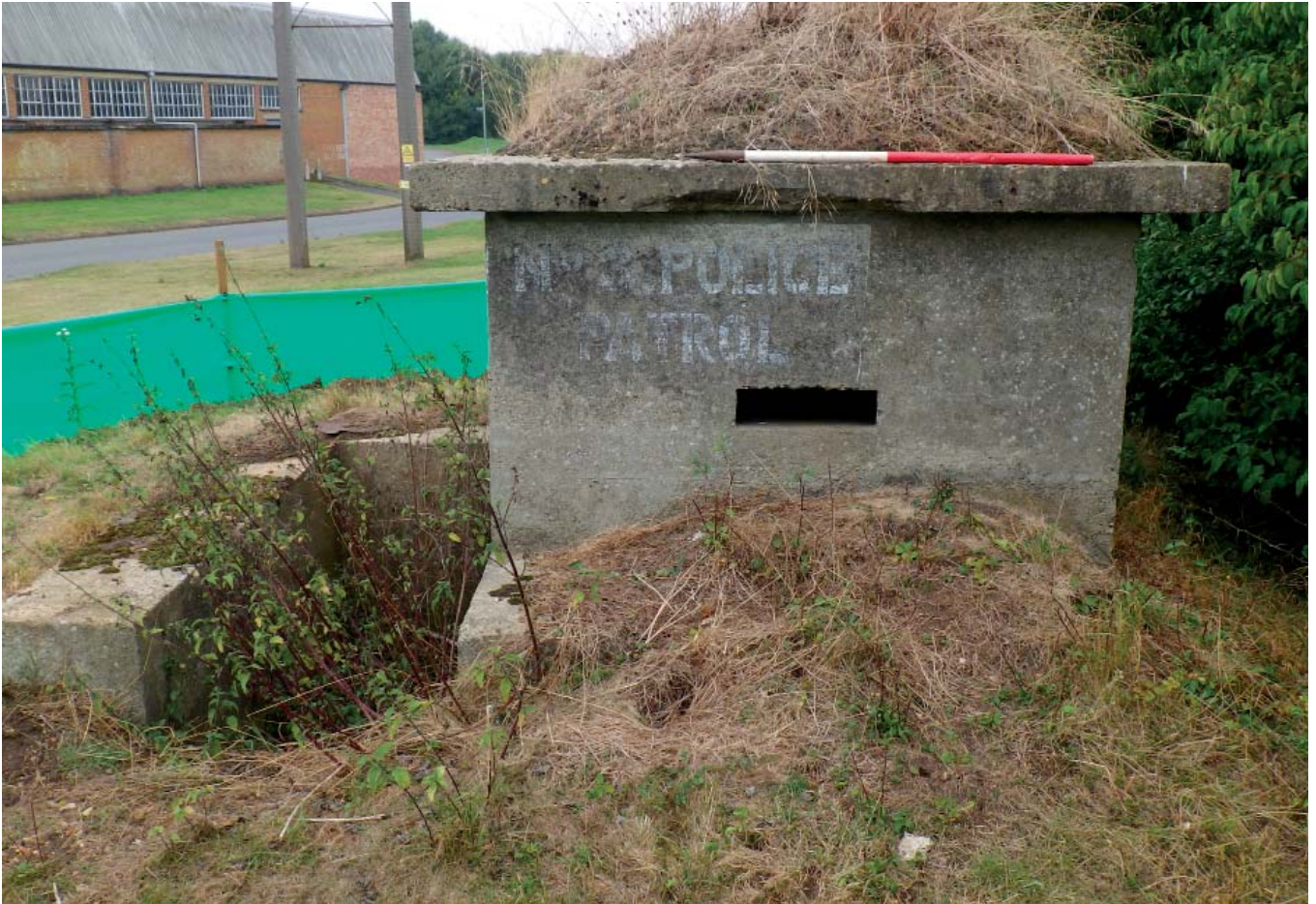
Plate 17 Eastern Pillbox, looking west
