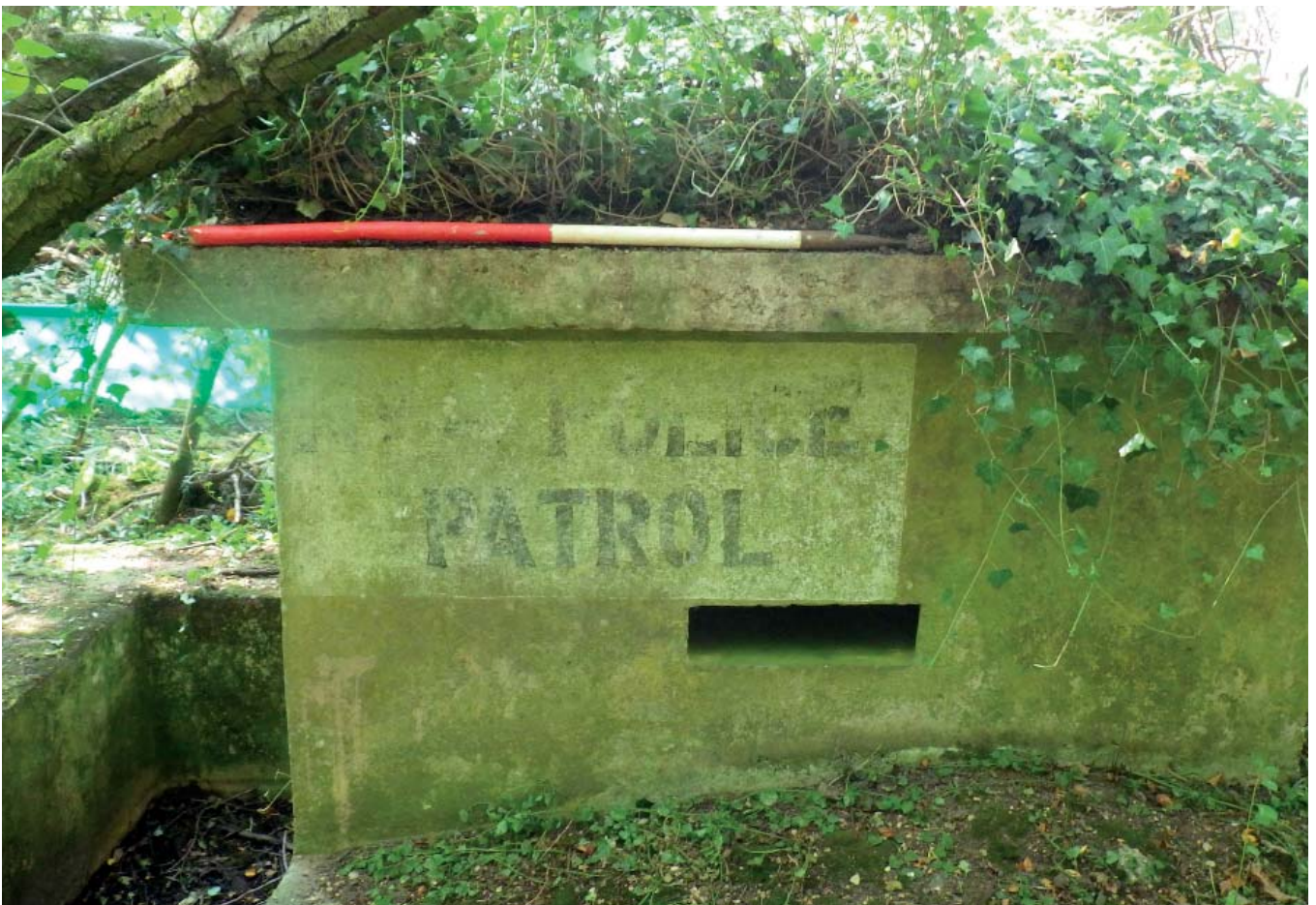
Plate 18 Western Pillbox, looking west
