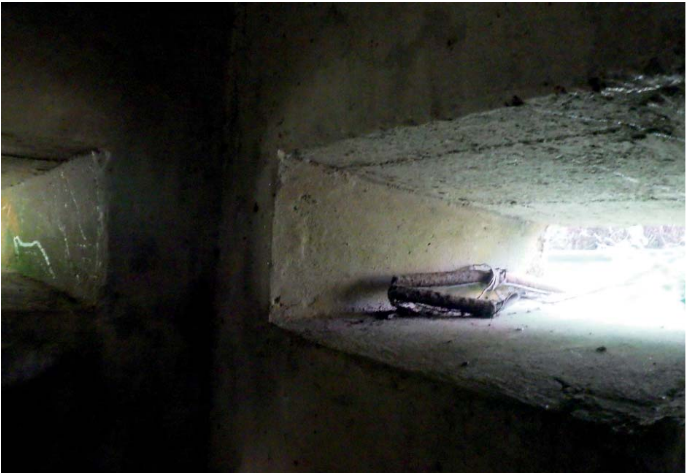
Plate 20 Loopholes in Western Pillbox, looking north-west
