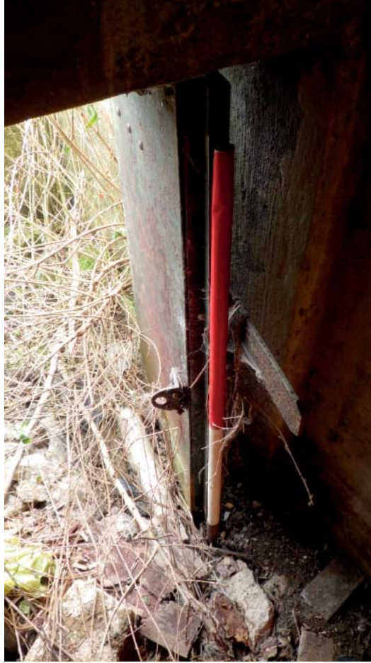
Plate 19 Door in Eastern Pillbox, looking south-west
