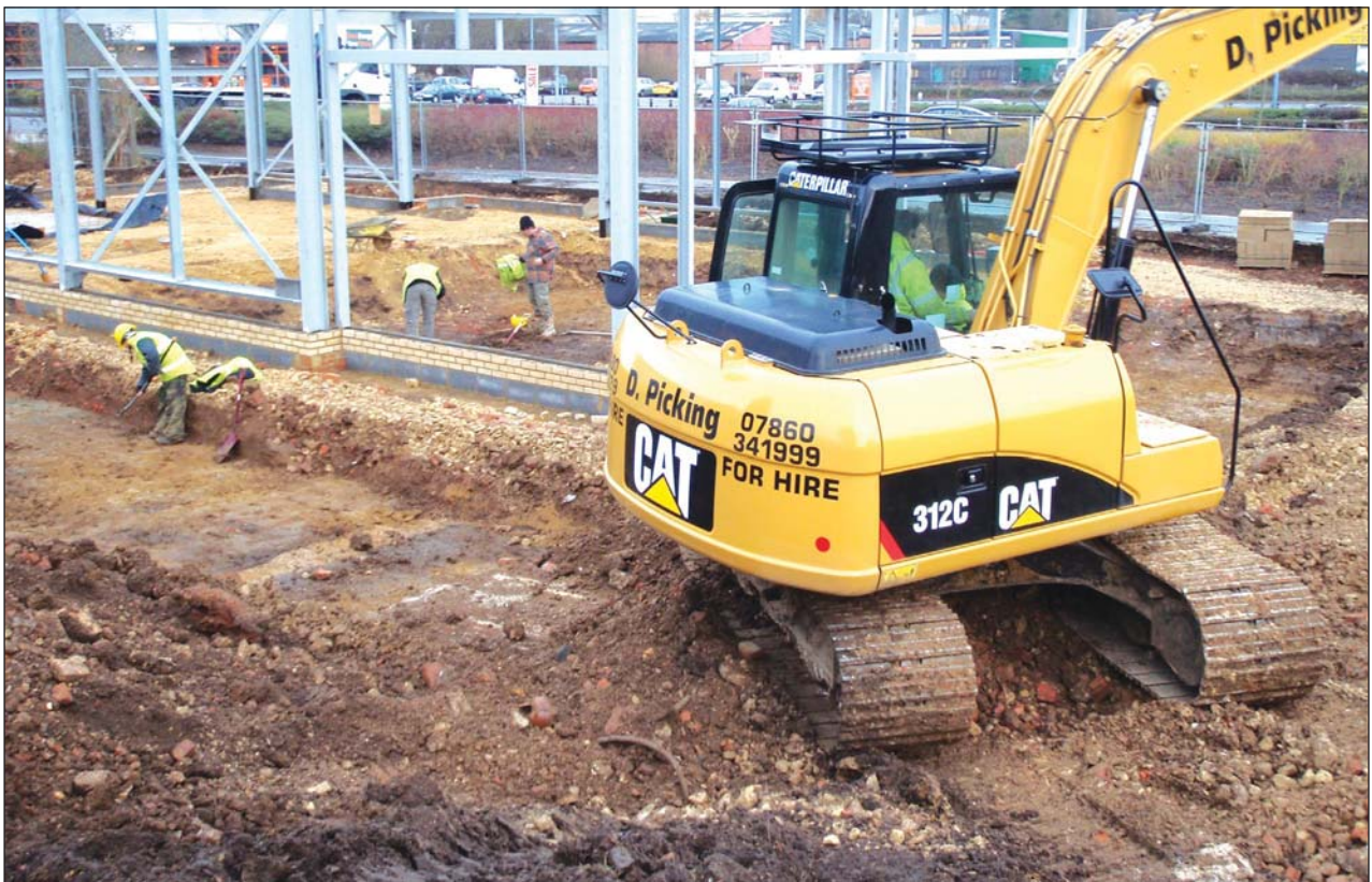
Plate 1: Machine stripping south side of the building
