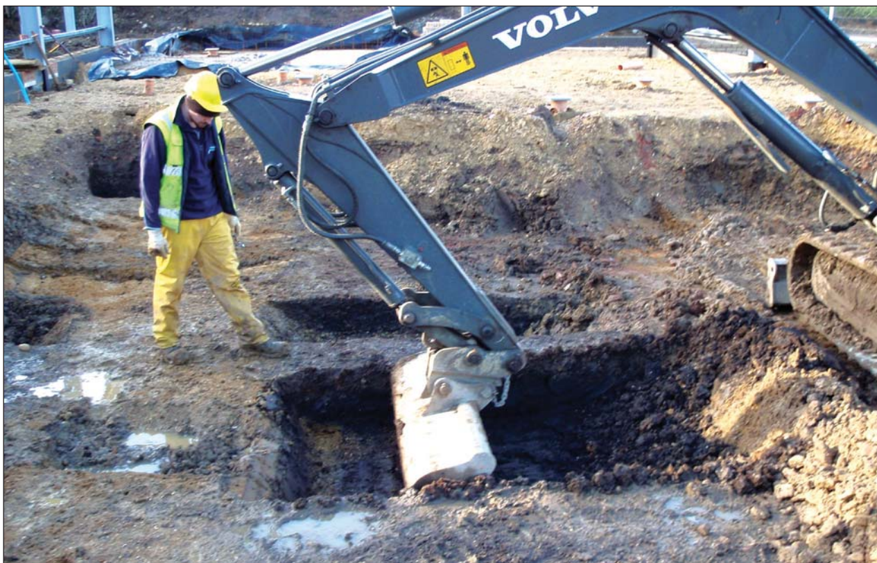
Plate 4: Machining within the structure
