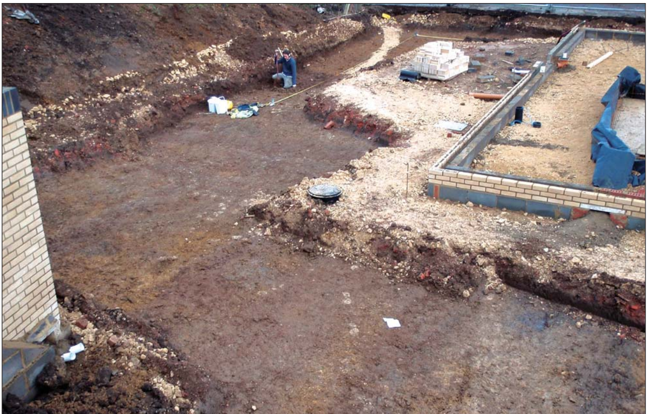
Plate 2: Western extent of area 3 with work beginning on ditch 450 and 435
