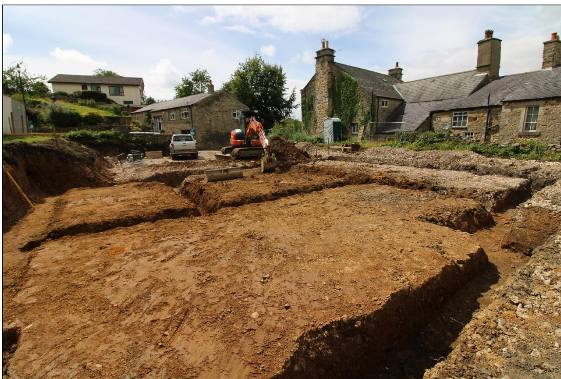
Plate 4: General site view during excavation of the footings. Note the levelling deposit in the top right corner, discernable by its lighter colouration
