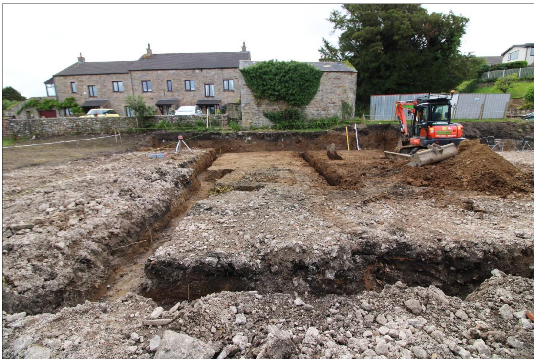
Plate 5: General view of site, facing east, with levelling deposit in the foreground
