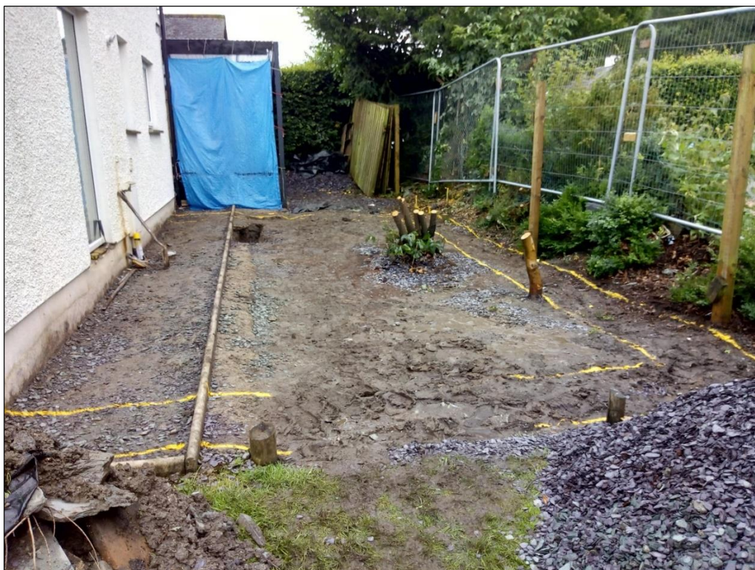
Plate 5: Layout of the foundation trench, facing north
