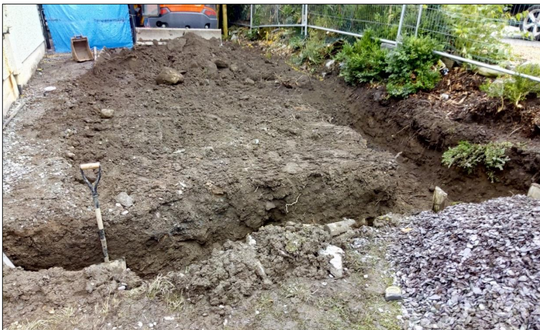
Plate 6: Foundation trench during excavation, facing north
