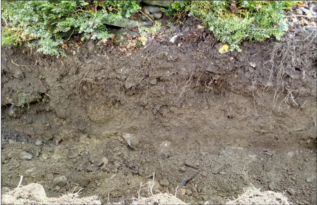
Plate 8: Representative close-up section through the sub-surface deposits, facing east
