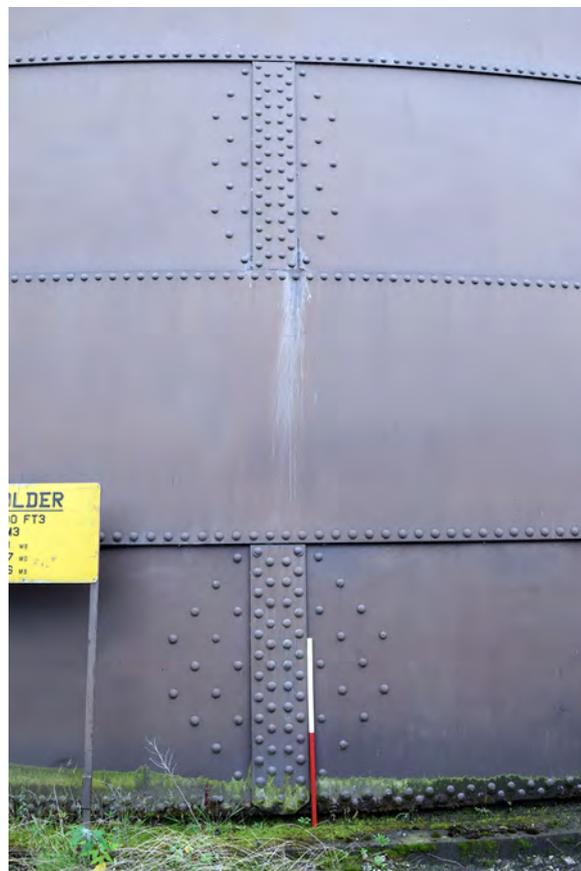
Plate 8: Example of the riveting of Gasholder 3
