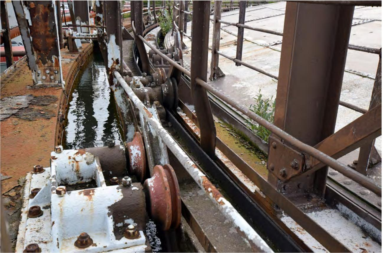
Plate 13: An example of the roller carriages of Gasholder 3
