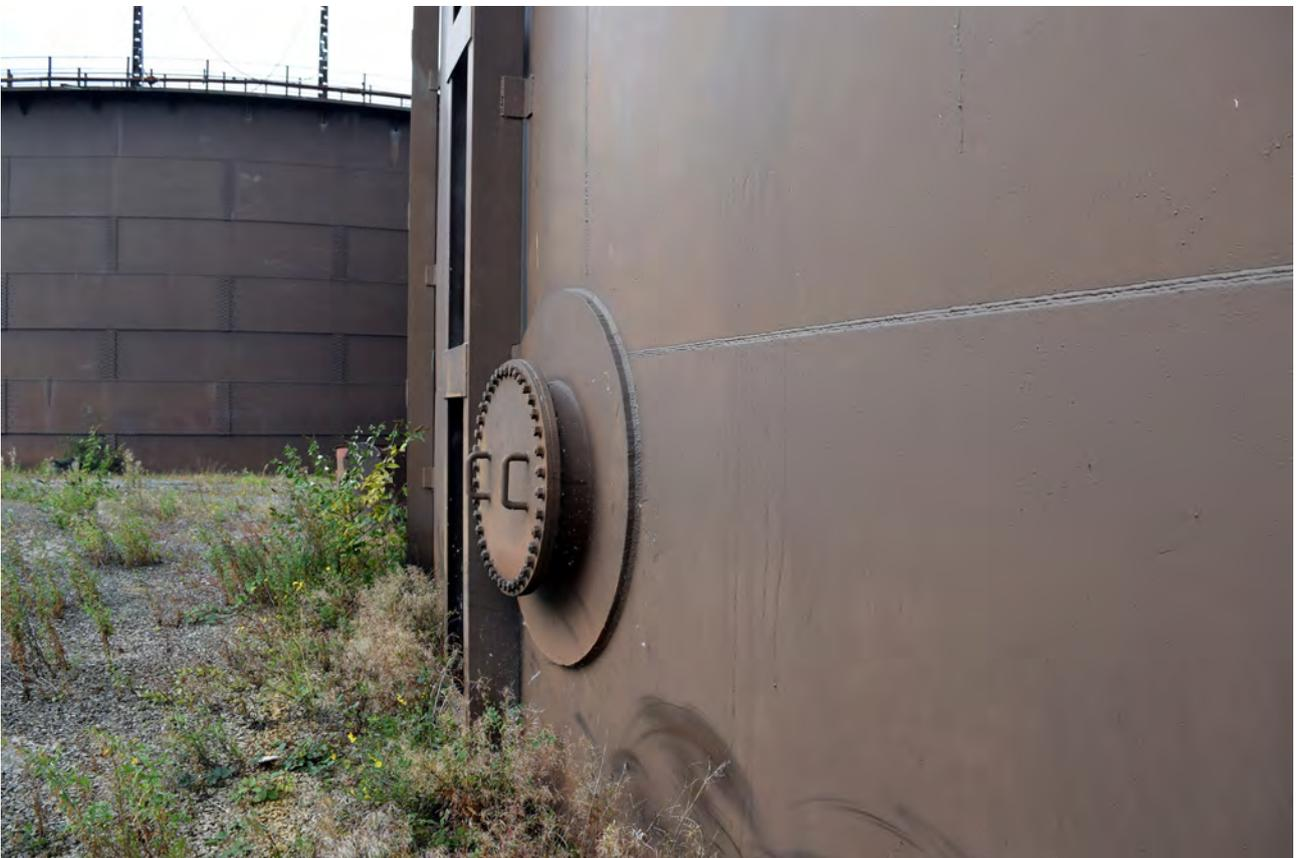
Plate 27: The access hatch to Gasholder 4
