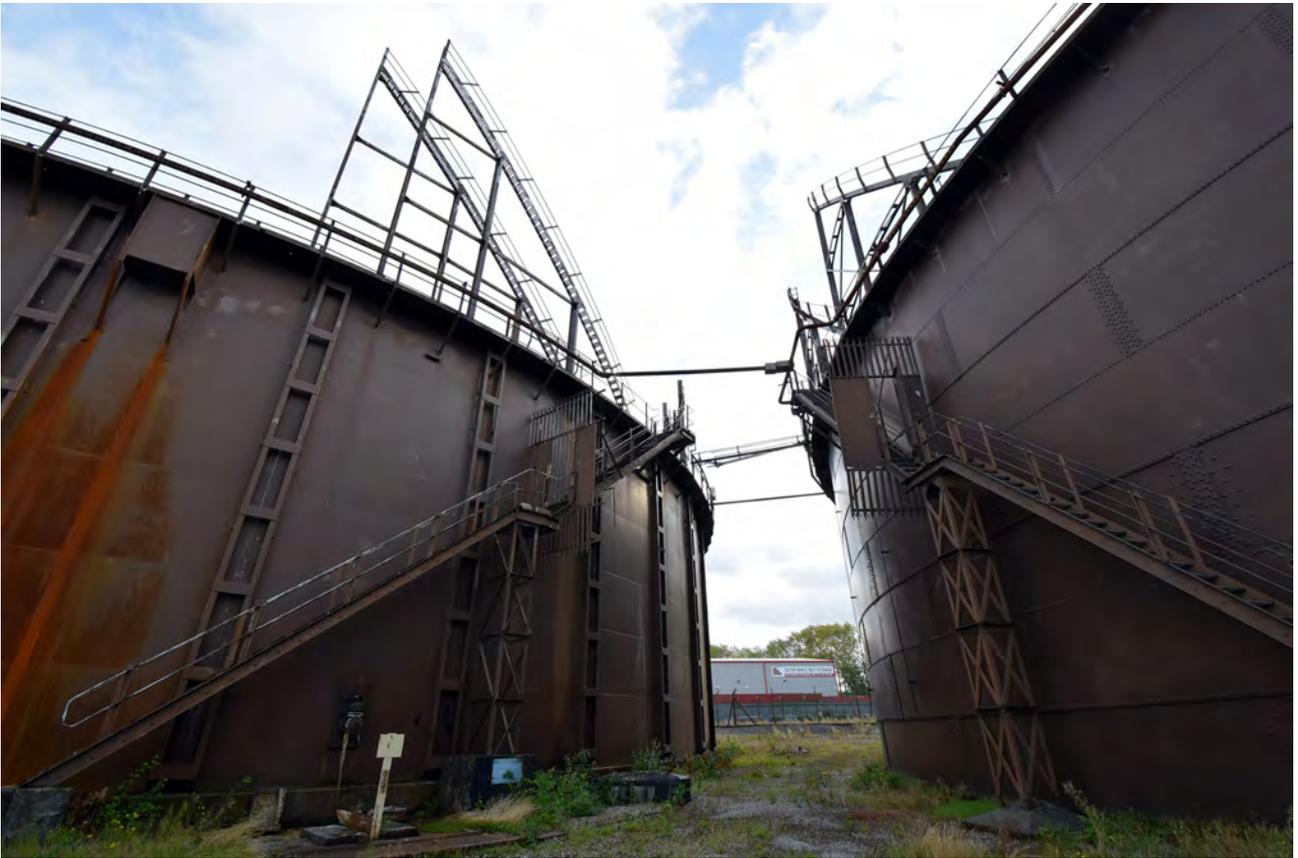
Plate 12: The anti-freeze pipes running between the two gasholders
