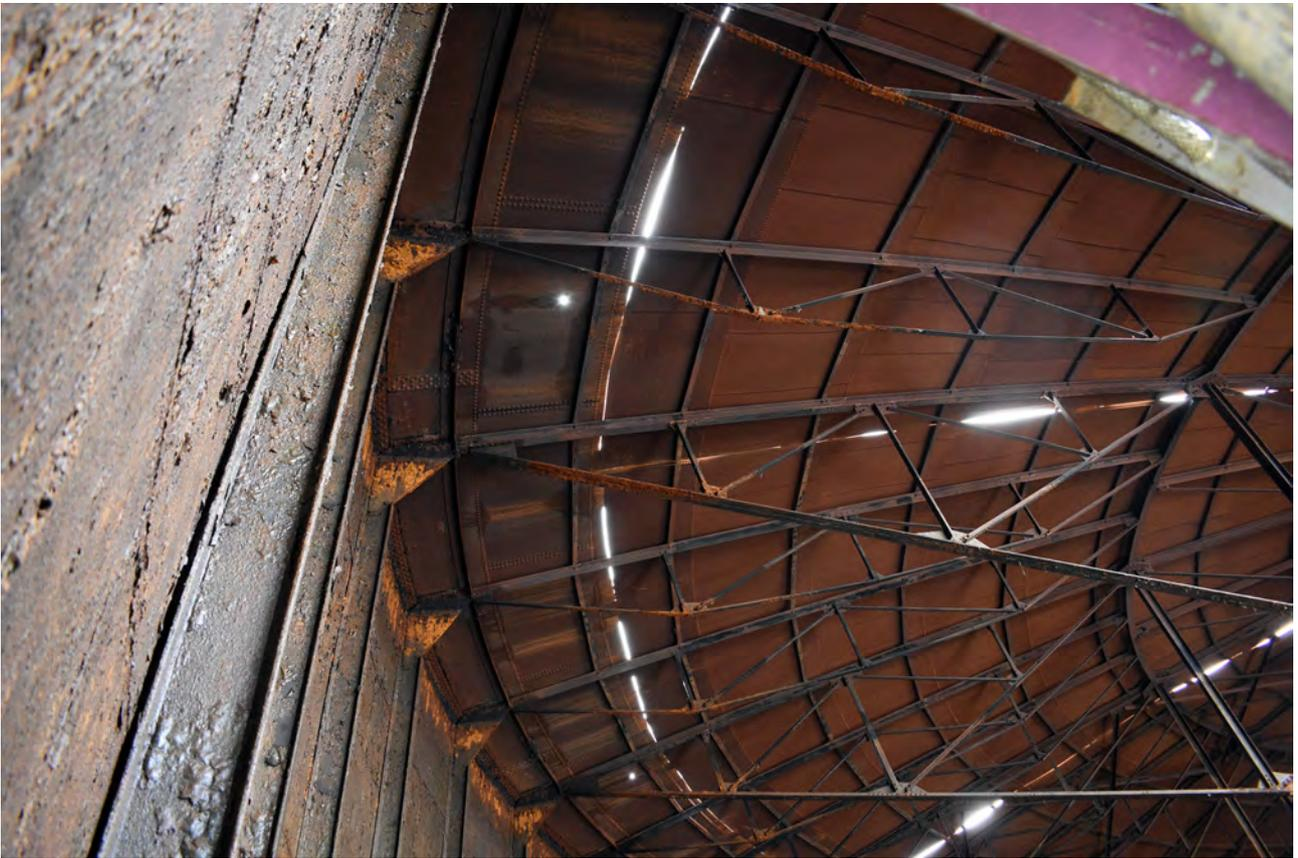
Plate 21: The underside of the crown of Gasholder 3
