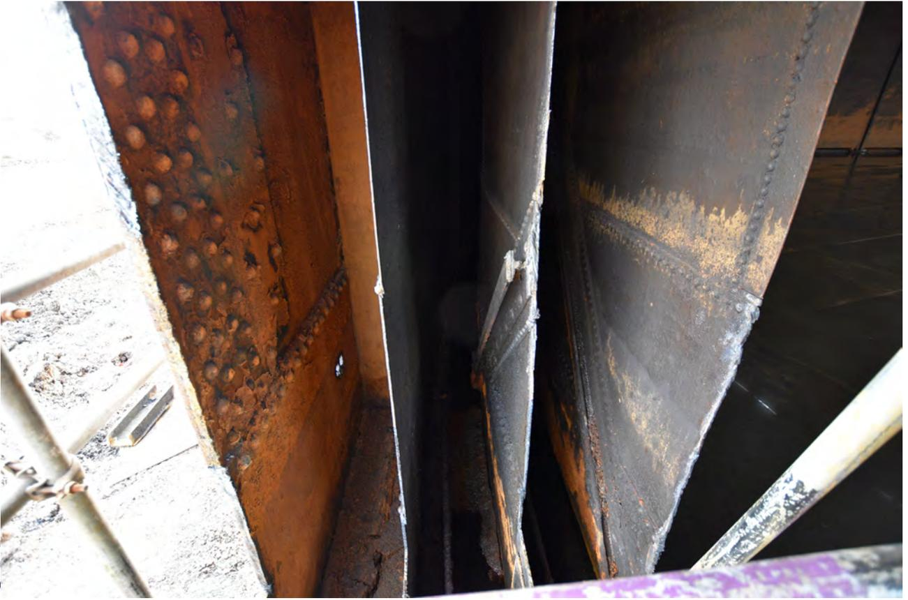
Plate 18: A section through the tank and lifts of Gasholder 3
