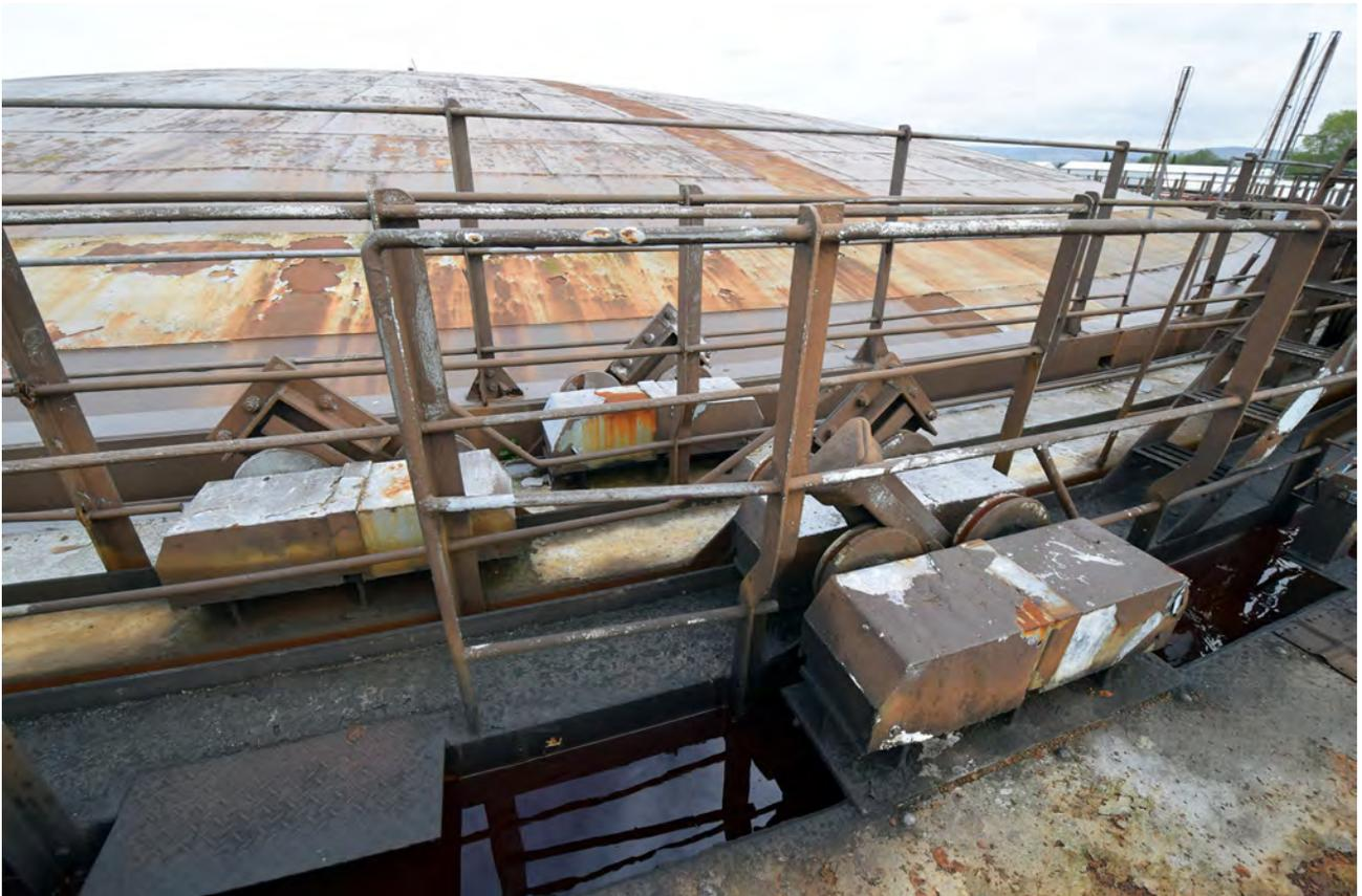
Plate 29: An example of the roller carriages of Gasholder 4
