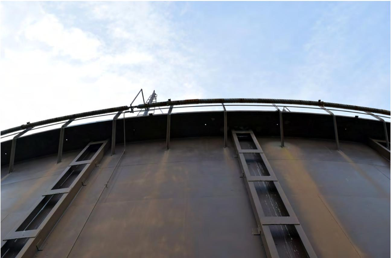
Plate 25: An example of the walkway and railing fittings to Gasholder 4
