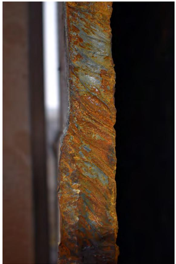
Plate 34: An example of the join in panels of the tank of Gasholder 4
