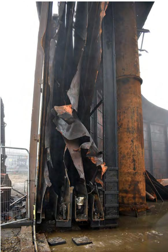
Plate 33: A section through the tank and lifts of Gasholder 4
