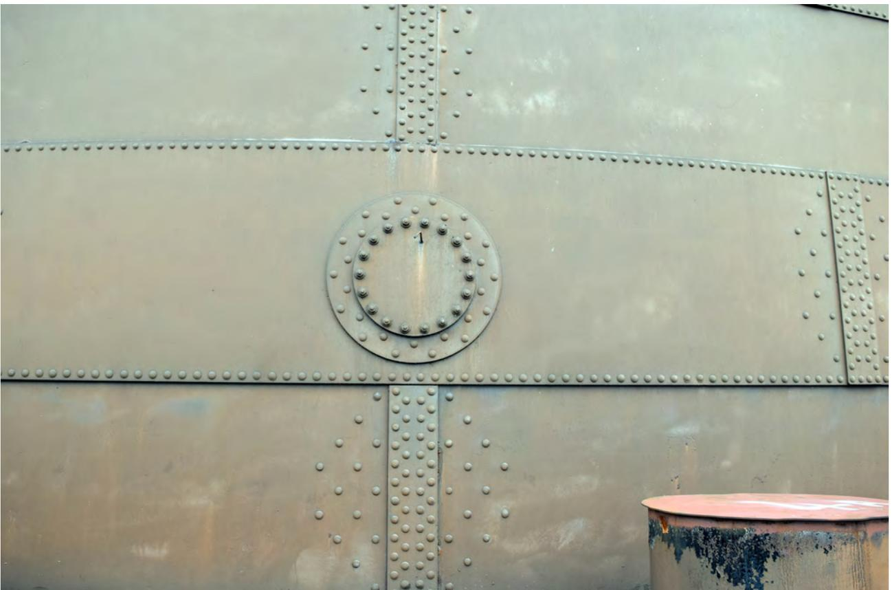
Plate 10: The access hatch to Gasholder 3
