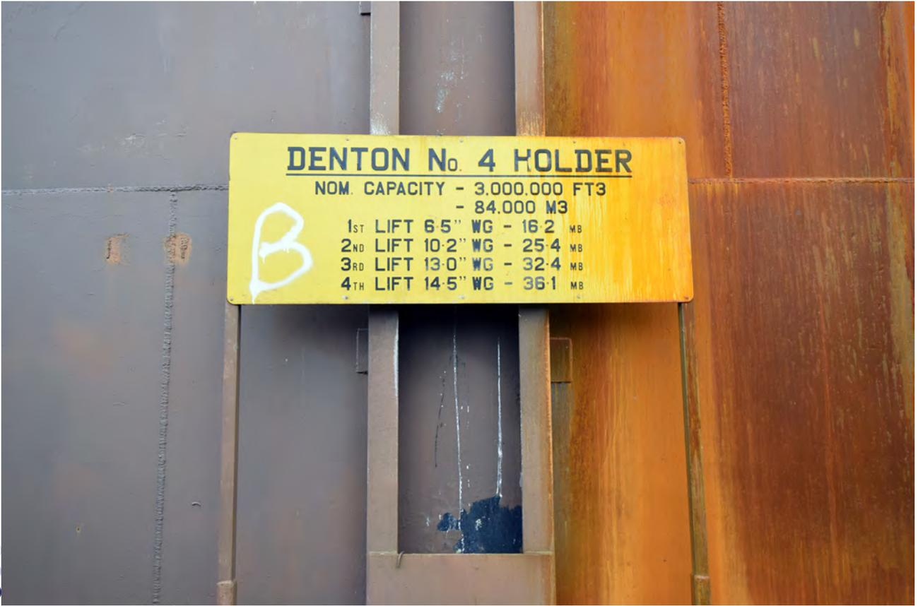
Plate 24: Information plate fitted to Gasholder 4
