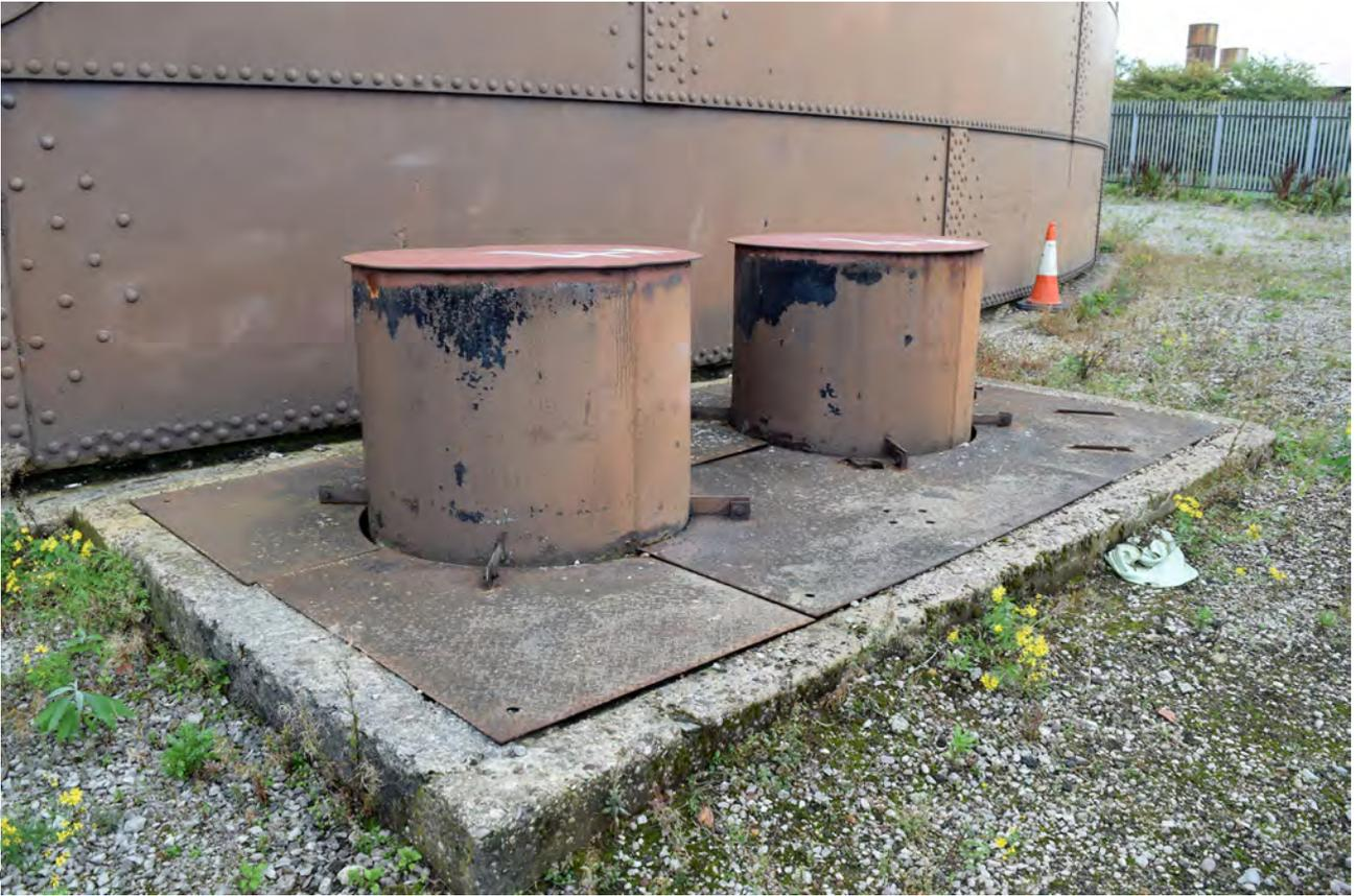
Plate 9: The cut-off remains of the inlet-outlet pipes at the south-west of Gasholder 3
