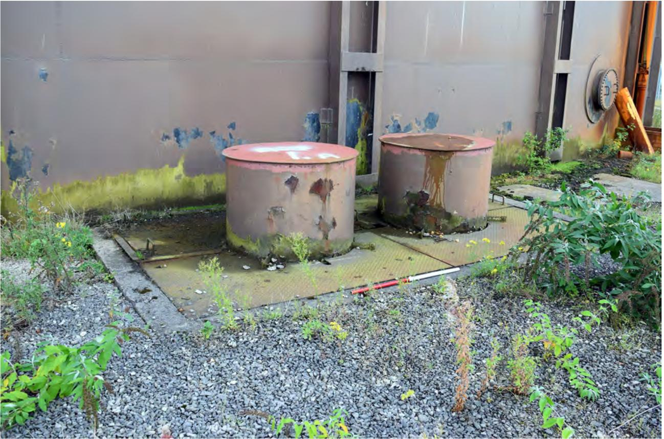
Plate 26: The cut-off remains of the inlet-outlet pipes at the north-west of Gasholder 4
