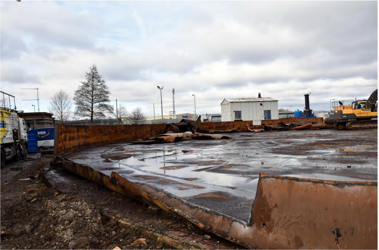
Plate 37: The partially demolished Gasholder 4
