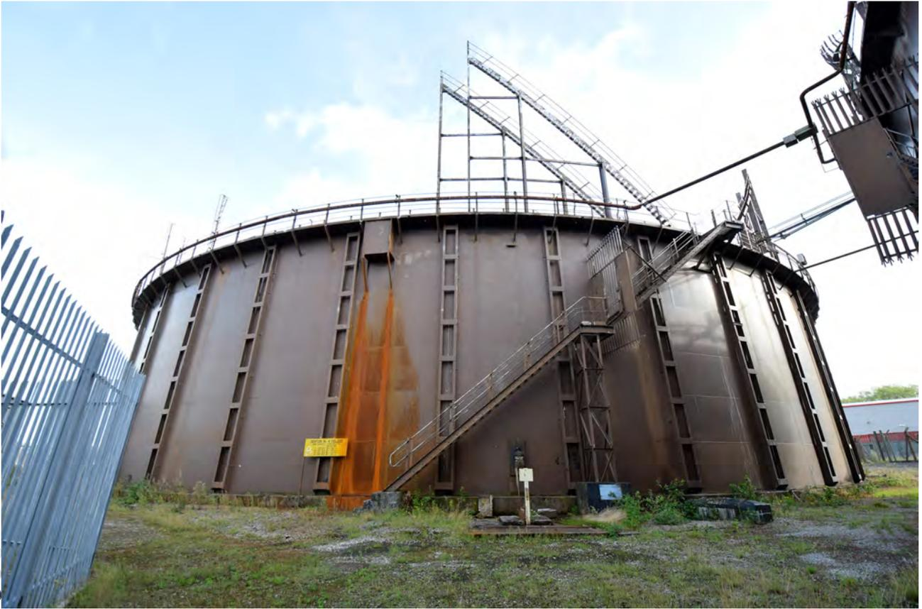
Plate 28: The staircase and lift steps of Gasholder 4
