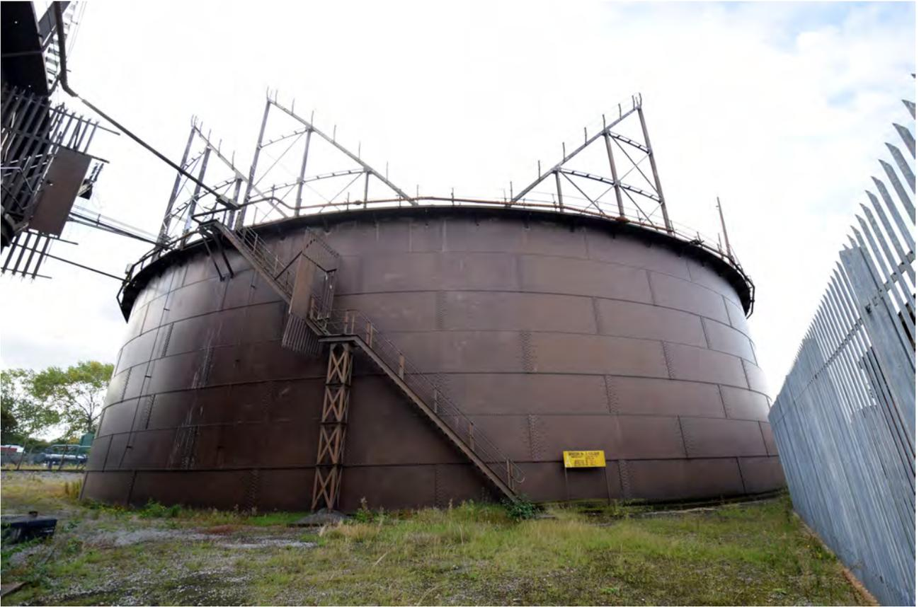
Plate 11: The staircase and lift steps of Gasholder 3
