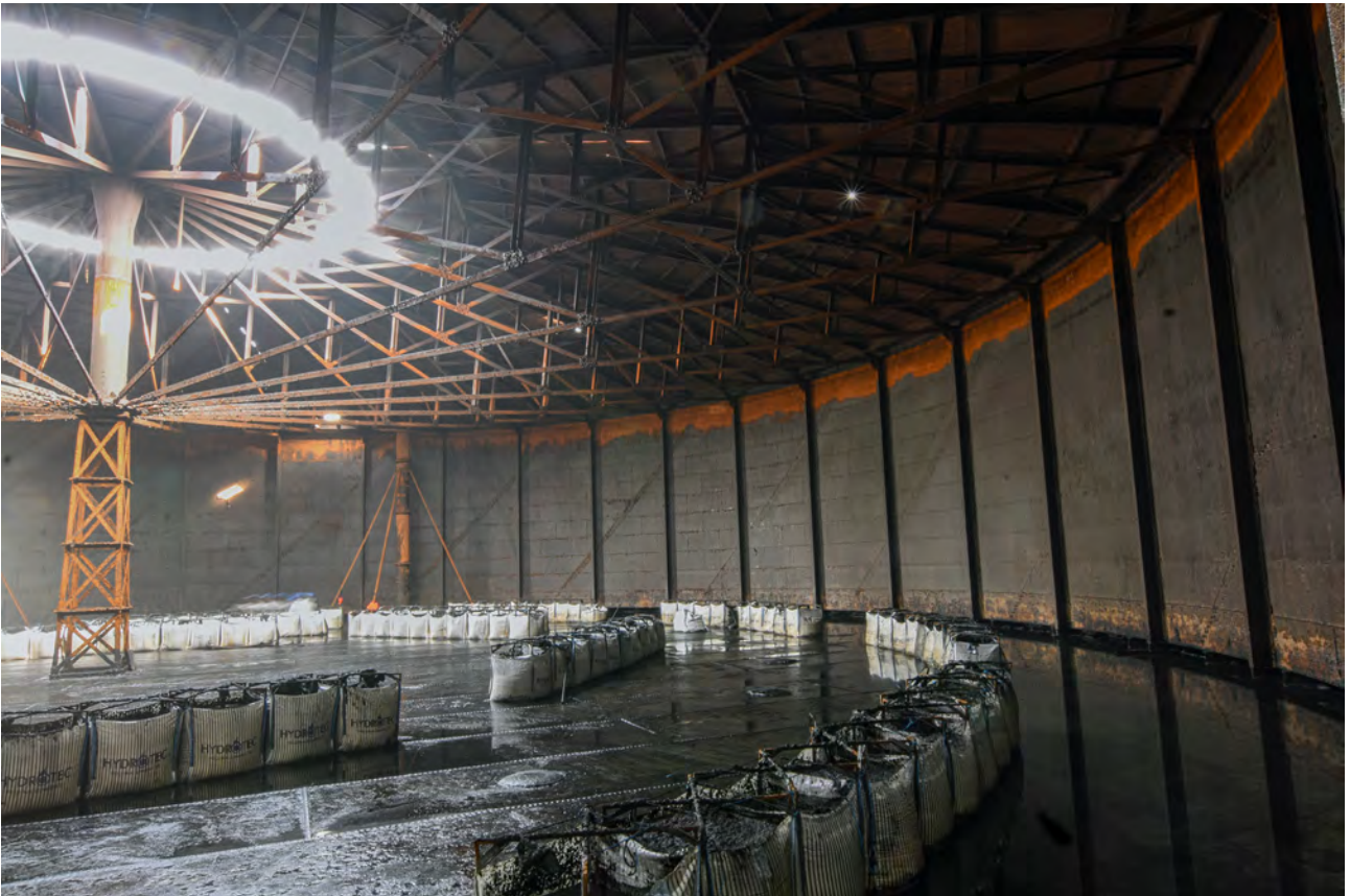
Plate 34: The columns supporting the crown structure of Gasholder 4
