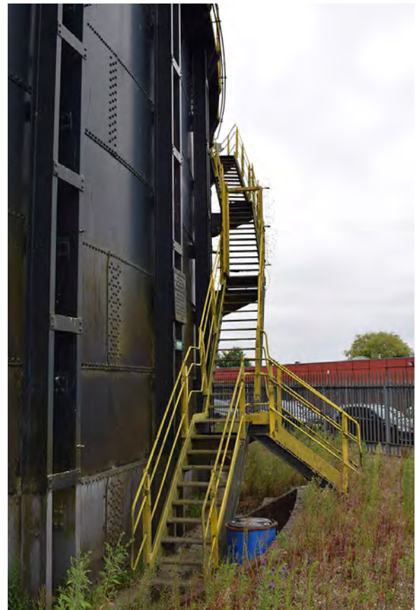
Plate 24: The staircase of Gasholder 4
