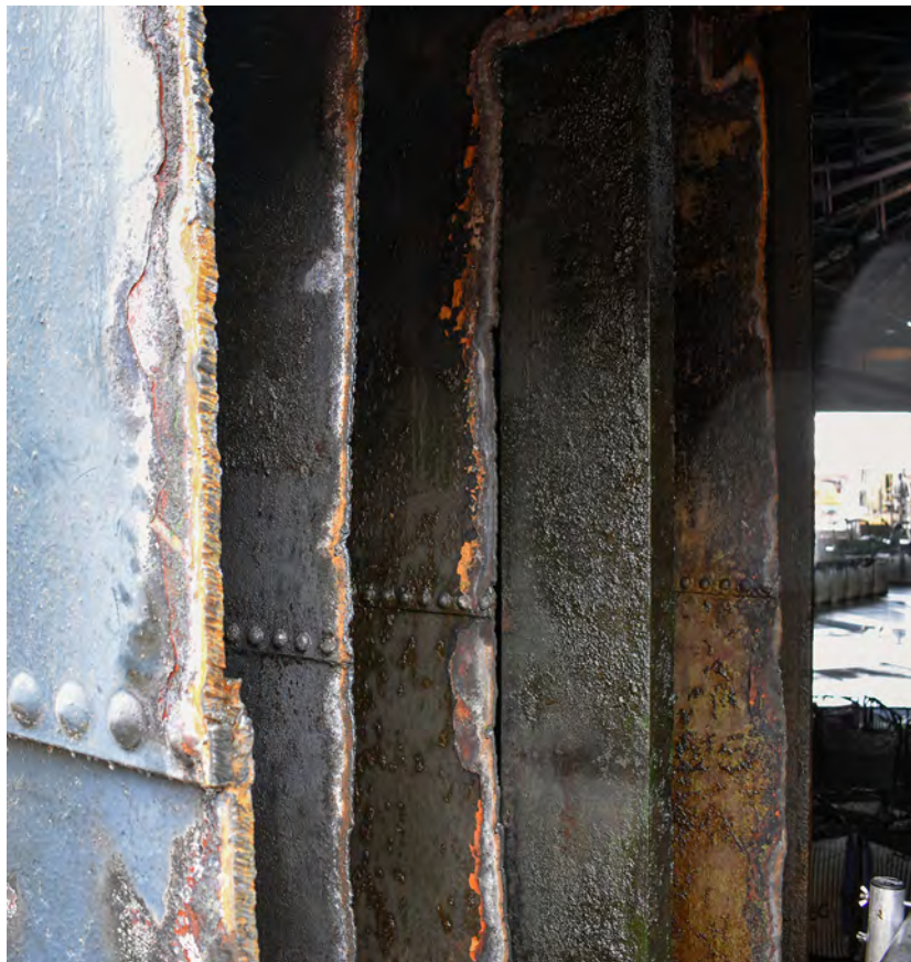
Plate 12: A cross-section of the tank and lifts of Gasholder 3
