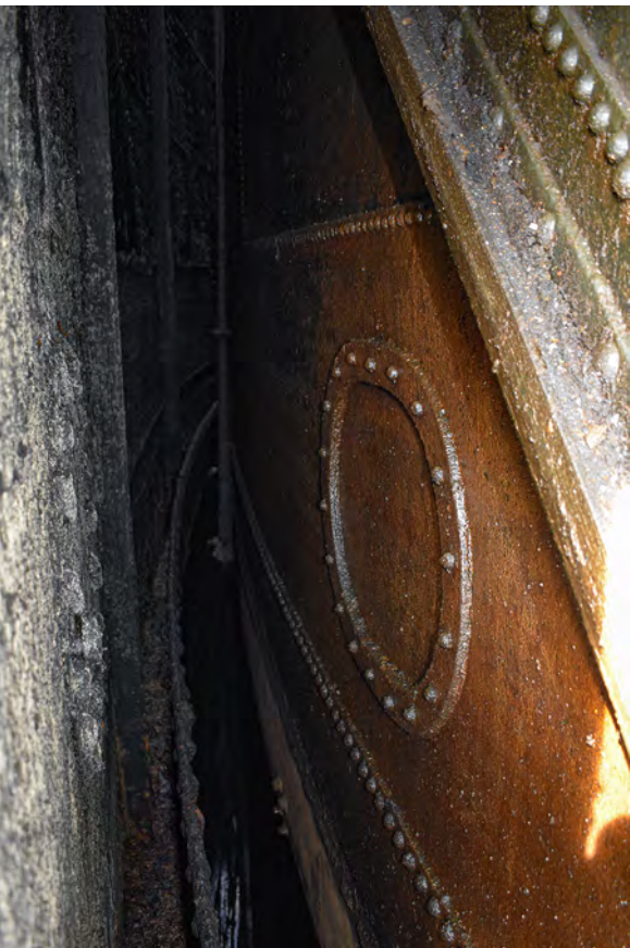
Plate 31: An example of a former access between the lifts of Gasholder 4
