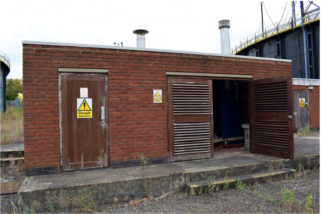
Plate 39: The west elevation of the control block
