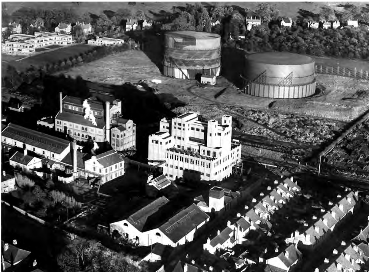
Plate 2: Aerial photo of the site taken between 1940-1952. National Gas Archive ref: AA1204P
