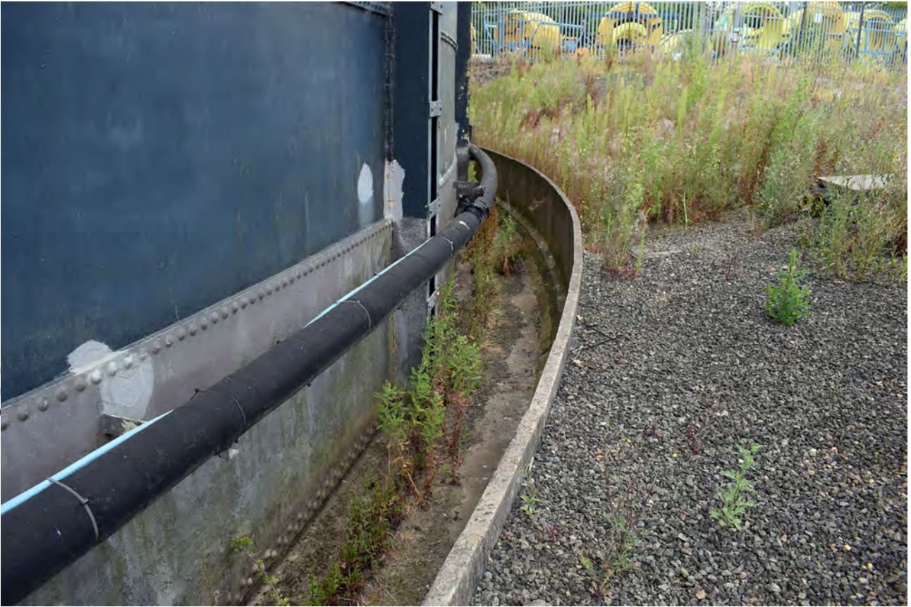
Plate 7: The bund surrounding Gasholder 3
