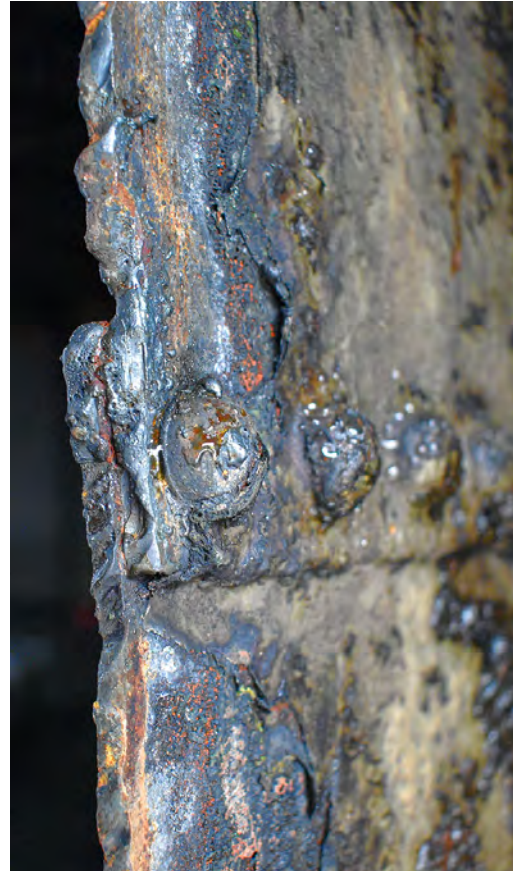
Plate 14: An example of the rivetted joint between steel plates of a lift in Gasholder 3
