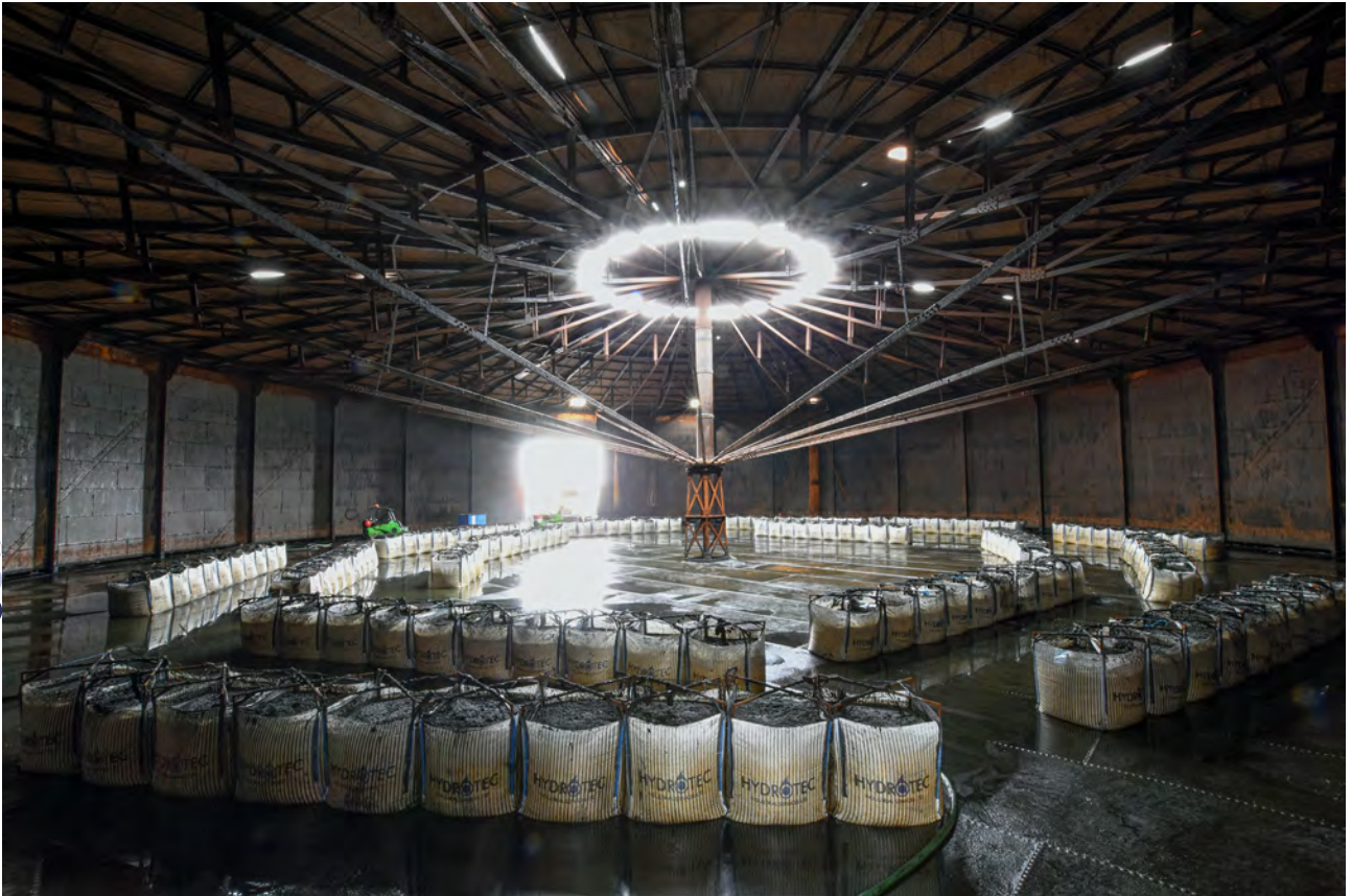
Plate 11: The interior of Gasholder 3, looking west
