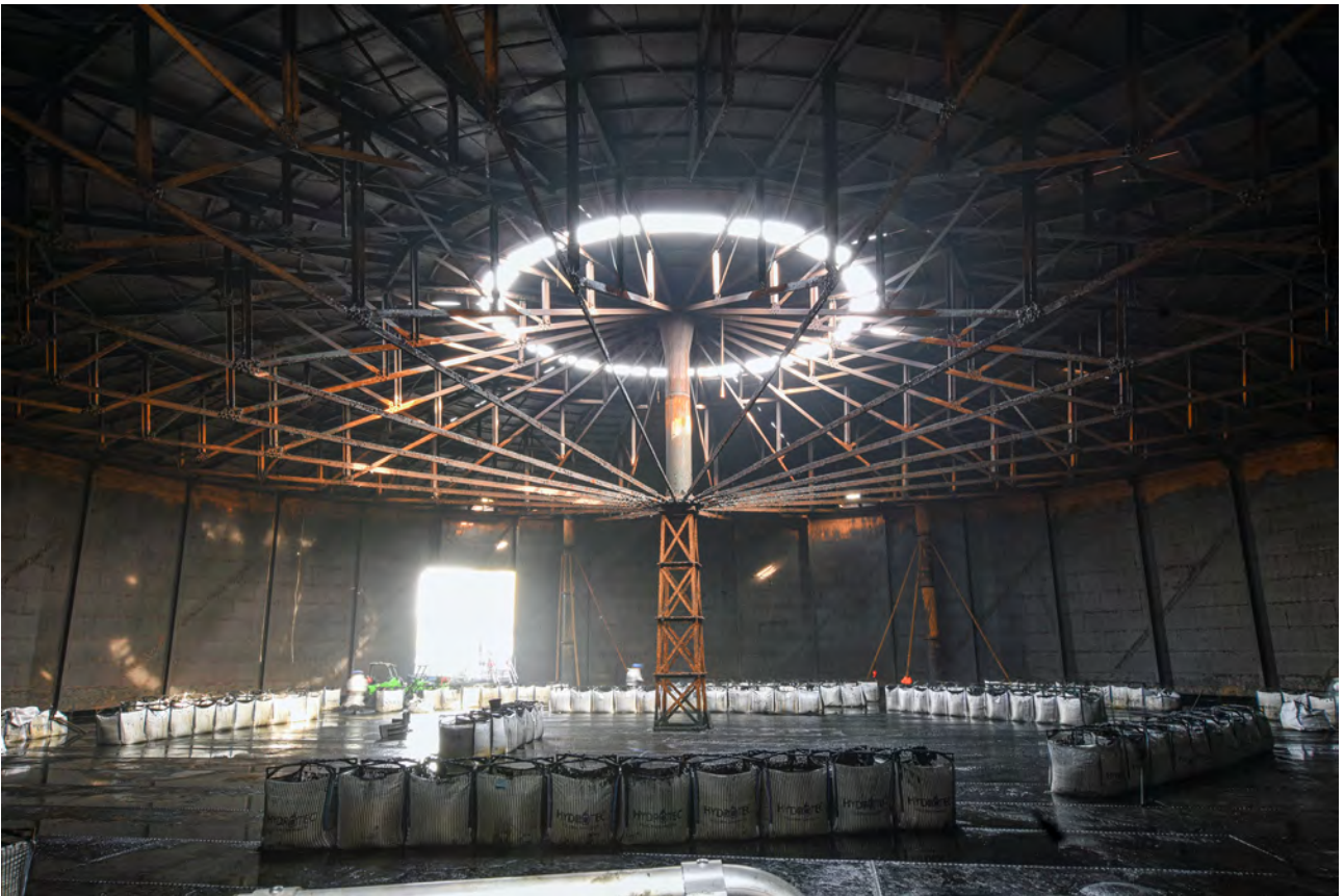
Plate 28: The interior of Gasholder 4, looking north
