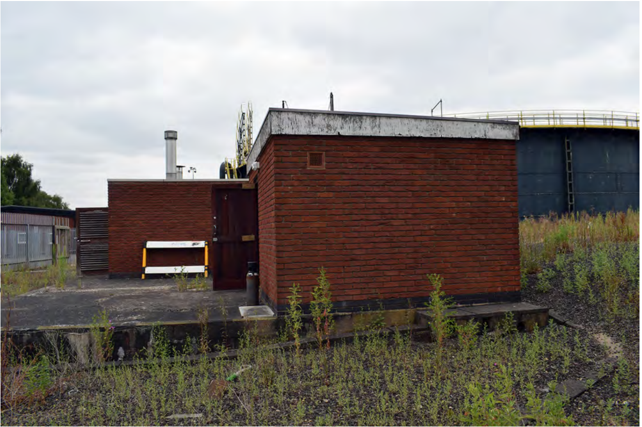
Plate 41: The south elevations of the ancillary buildings
