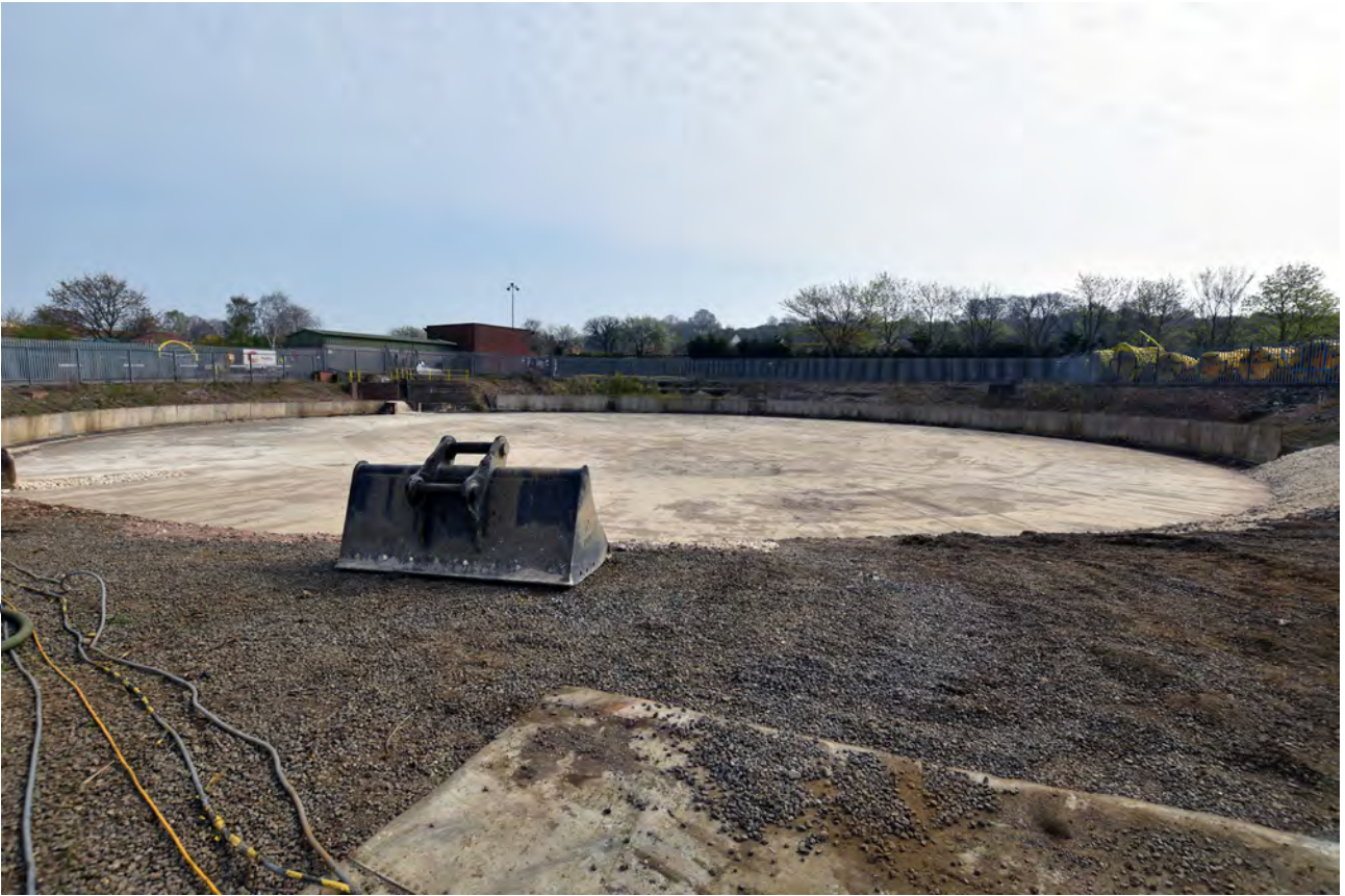
Plate 18: The concrete base of Gasholder 3 following the removal of the tank
