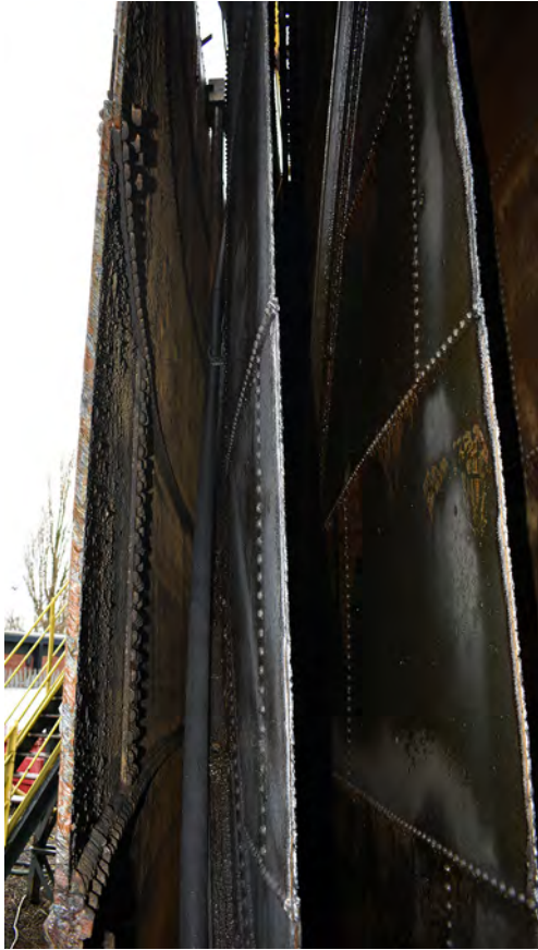
Plate 13: A cross-section of the tank and lifts of Gasholder 3
