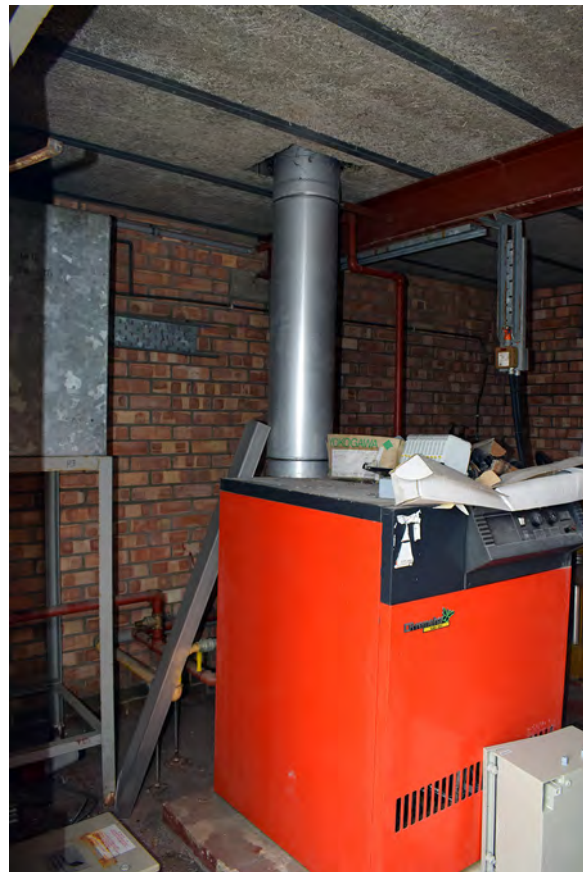
Plate 40: The interior of the boiler house
