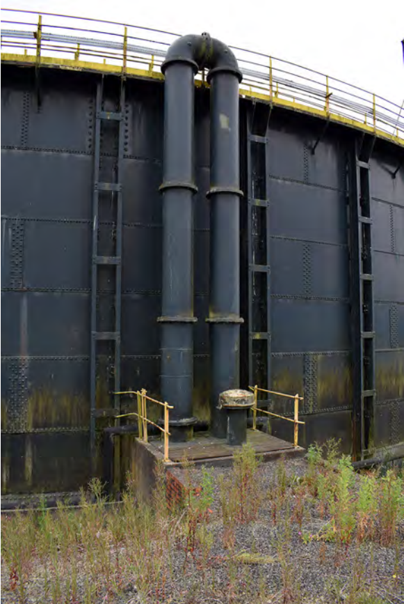
Plate 23: The inlet and outlet pipes at the north-east of Gasholder 4
