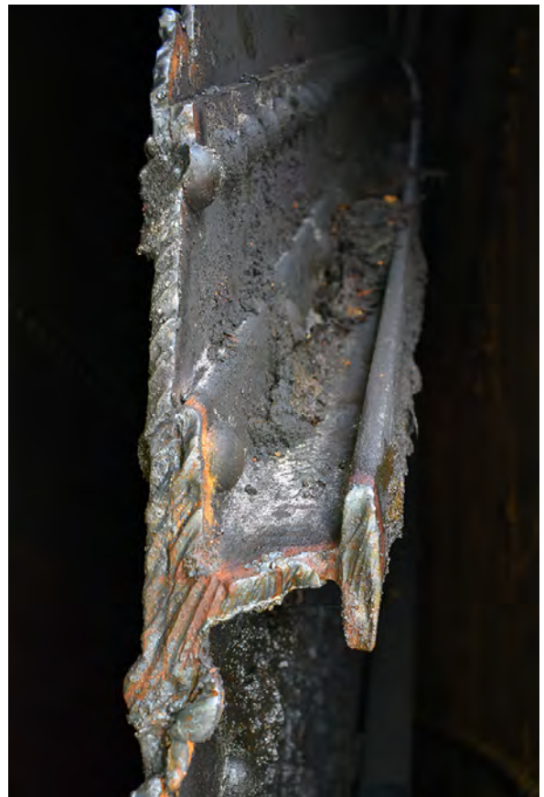
Plate 32: A cross-section of a guide of Gasholder 4
