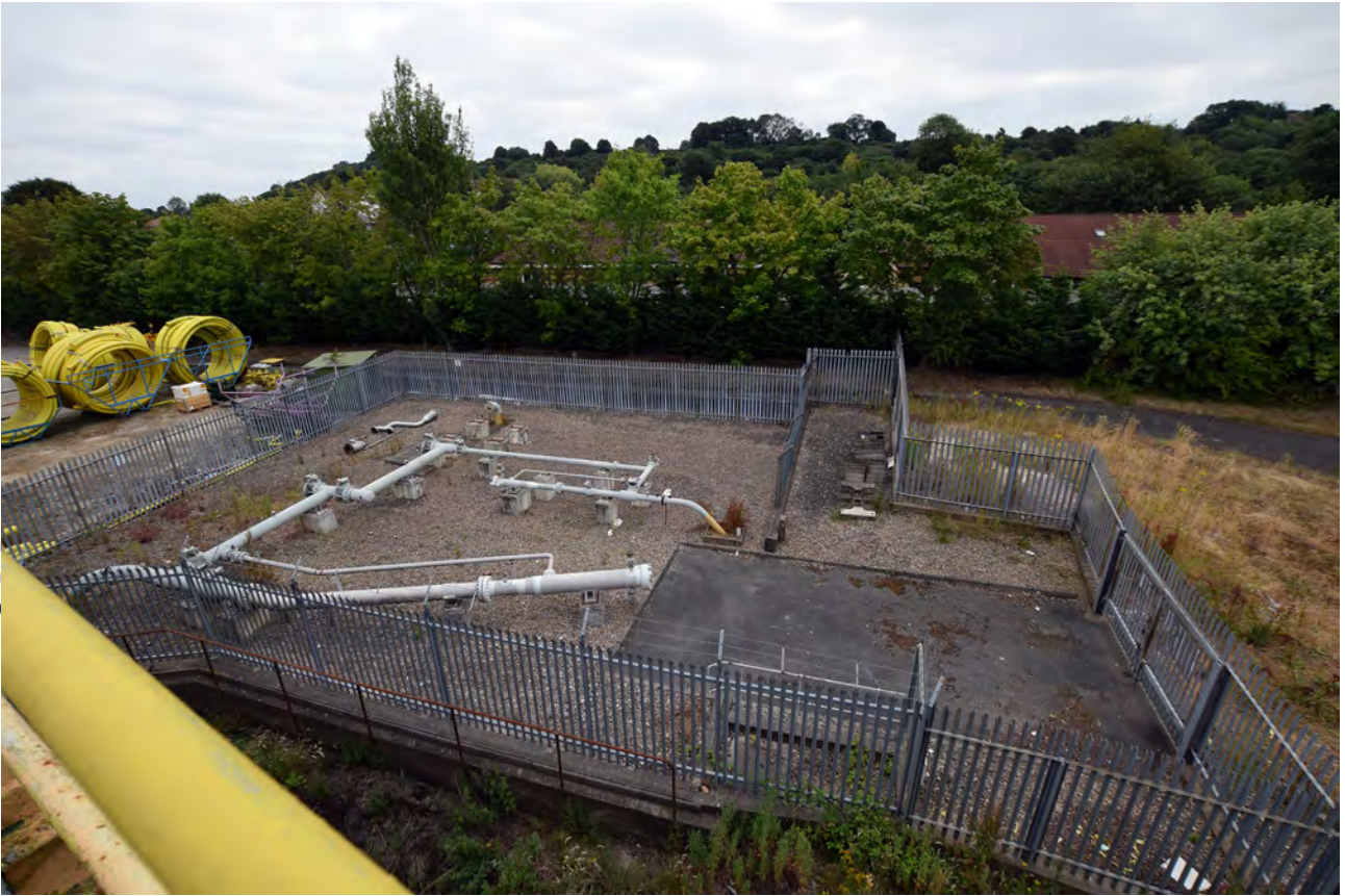
Plate 3: Distribution plant to the east of the gasholders
