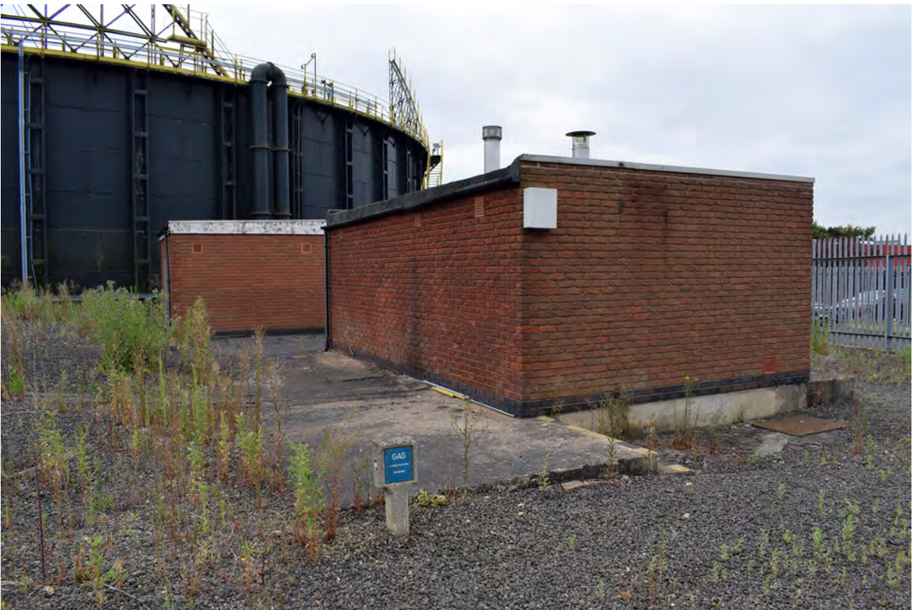
Plate 38: The two ancillary buildings in relation to Gasholder 4, looking south
