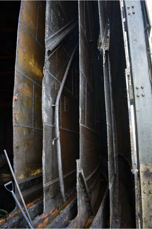
Plate 29: A cross-section of the tank and lifts of Gasholder 4
