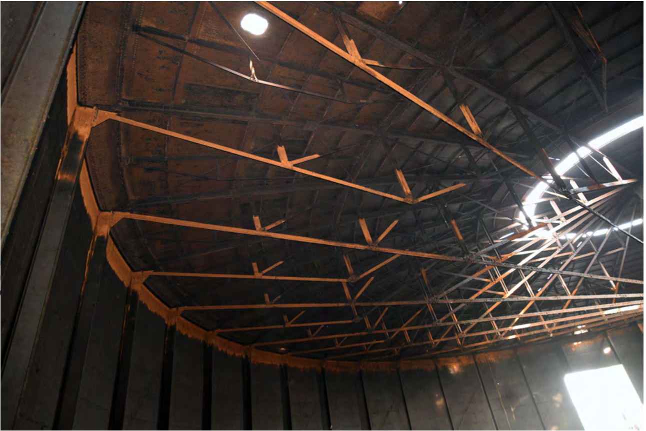
Plate 35: The crown structure of Gasholder 4
