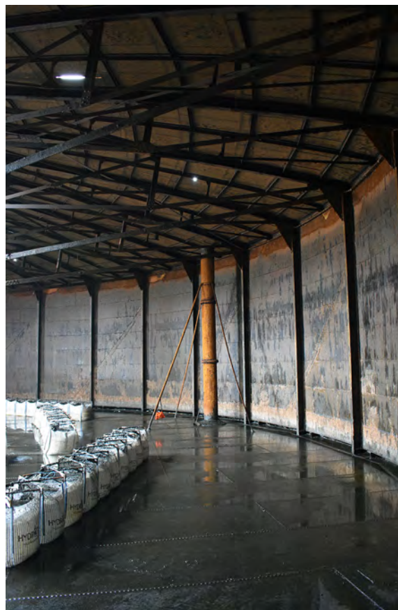
Plate 17: The remains of an inlet/outlet pipe in Gasholder 3
