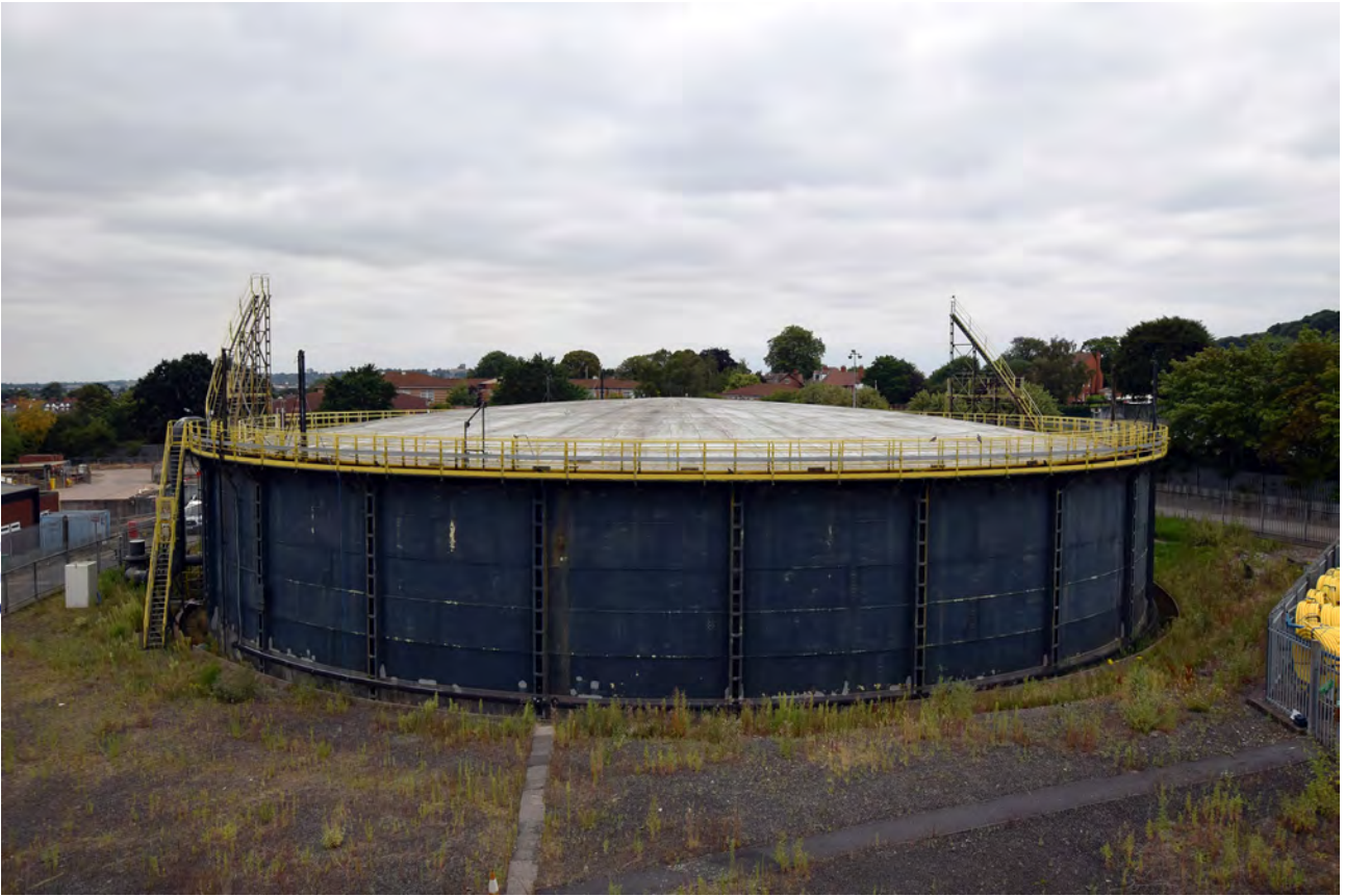
Plate 5: Gasholder 3 taken from the top of the tank of Gasholder 4, looking north
