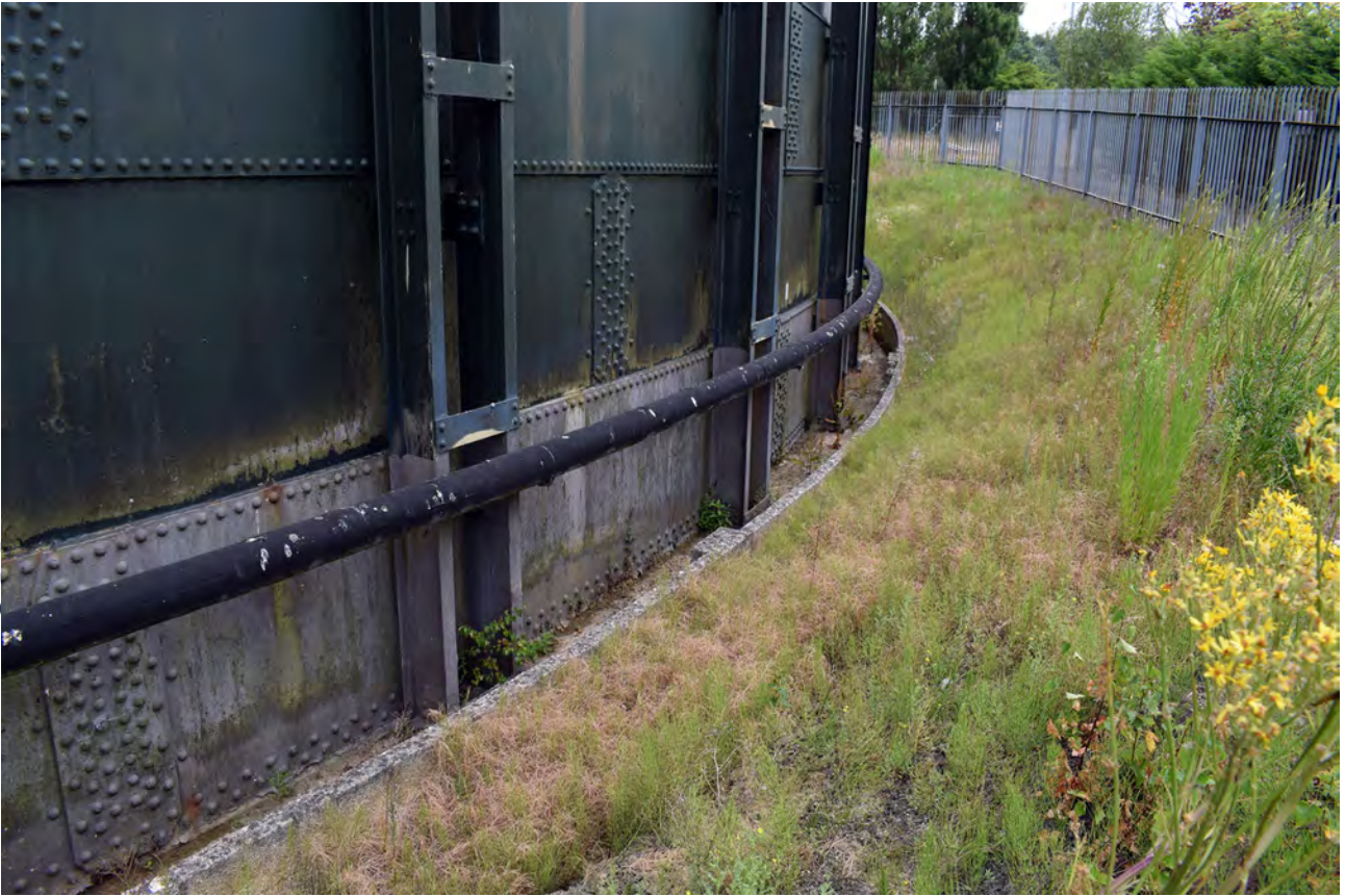
Plate 22: The bund surrounding Gasholder 4
