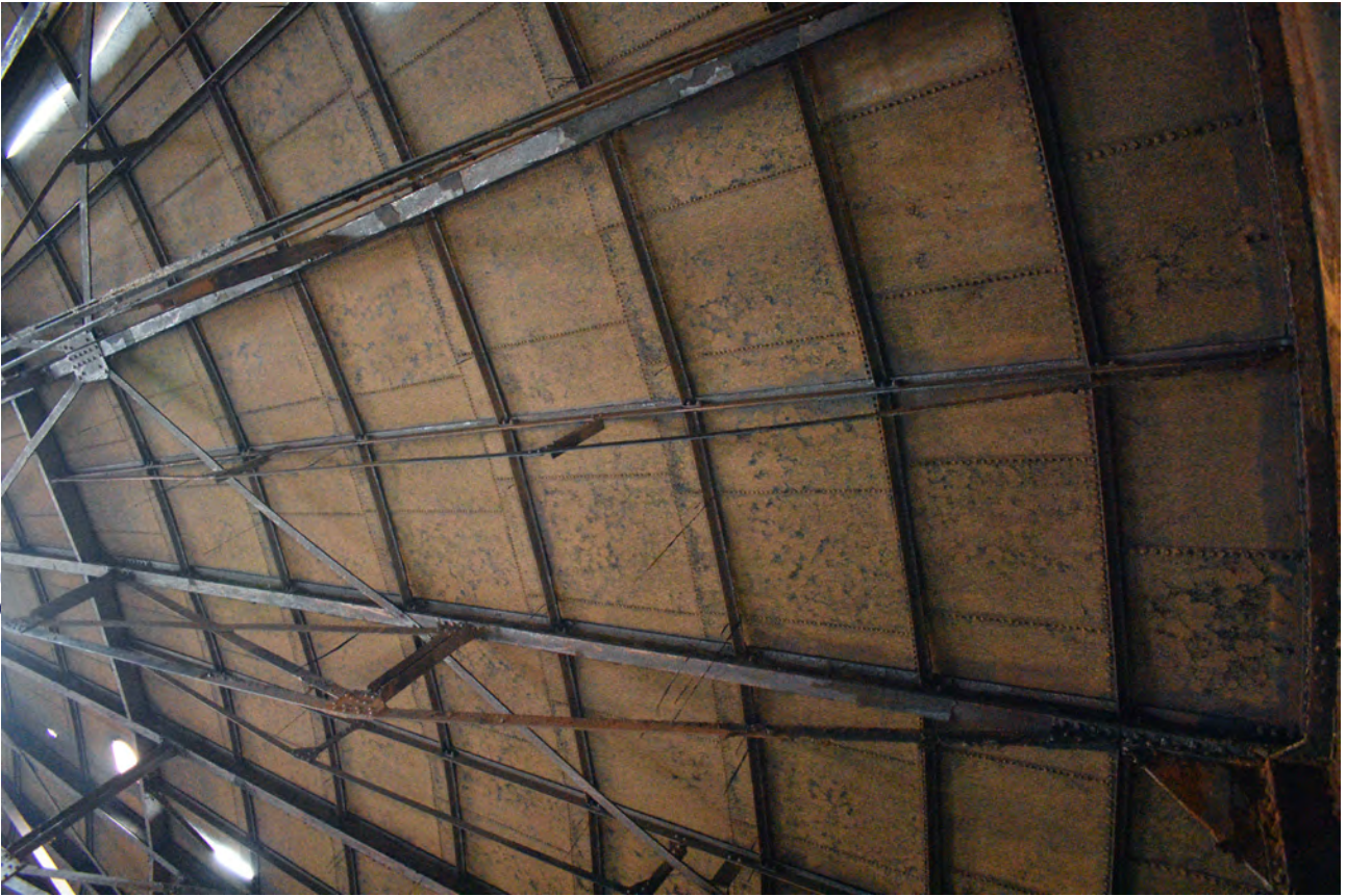
Plate 16: The crown structure of Gasholder 3
