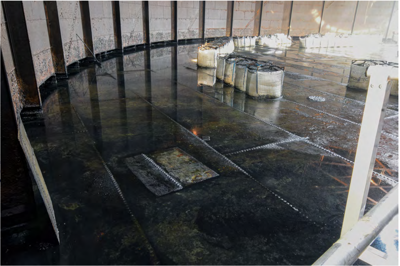
Plate 37: The floor of Gasholder 4 with a removed section of the crown
