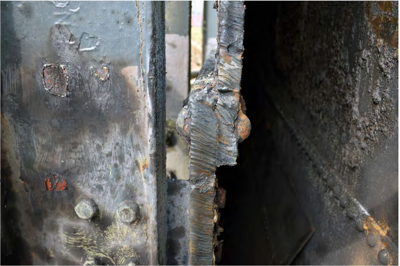
Plate 33: An example of the rivetted joint between plates of the tank of Gasholder 4
