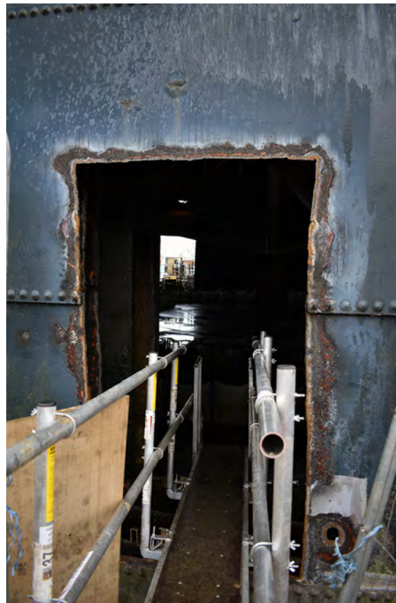
Plate 10: The east cutting through the tank and lifts of Gasholder 3
