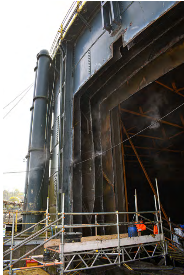
Plate 27: The north-west cutting through the tank and lifts of Gasholder 4
