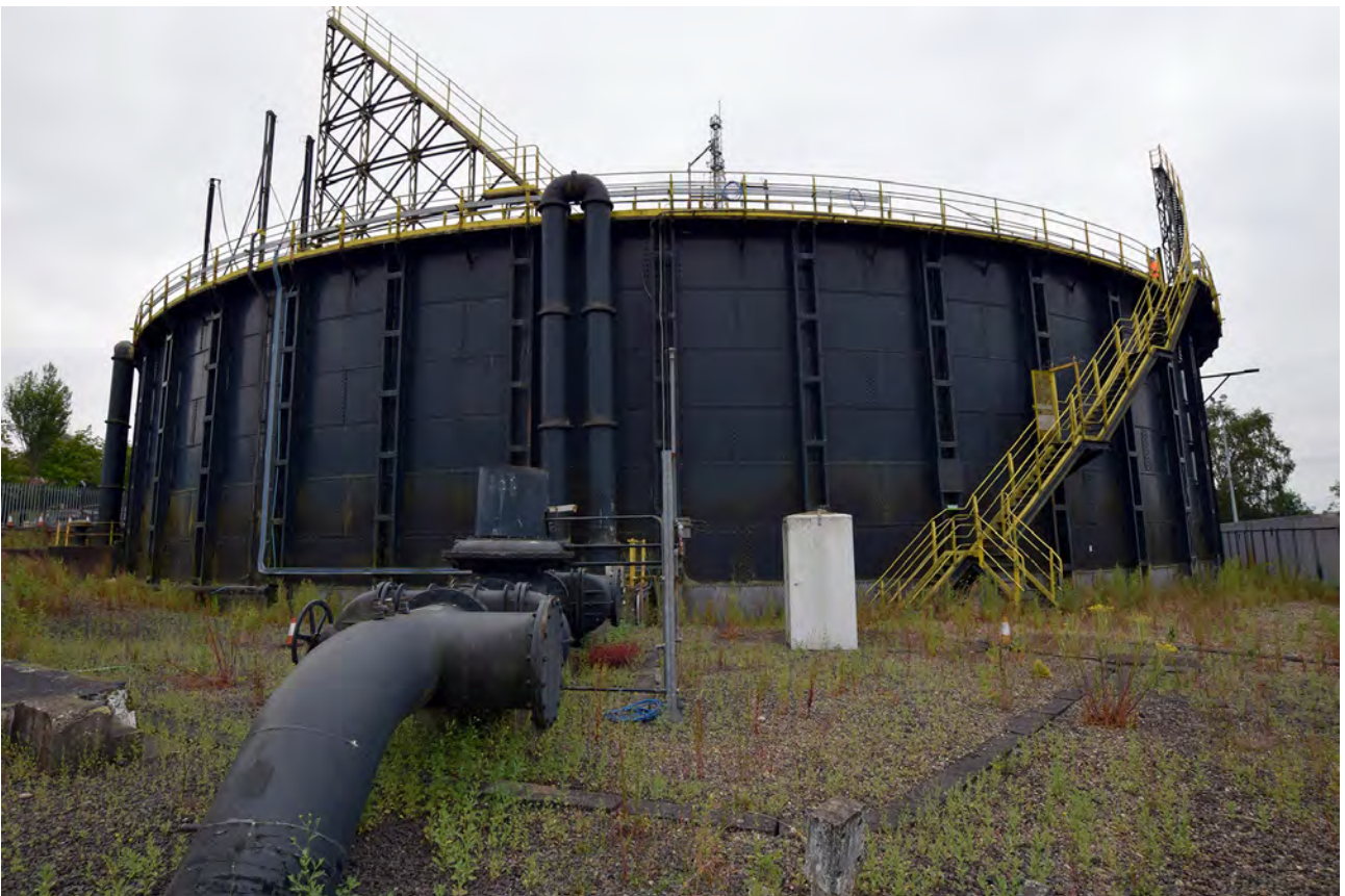
Plate 19: Gasholder 4, looking south
