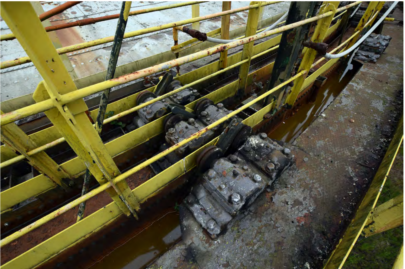
Plate 26: An example of the roller carriages of Gasholder 4
