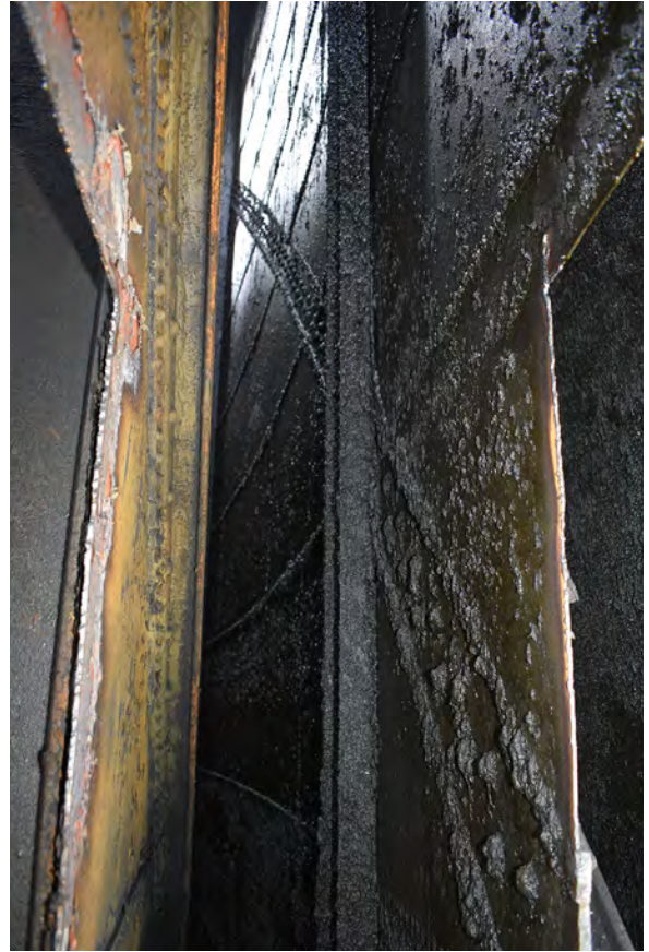
Plate 30: A cross-section of the lifts of Gasholder 4
