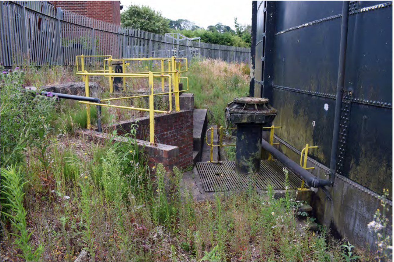
Plate 9: The blanked-off pipe at the north of Gasholder 3
