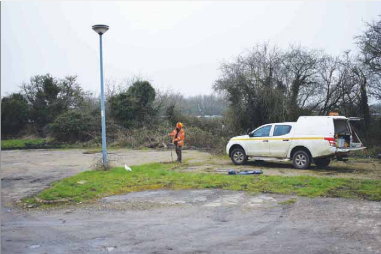
Plate 4: Drilling borehole WS13, looking south
