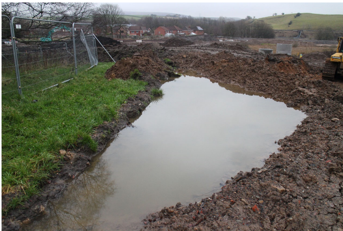
Plate 1: An example of adverse ground conditions during fieldwork.
