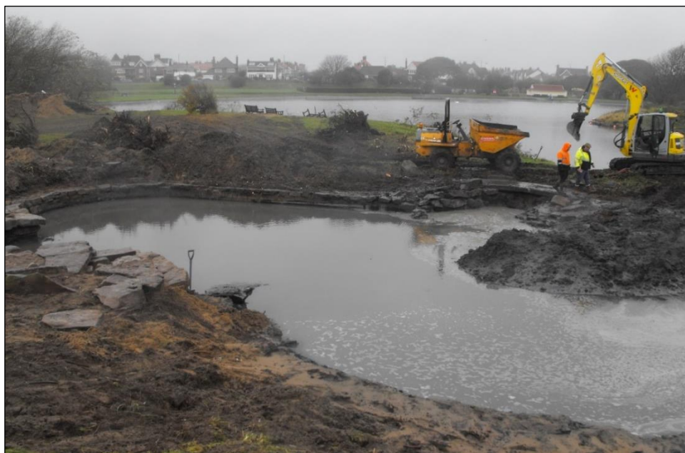
Plate 5: North side of the lagoon with bridge 108 and Fairhaven Lake behind and ‘outcrop’ rockery 107 to the left of the image
