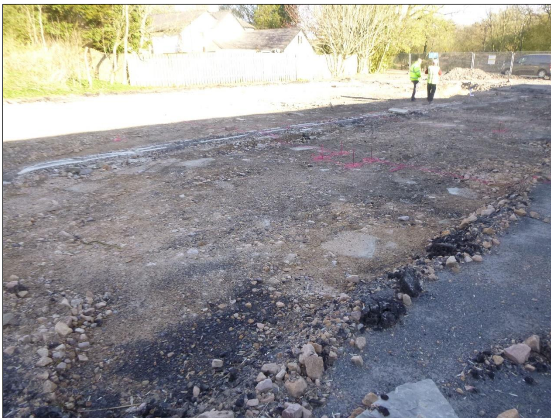
Plate 1: Site following removal of tarmacadam 1000 , looking north-west
