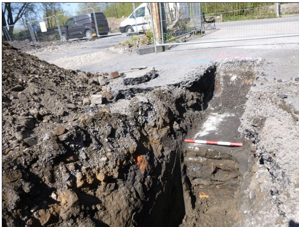
Plate 4: Wall foundation 306, looking north-west, scale 0.5m
