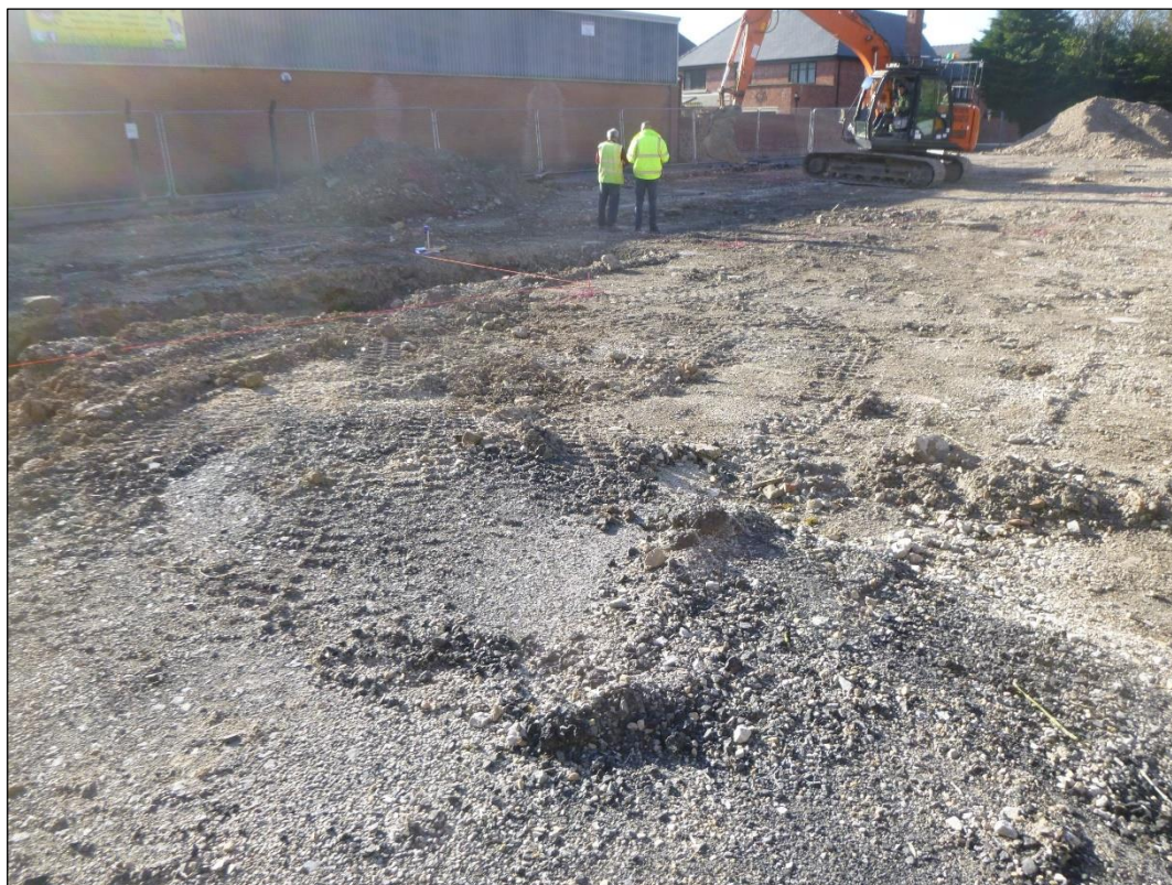
Plate 2: Site following the removal of tarmacadam 1000, looking south-east
