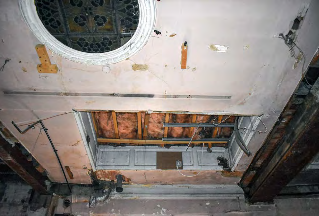
Plate 35: Ceiling in the ground floor of 31 Cornmarket Street, looking north
