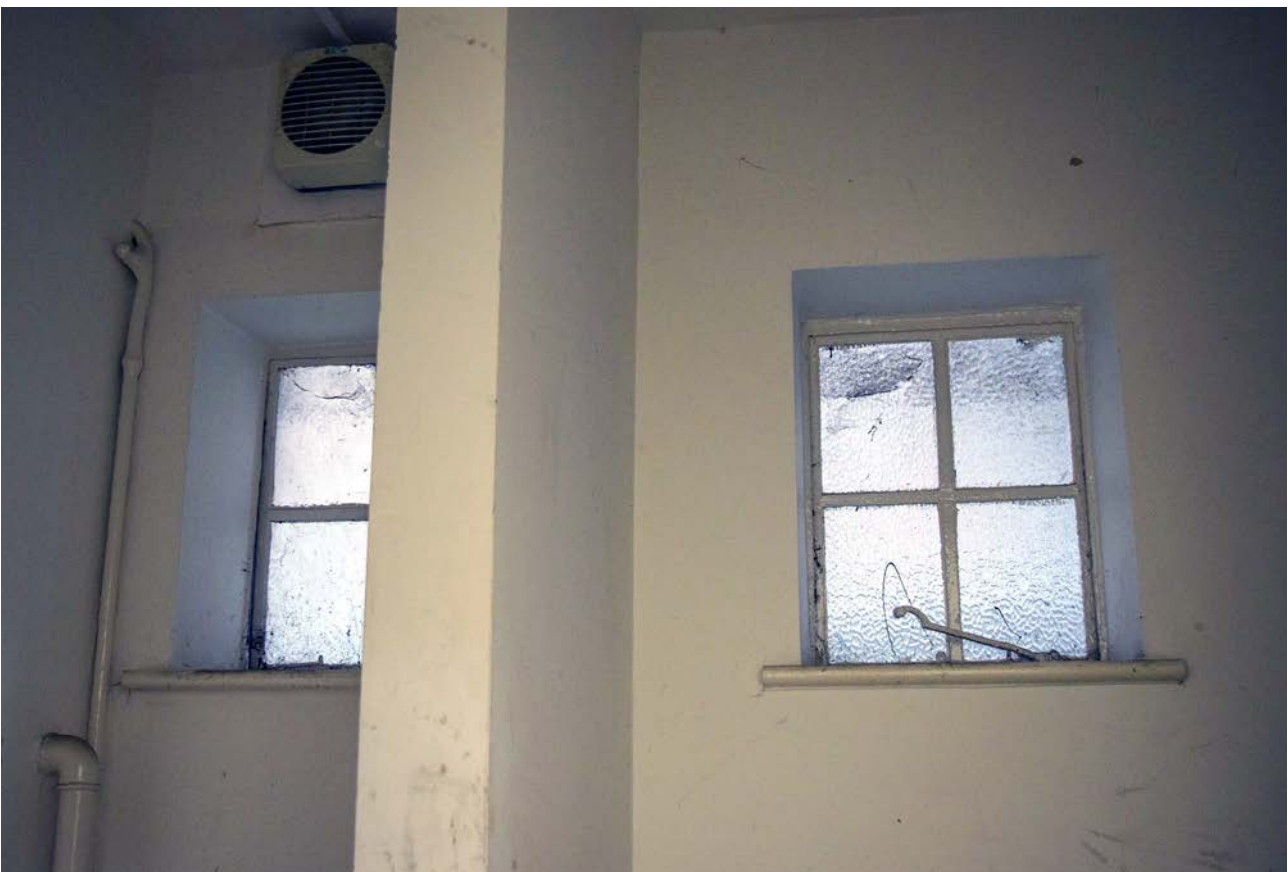
Plate 116: The half landing room between the ground and first floor of Oxford Language School, looking south
