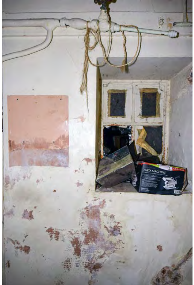
Plate 14: WC in the basement of 1 to 5 Broad Street, looking south
