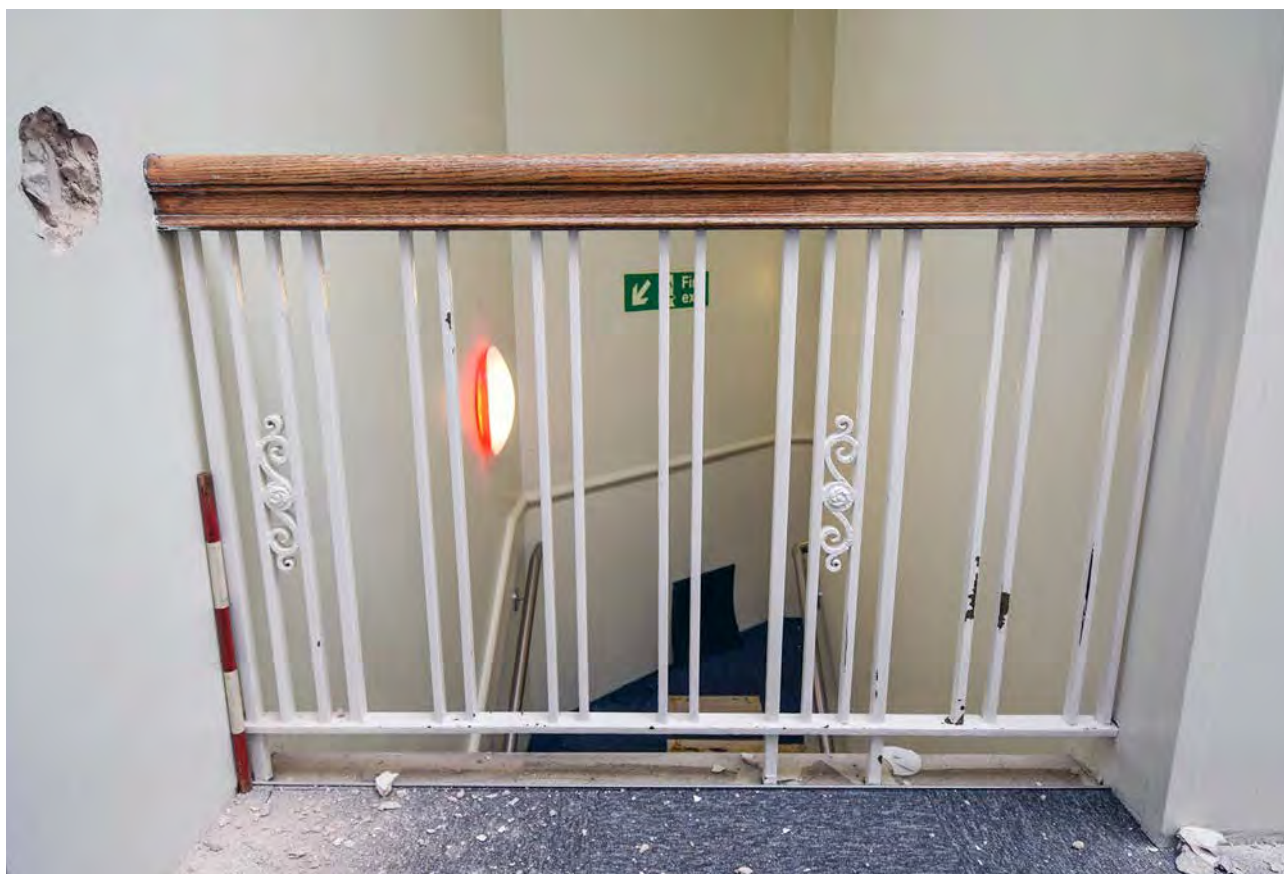
Plate 136: The fourth floor landing of Oxford Language School, looking south
