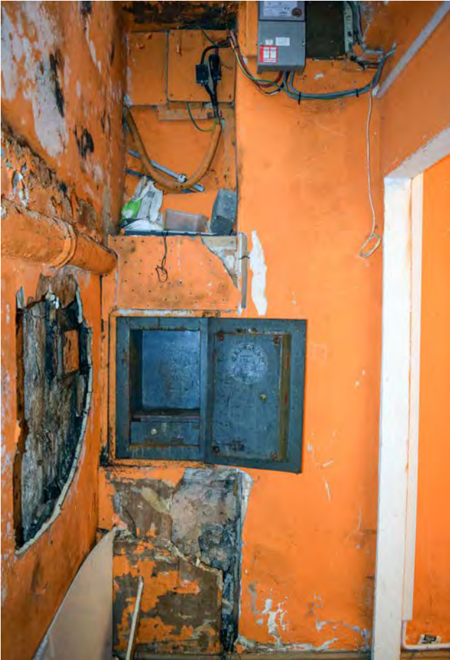
Plate 109: The basement of no. 4 Broad Street, looking east
