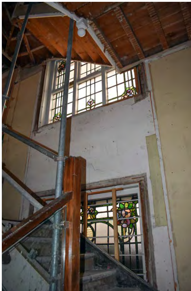
Plate 32: Windows in the stairway of 31 Cornmarket Street, looking south-east
