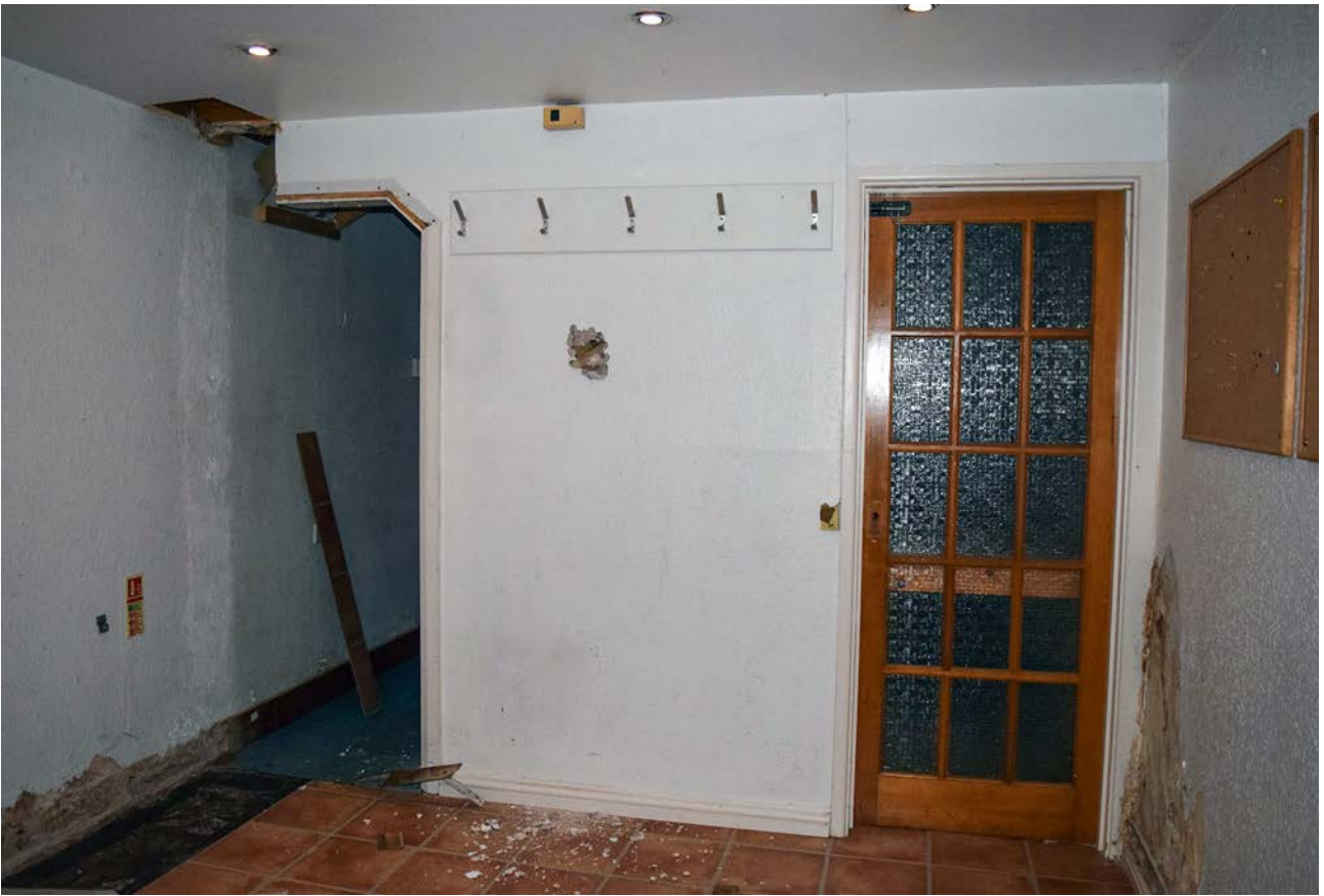
Plate 112: The basement of no. 5 Broad Street, looking north
