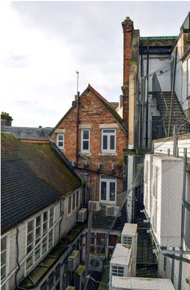
Plate 2: The lightwell between Boswells and the building occupied by Waterstones, looking west
