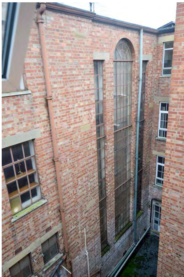
Plate 4: The central lightwell in 1 to 5 Broad Street, looking south-west
