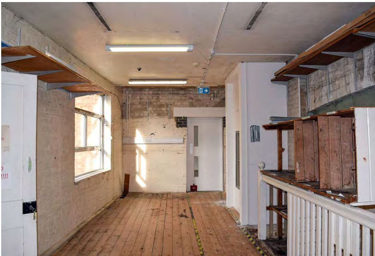
Plate 90: The third floor of 31 Cornmarket Street, looking north
