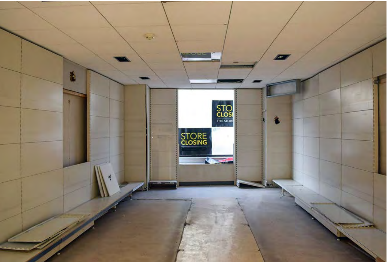
Plate 53: The first floor of 31 Cornmarket Street, looking west
