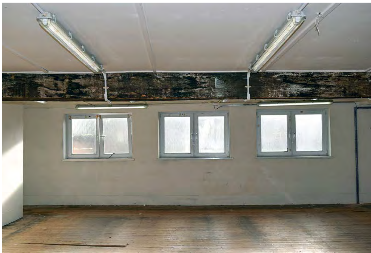
Plate 96: The third floor of 1 to 5 Broad Street, looking south-east
