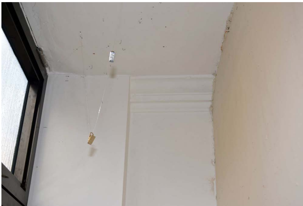
Plate 58: Cornice on the north side of the window opening in the second floor of 31 Cornmarket Street, looking north
