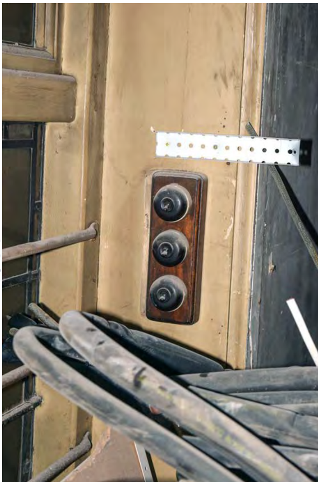
Plate 31: Light switches in the ground floor of 31 Cornmarket Street, looking west
