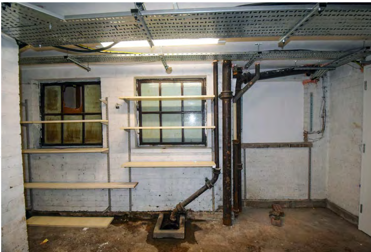
Plate 20: The basement of 1 to 5 Broad Street, looking west
