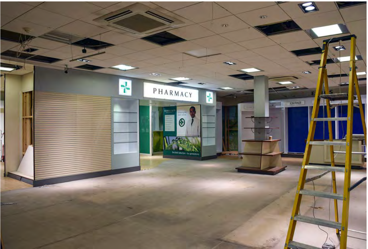
Plate 43: The ground floor of 1 to 5 Broad Street, looking south-east
