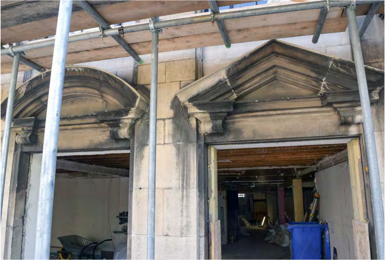
Plate 1: Window openings in the north facing elevation of Boswells
