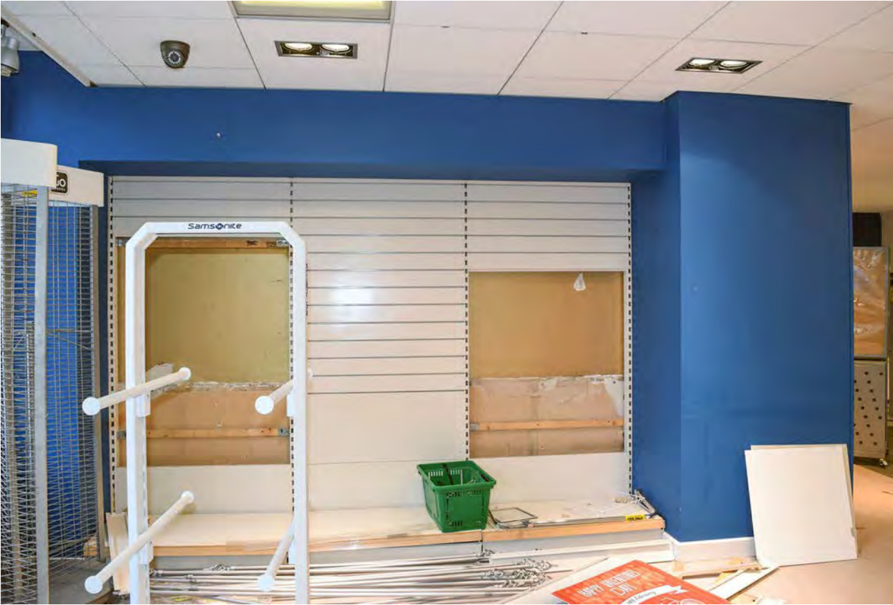
Plate 66: Gold paintwork behind modern panelling in the first floor of 1 to 5 Broad Street, looking east
