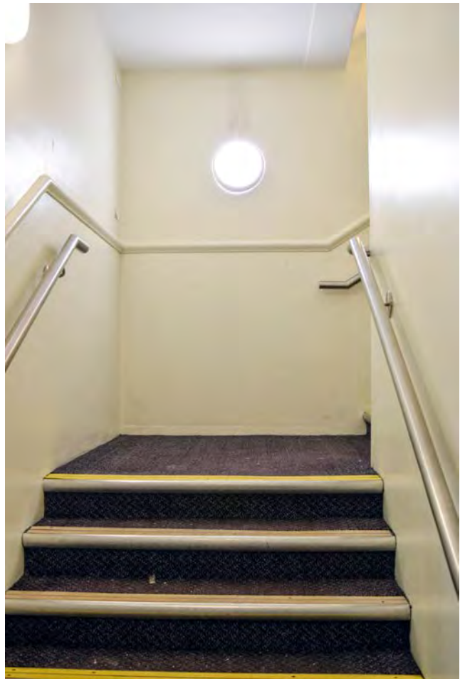
Plate 115: The stairway from the ground floor to the first floor in Oxford Language School, looking east
