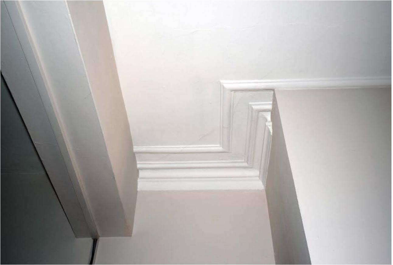
Plate 71: The second floor of 31 Cornmarket Street, looking south
