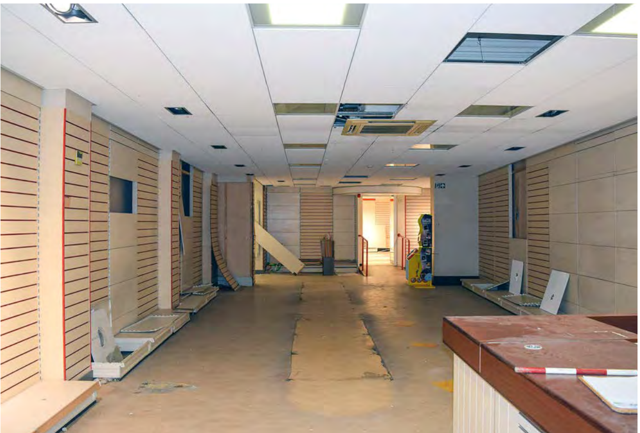
Plate 54: The first floor of 31 Cornmarket Street, looking east
