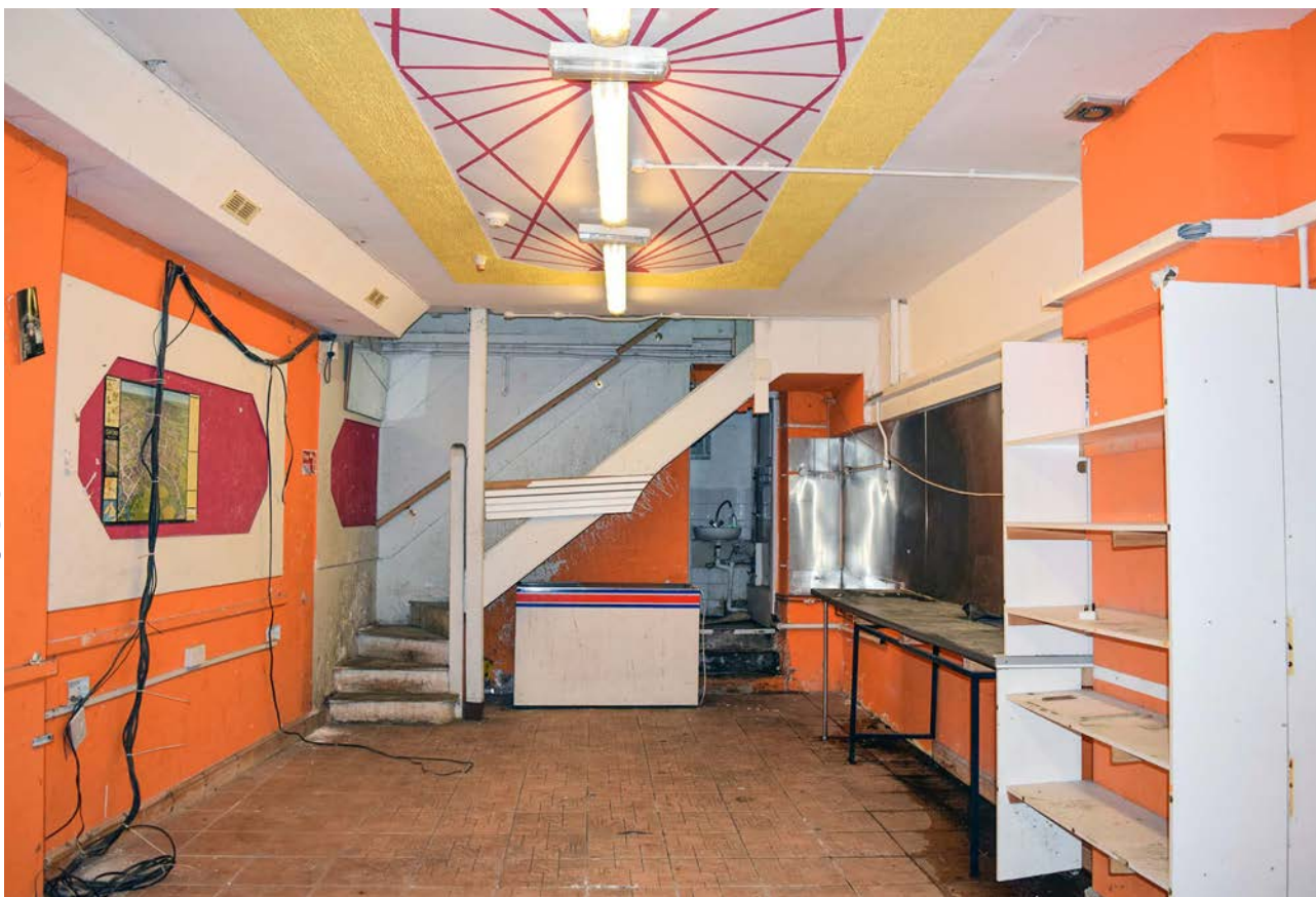
Plate 107: The basement of no. 4 Broad Street, looking south
