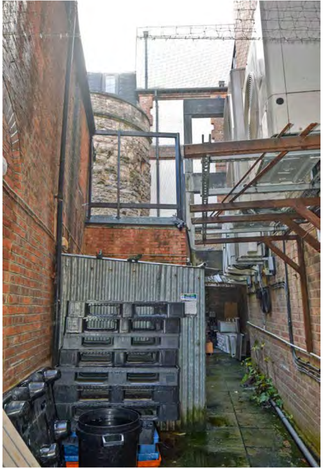
Plate 51: The alleyway on the east side of Boswells, where the bastion of Oxford City Walls can be viewed, looking south
