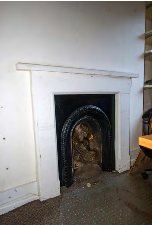
Plate 72: The second floor of 31 Cornmarket Street, looking north-east
