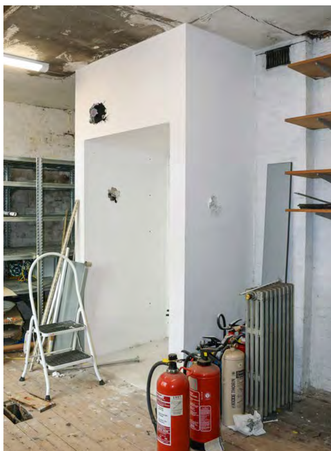
Plate 103: The fourth floor of 31 Cornmarket Street, looking north-east
