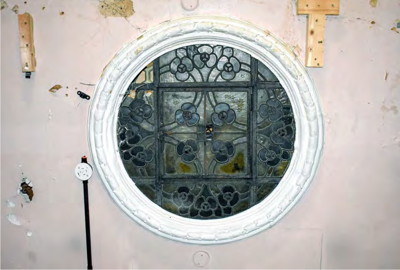
Plate 34: Ceiling in the ground floor of 31 Cornmarket Street
