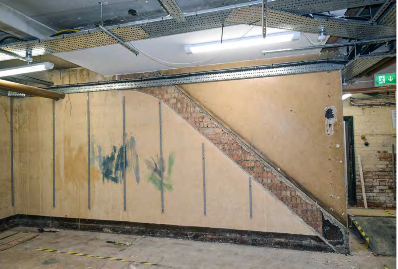
Plate 22: The basement of 1 to 5 Broad Street, looking south-west
