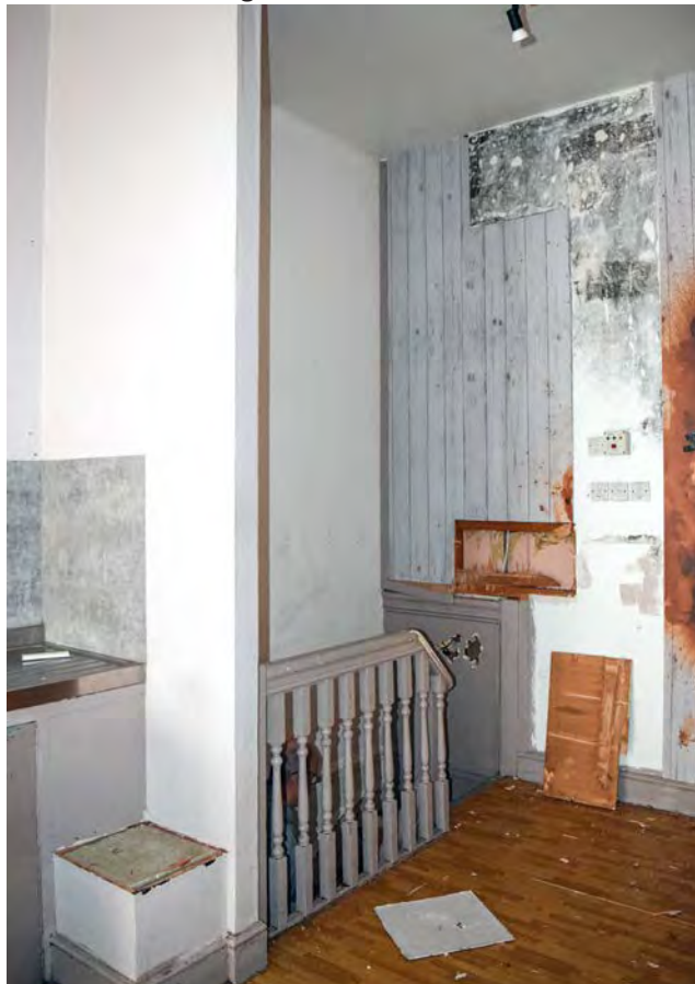
Plate 111: The ground floor of no. 5 Broad Street, looking south-east
