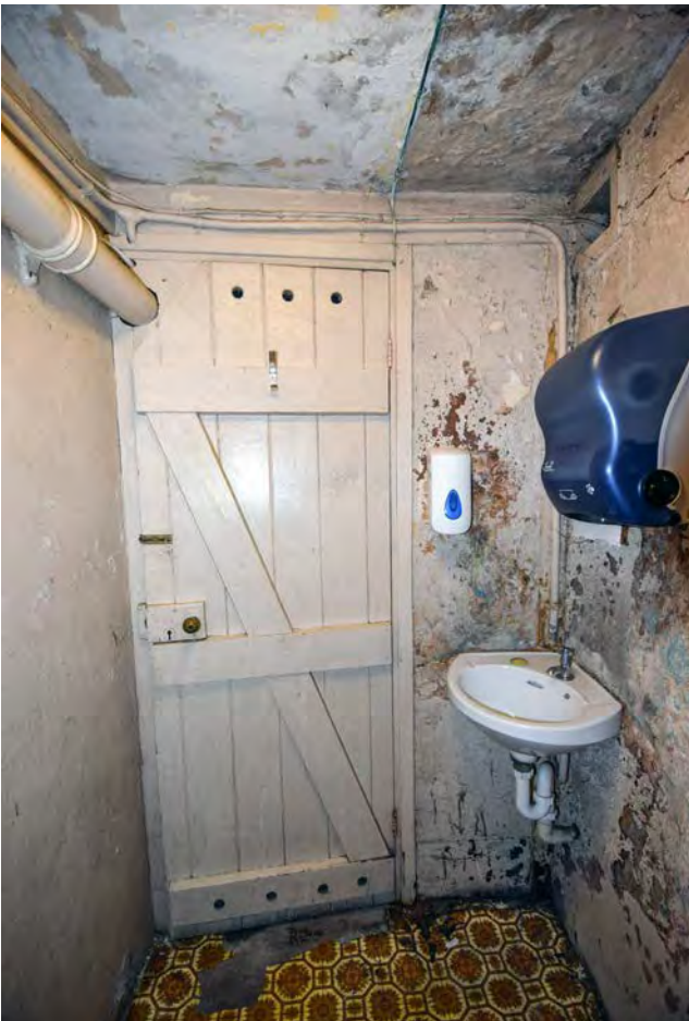
Plate 23: WC in the basement of 1 to 5 Broad Street, looking east
