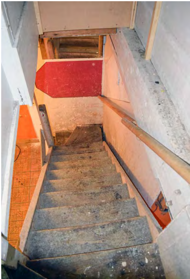
Plate 106: The stairway between the ground floor and basement of no. 4 Broad Street, looking north
