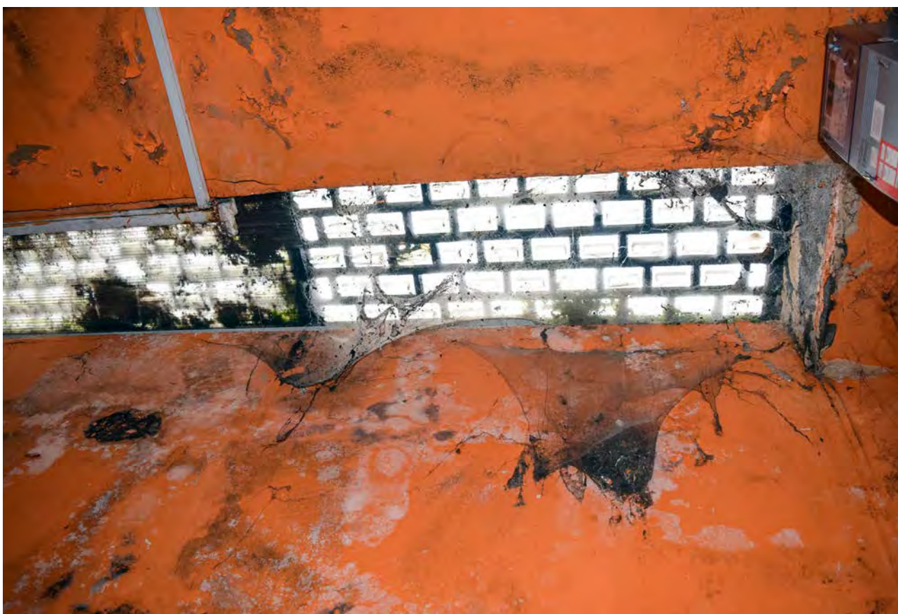
Plate 108: The basement of no. 4 Broad Street, looking north
