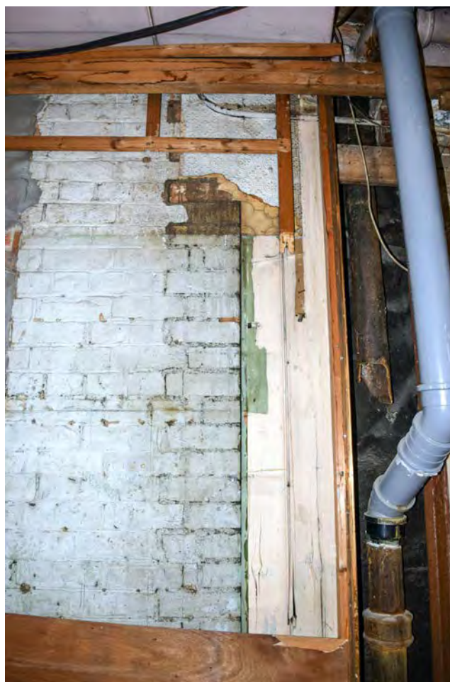
Plate 28: The ground floor of 31 Cornmarket Street, looking south
