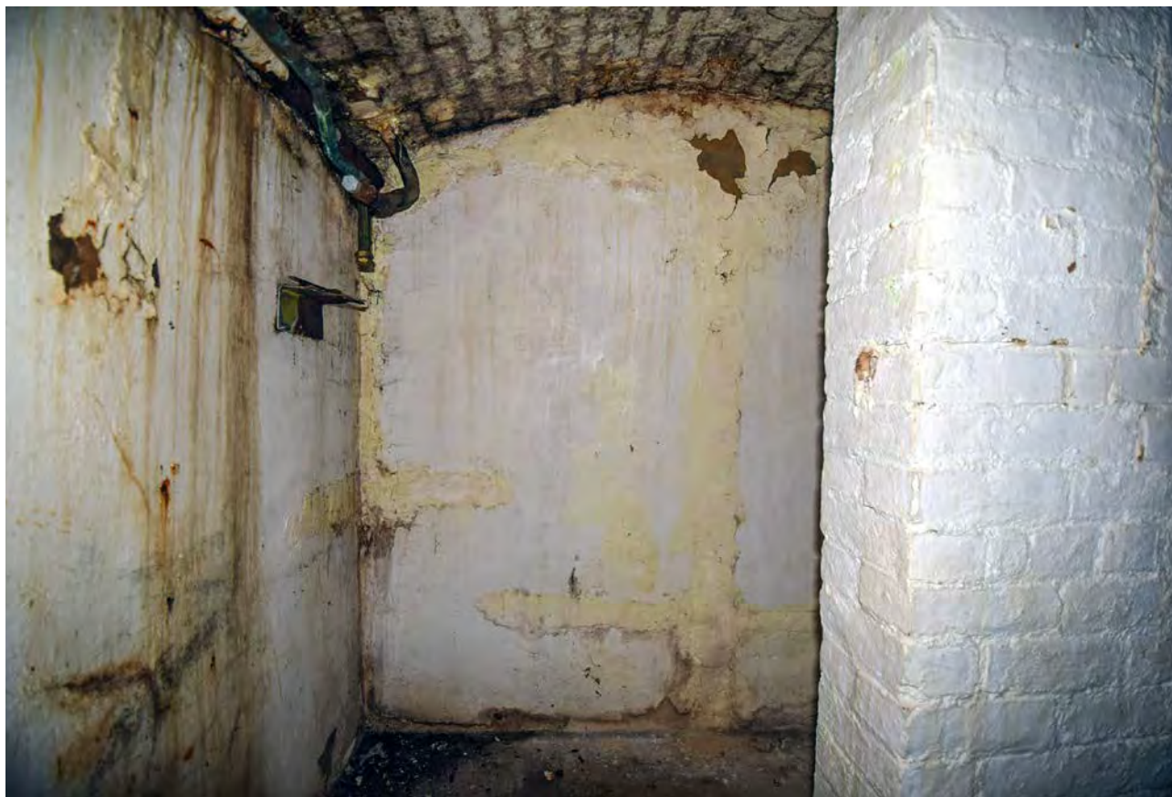
Plate 11: The basement of 31 Cornmarket Street, looking west
