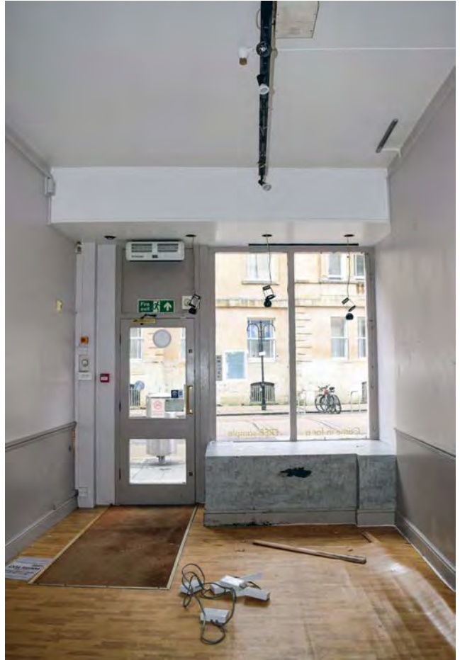
Plate 110: The ground floor of no. 5 Broad Street, looking north
