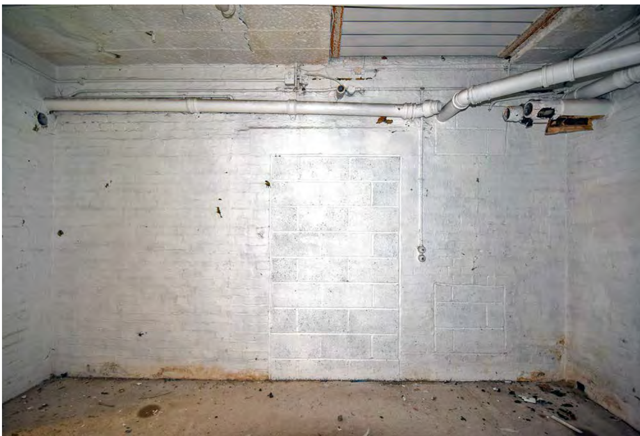
Plate 21: The basement of 1 to 5 Broad Street, looking west
