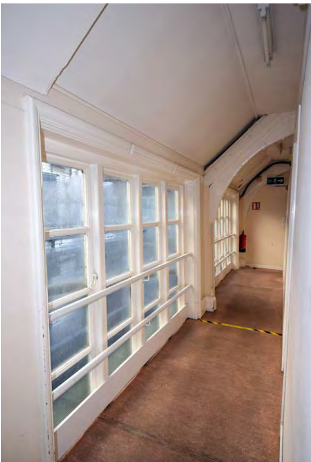
Plate 69: The second floor of 31 Cornmarket Street, looking north-east
