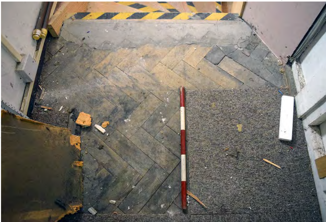
Plate 8: The floor of the south stairway in the basement of 31 Cornmarket Street, looking west
