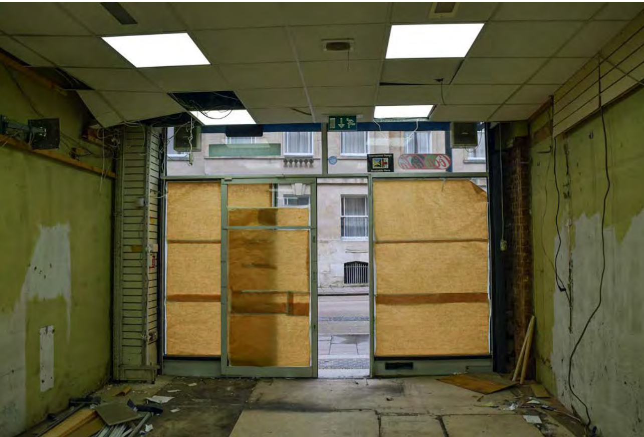
Plate 104: The ground floor of no. 4 Broad Street, looking north
