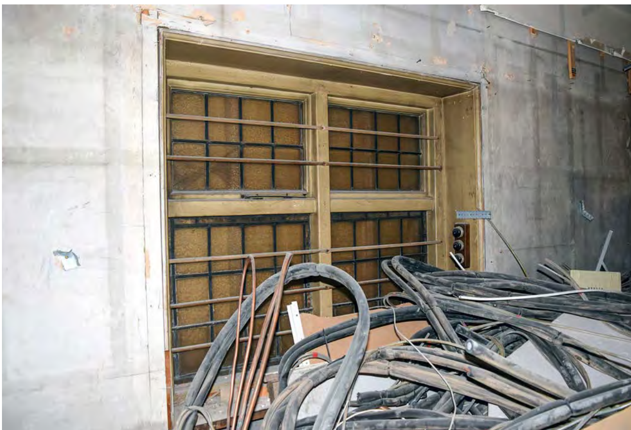
Plate 30: Window in the ground floor of 31 Cornmarket Street, looking south-west
