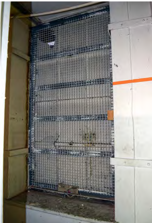
Plate 105: The ground floor of no. 4 Broad Street, looking south-east
