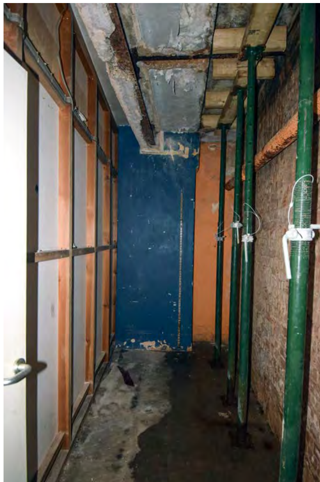
Plate 16: The basement of 1 to 5 Broad Street, looking west
