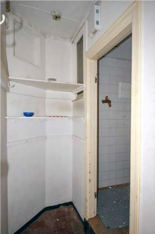
Plate 13: WC in the basement of 1 to 5 Broad Street, looking south-east
