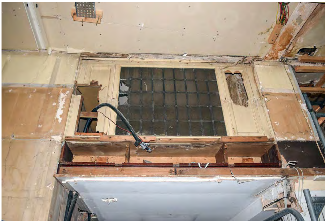
Plate 39: The ground floor of 1 to 5 Broad Street, looking east
