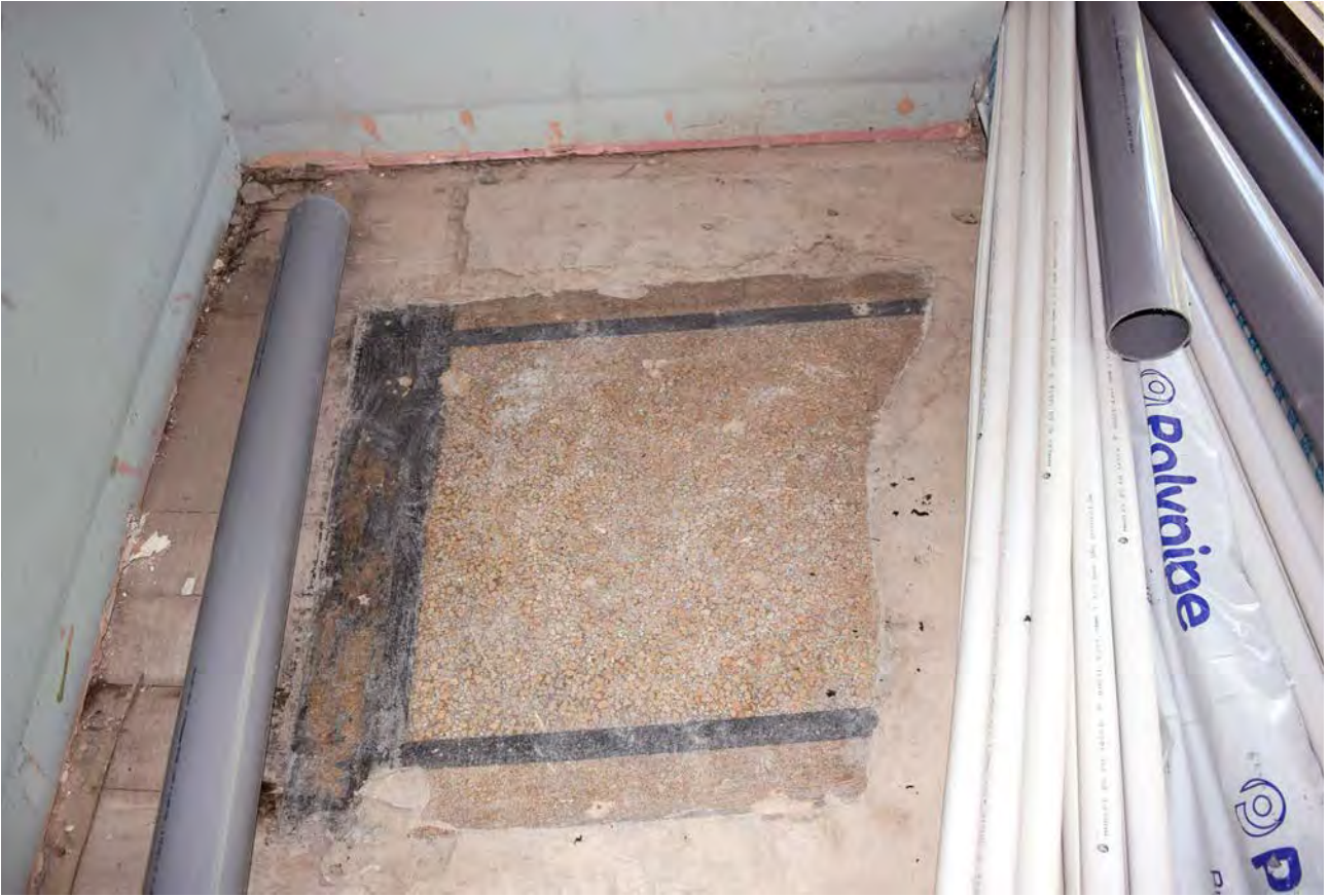
Plate 42: Terrazzo floor inside the ground floor entrance of 1 to 5 Broad Street
