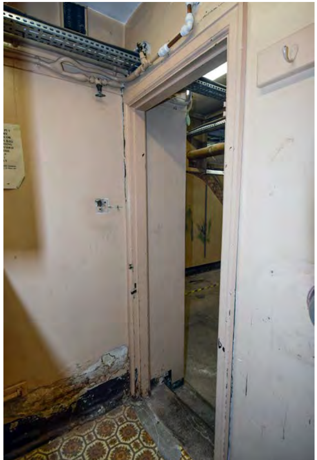
Plate 24: Kitchenette in the basement of 1 to 5 Broad Street, looking north-west
