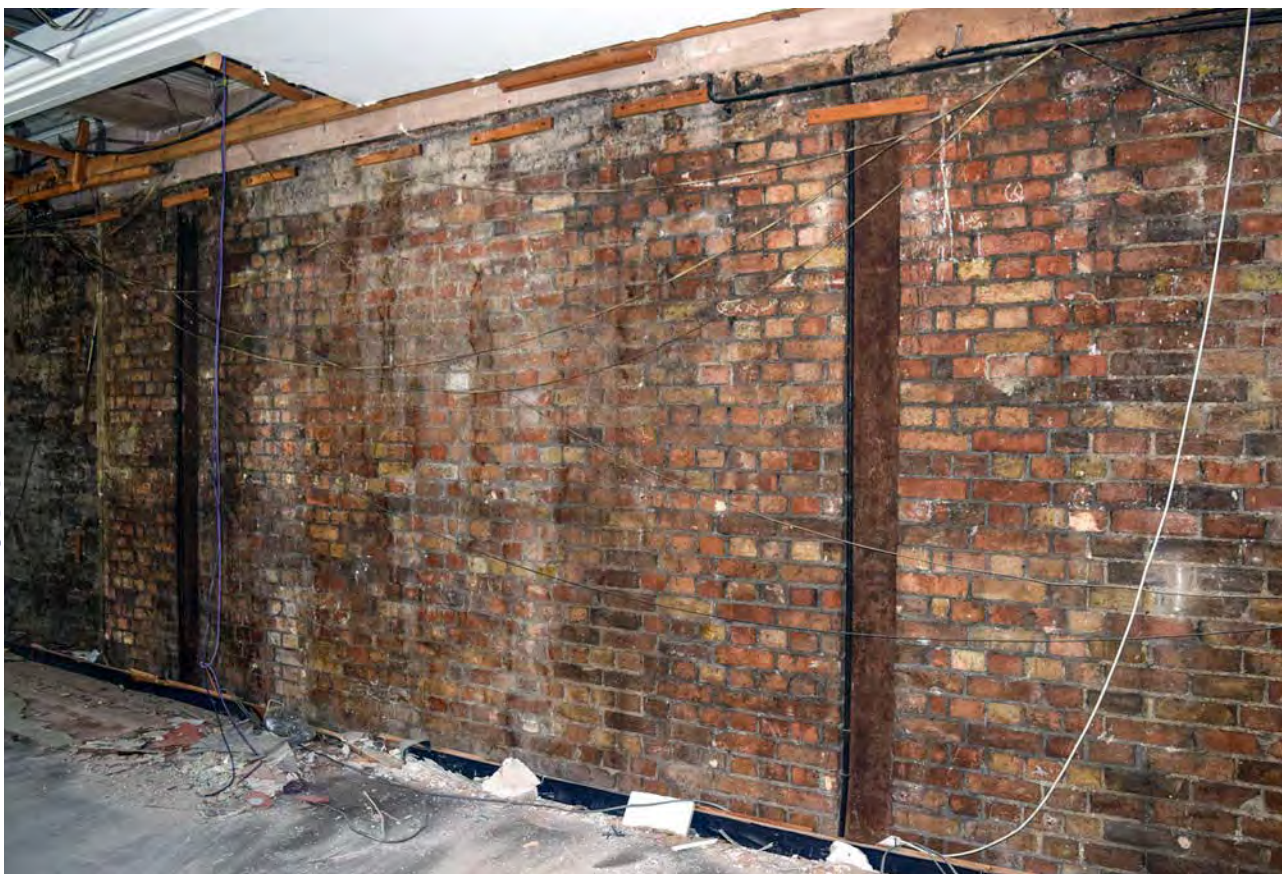
Plate 27: The ground floor of 31 Cornmarket Street, looking north-west
