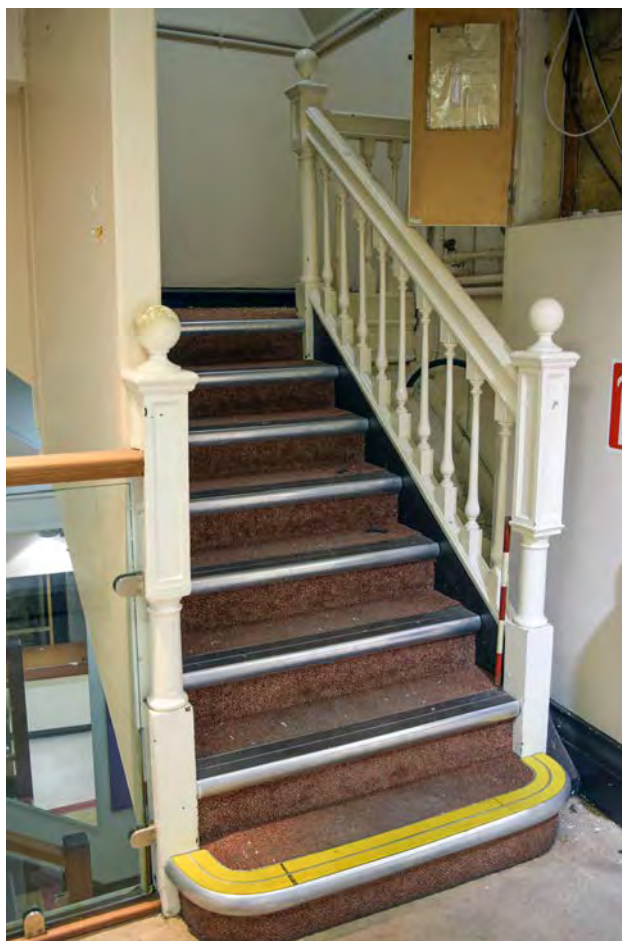
Plate 59: The stairway between the first and second floor in 31 Cornmarket Street, looking south-west
