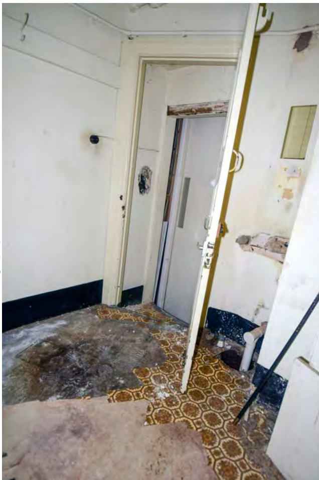
Plate 15: WC in the basement of 1 to 5 Broad Street, looking south-east
