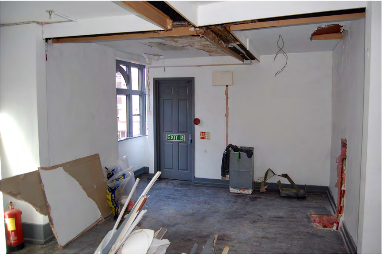
Plate 21: General view in first floor Room D & E looking east
