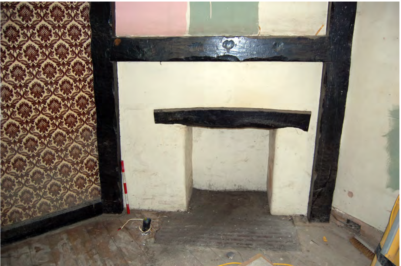
Plate 7: Angled fireplace at SW corner of 27B
