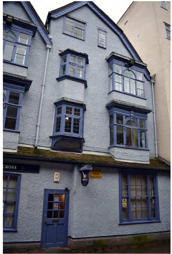
Plate 2: Western section of the north elevation facing the courtyard
