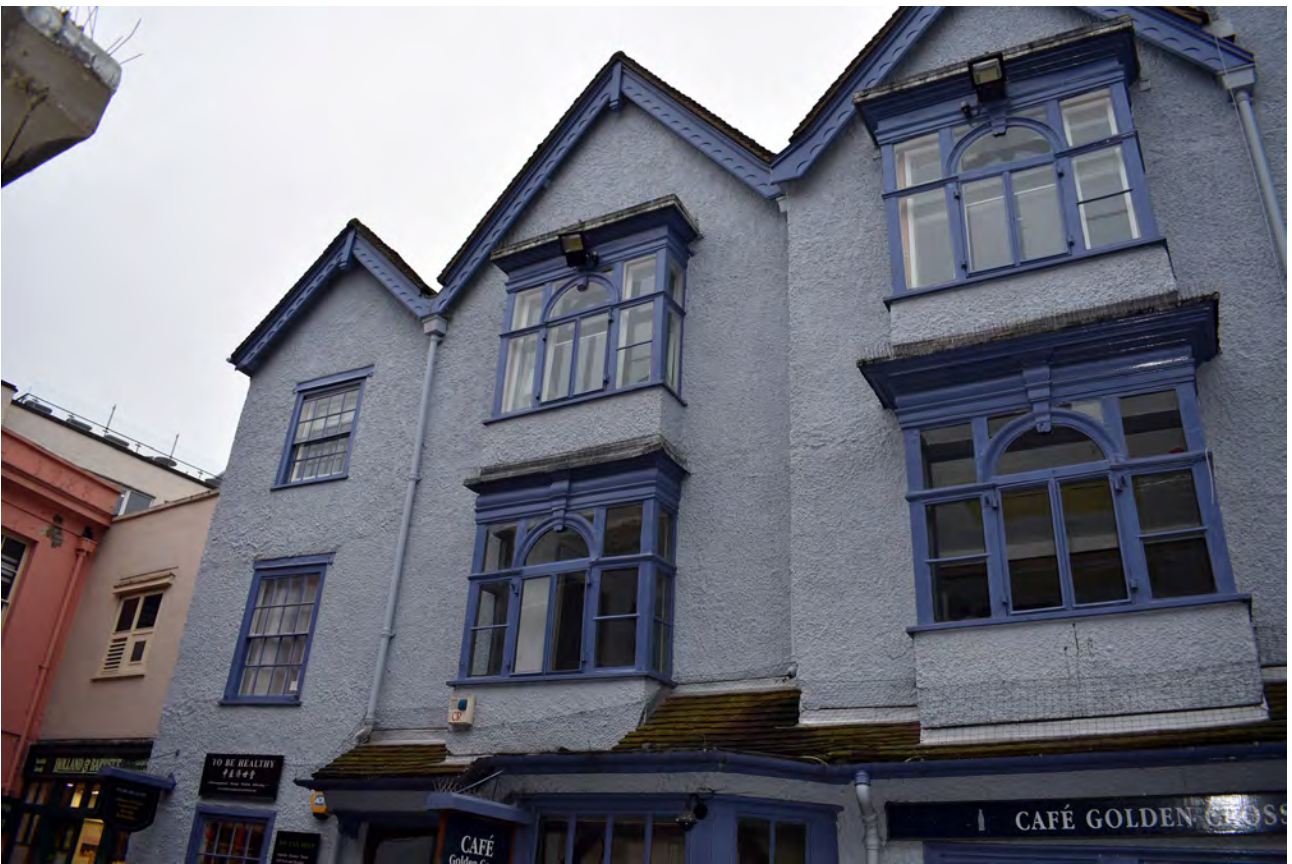
Plate 3: Eastern section of the north elevation facing the courtyard
