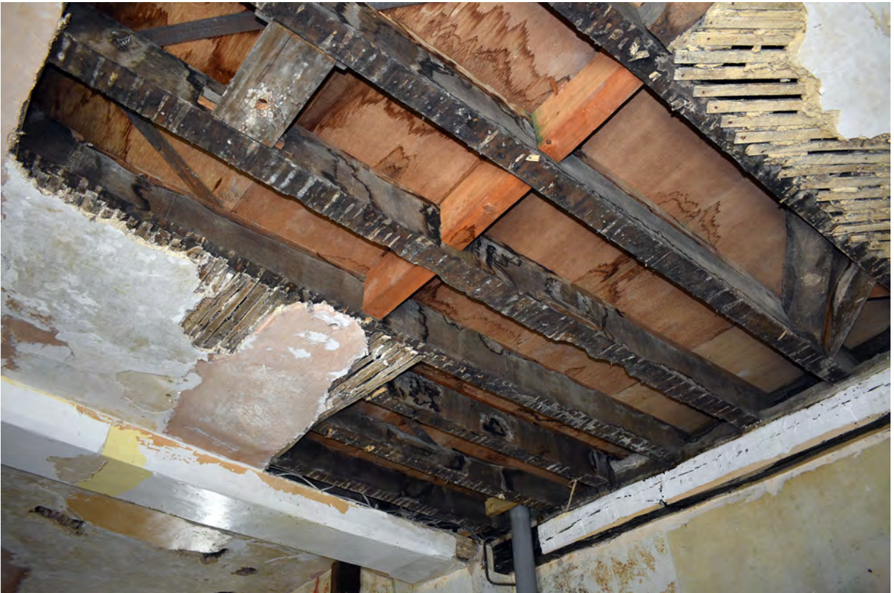
Plate 14: Underside of joists exposed in 27B, looking SE
