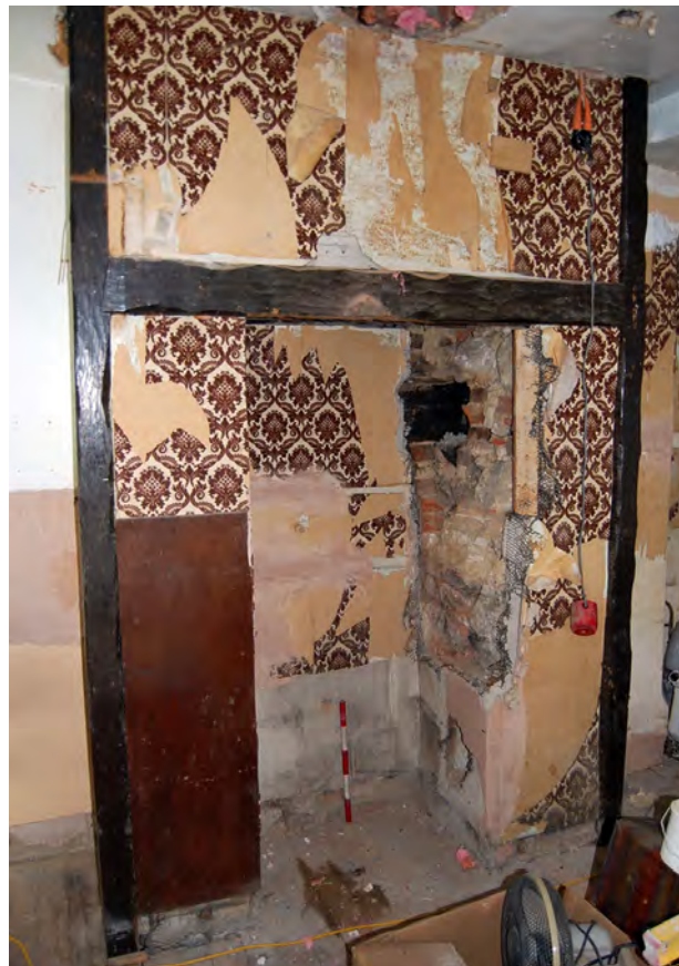
Plate 9: Exposed fireplace and chimney breast in 27C
