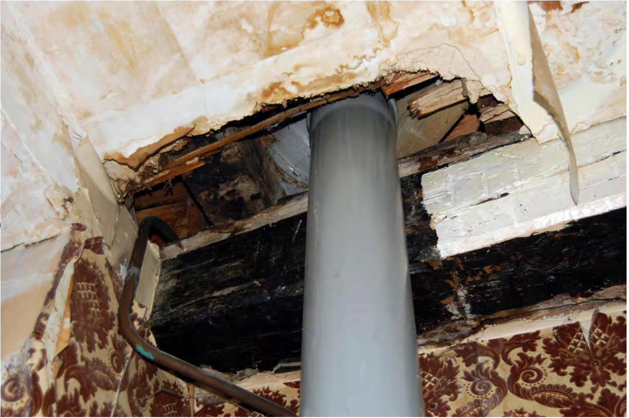
Plate 13: Detail of beam at SE corner of 27B
