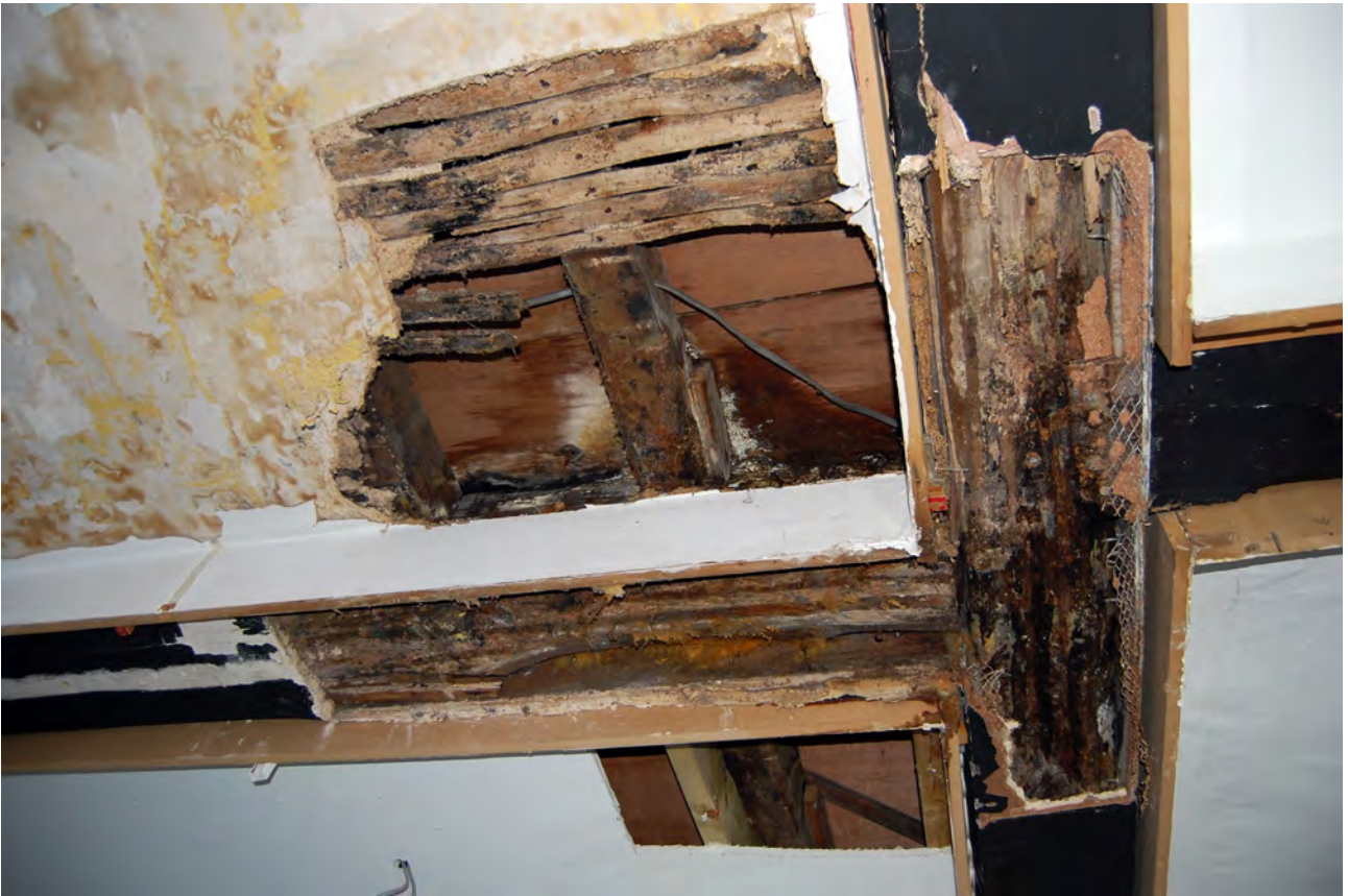
Plate 27: Exposed floor joists in Room D looking south
