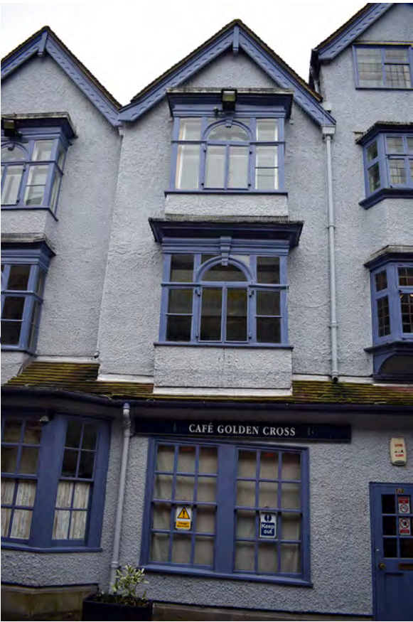
Plate 1: Central section of the north elevation facing the courtyard
