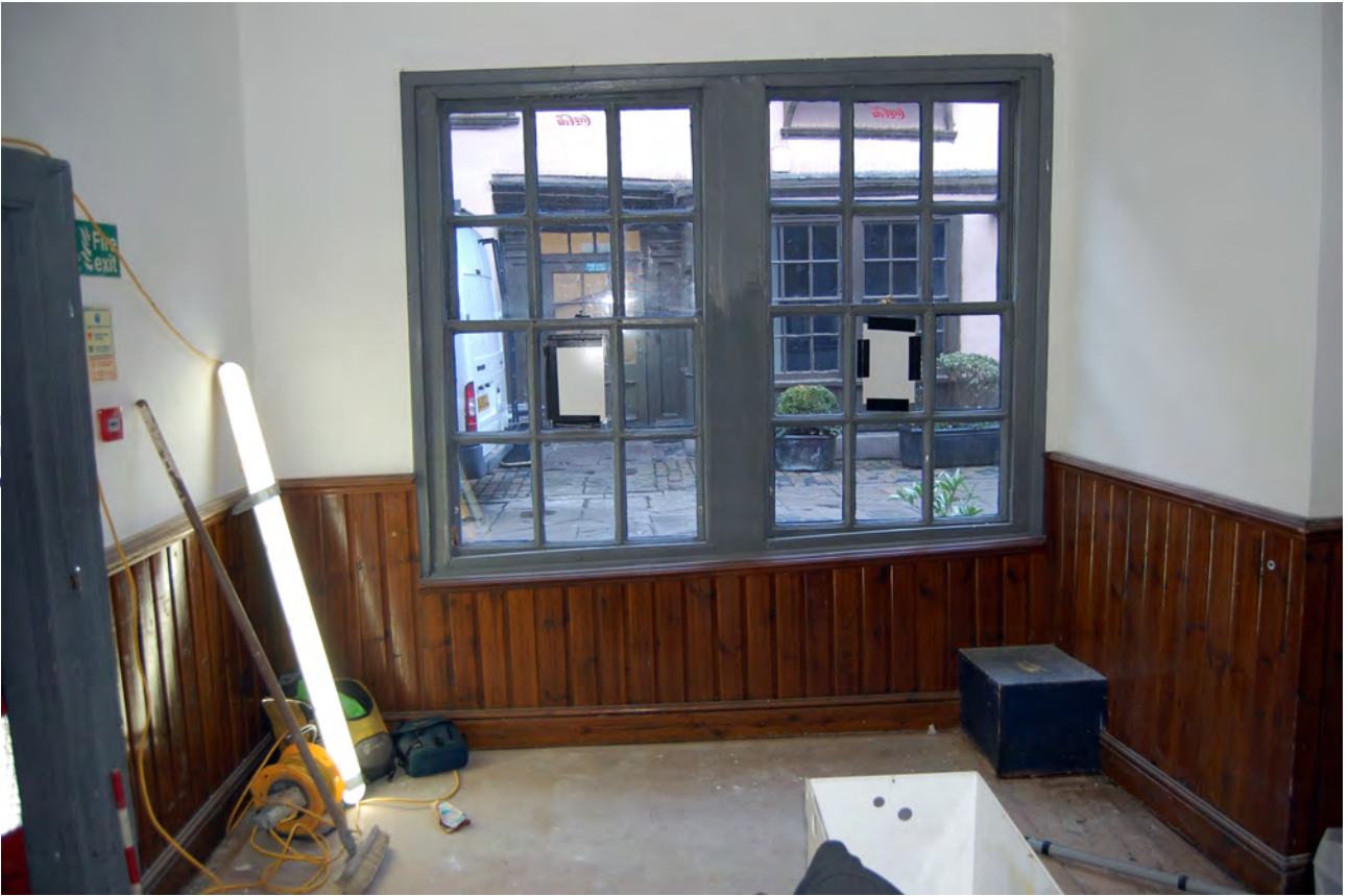
Plate 19: Window in 27B
