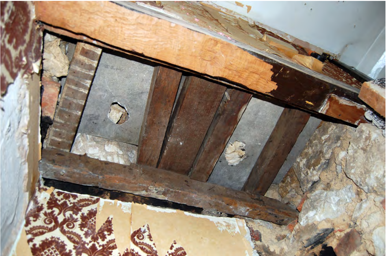
Plate 12: Blocking above fireplace void in 27C
