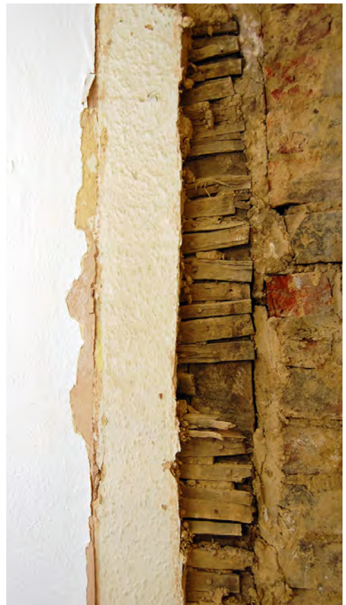
Plate 32: Detail of east wall in Room C after plaster removal
