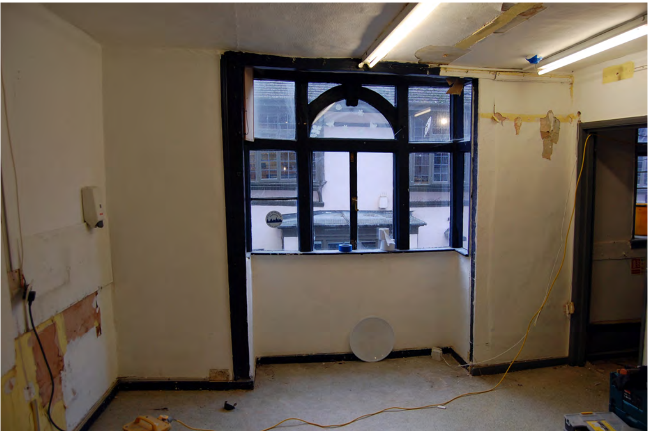
Plate 35: General view looking north in Room C after removal of partitions
