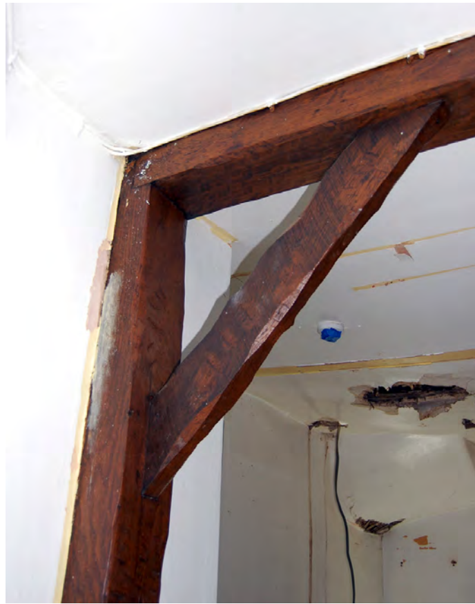
Plate 17: Detail of secondary bracing in 27C
