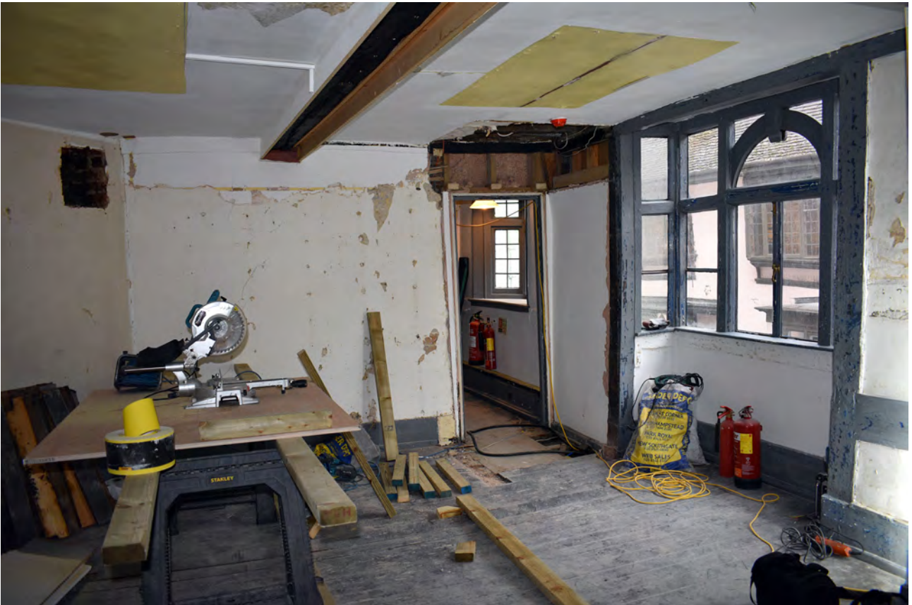
Plate 20: General view in first floor Room D looking west
