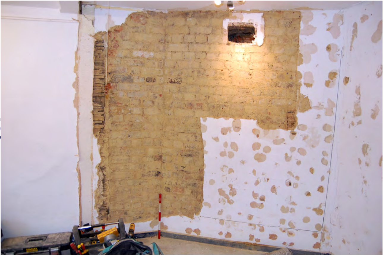
Plate 30: Chimney breast at SE corner of Room C after plaster removal
