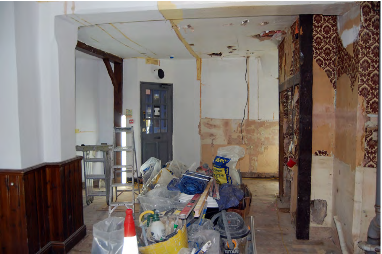
Plate 5: Ground floor Room 27C looking east
