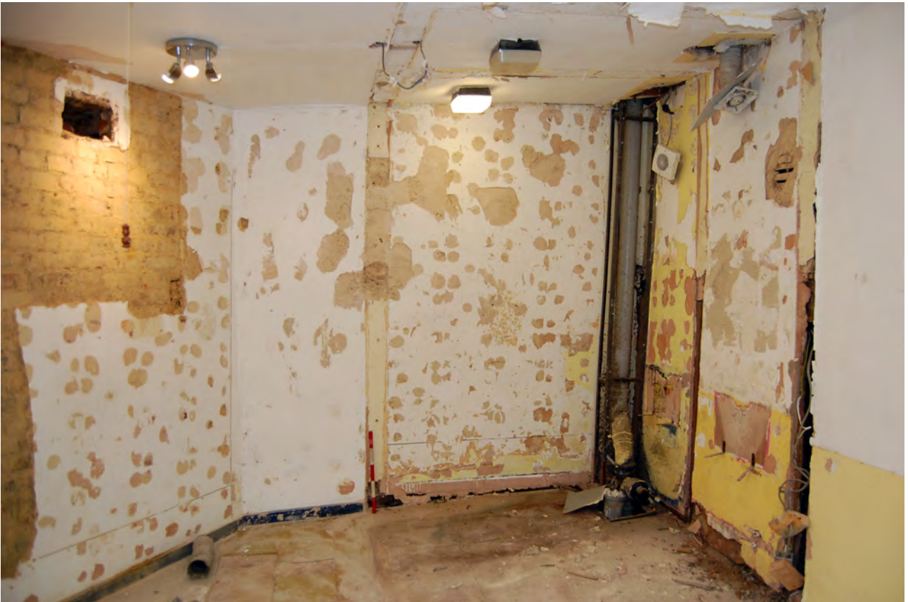
Plate 29: First floor room C looking south after removal of partitions
