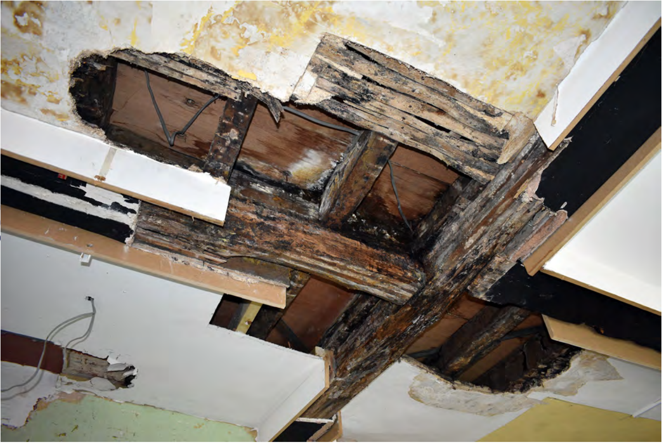
Plate 26: Exposed floor joists in Room D looking south
