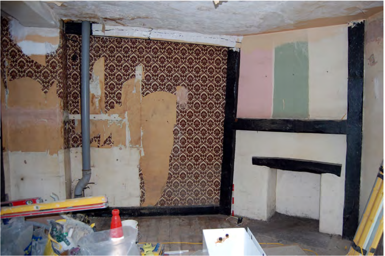
Plate 6: Ground floor Room 27B looking south
