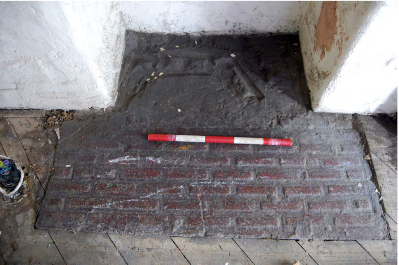
Plate 8: Brick paved hearth to fireplace at SW corner of 27B
