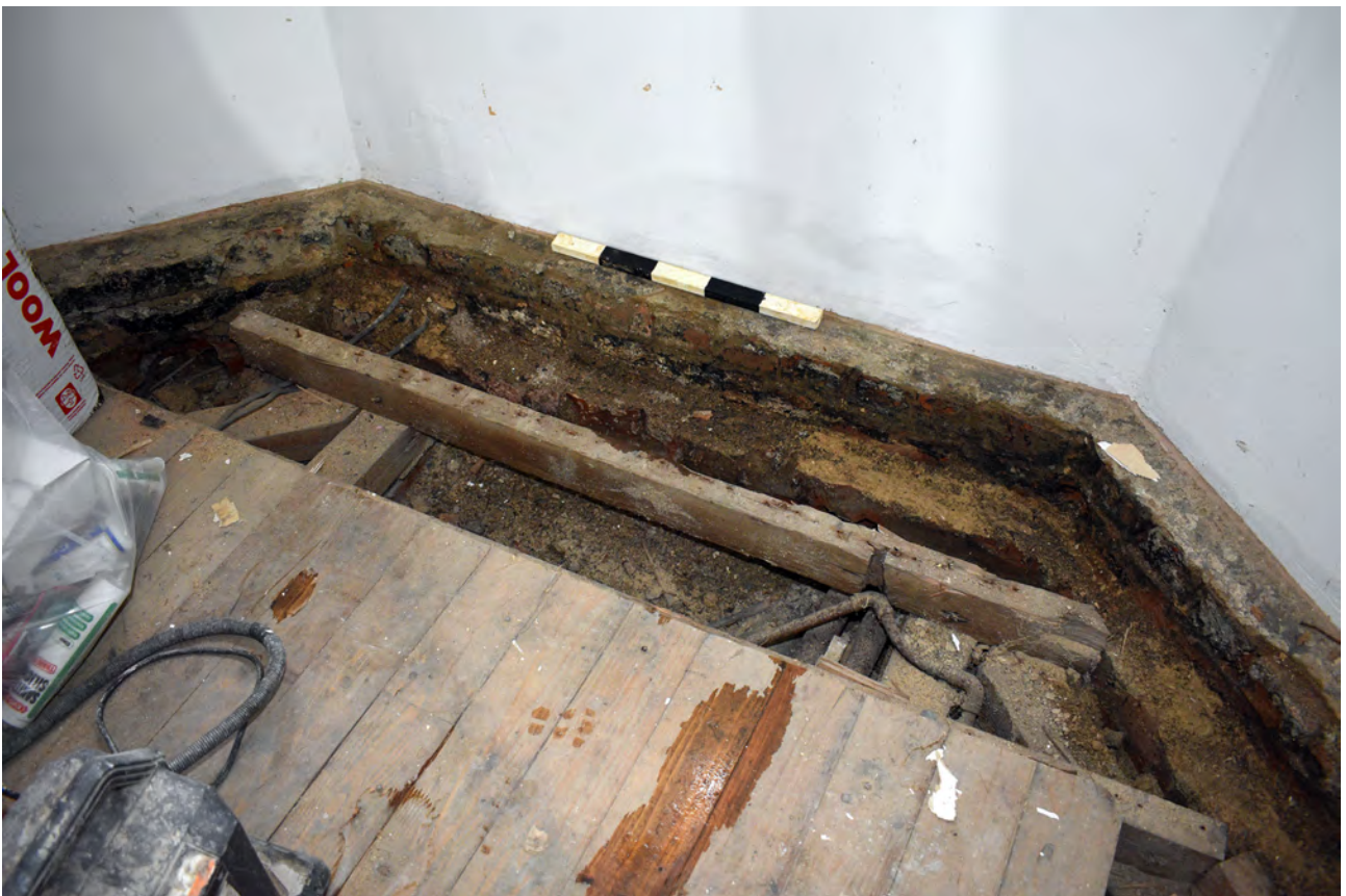
Plate 18: Exposed plinth to bay window in 27C.
