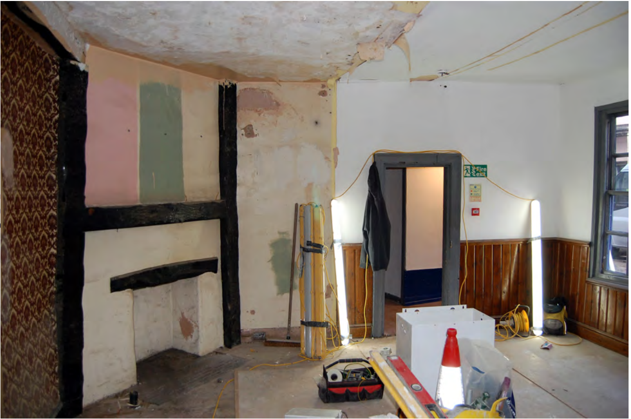
Plate 4: Ground floor Room 27B looking west
