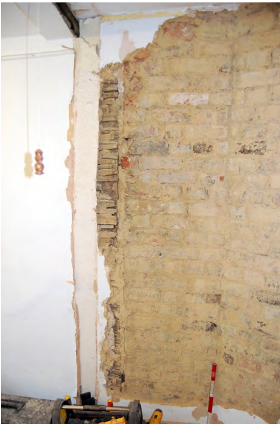
Plate 31: Detail of east wall in Room C after plaster removal
