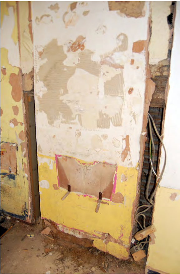
Plate 33: Detail of west wall in Room C after plaster removal
