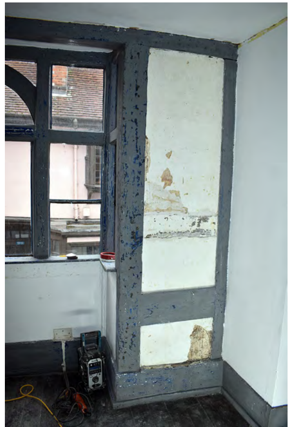
Plate 23: East side of oriel window in first floor Room D
