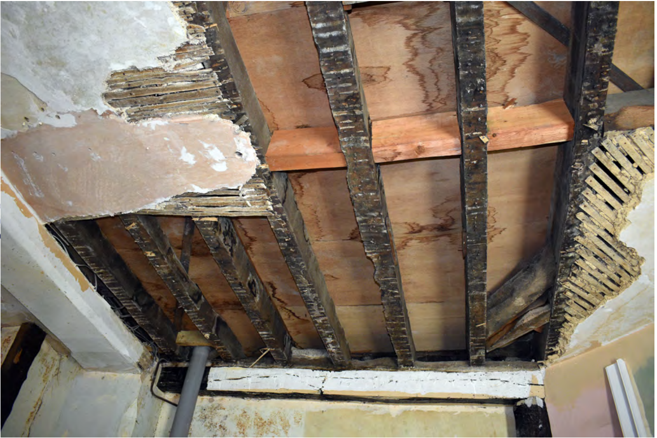
Plate 15: Underside of joists exposed in 27B, looking S
