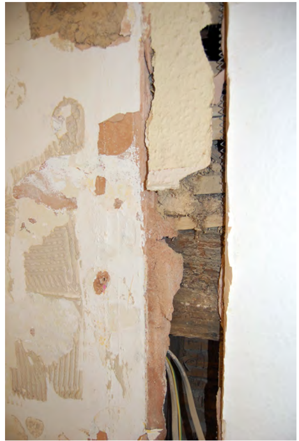
Plate 34: Exposed timber rail in west wall of Room C after plaster removal
