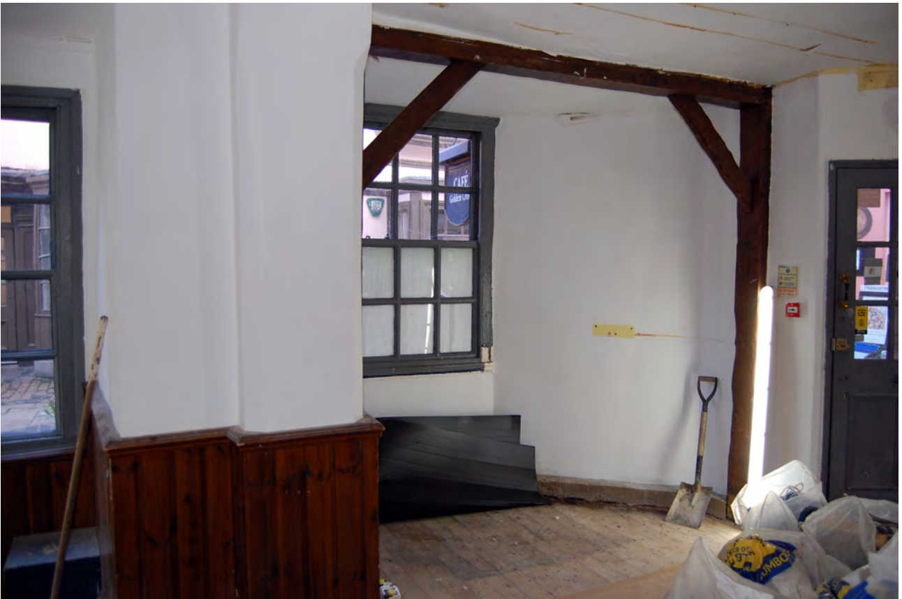
Plate 16: View in 27B-27C looking NE
