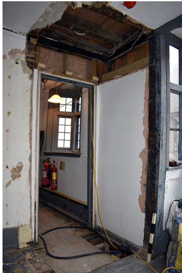
Plate 24: NW corner of Room D after removal of modern lobby
