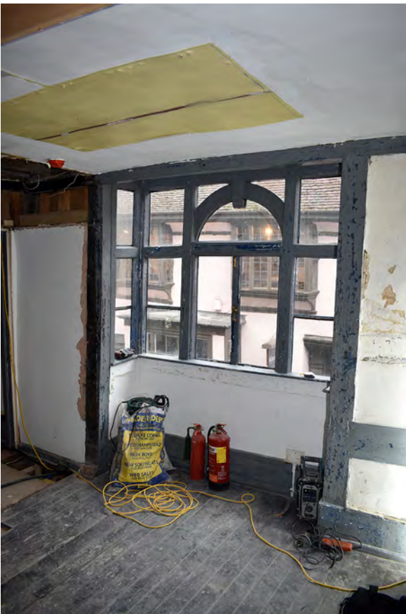
Plate 22: Oriel window in first floor Room D
