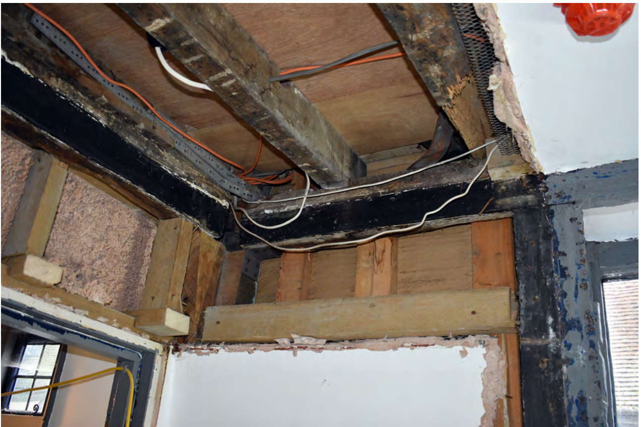
Plate 25: NW corner of Room D after removal of modern lobby
