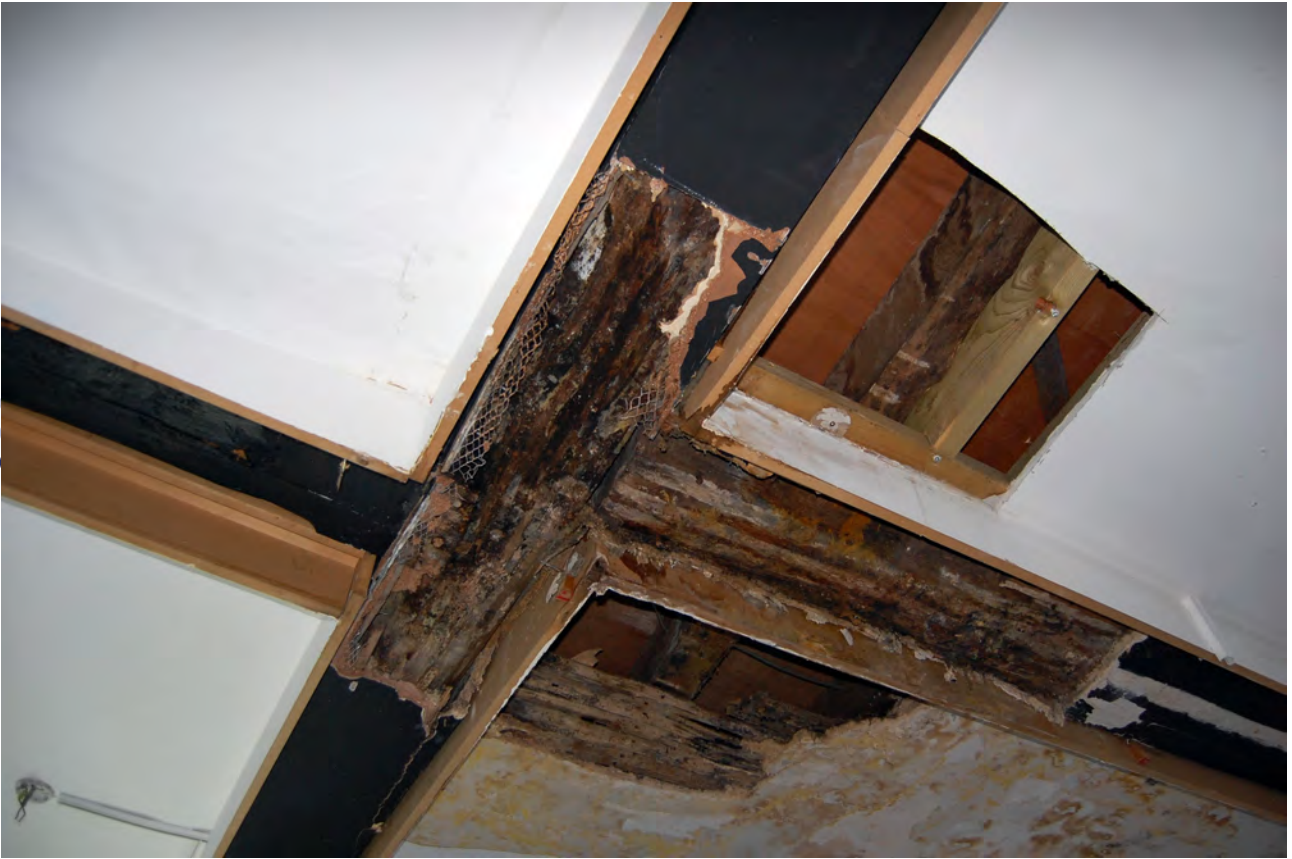
Plate 28: Exposed floor joists in Room D looking north
