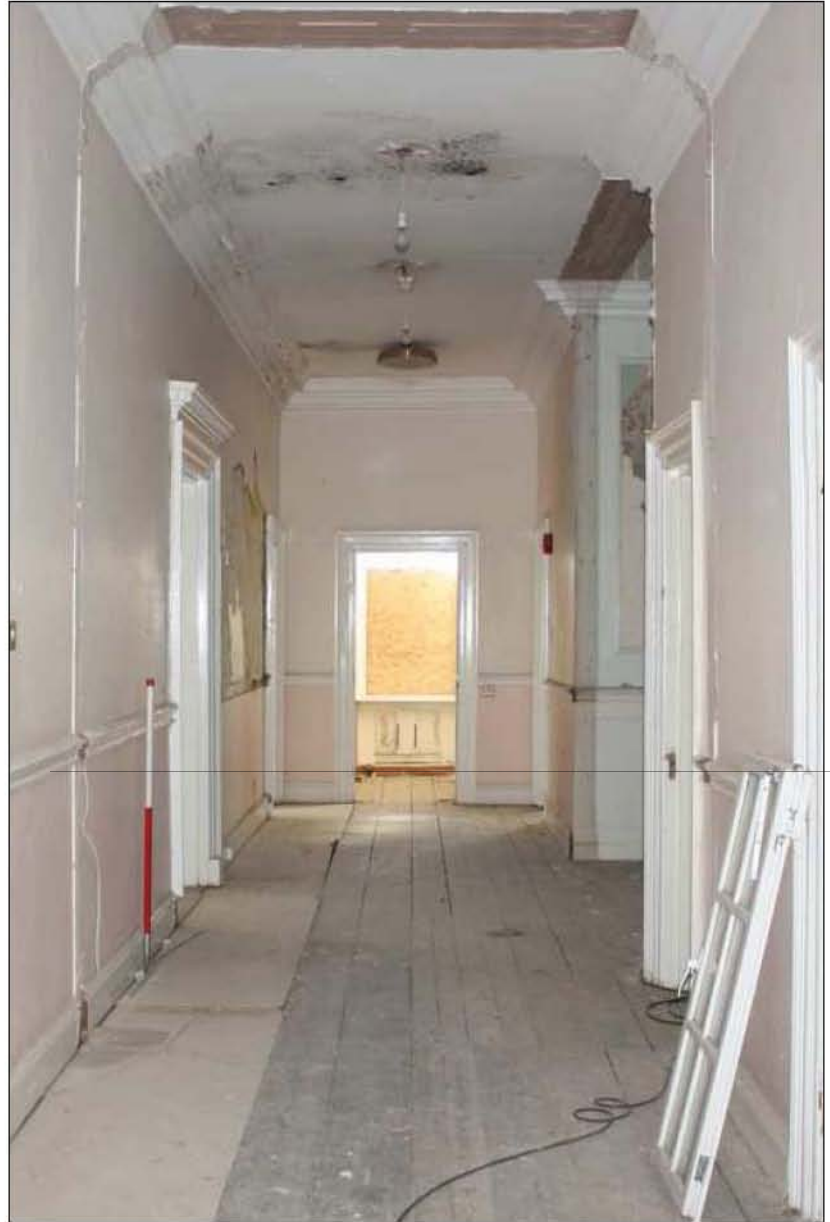
Plate 40: first floor landing, F2
