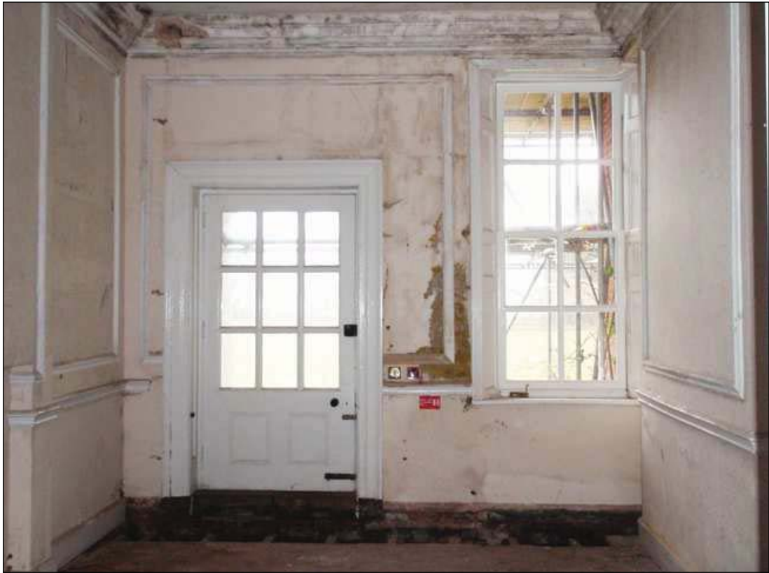
Plate 32: Door and window, G16
