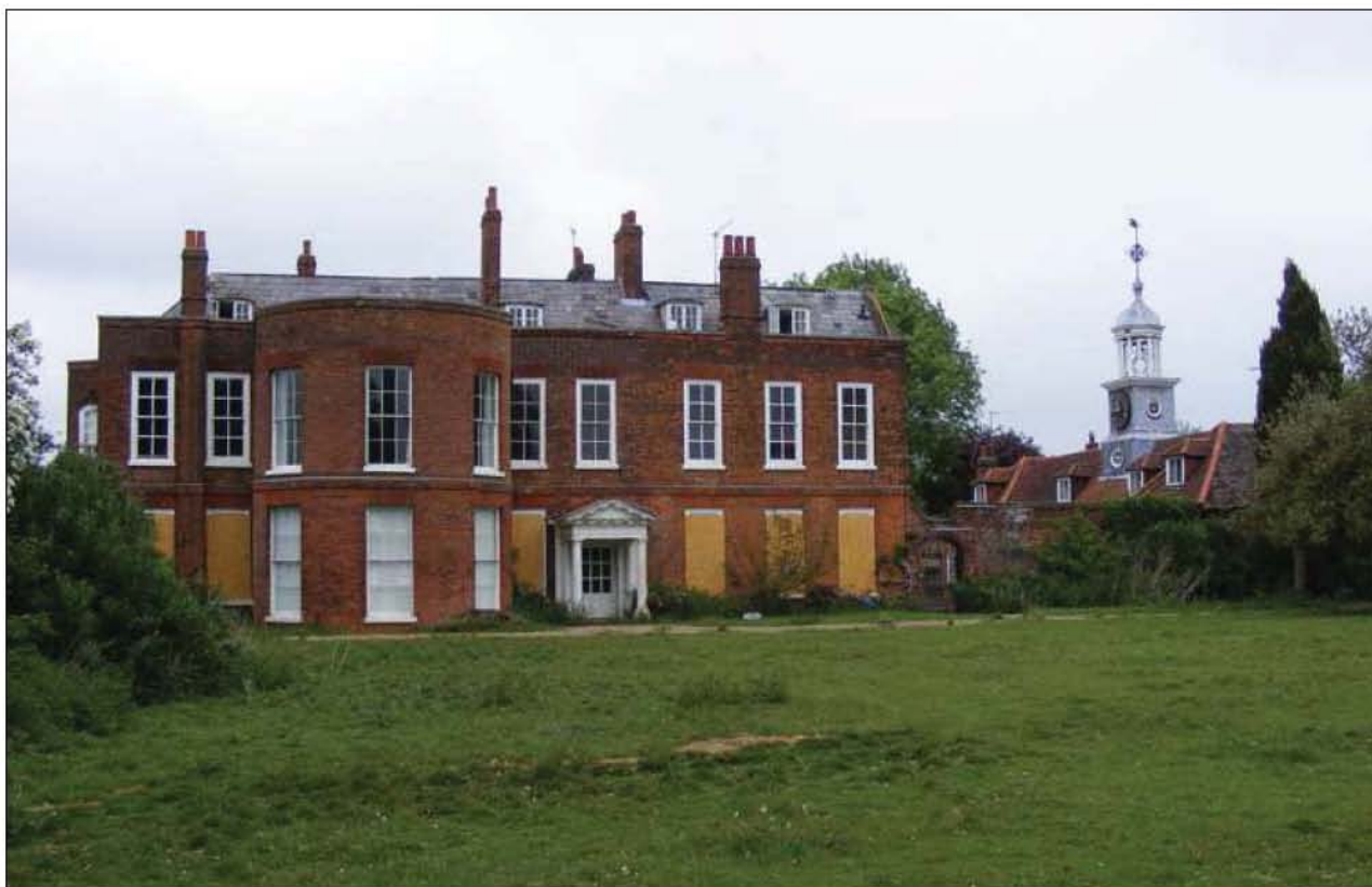
Plate 5: South facing elevation, Orford House
