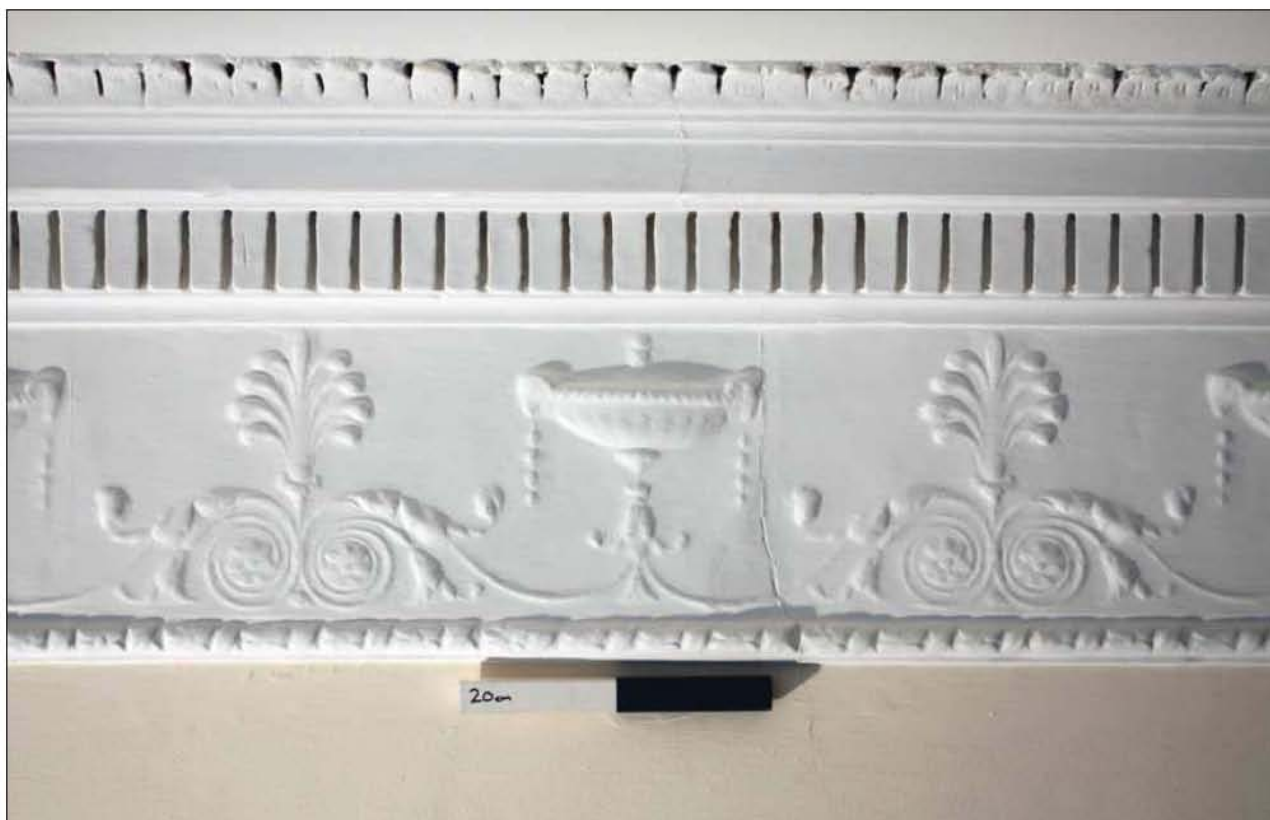
Plate 52: Detail of ceiling cornice, F9
