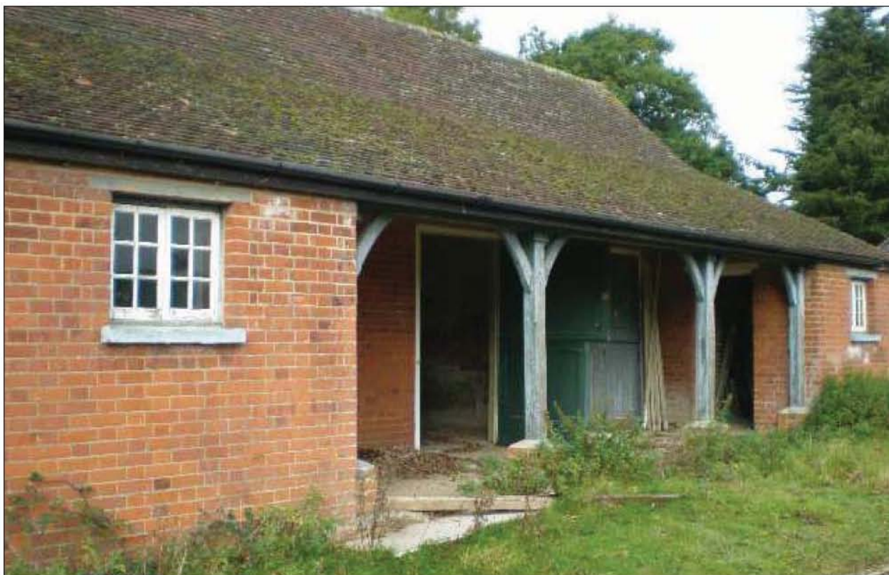
Plate 82: East facing elevation of "The Stables"
