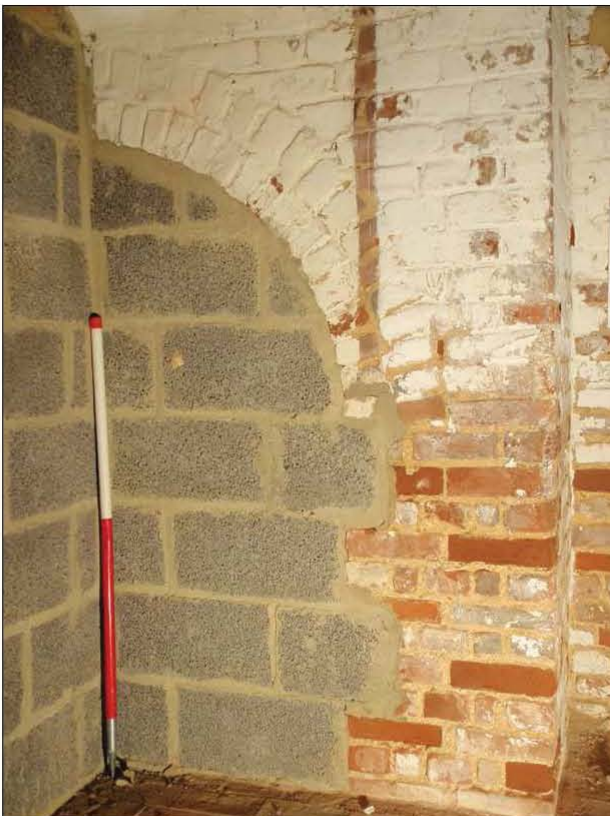
Plate 64: Blocked brick arch, B5
