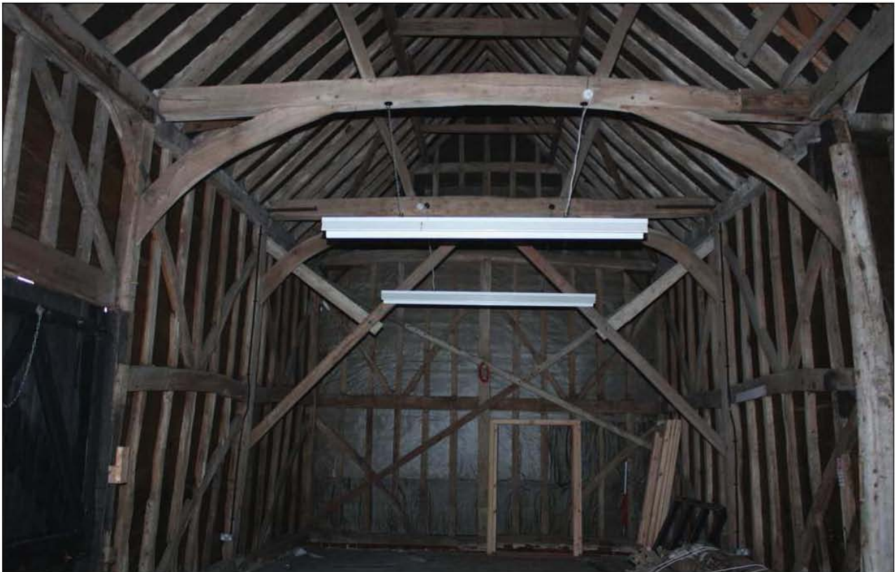
Plate 76: Scissor bracing on rear elevation, phase 2 barn
