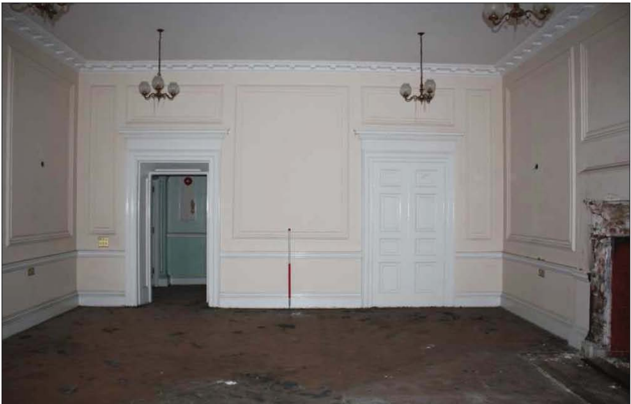
Plate 29: Internal view of doors, G15
