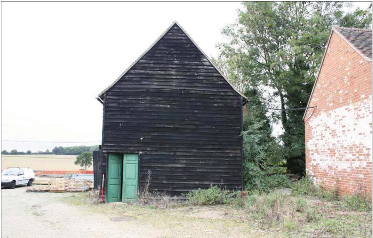
Plate 74: East facing gable end of barn
