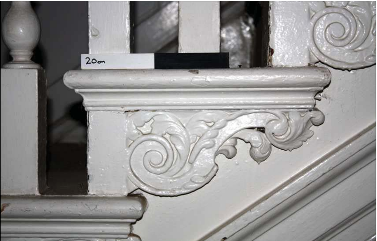
Plate 16: Detail of staircase tread-end, G12
