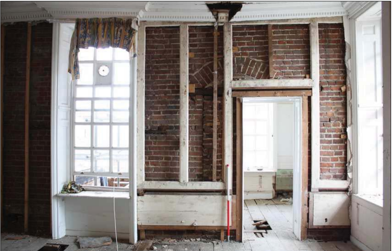
Plate 54: Exposed brickwork, F10
