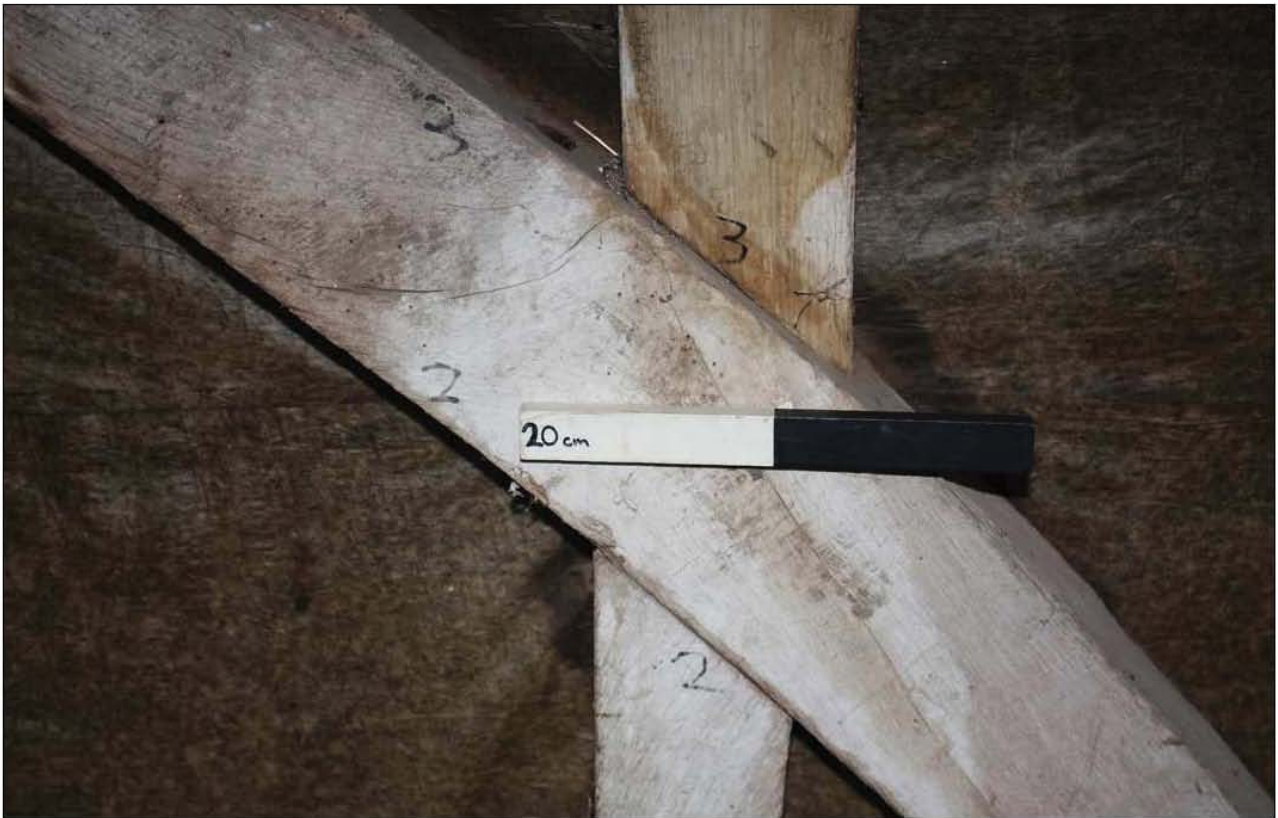
Plate 77: Detail of modern carpenters construction marks
