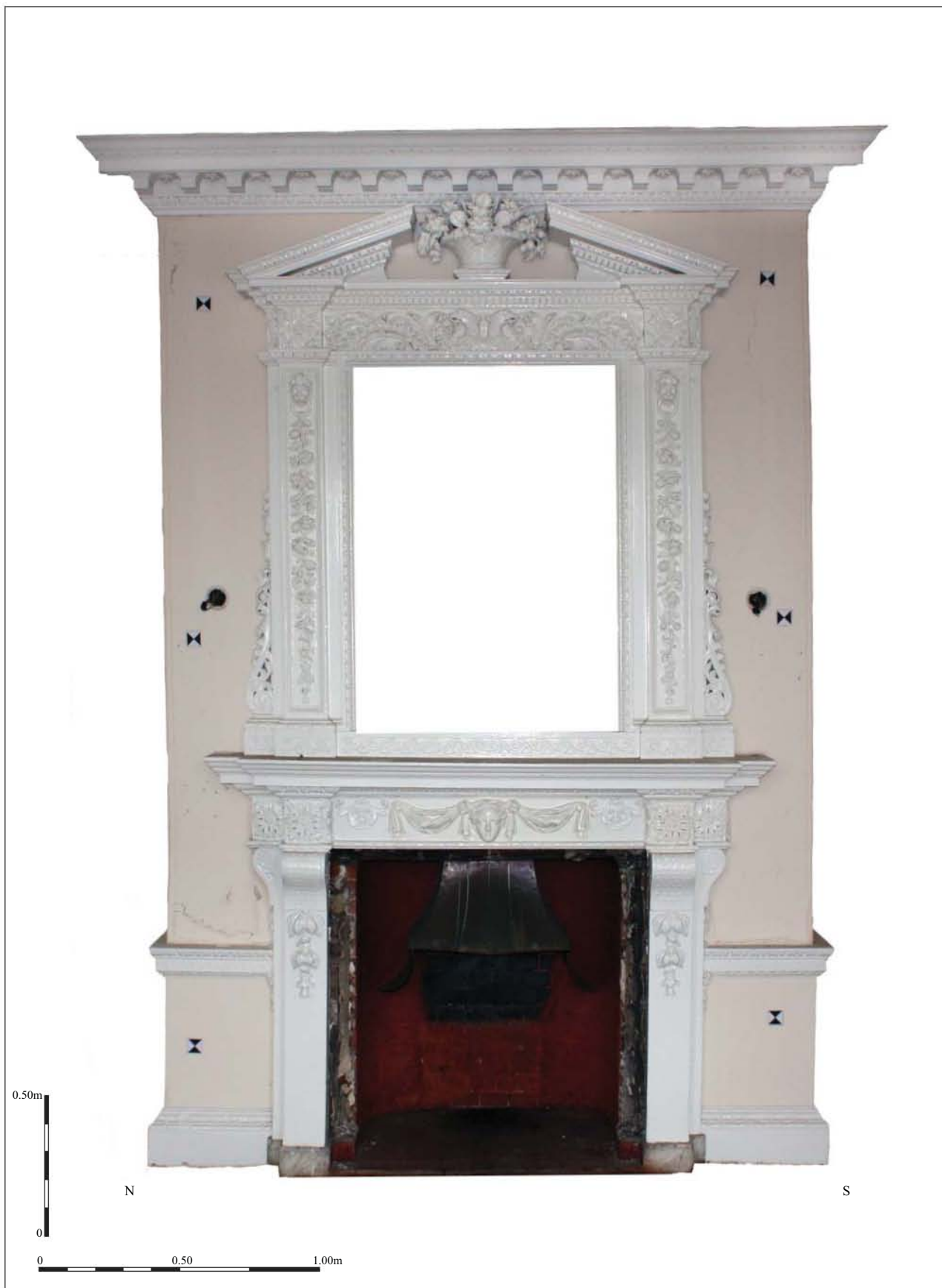
Figure 12: Rectified image of fireplace and carved chimney peice overmantle, G13
