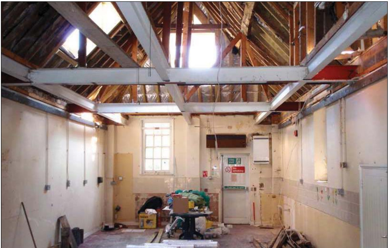
Plate 67: Interior of "motor house", Coachman's Cottage
