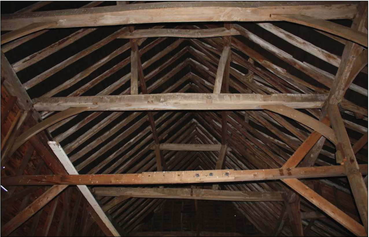
Plate 71: Detail of repair to roof structure, phase 1 barn
