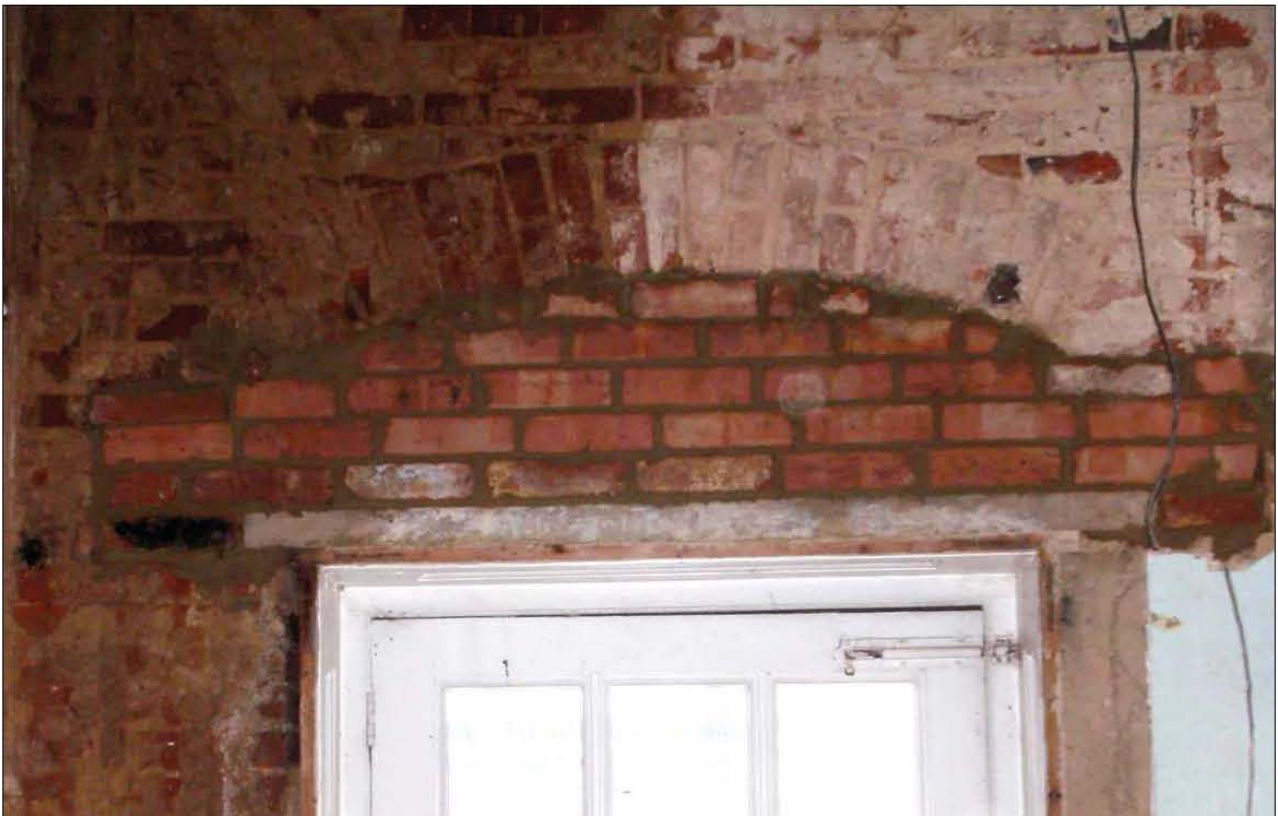
Plate 20: Detail of exposed brickwork above door, G12
