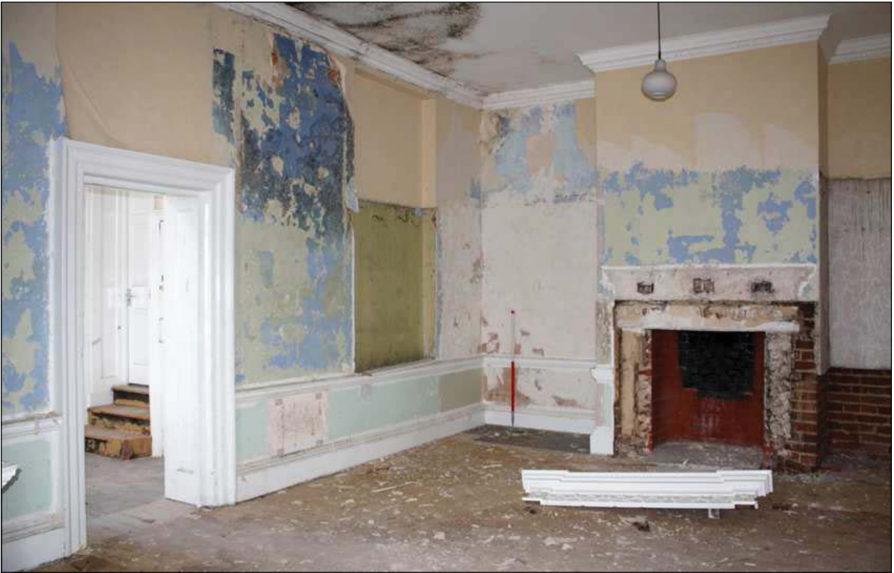
Plate 43: Blocked-up window, F3
