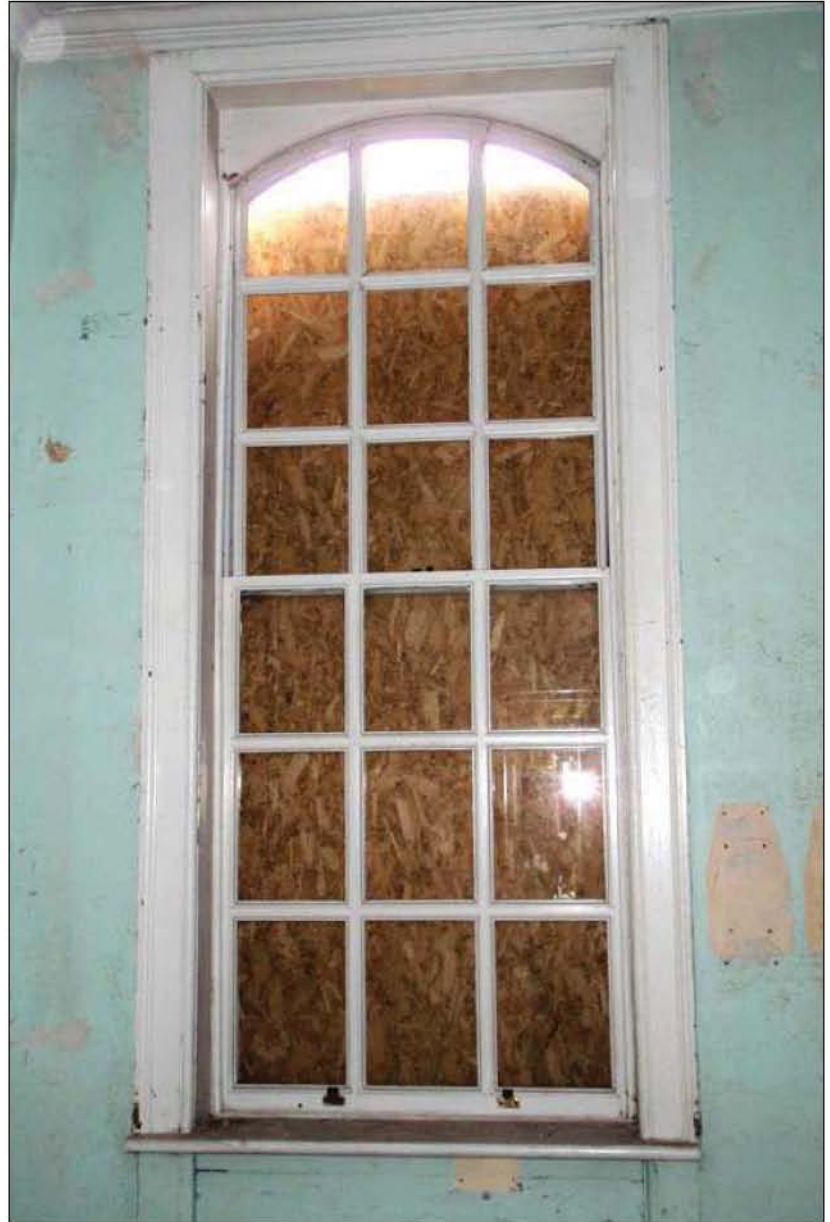
Plate 12: Internal view of window, G8
