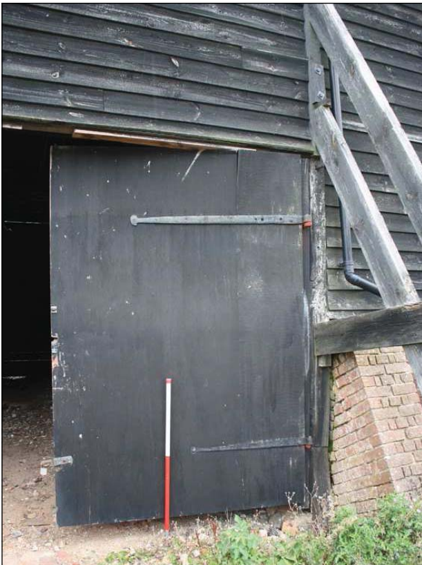
Plate 72: Detail of exterior of phase 1 barn door
