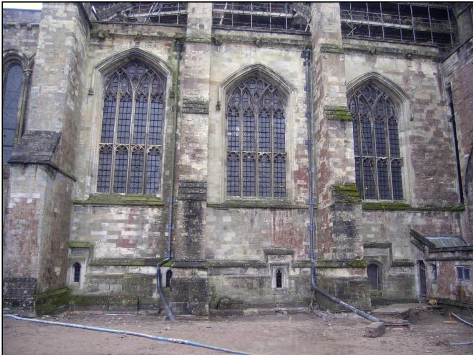
Plate 3: General shot of Romanesque plinth under 16th century presbytery aisle walls
