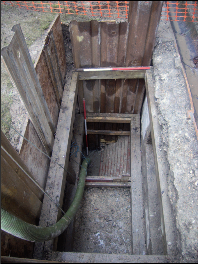
Plate 1: Stepped brick underpinning of north transept
