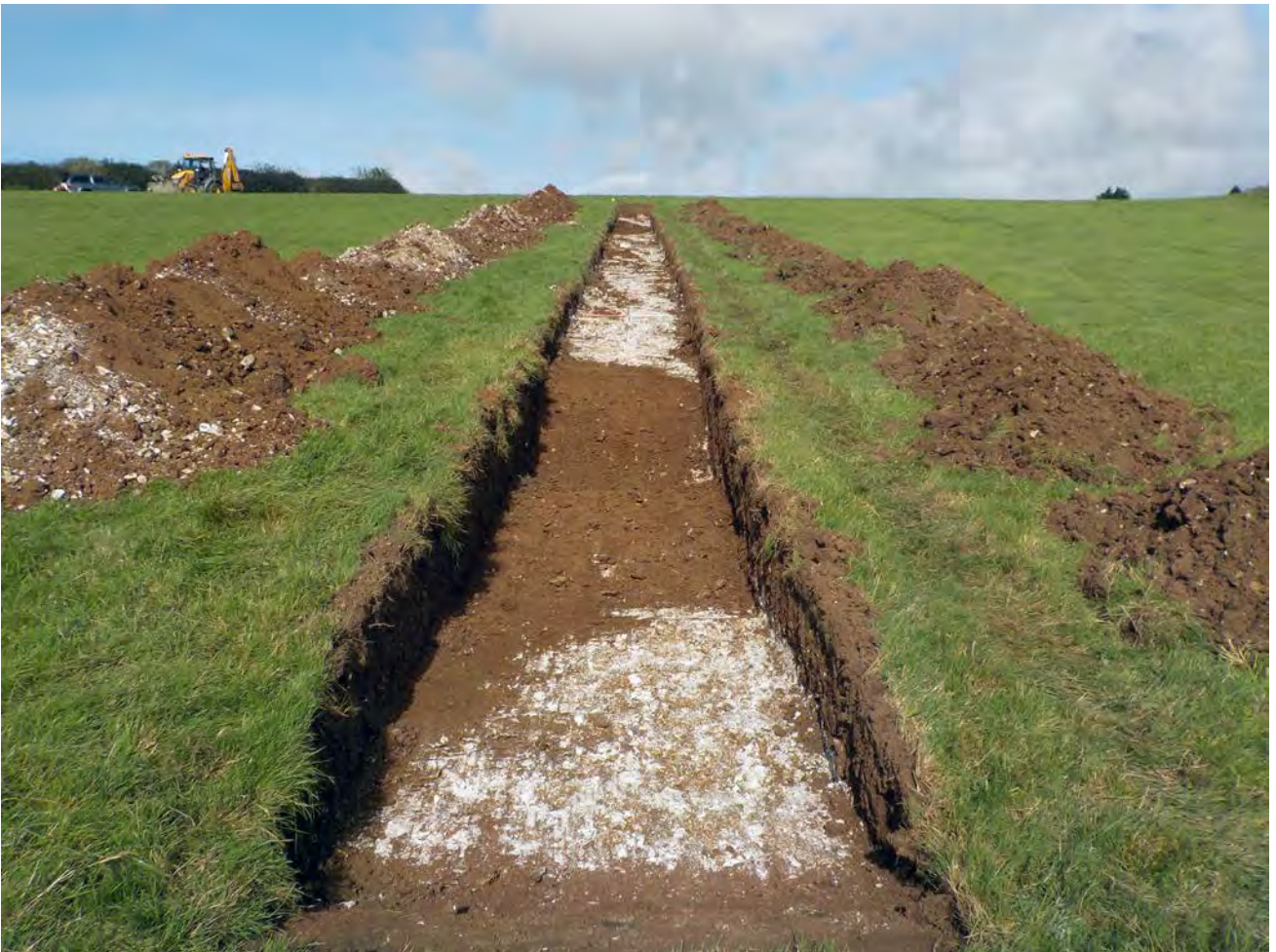
Plate 8: Trench 75 - view to NW
