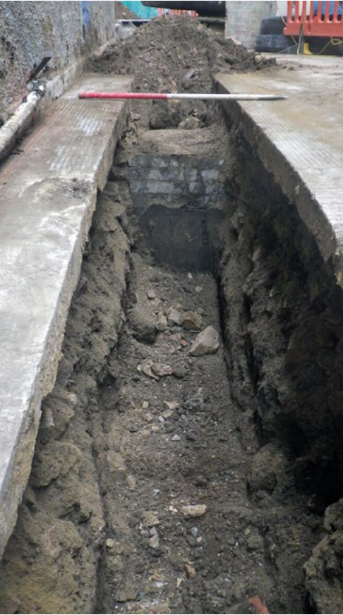
Plate 7: 20th century basement wall 446
