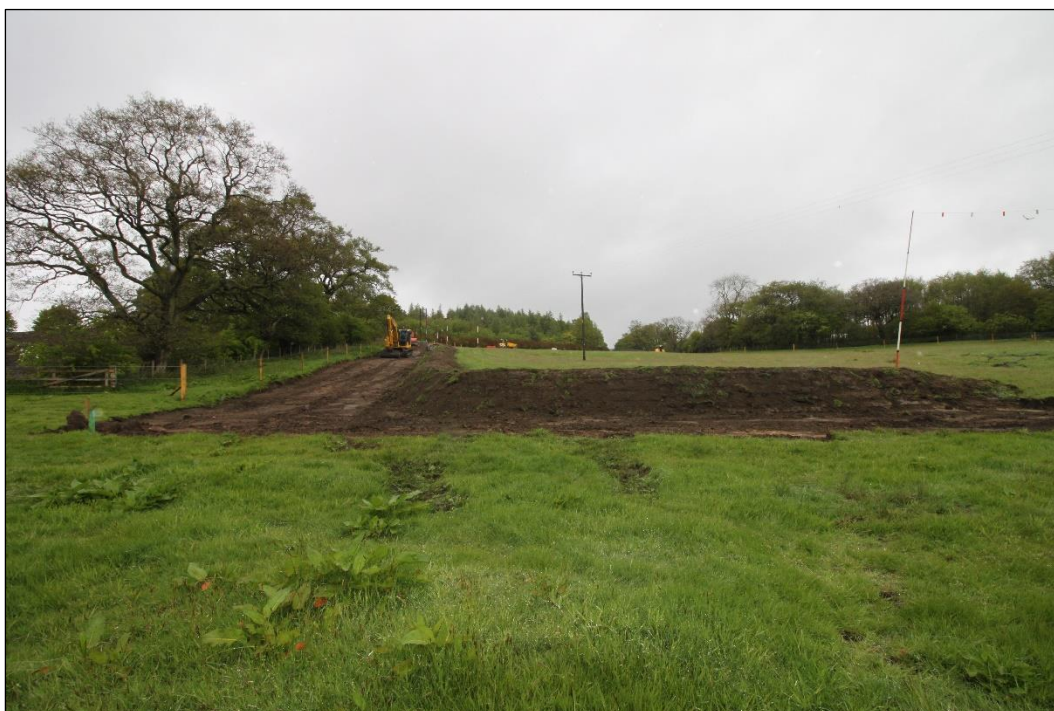
Plate 1: Field 1, facing north, showing topsoil stripping for the relocation of overhead wires, located within western area of Field 1
