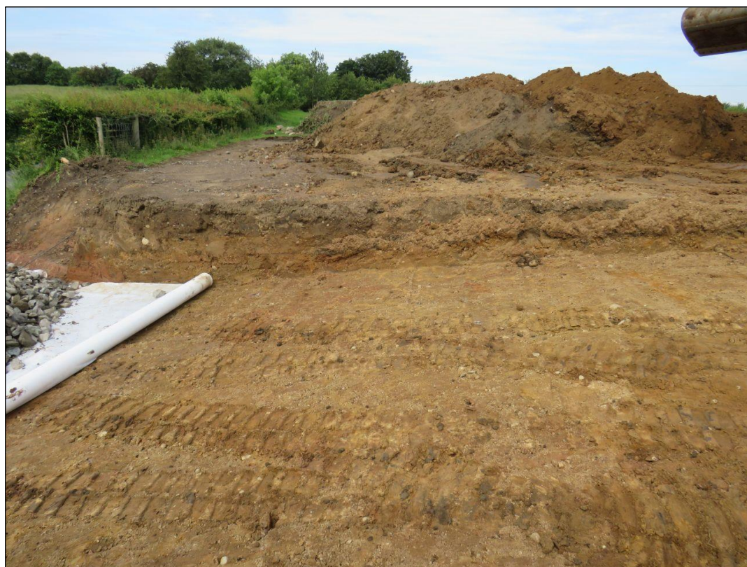
Plate 3: Access ramp from Main Street to the Main Street Compound, looking north-west
