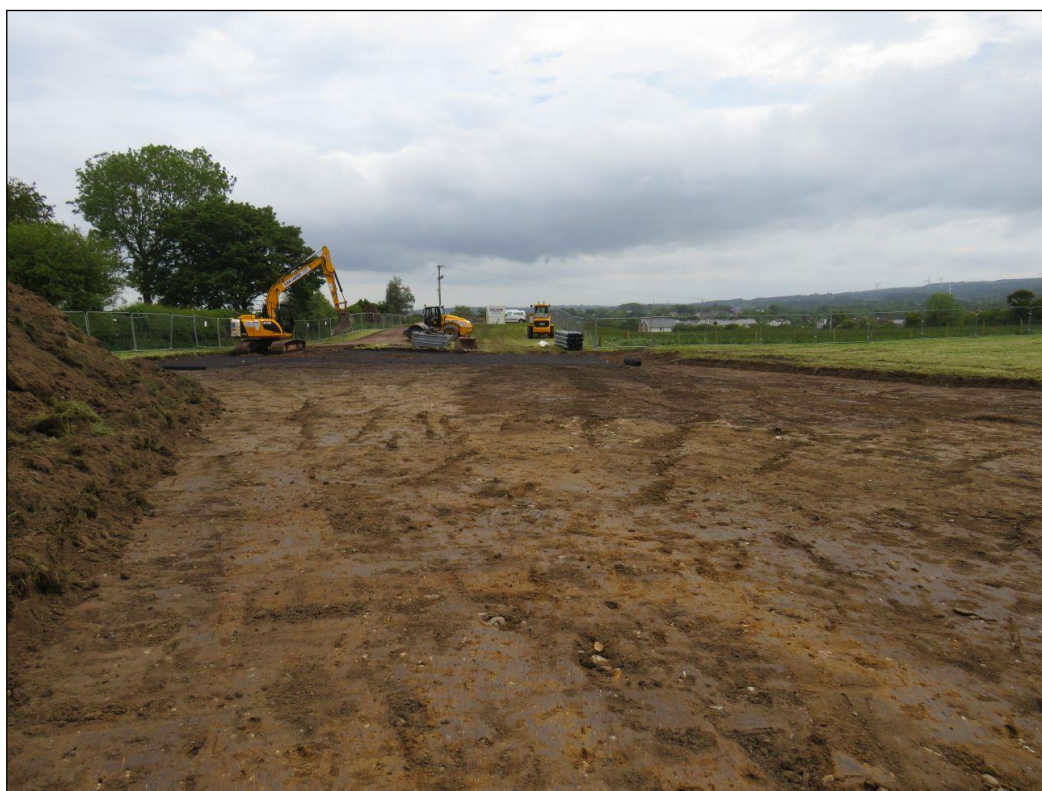
Plate 1: General view of the Central Road Compound, looking north-east
