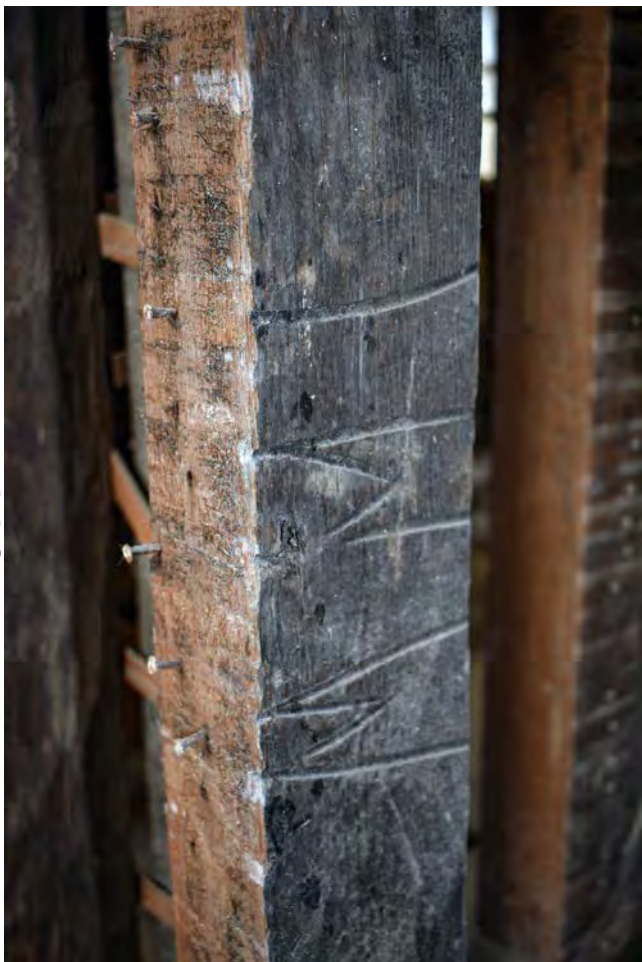
Plate 93: Baltic timber marks to first floor frame
