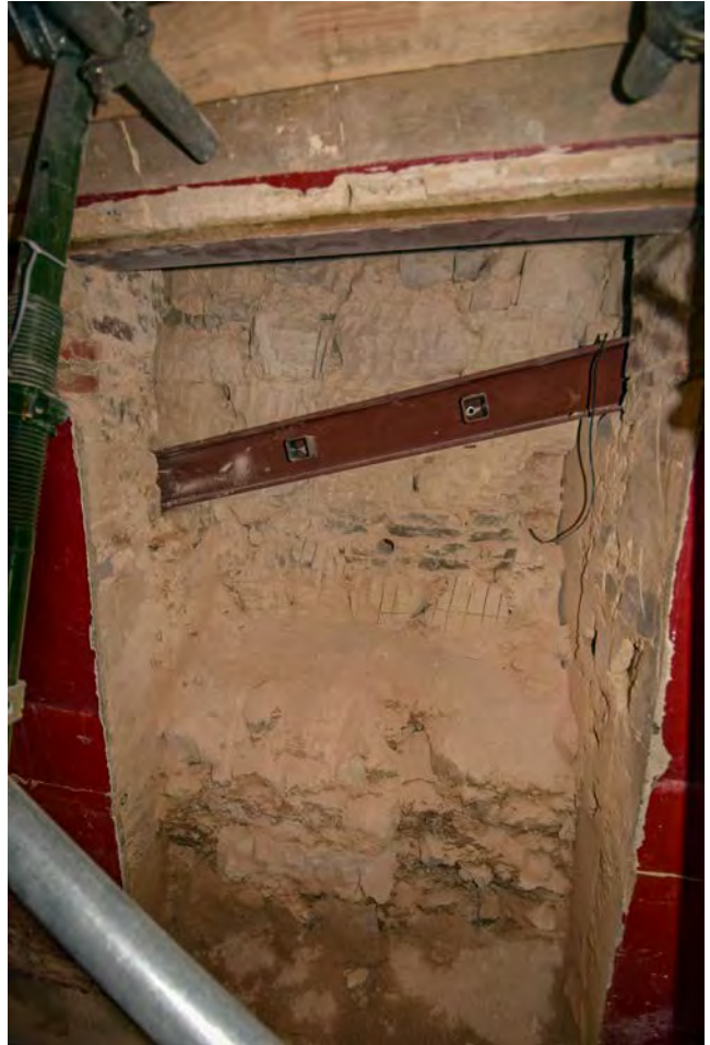
Plate 39: Doorway being created in east wall of passage
