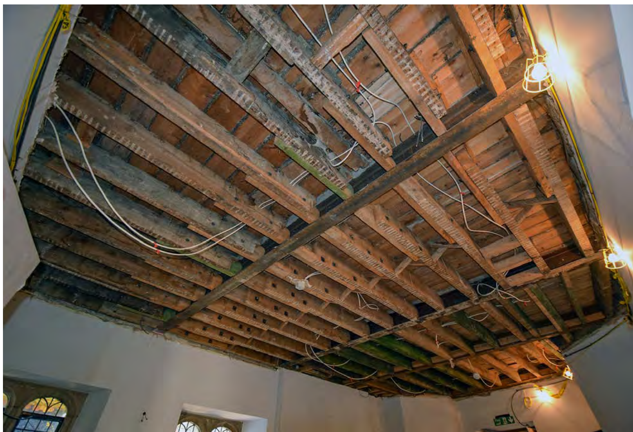
Plate 63: Underside of first floor above Ante Room
