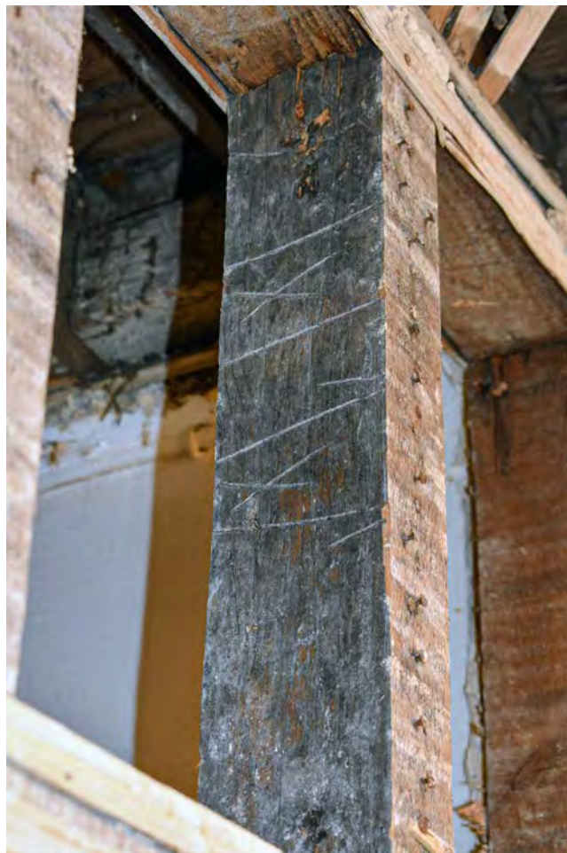
Plate 94: Baltic timber marks to first floor frame
