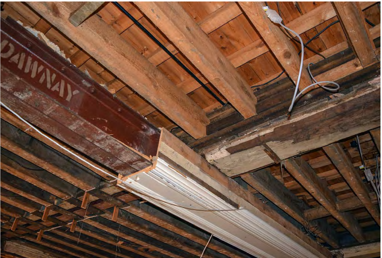
Plate 26: Exposed floor in Old Bursary looking north-west
