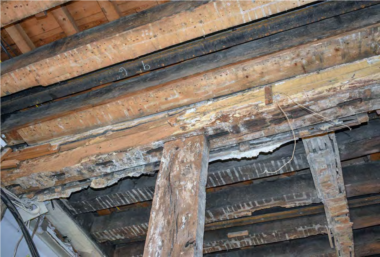
Plate 15: Underside of head rail showing empty mortices
