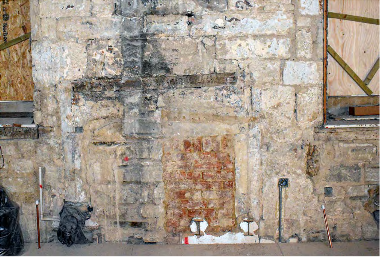
Plate 107: Exposed fireplace in east wall of first floor of Chaplains
