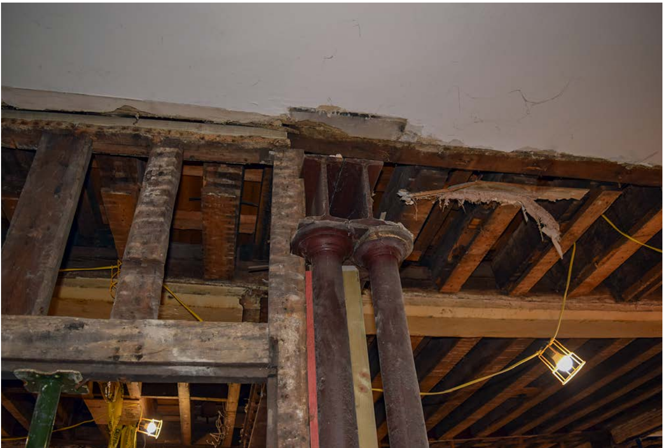
Plate 24: Cast iron columns inserted in 1950s
