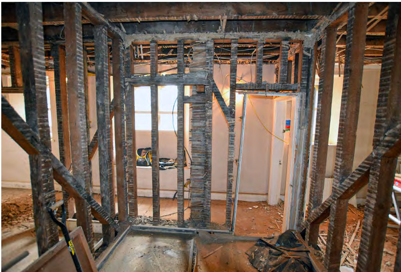
Plate 89: Exposed first floor partition with inserted doorway
