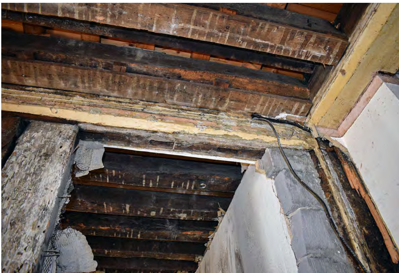
Plate 10: Northern end of head rail
