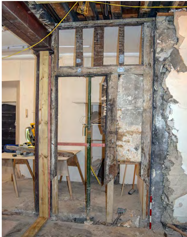
Plate 21: 16th-century frame after works to raise it
