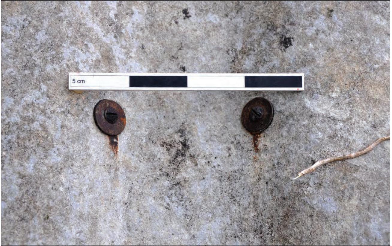
Plate 5: Detail of external fixings
