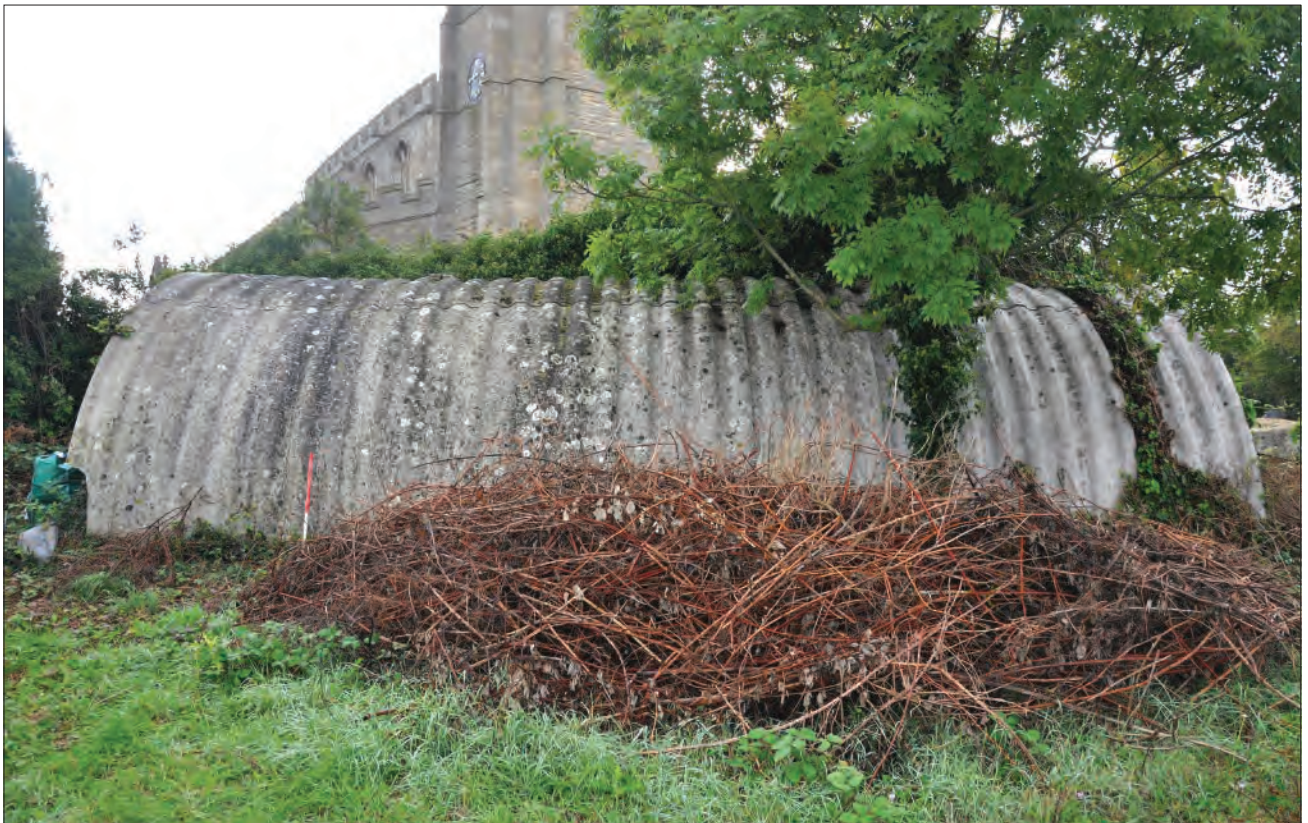
Plate 6: North-west facing elevation, looking south-east, showing sheets of corrugated asbestos
