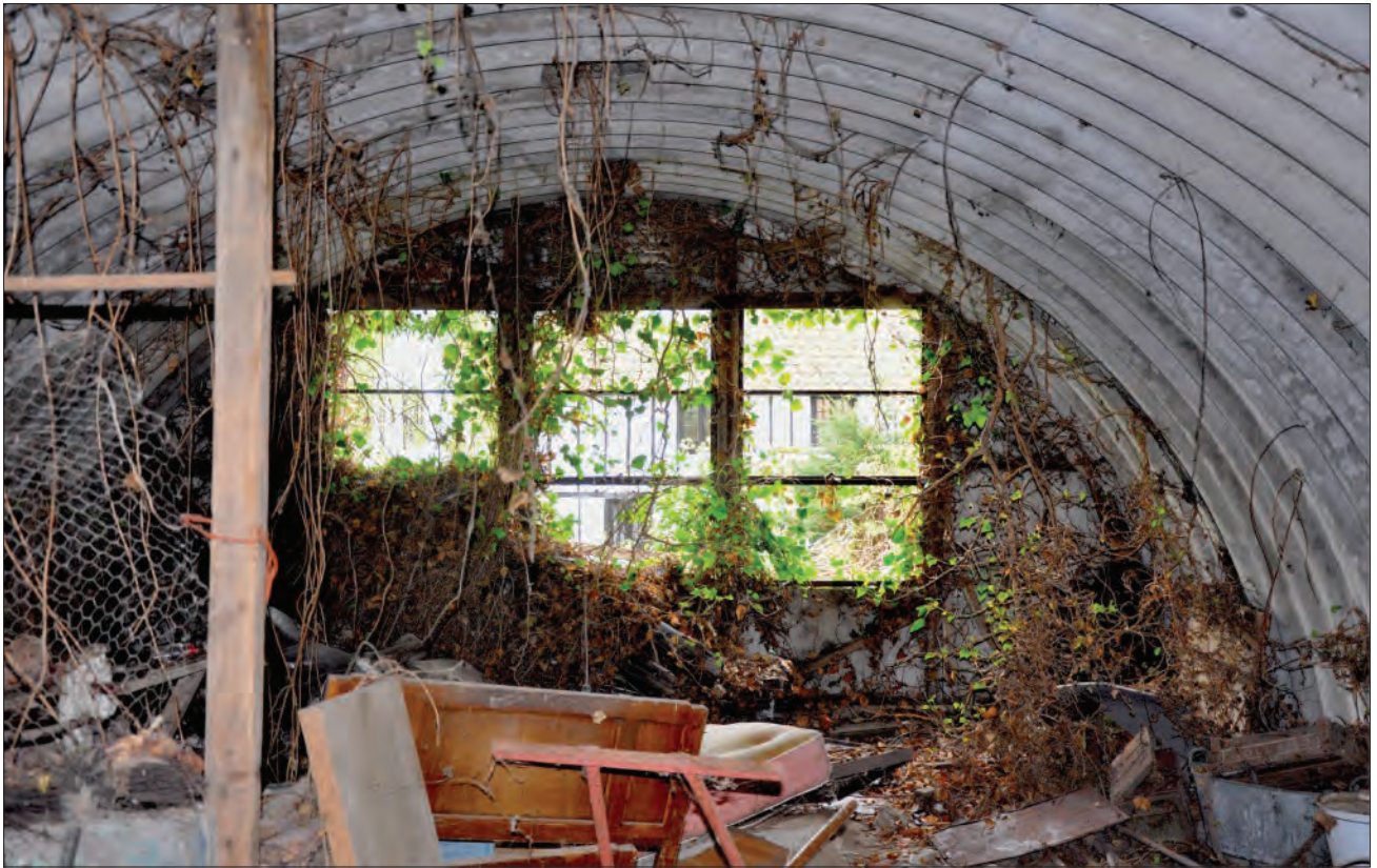
Plate 16: Internal view, looking southwest
