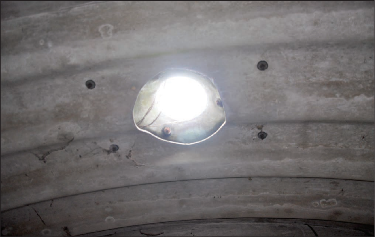
Plate 18: Detail of opening in the roof
