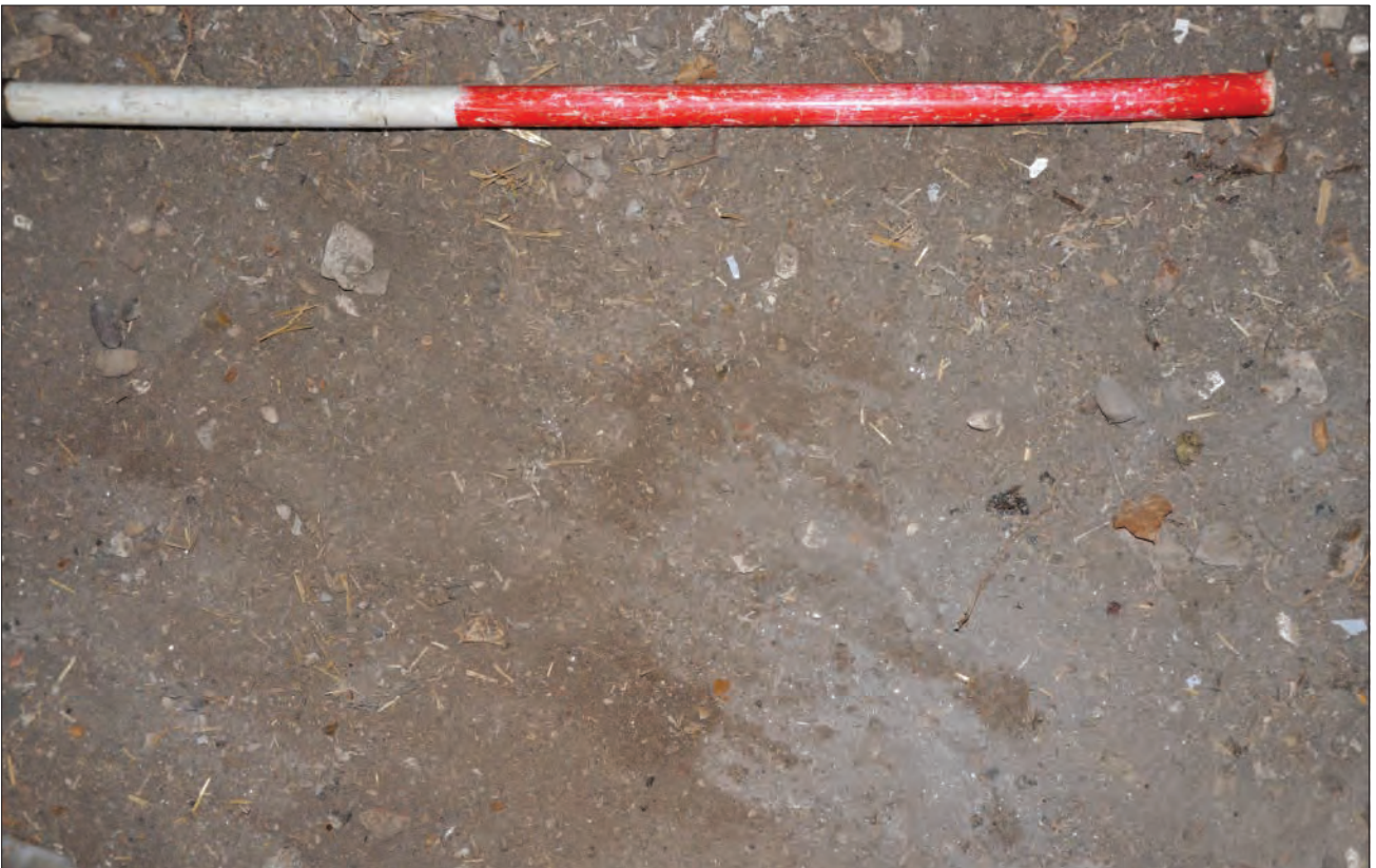
Plate 19: Internal earthen floor
