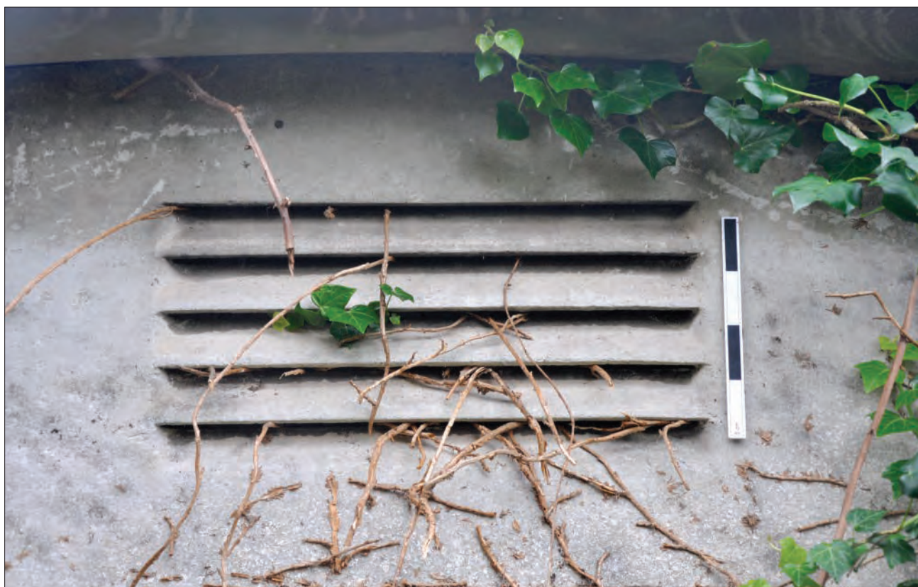
Plate 13: Detail of vent above door on the northeast facing elevation
