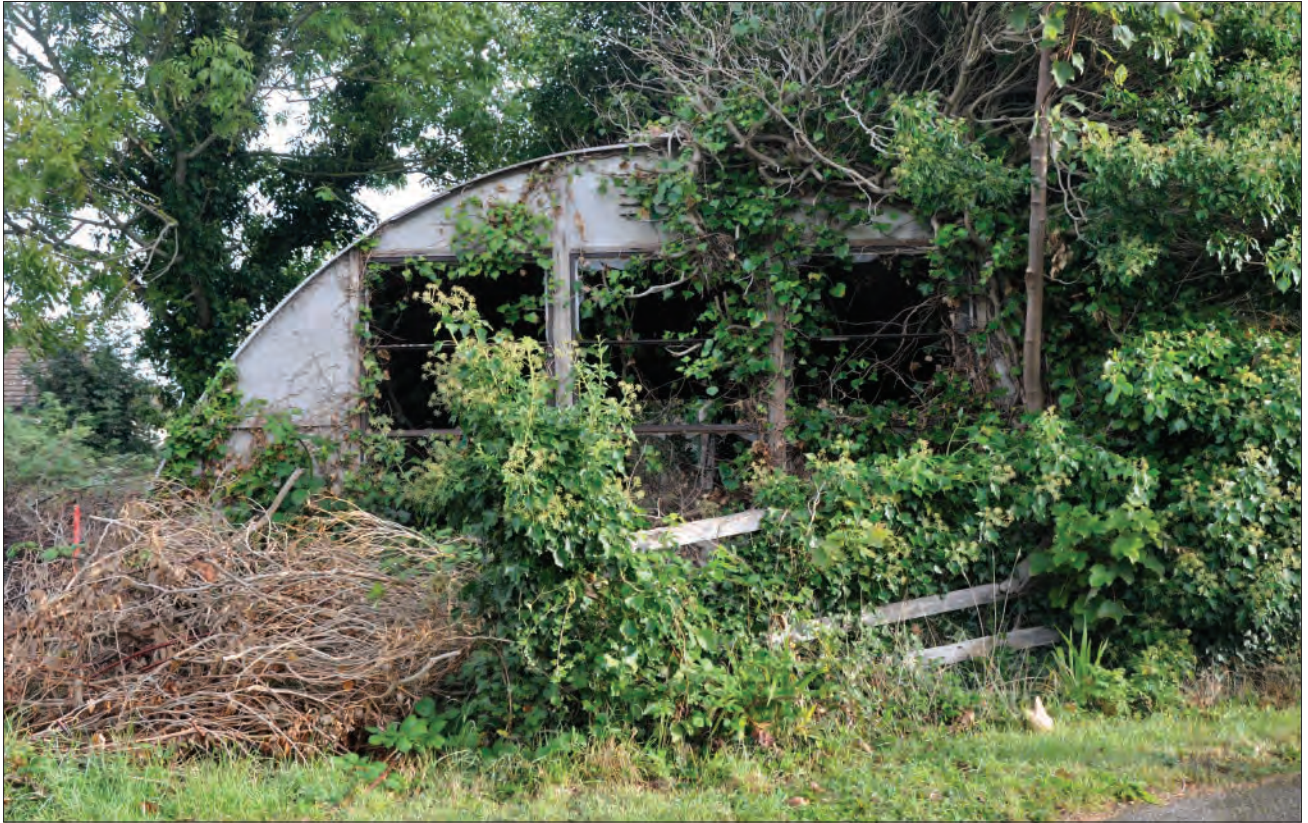
Plate 14: Southwest facing elevation, looking northeast
