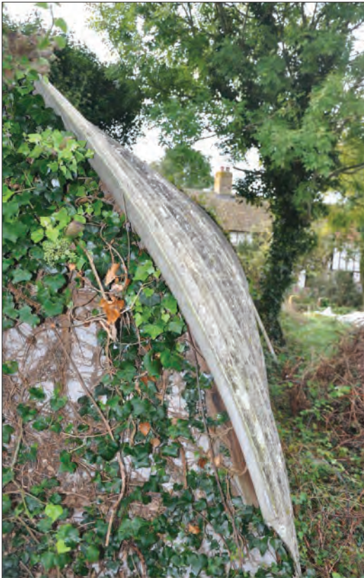
Plate 4: Detail of curved asbestos sheeting, looking south-west
