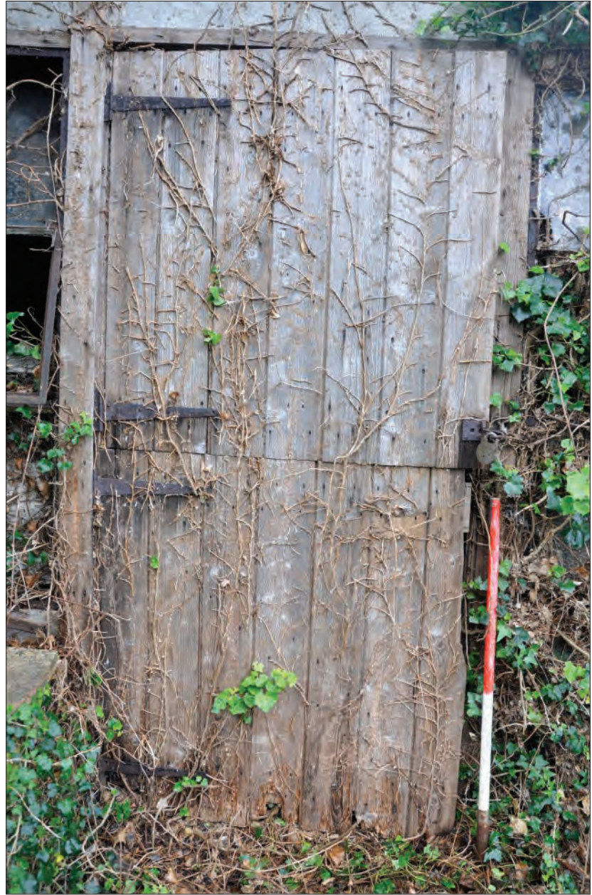
Plate 10: Detail of door, external view
