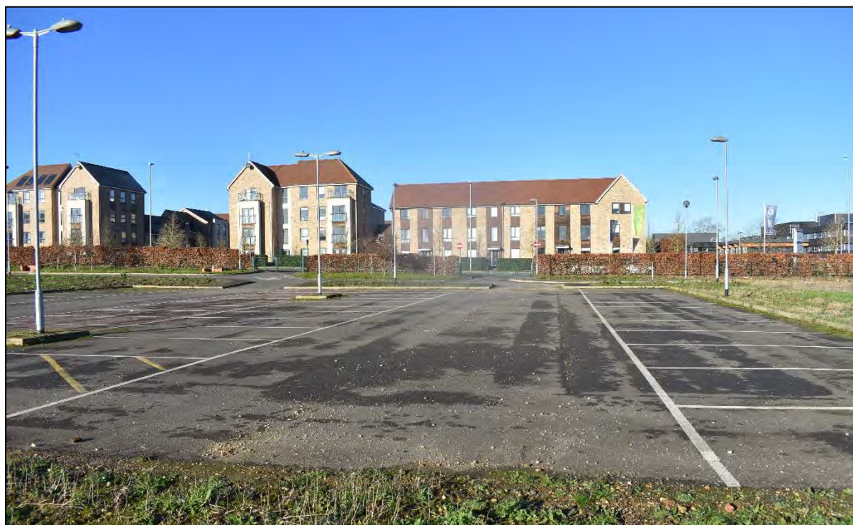
Plate 11: The northern carpark area with associated lighting all the way round and through the middle, looking north-west
