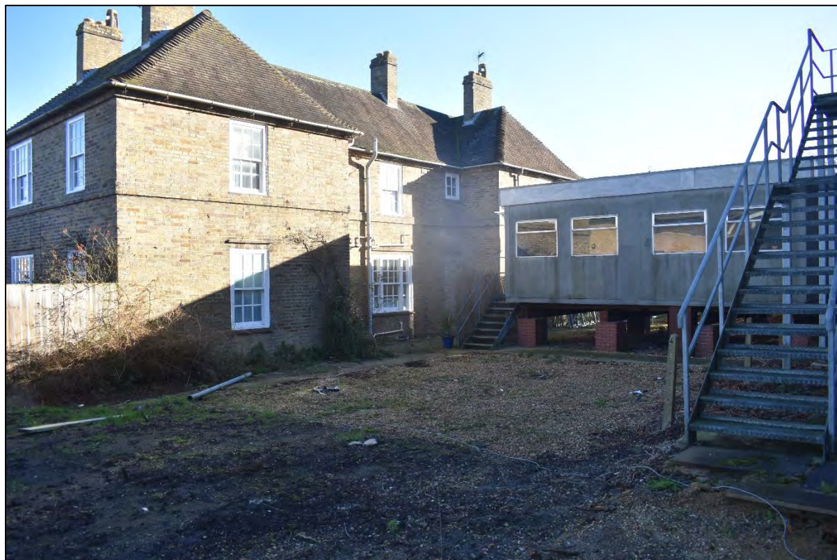
Plate 5: The area between the 1955 building and 14-15 Howes Place where it appears a raised building has been removed, looking north-east
