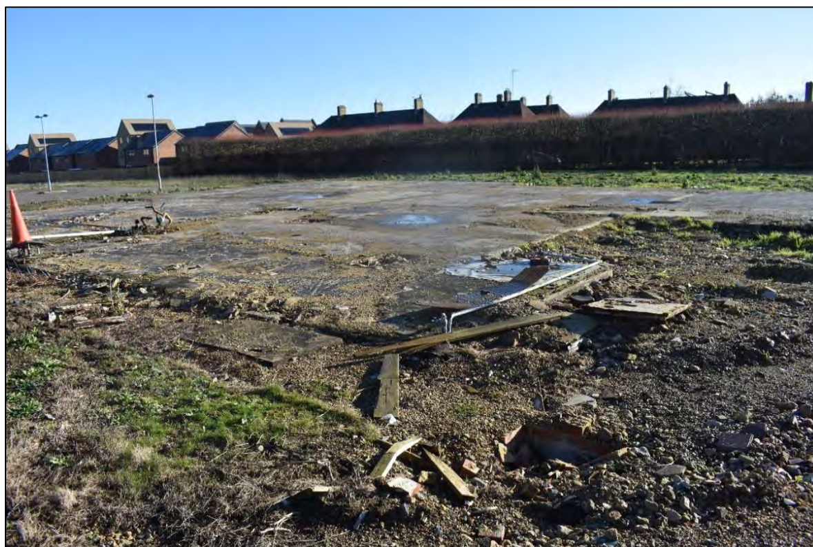
Plate 6: The concrete footing of a demolished structure, showing some of the disturbance that goes below ground-level, looking north-east
