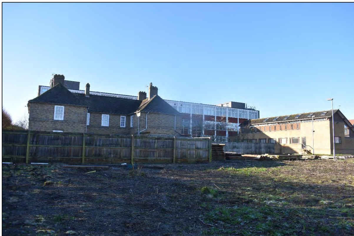
Plate 13: The back of the 1955 building and side of 14-15 Howes Place, both expected to be demolished as part of the development, looking south-west
