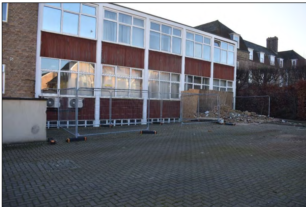
Plate 4: The 1955 building extending below ground-level, with a manhole cover in the foreground, looking south
