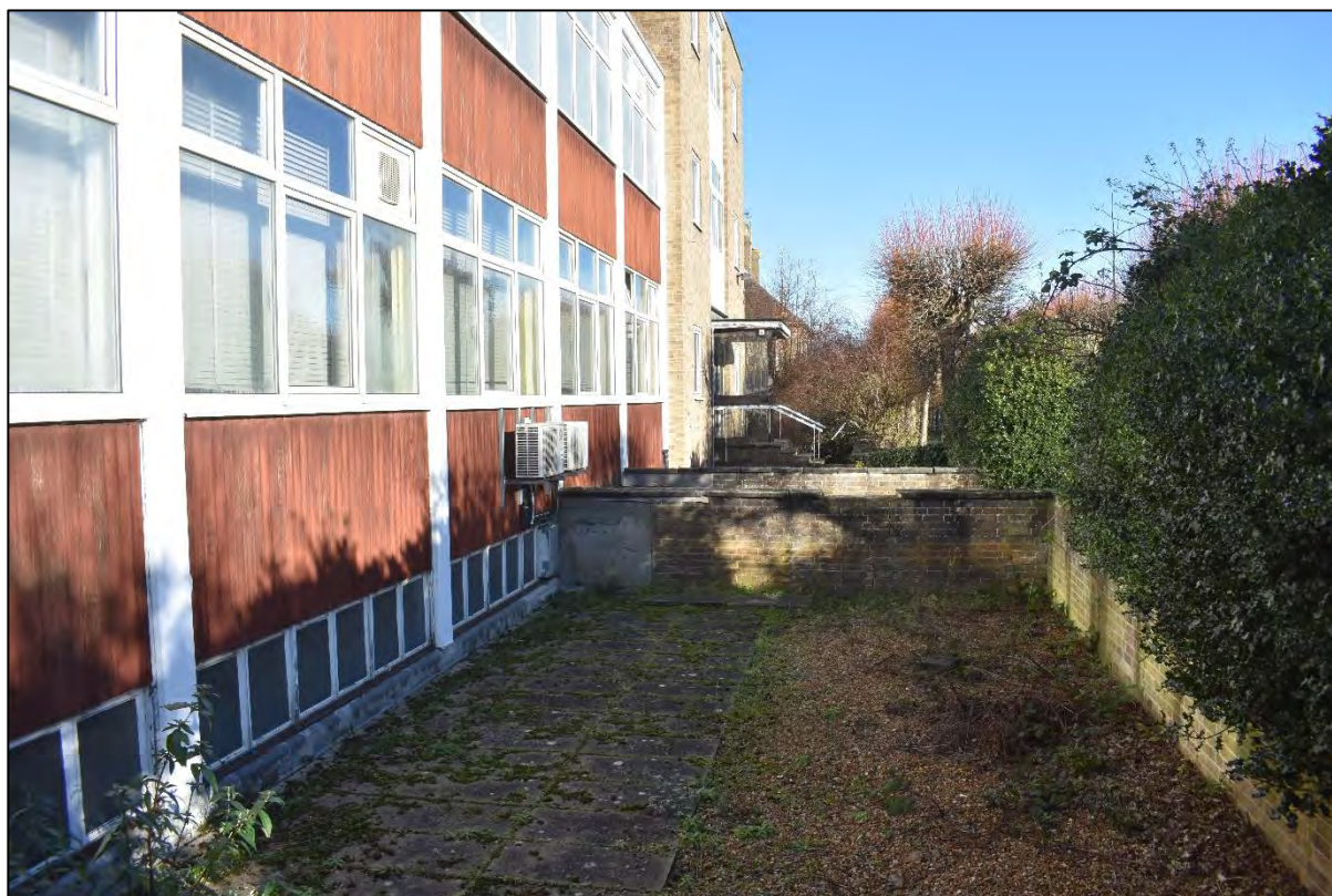
Plate 12: The south-eastern side of the 1955, building showing the narrow strip of land outside the building footprint, which itself is affected by access points and landscaping. Looking north-east
