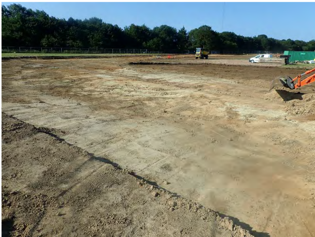
Plate 2. Pond 9 (view to south)
