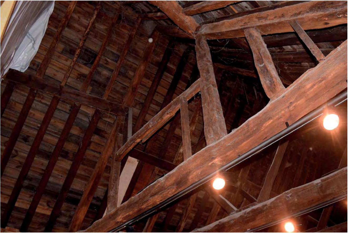
Plate 45: Truss 1 looking north-east
