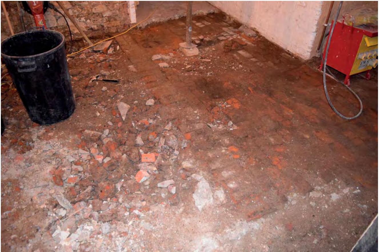
Plate 36: Features [1] in basement floor looking SE
