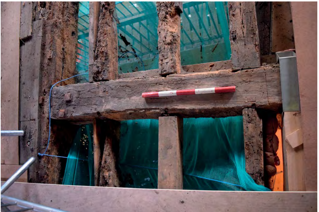
Plate 30: Joists in Area O looking west
