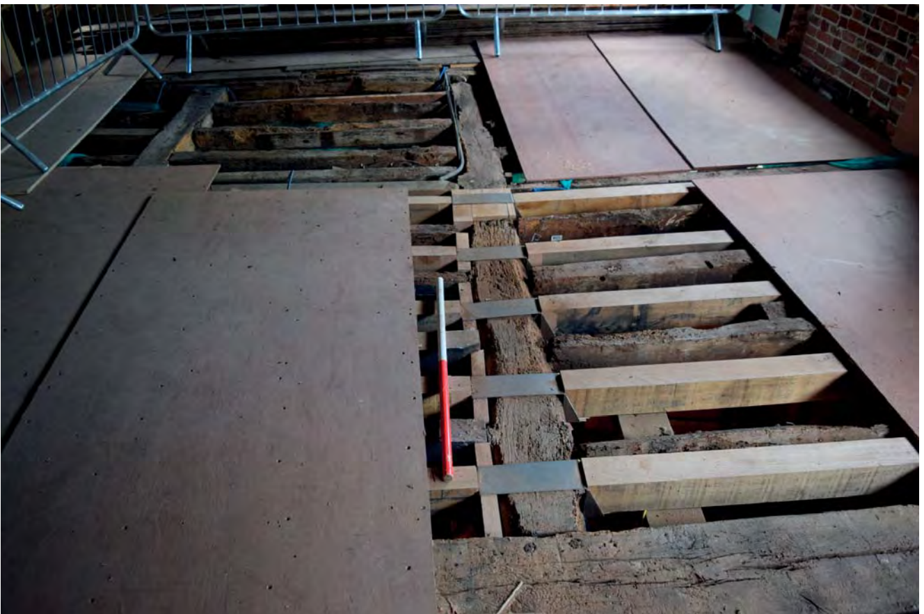
Plate 28: Floor looking west; Areas M, O, QM
