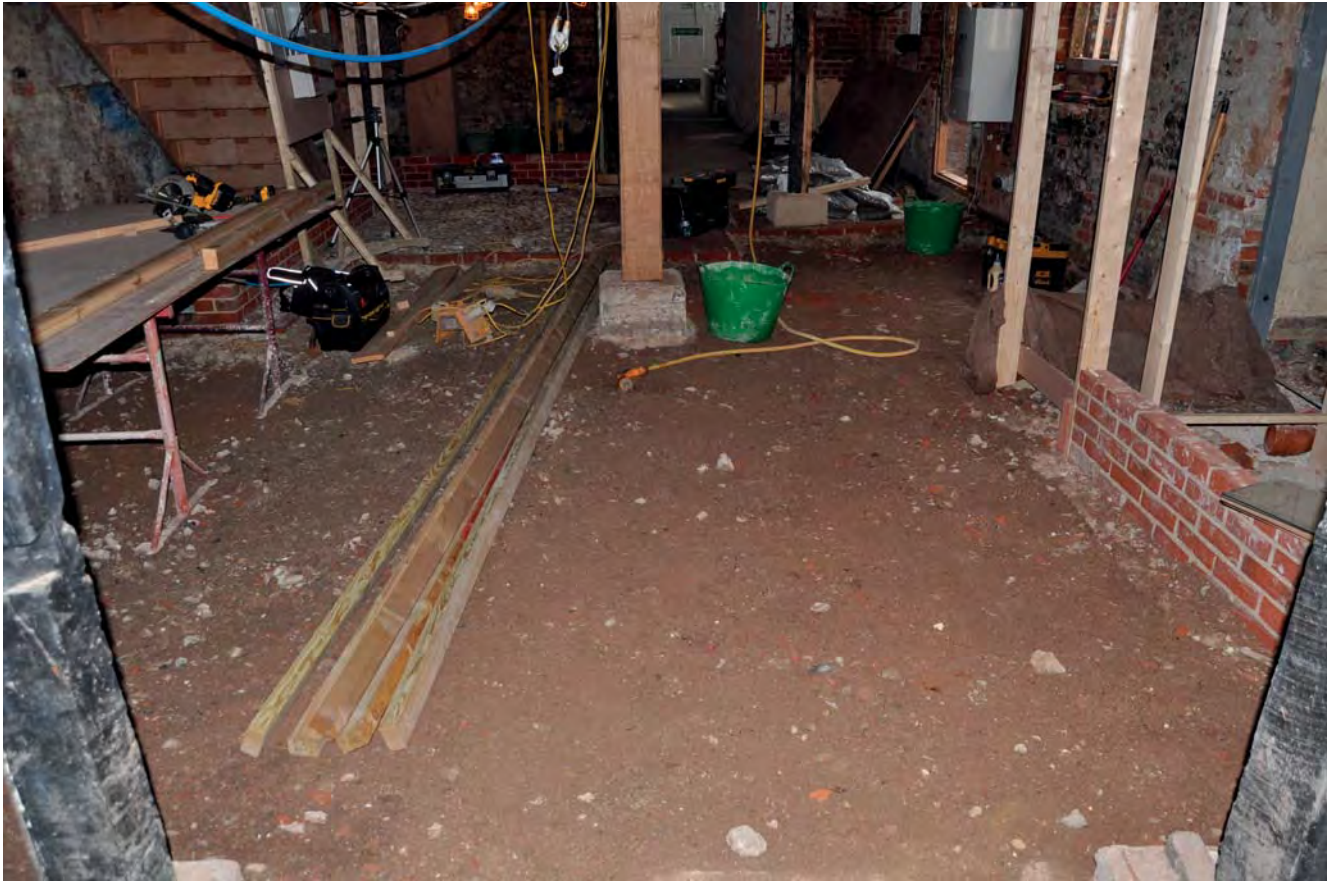
Plate 41: Floor towards west end of basement
