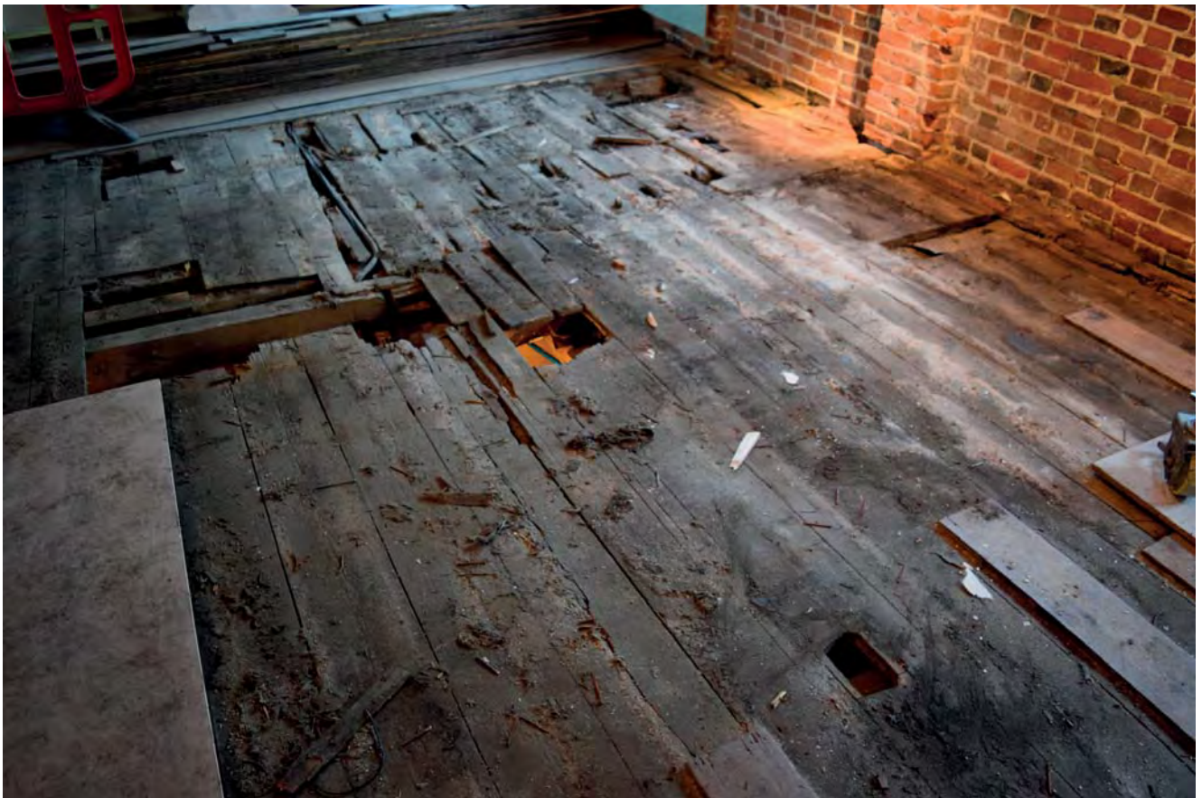
Plate 2: Floorboards at ground floor level prior to removal, looking north-west
