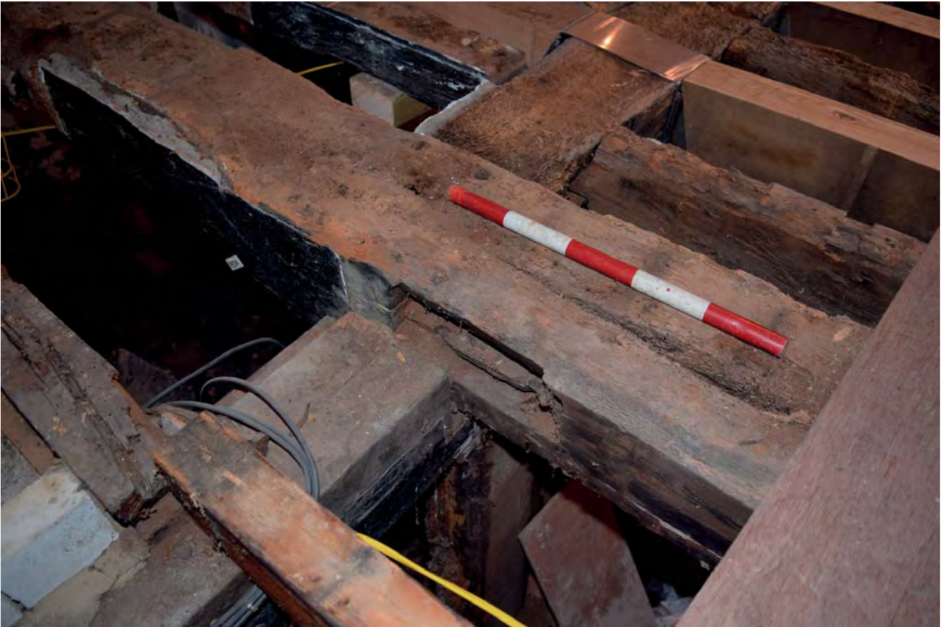
Plate 25: Mortise in beam 105 (Area G) looking south-west
