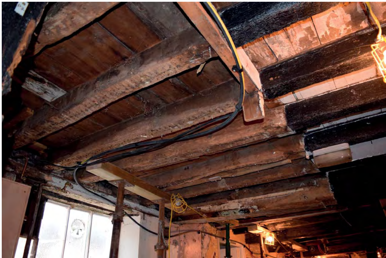
Plate 12: Recently exposed joists in Area G looking south-west
