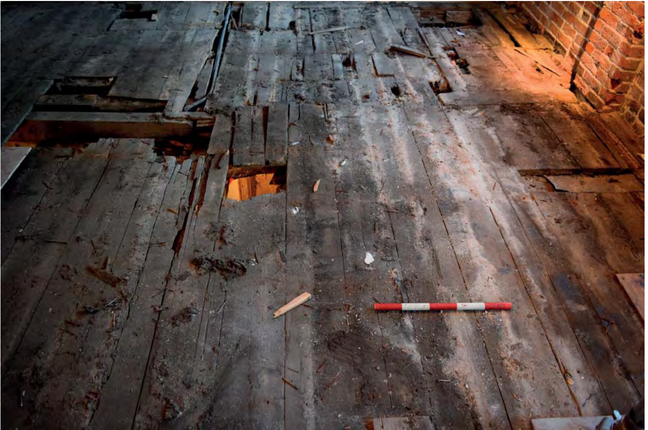
Plate 3: Exposed ground floor joists
