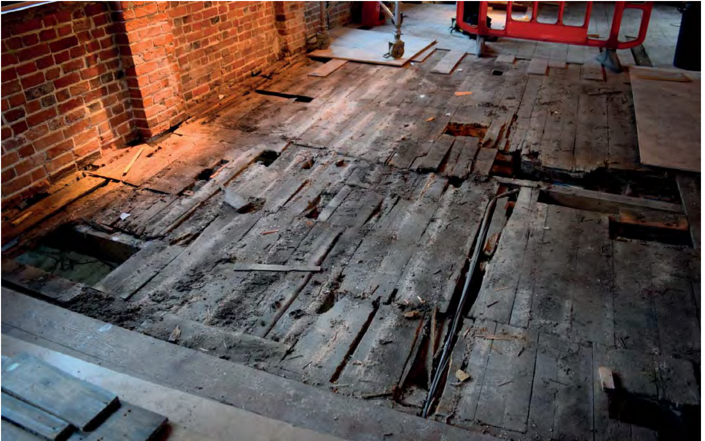
Plate 1: General view of ground floor floorboards looking east
