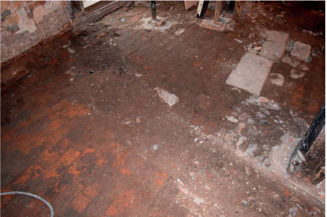
Plate 33: Infilled channel in basement looking SW
