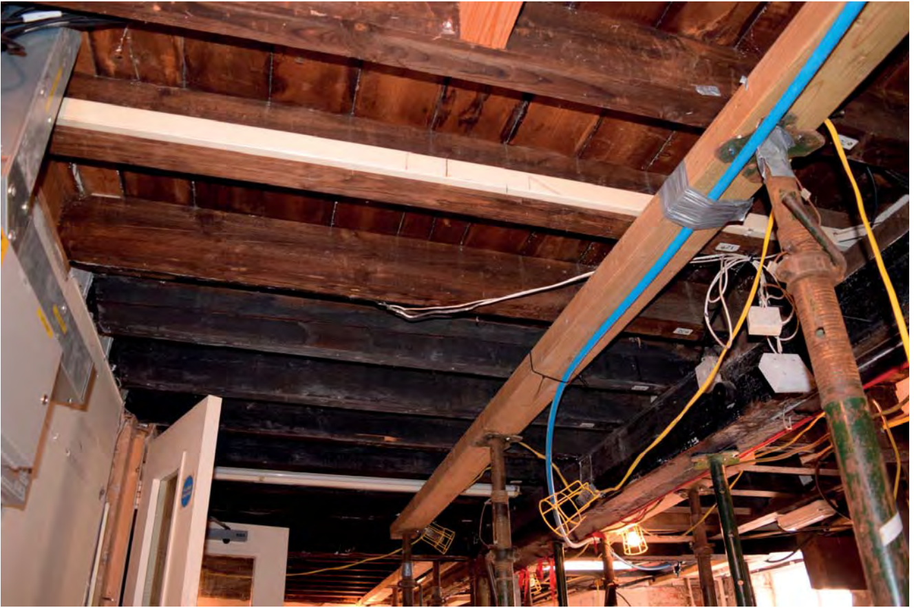
Plate 13: Underside of ground floor joists in Area H looking east
