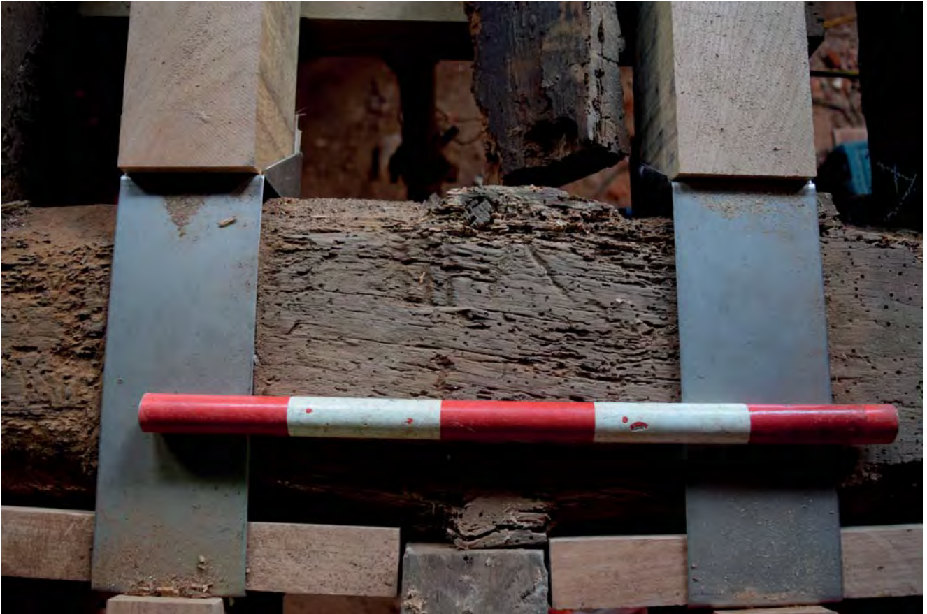
Plate 29: Mark on joist 110, by joist 70, in Area N
