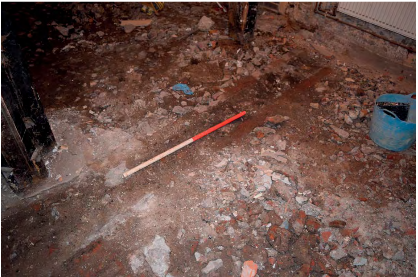
Plate 32: Floor in basement looking NW
