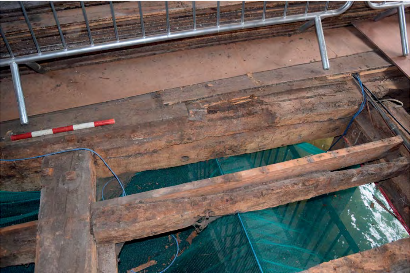
Plate 23: Trench mortice in beam III (Area Q) looking west
