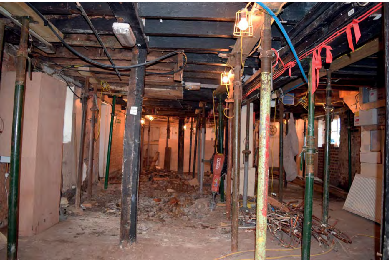
Plate 8: Basement looking west
