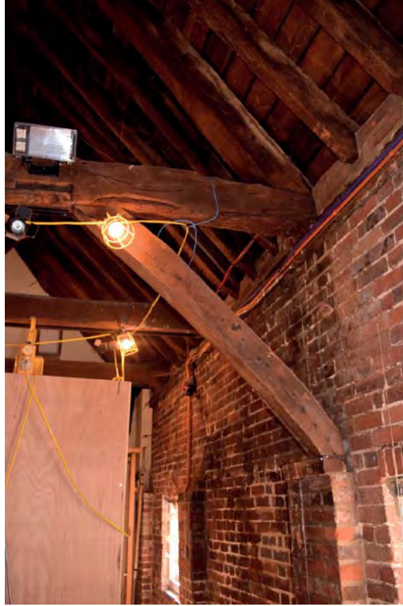
Plate 53: South end of Truss 4 looking east
