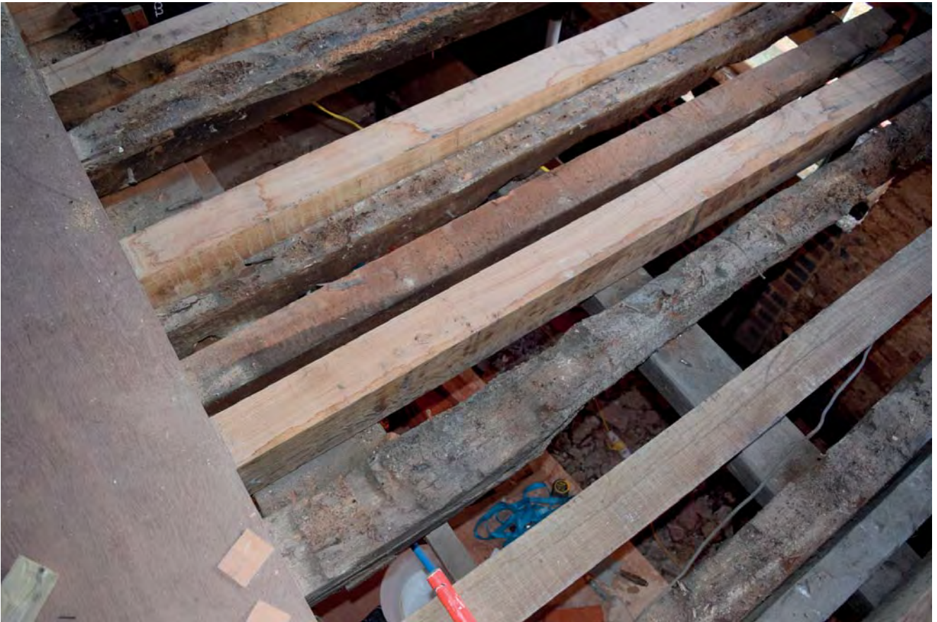
Plate 20: Joists in Area K looking north-west
