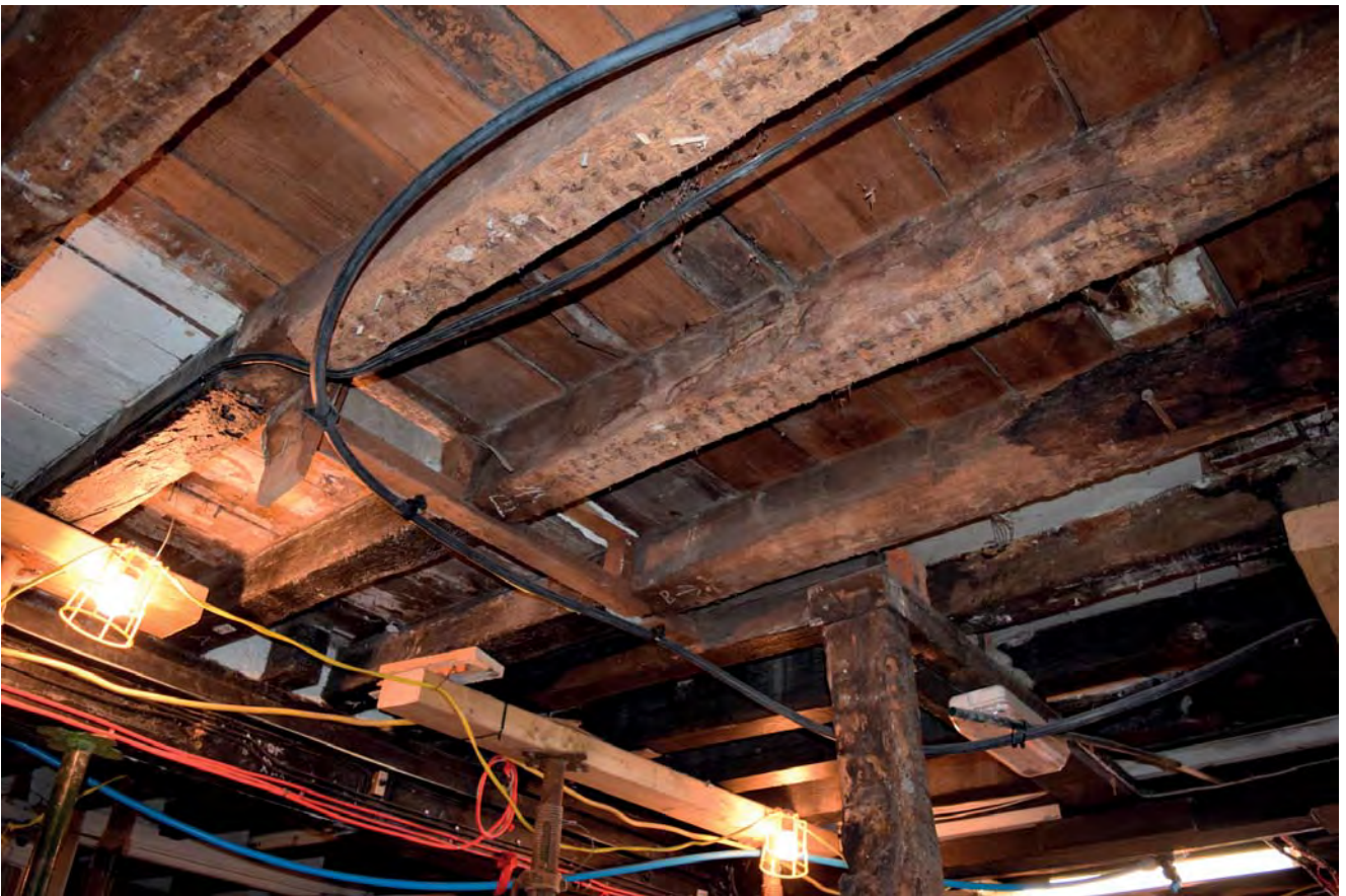
Plate 10: Underside of joists in Area G looking NE towards stairs
