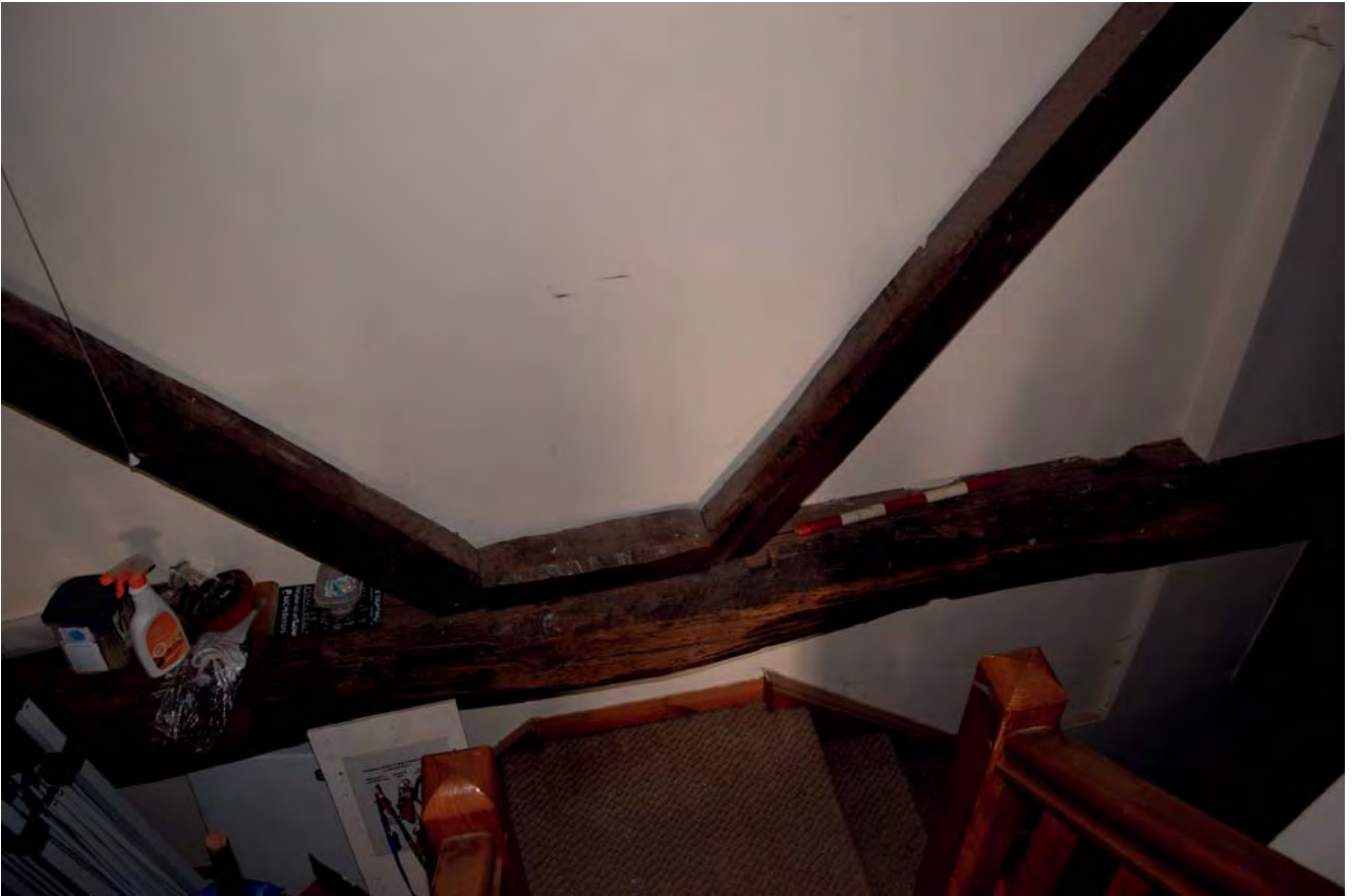
Plate 57: Top of easternmost truss (Truss 6)
