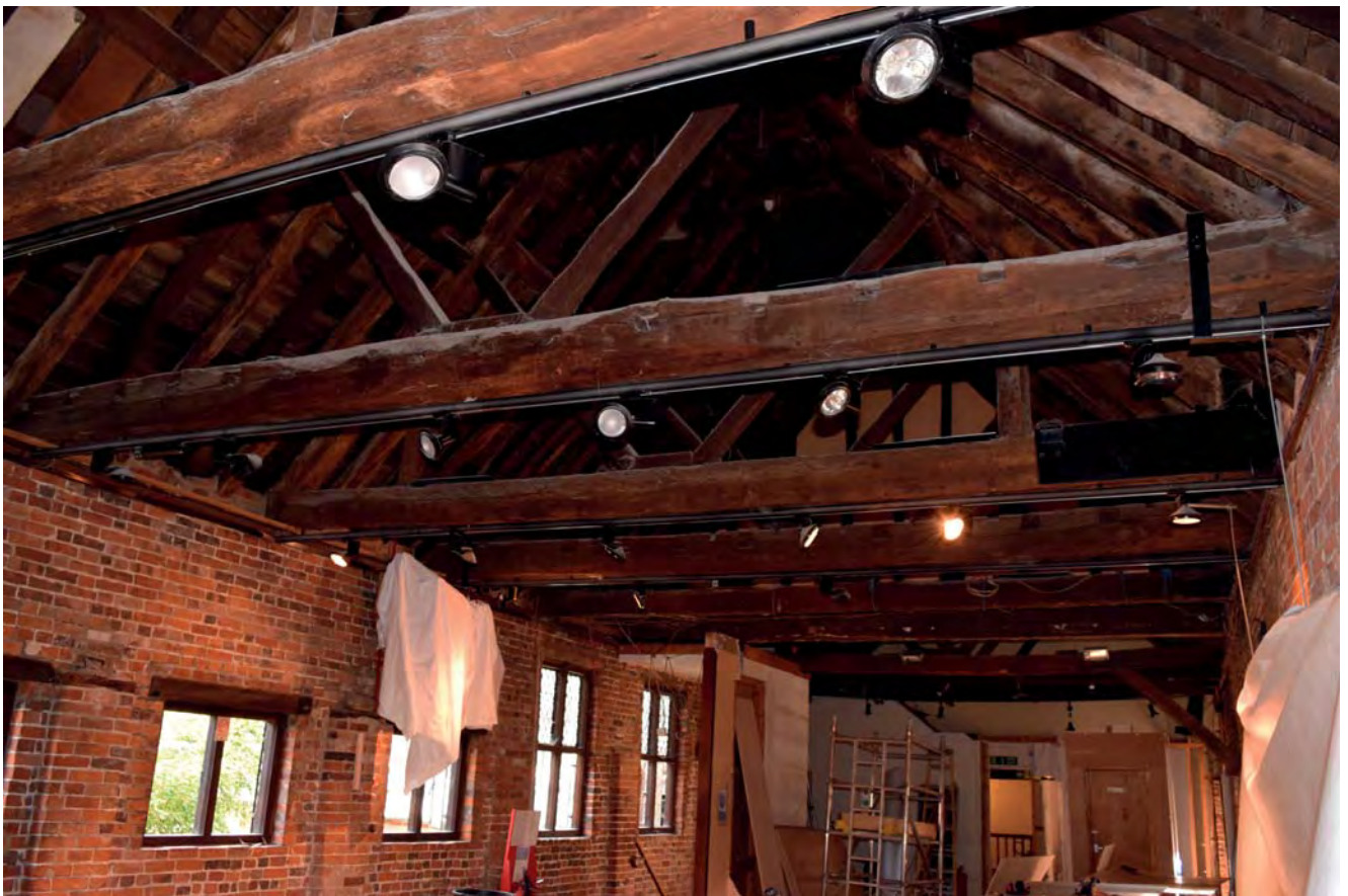
Plate 44: General view of roof looking east
