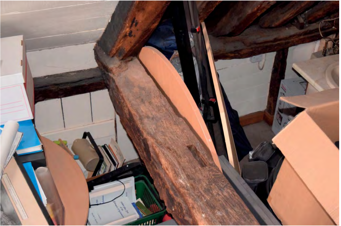
Plate 61: Mortise in top of tie of easternmost truss (Truss 6)
