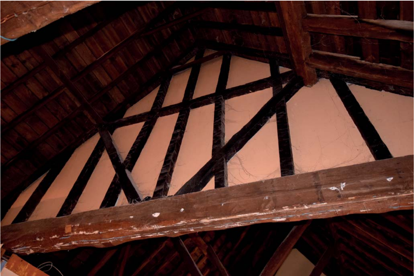
Plate 51: Closed intermediate truss at centre looking east
