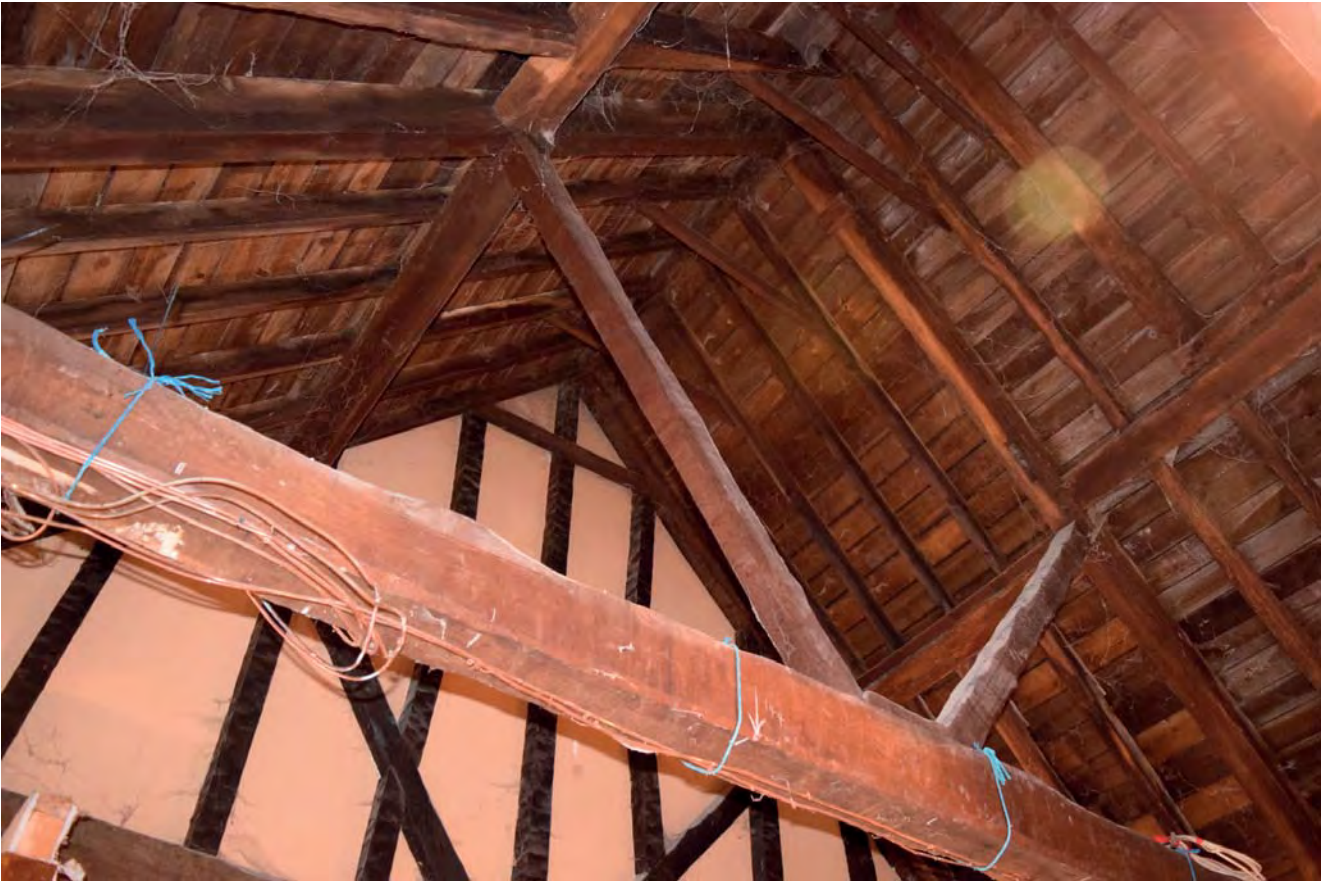
Plate 49: Truss 3 looking south-east
