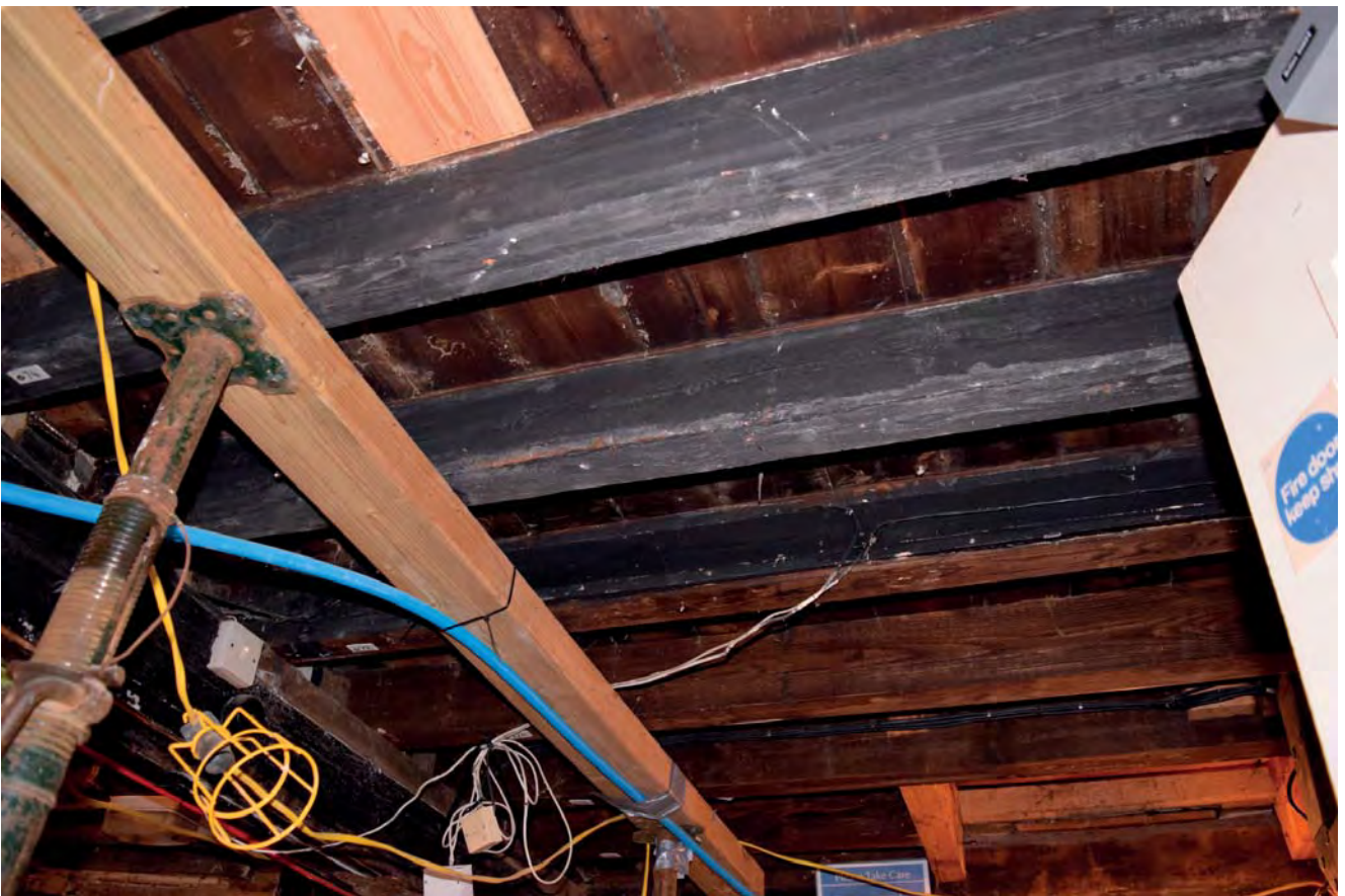
Plate 14: Joists in Area H looking west
