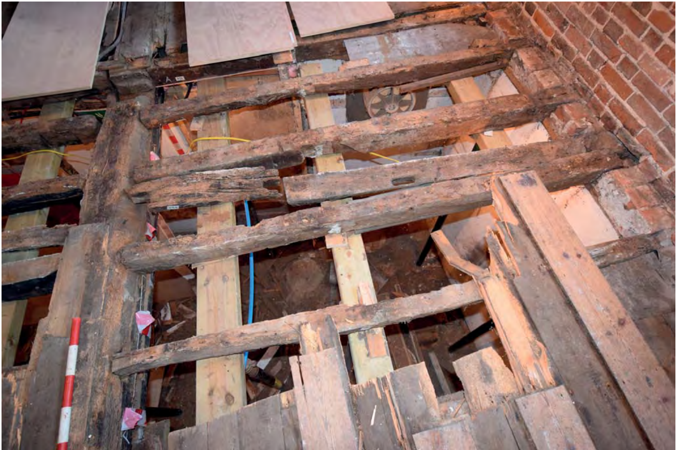
Plate 6: Joists at west end of floor looking west
