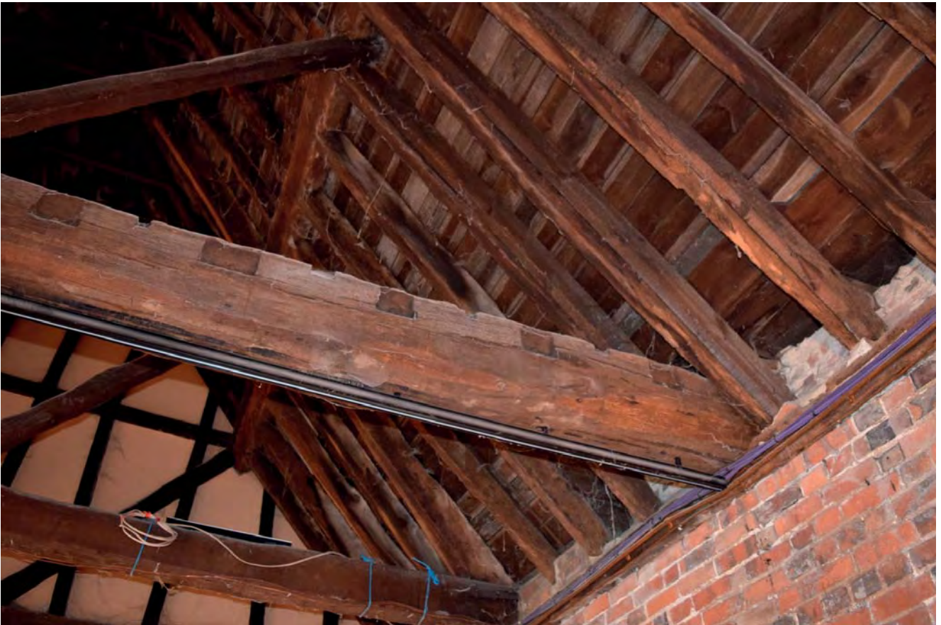
Plate 48: Intermediate truss looking east
