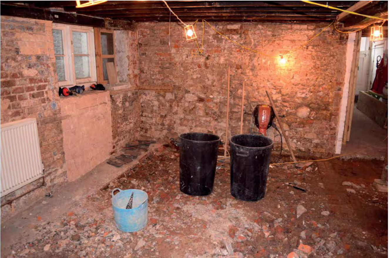
Plate 37: Basement (Area D) looking east
