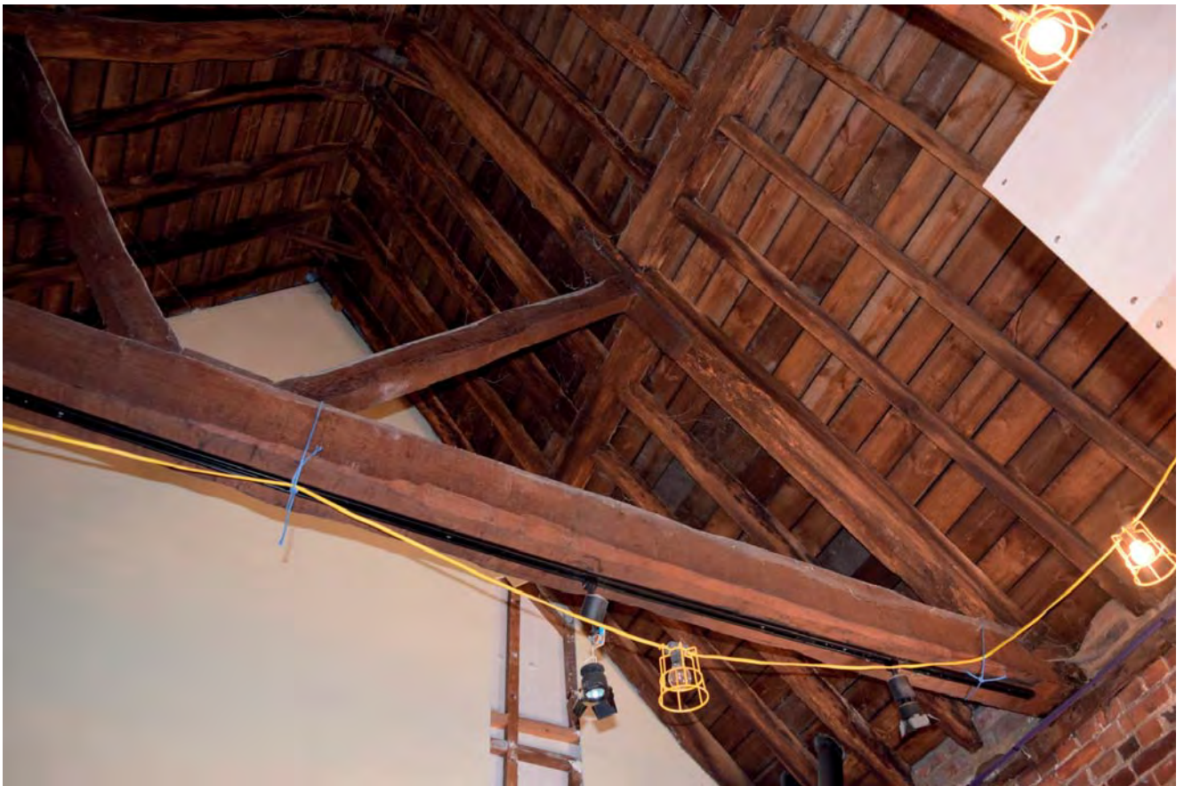
Plate 54: Truss 5 looking east
