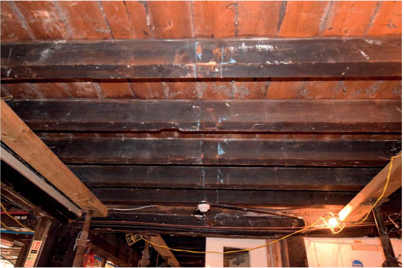
Plate 15: Joists in Area D looking west
