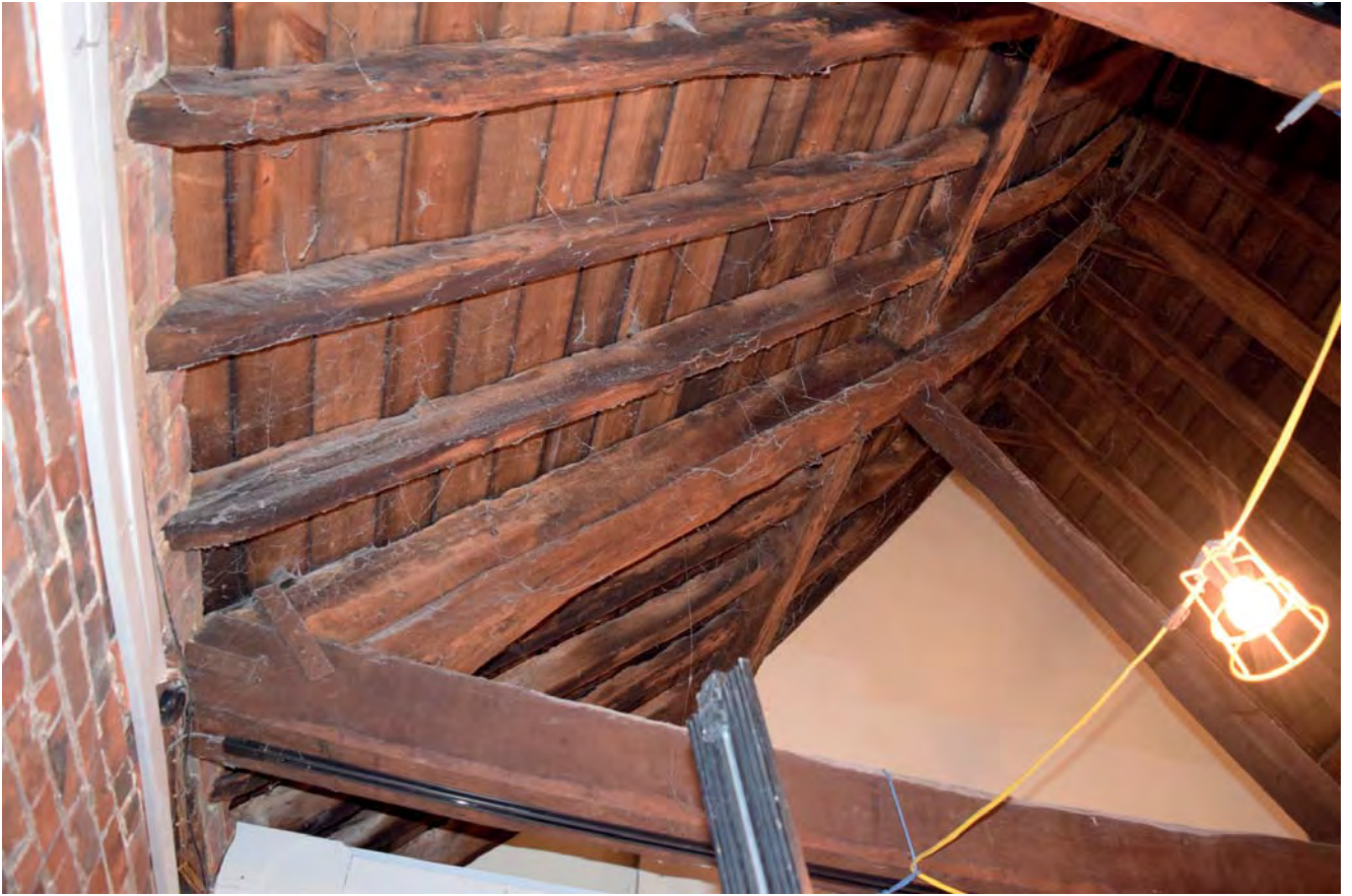
Plate 55: Truss 5 looking east
