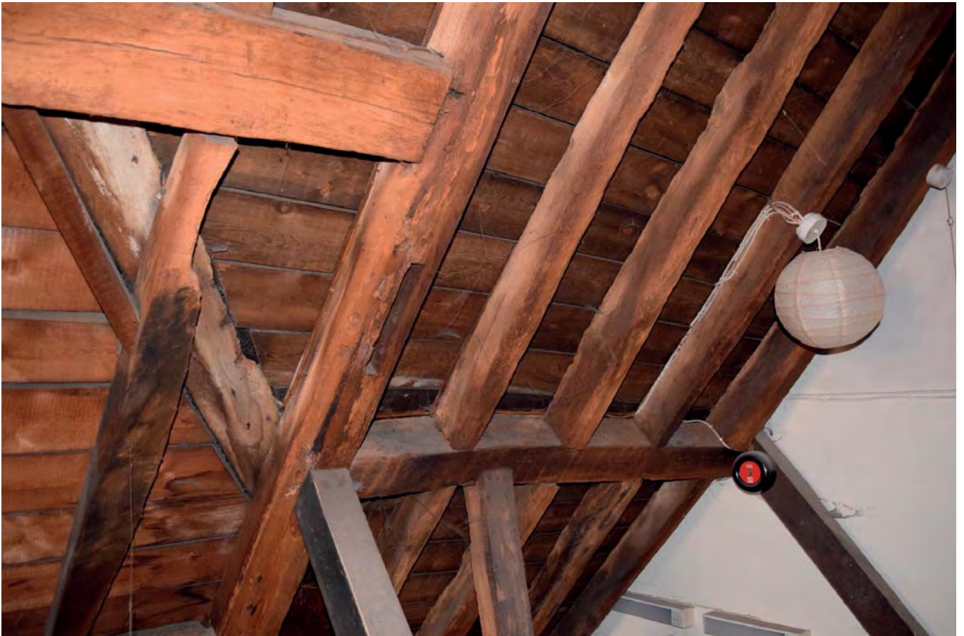
Plate 60: Mortise in principal rafter of easternmost truss (Truss 6)
