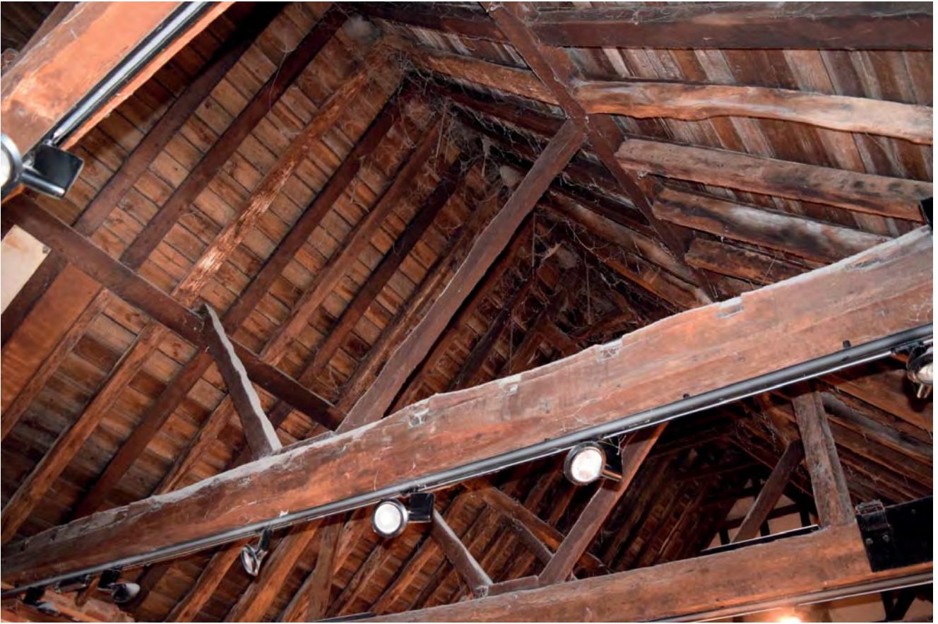
Plate 47: Intermediate truss (T.1.5) looking north-east
