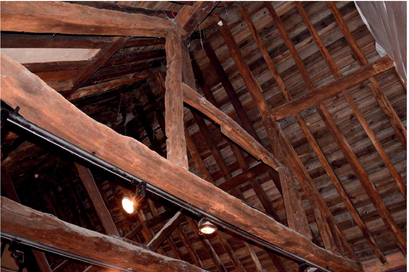
Plate 46: Truss 1 looking south-east
