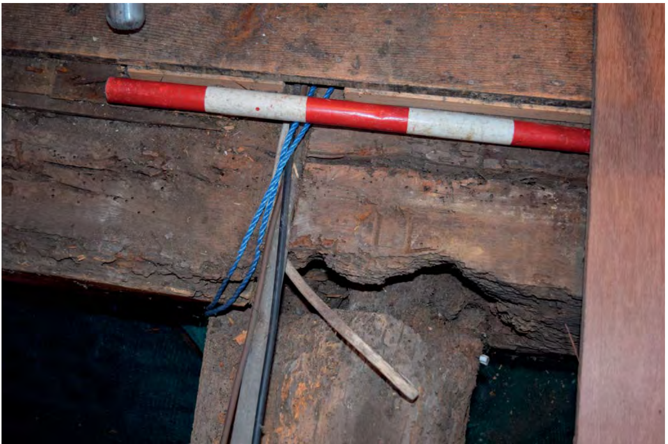
Plate 26: Marks on joist 111 (Area G) looking west
