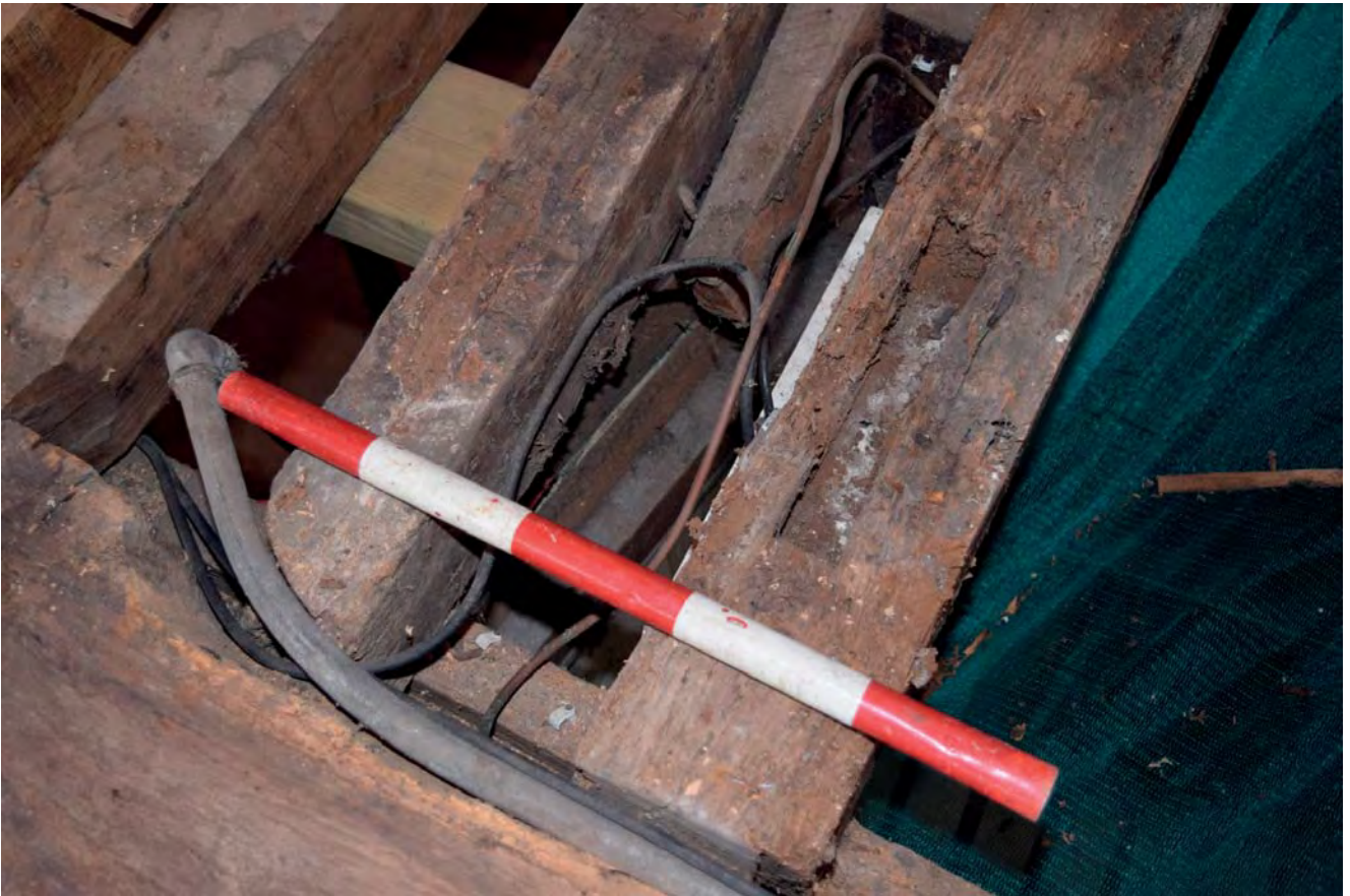
Plate 22: Trench mortise in Joist 79 (Area Q) looking south
