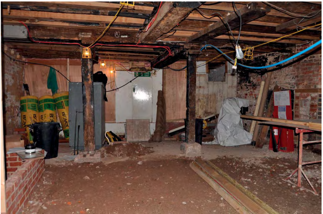
Plate 40: General view of basement looking west
