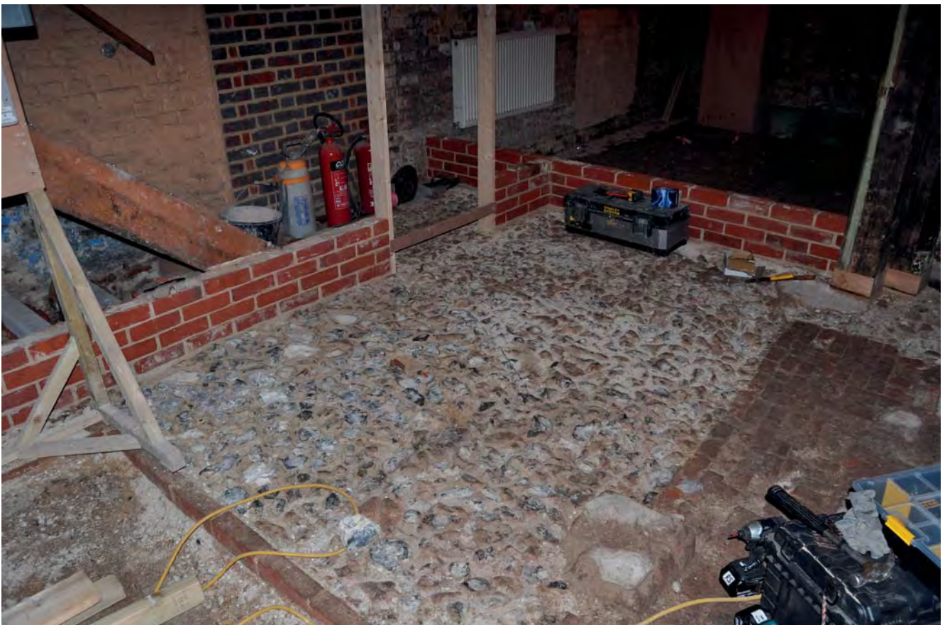
Plate 42: In-situ flint floor after repairs
