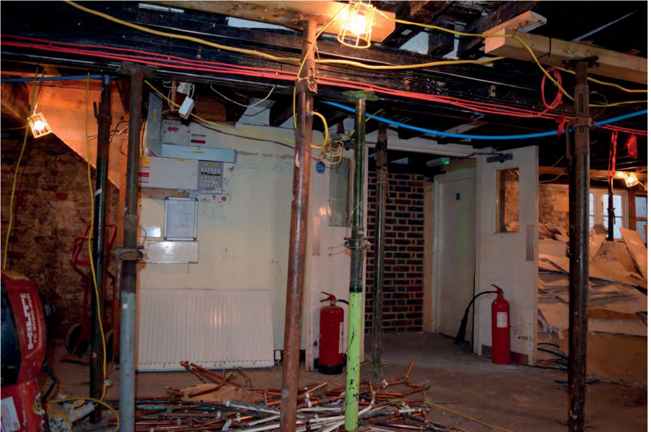
Plate 9: Basement looking north towards foot of stairs
