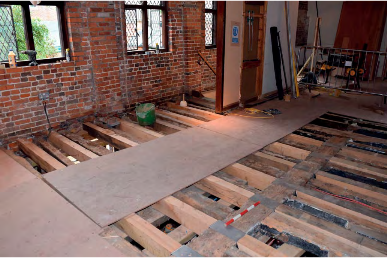
Plate 19: Exposed joists looking north-east
