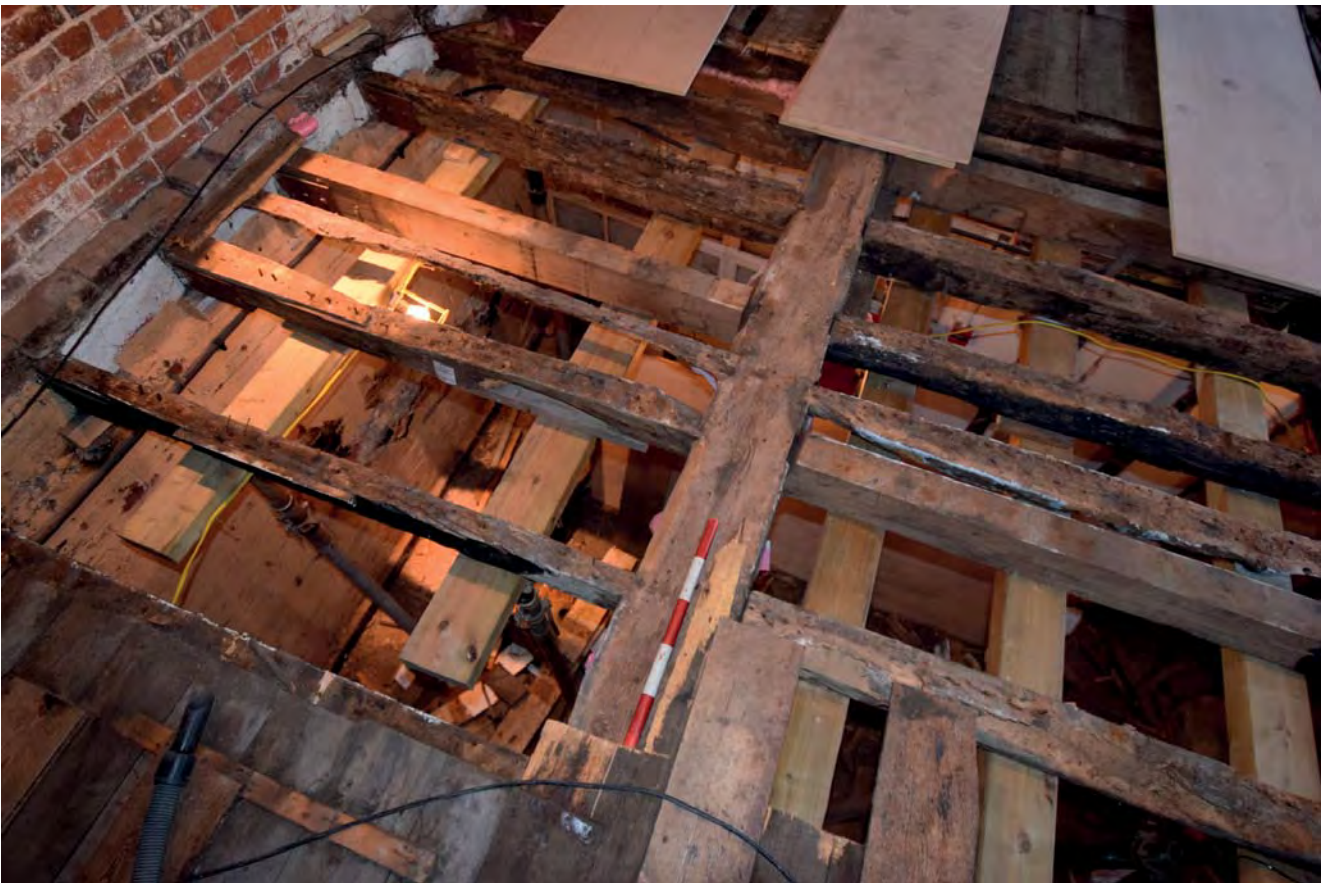
Plate 4: Joists at west end of floor looking west
