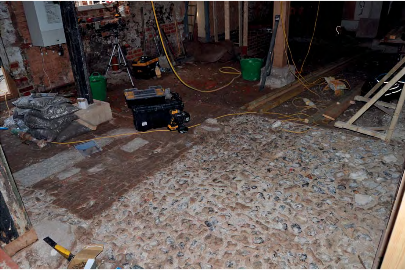
Plate 43: In-situ floor in basement after repairs
