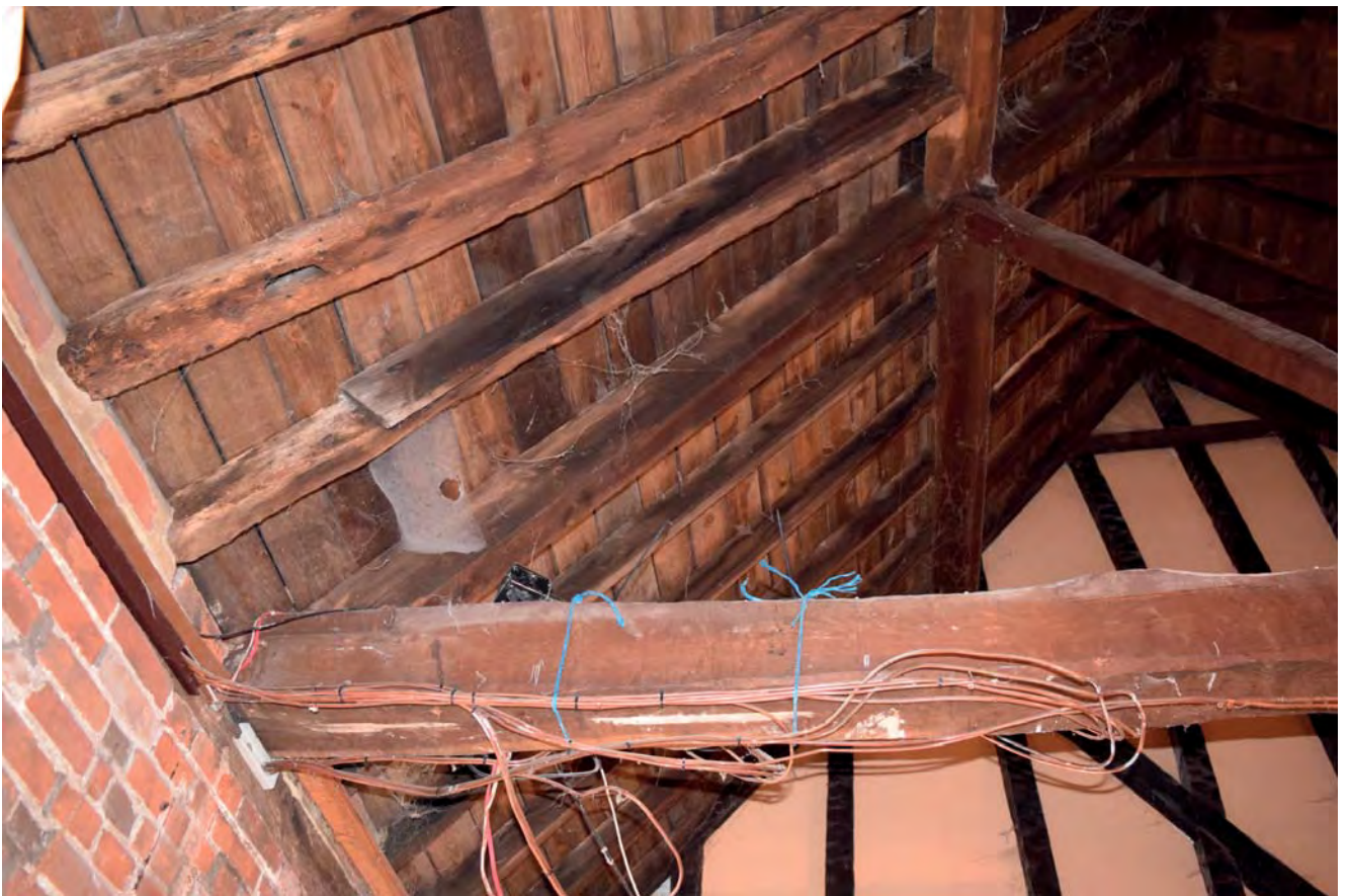
Plate 50: north end of Truss 3
