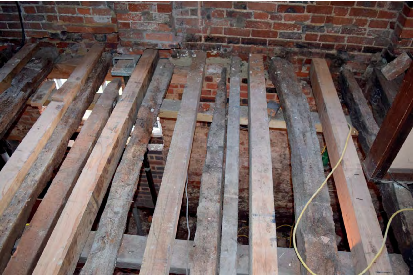
Plate 17: Joists during repair works in Area K looking north
