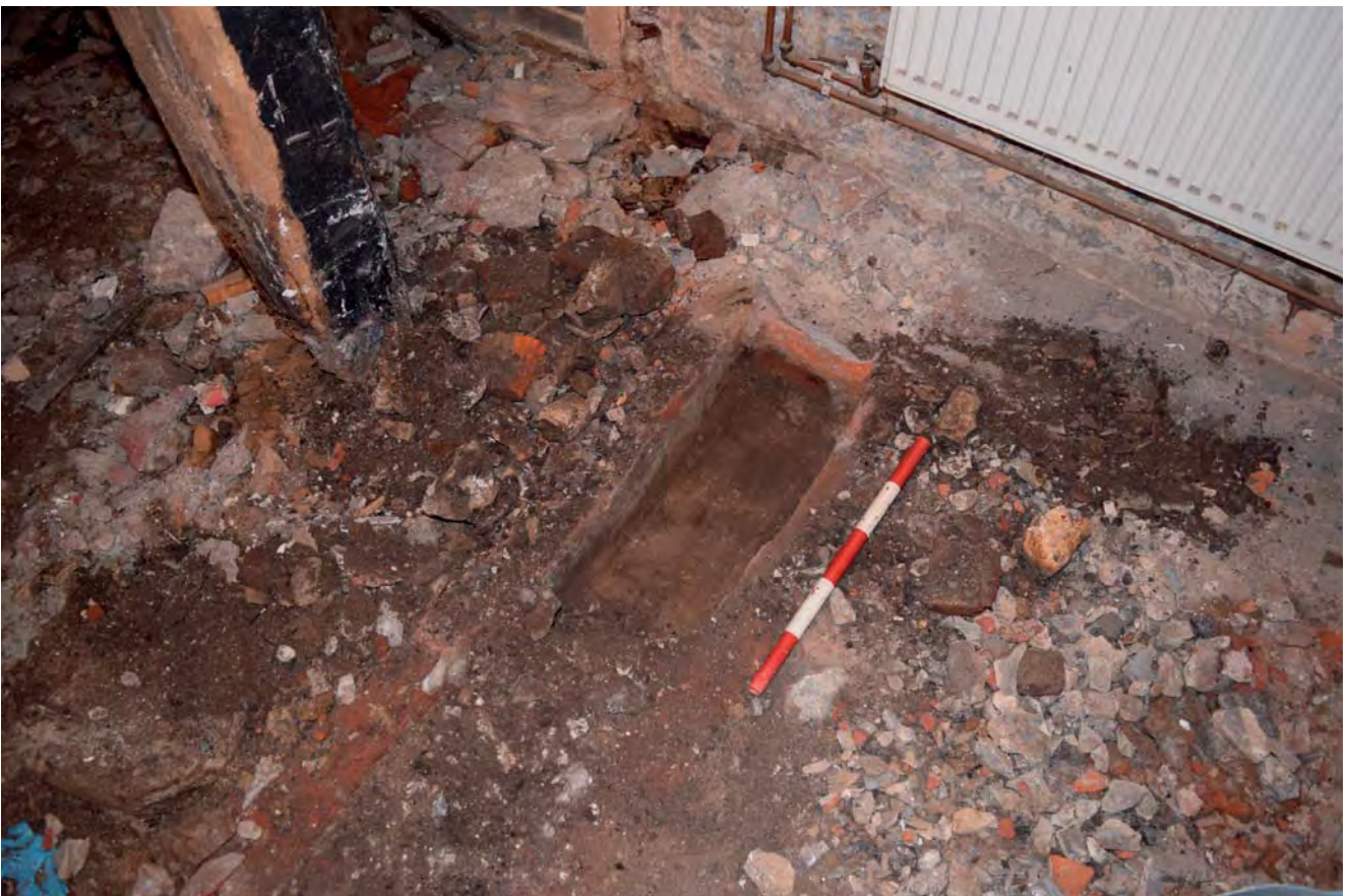
Plate 38: North end of infilled channel in basement
