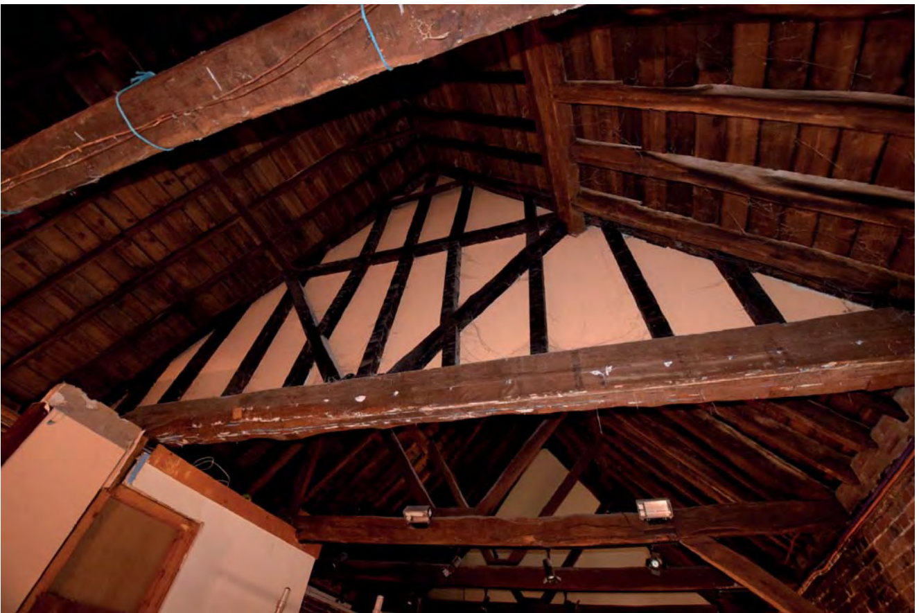
Plate 52: Closed intermediate truss at centre of building looking east
