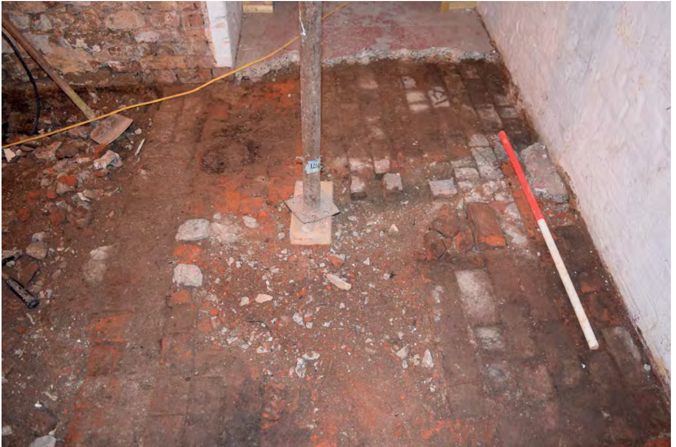
Plate 31: Exposed basement floor looking east (Feature 1)
