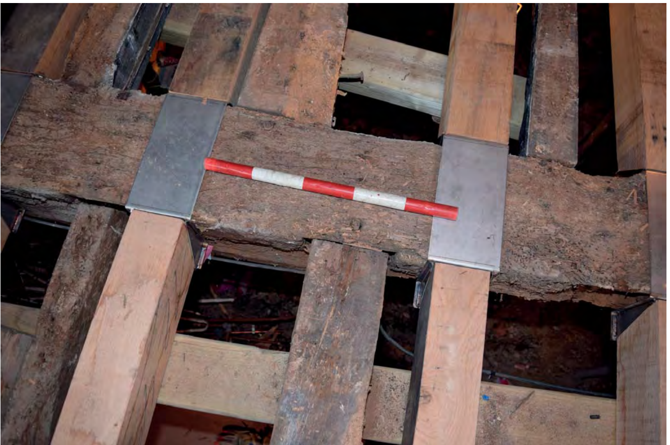
Plate 24: Bridging beam between Areas K & J looking south
