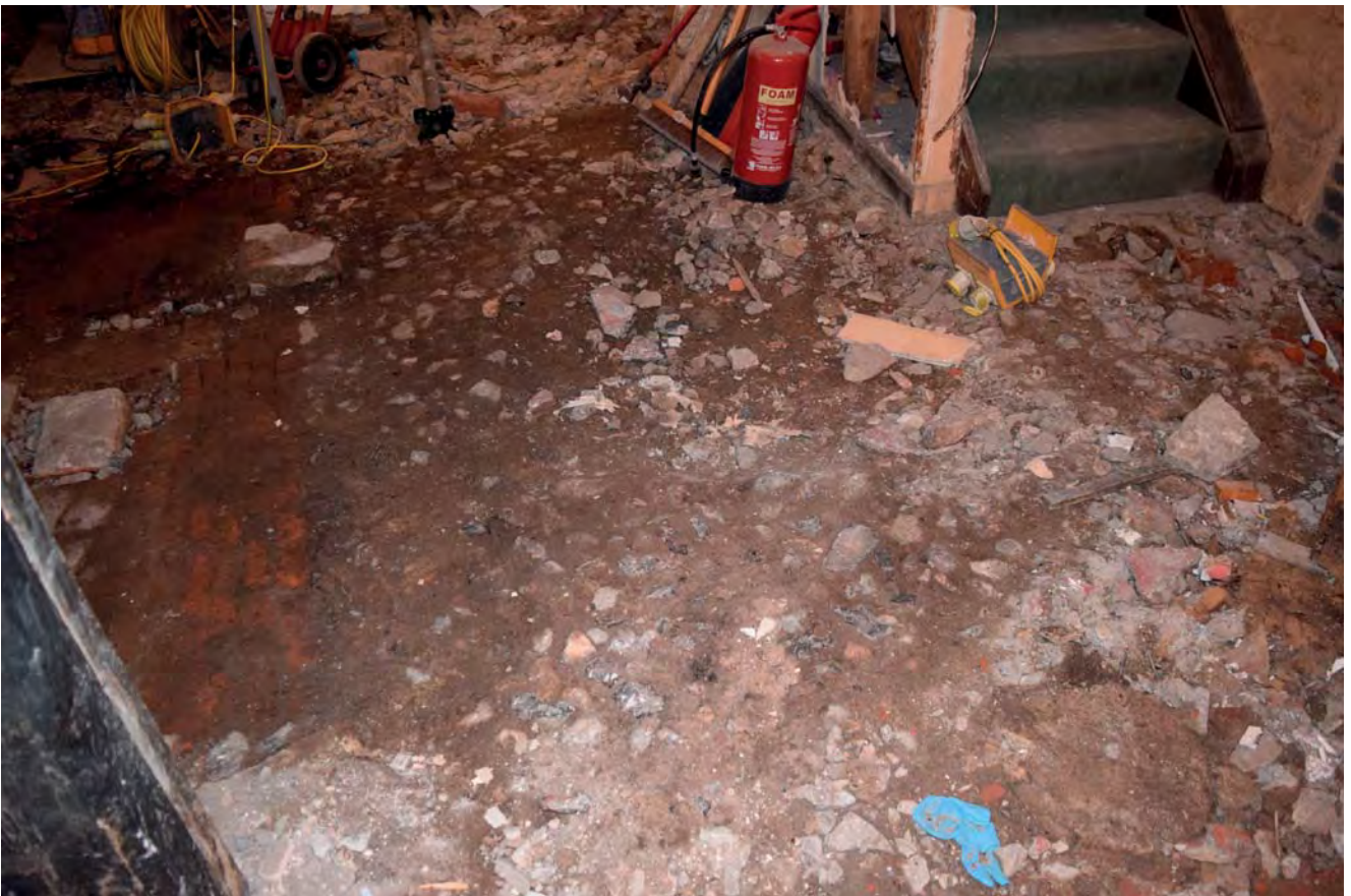
Plate 34: Flint in floor of basement
