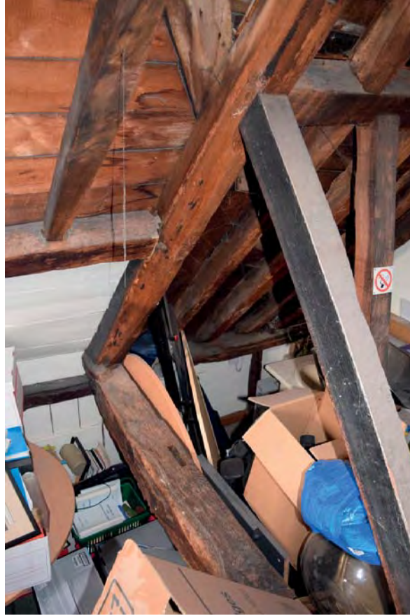
Plate 59: South end of Truss 6 at east end of building
