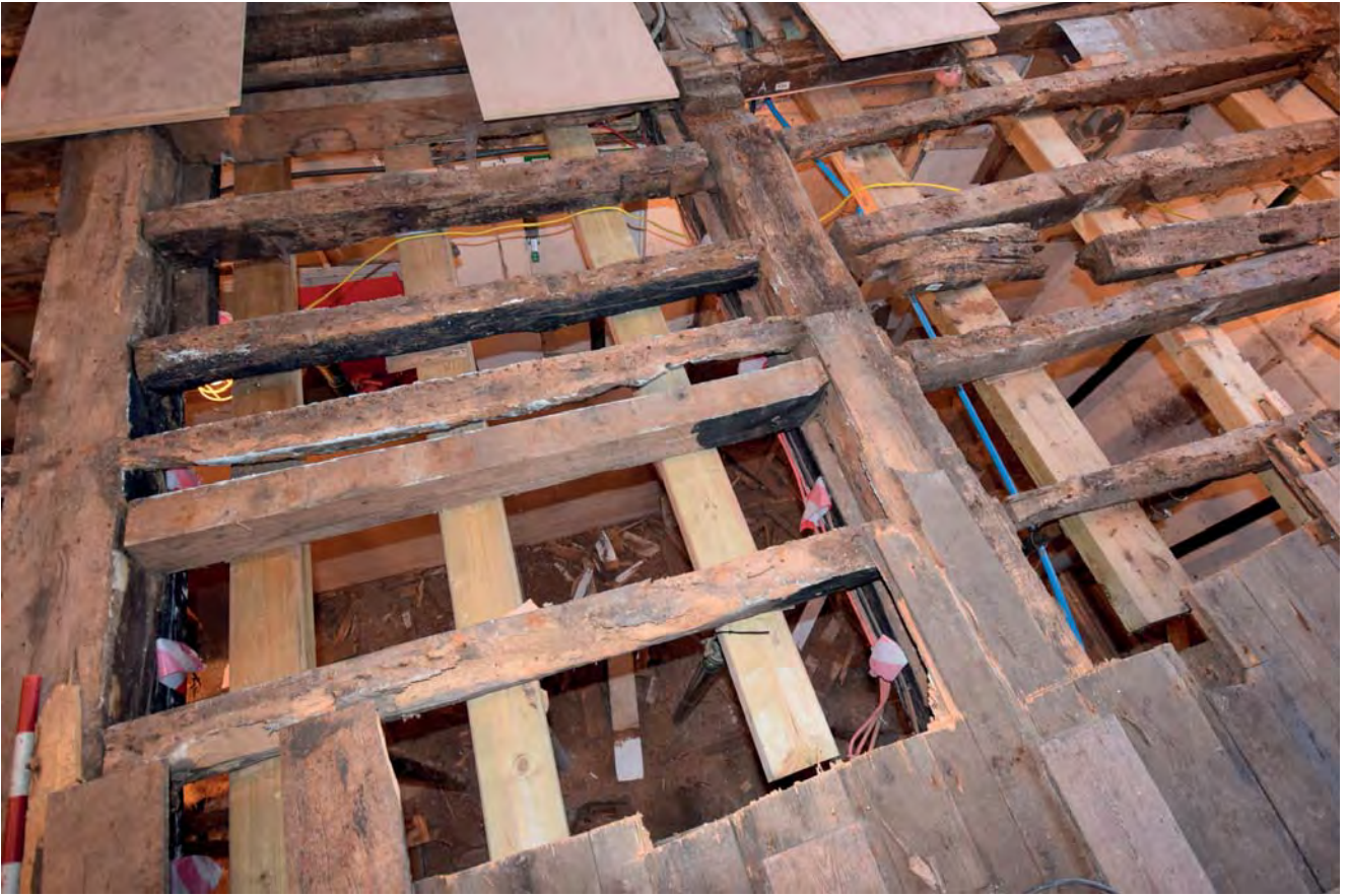
Plate 5: Joists at west end of floor looking west
