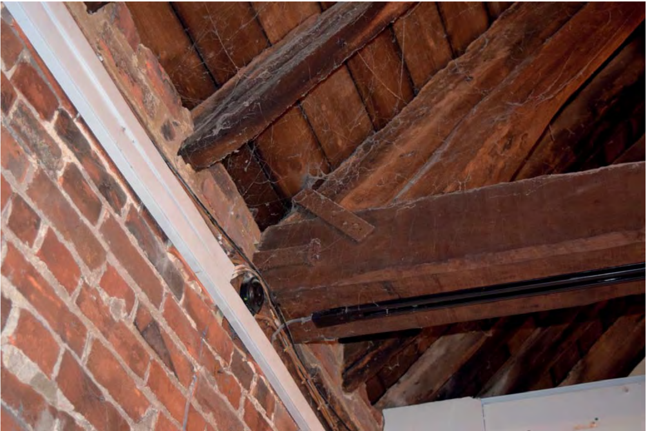
Plate 56: Detail of end of Truss 5
