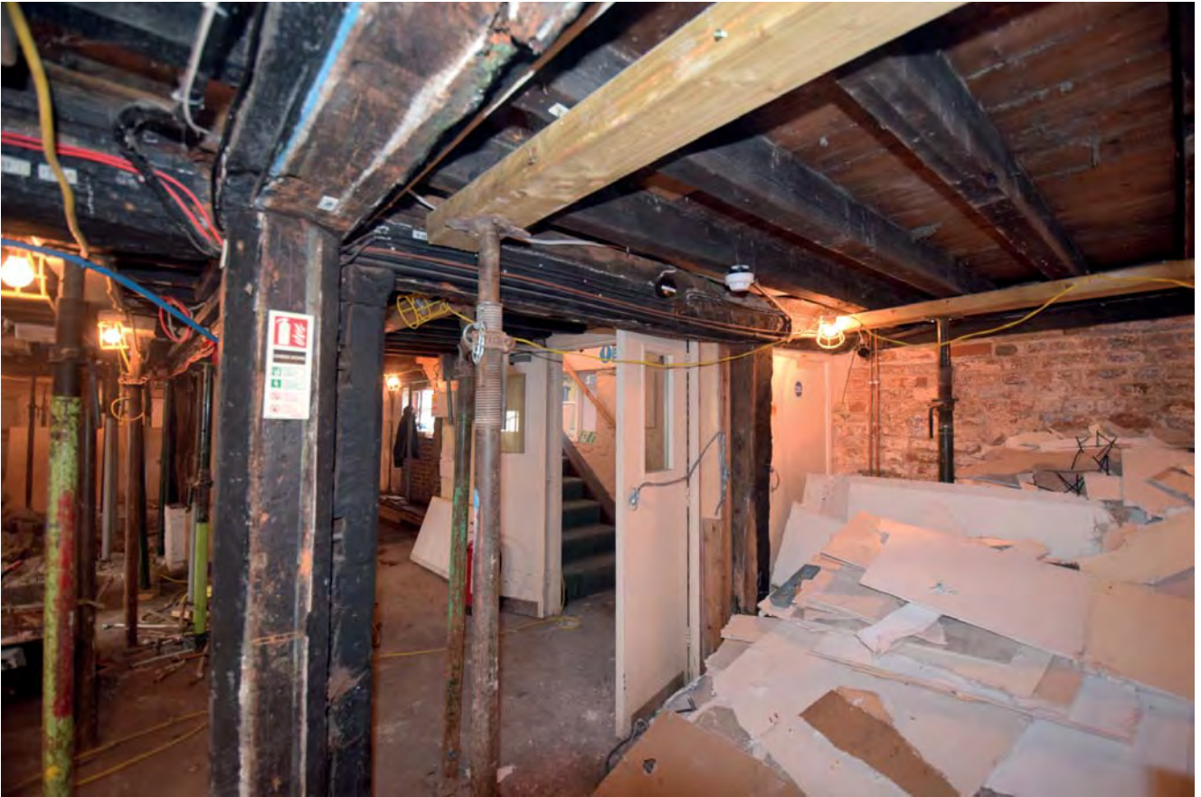
Plate 7: Basement view towards stairs
