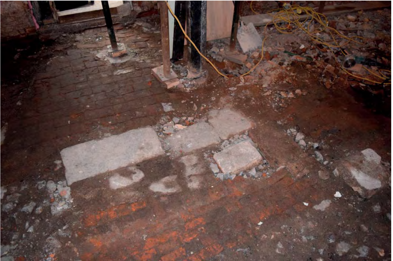
Plate 35: Features in basement floor looking south
