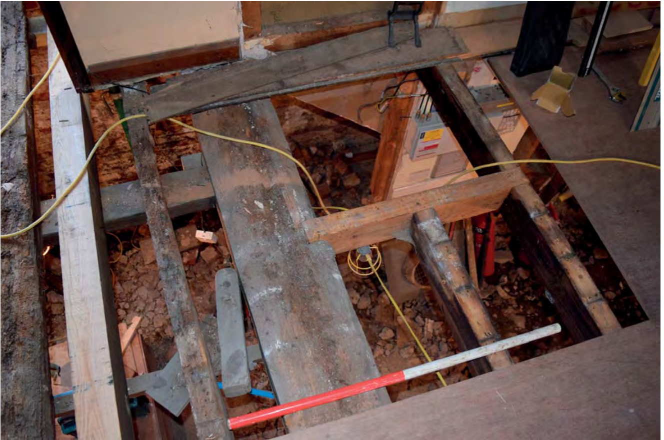
Plate 27: Hatch in Area H looking north
