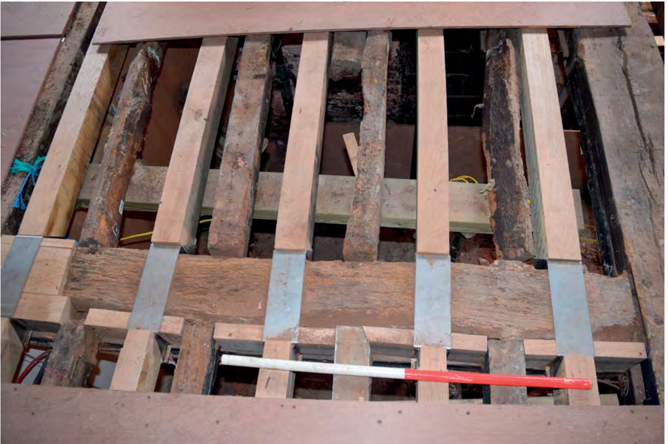
Plate 18: Joists in Area N during works looking north
