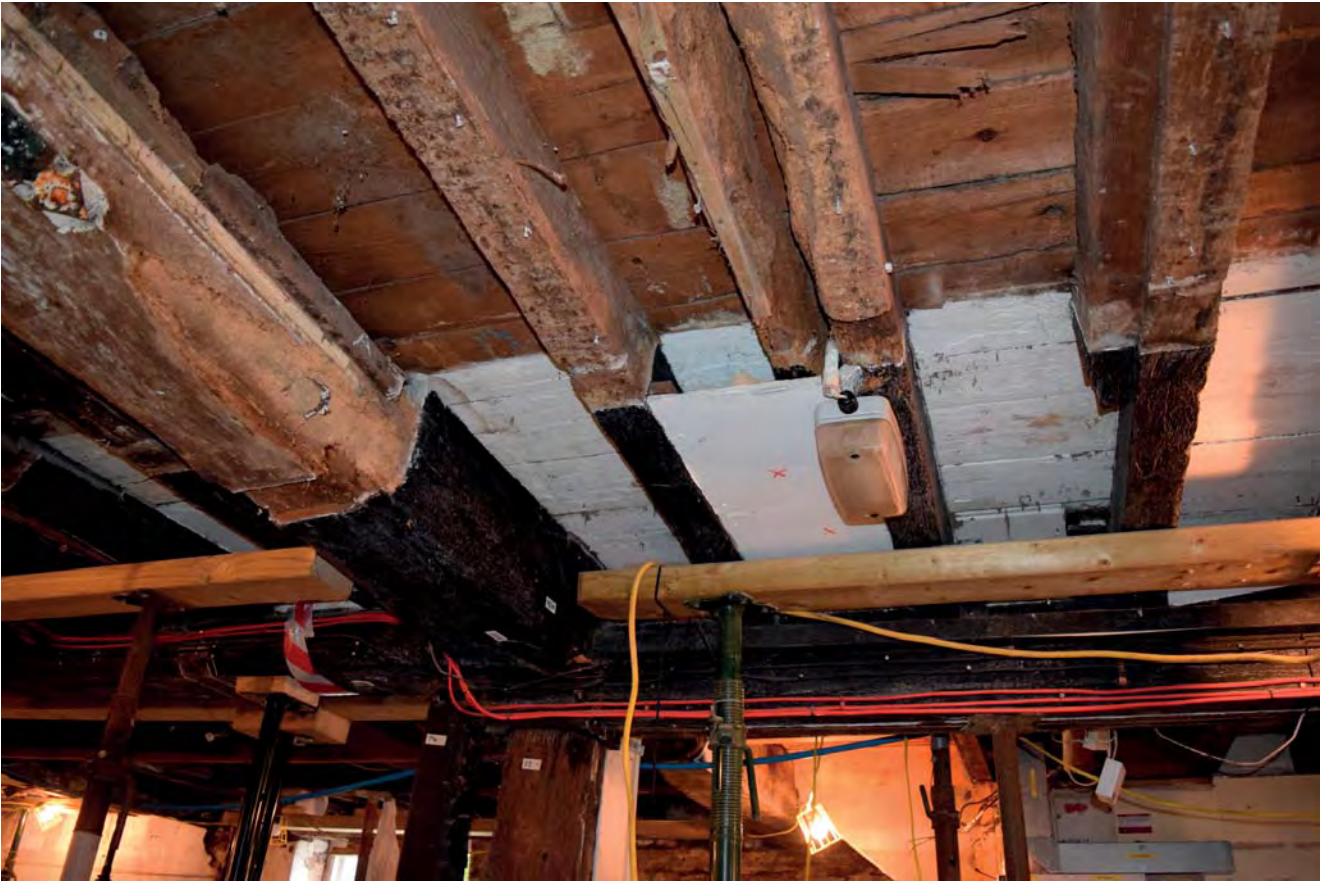
Plate 11: Joists in Area G looking north
