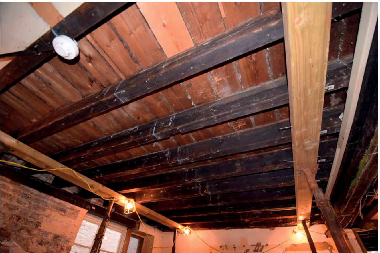
Plate 16: Joists in Area D looking north-east
