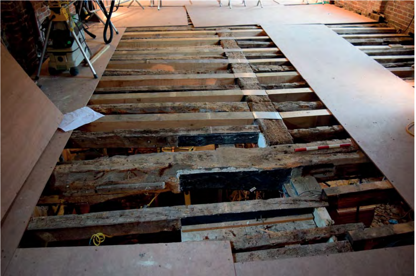
Plate 21: Joists in Area J&K looking west
